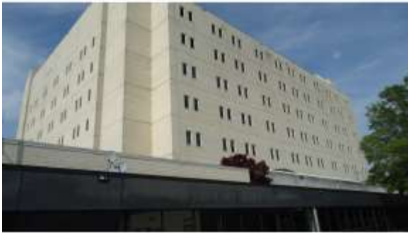
BROD071a 4/19/2016 Exterior brick masonry and original aluminum-framed windows Exterior
