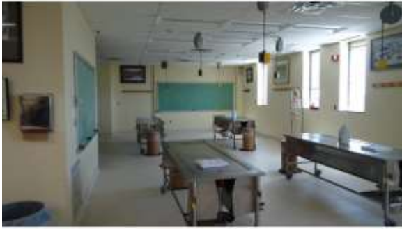
BROD022a 4/19/2016 Sheet vinyl flooring with painted walls and suspended grid ceilings Eight floor, teaching lab
