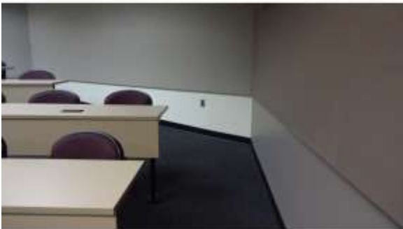
BROD053a 4/19/2016 Terraced classroom without adequate handrails Second floor
