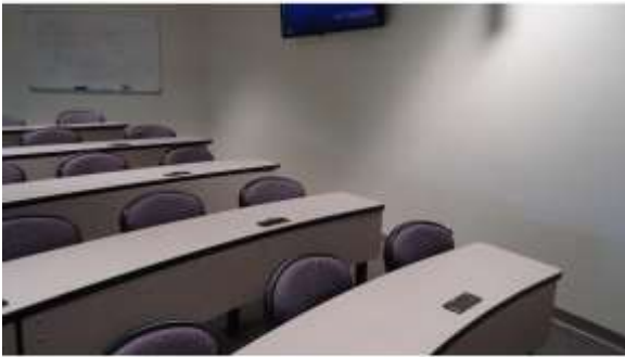
BROD050a 4/19/2016 Terraced classroom without adequate handrails Second floor
