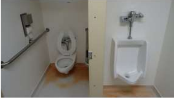
BROD031a 4/19/2016 Partially accessible toilet Seventh floor, men's restroom
