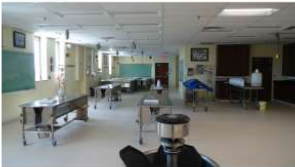
BROD023a 4/19/2016 Sheet vinyl flooring with painted walls and suspended grid ceilings Eight floor, teaching lab
