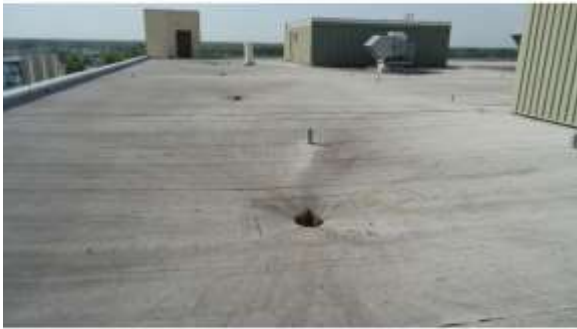
BROD005a 4/19/2016 Rolled asphalt built-up roof Roof
