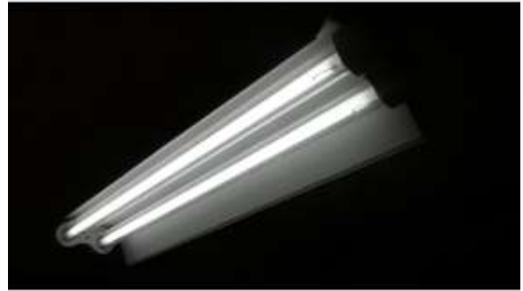
BROD040e 4/19/2016 Explosion proof lighting with T8 lamps Room 8S08D
