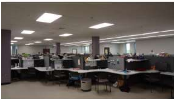
BROD048a 4/19/2016 Carpeted floors and suspended grid ceilings in open work area Second floor
