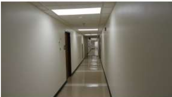
BROD045a 4/19/2016 Vinyl tile in corridors, with suspended grid ceilings and painted walls Third floor
