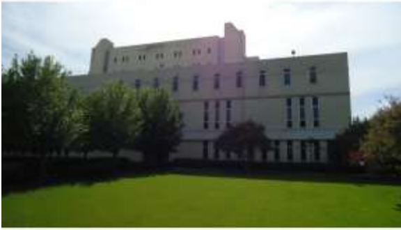
BROD076a 4/19/2016 Exterior brick masonry and original aluminum-framed windows Exterior
