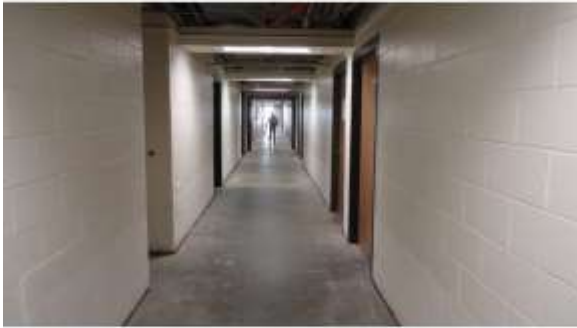
BROD073a 4/19/2016 Concrete floors and CMU walls and ceilings under renovation Basement
