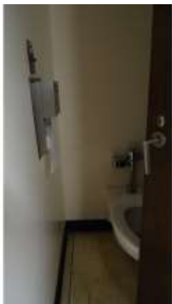
BROD039a 4/19/2016 Vinyl tiled floor with painted walls and inaccessible fixtures Small private restroom
