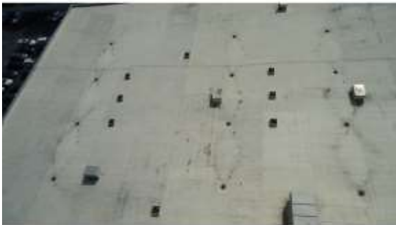
BROD006a 4/19/2016 Rolled asphalt built-up roof Lower roof
