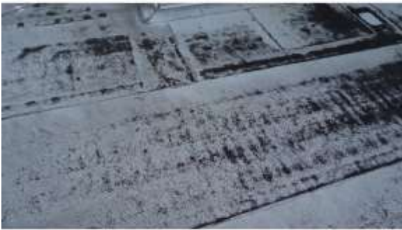
BROD003a 4/19/2016 Rolled asphalt built-up roof Roof
