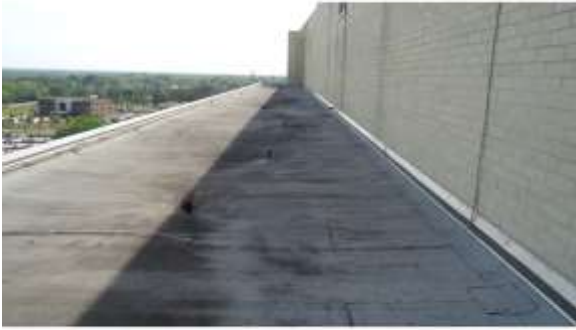
BROD001a 4/19/2016 Rolled asphalt built-up roof Roof
