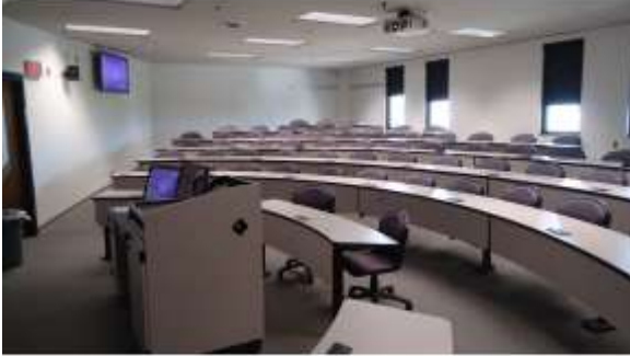
BROD049a 4/19/2016 Terraced classroom without adequate handrails Second floor
