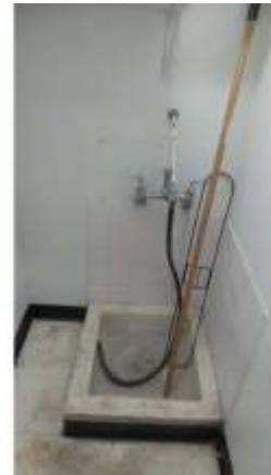
BROD053e 4/19/2016 Original service sink Room 8S04
