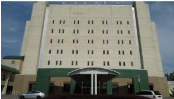
BROD069a 4/19/2016 Exterior brick masonry and original aluminum-framed windows Exterior
