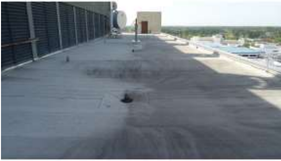
BROD002a 4/19/2016 Rolled asphalt built-up roof Roof
