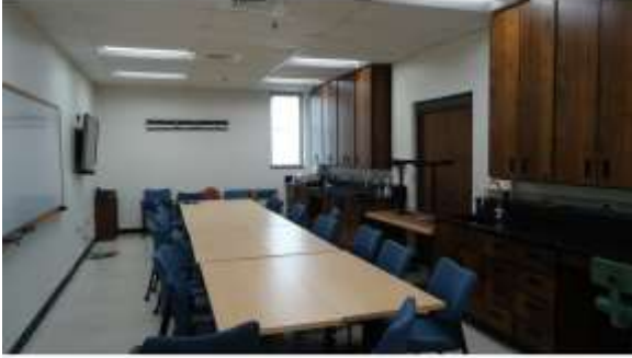
BROD037a 4/19/2016 Wooden cabinetry and vinyl tiled floors and suspended ceilings Sixth floor, teaching lab
