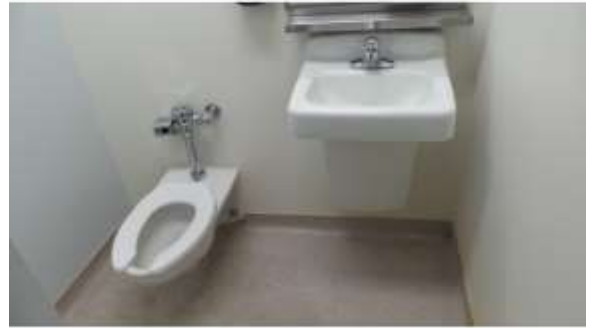
BROD052e 4/19/2016 Original plumbing fixtures Room 8S06
