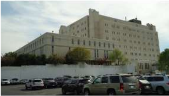
BROD077a 4/19/2016 Exterior brick masonry and original aluminum-framed windows Exterior
