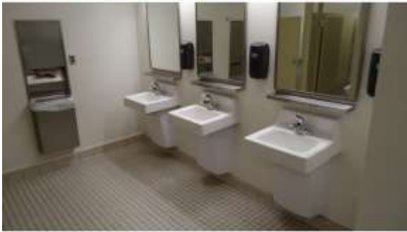
BROD056a 4/19/2016 Ceramic tiled floor and accessible fixtures Second floor
