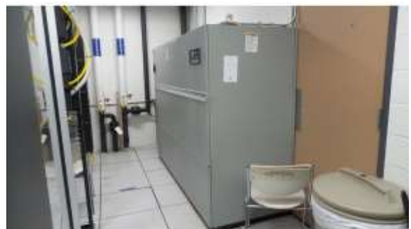
BROD083e 4/19/2016 Computer room air conditioner Ground floor, old data room
