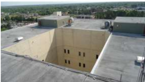
BROD012a 4/19/2016 Brick masonry exterior veneer finish Roof
