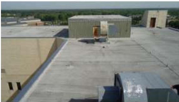
BROD009a 4/19/2016 Rolled asphalt built-up roof Roof
