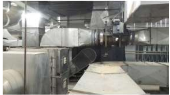
BROD029e 4/19/2016 Biosafety filters and inline fan Room 8N08
