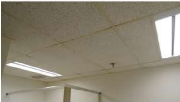
BROD057a 4/19/2016 Aged suspended grid ceiling system Second floor
