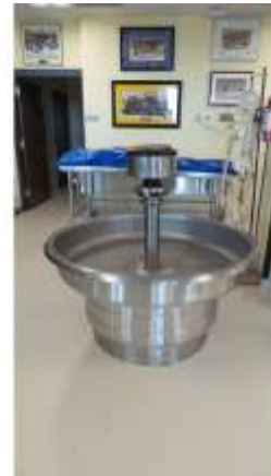
BROD055e 4/19/2016 Hand wash basin Room 8E18
