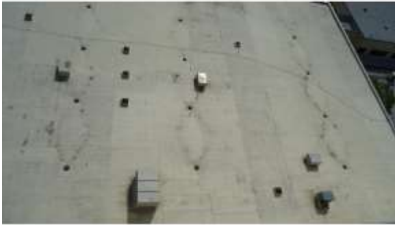
BROD007a 4/19/2016 Rolled asphalt built-up roof Lower roof
