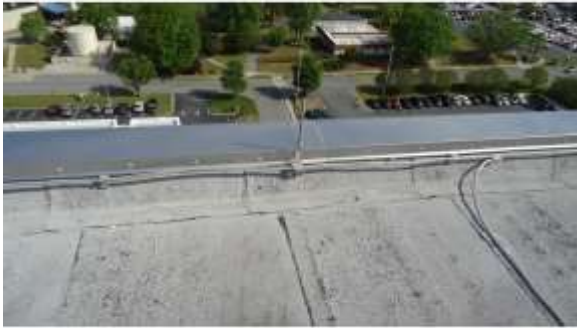
BROD004a 4/19/2016 Parapet wall flashing and lightning protection Roof
