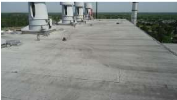
BROD011a 4/19/2016 Rolled asphalt built-up roof Roof
