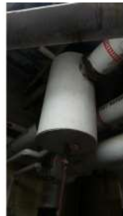
BROD078e 4/19/2016 Air separator Room GW58
