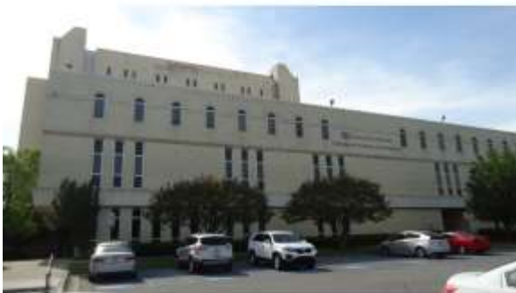
BROD075a 4/19/2016 Exterior brick masonry and original aluminum-framed windows Exterior
