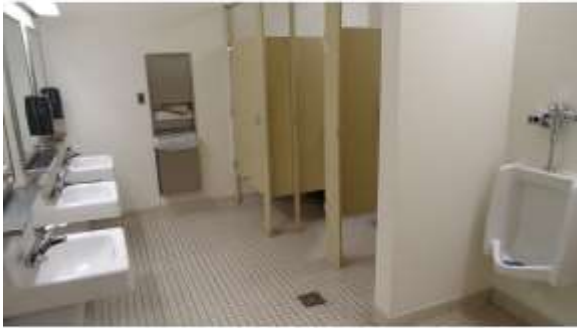
BROD055a 4/19/2016 Ceramic tiled floor and accessible fixtures Second floor
