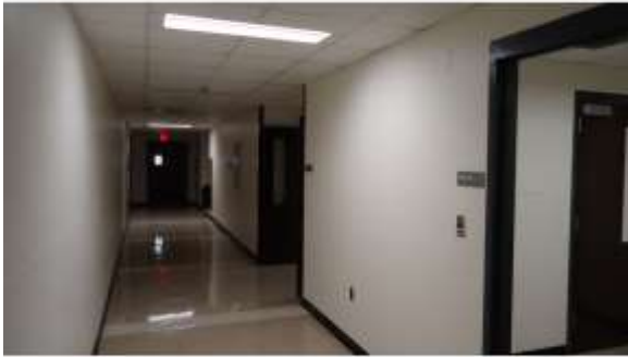
BROD016a 4/19/2016 Vinyl tile floor in corridors, with suspended grid ceilings and painted walls Eighth floor
