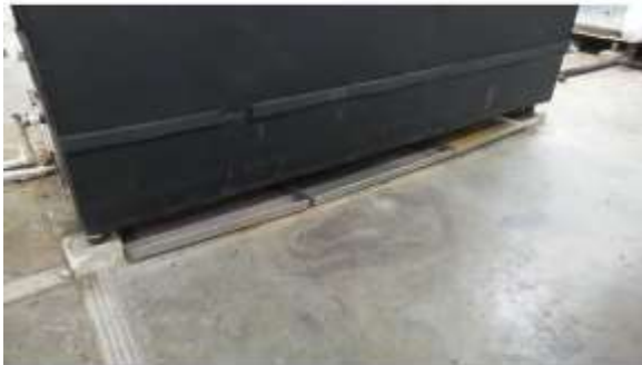
BROD088e 4/19/2016 After-market drip pan retrofit Room 3E144
