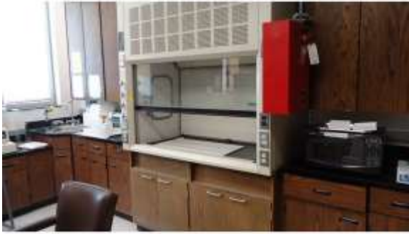
BROD028a 4/19/2016 Original fume hood Seventh floor, teaching lab
