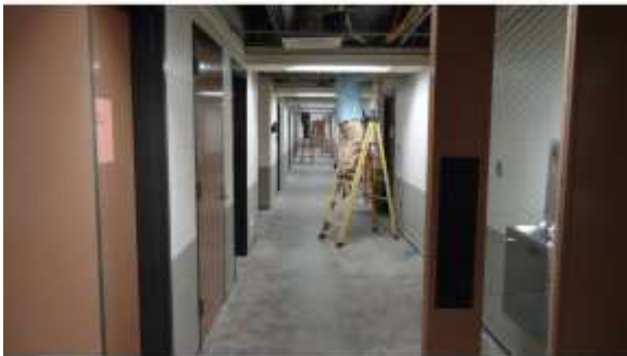
BROD074a 4/19/2016 Concrete floors and CMU walls and ceilings under renovation Basement
