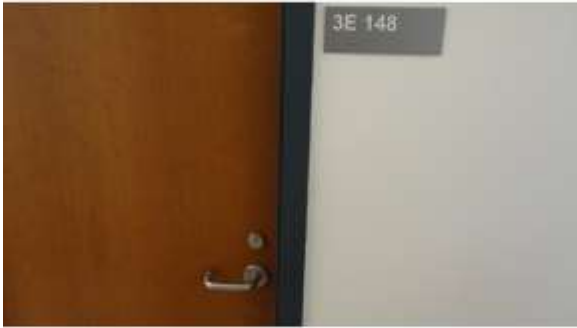
BROD046a 4/19/2016 Lever actuated door hardware and accessible signage Third floor
