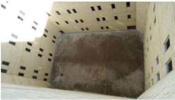
BROD008a 4/19/2016 Rolled asphalt built-up roof Lower center roof
