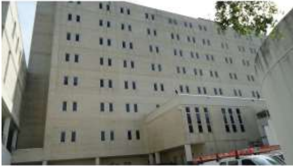
BROD079a 4/19/2016 Exterior brick masonry and original aluminum-framed windows Exterior
