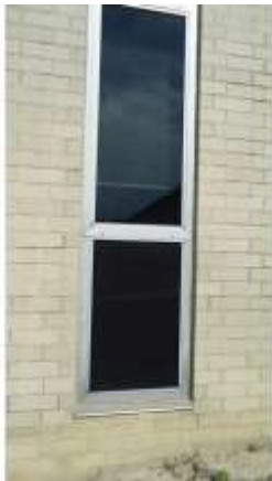
BROD065a 4/19/2016 Original aluminum-framed windows Exterior
