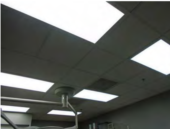
CARD027a 11/6/2018 Suspended grid ceiling Fourth floor exam room
