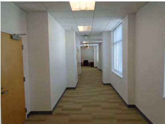
CARD009a 11/6/2018 Carpeting, painted walls, and suspended grid ceiling Fourth floor corridor
