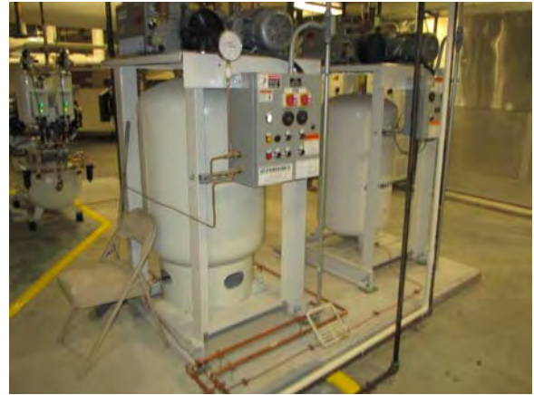
CARD034e 11/6/2018 Powerex vacuum systems VP1 and VP2 East mezzanine
