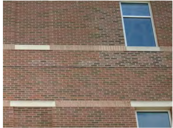
CARD173a 11/6/2018 Previous brick masonry repairs Northwest exterior
