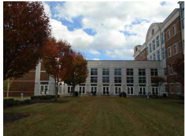
CARD169a 11/6/2018 Concrete exterior panels, dual-pane windows, and glass doors Northeast courtyard
