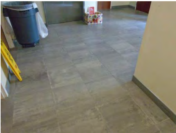
CARD110a 11/6/2018 Tiled floor First floor elevator lobby
