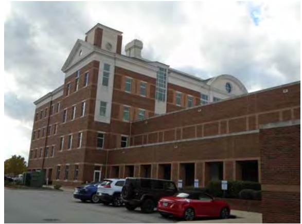
CARD185a 11/6/2018 Brick masonry exterior, dual-pane windows, and metal standing seam roof Southeast exterior
