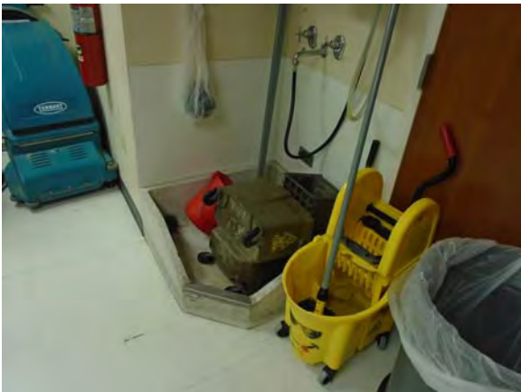
CARD146a 11/6/2018 Custodial floor sink First floor
