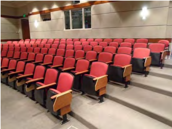
CARD148a 11/6/2018 Carpeting and wall-mounted sound dampening panels Auditorium 1430
