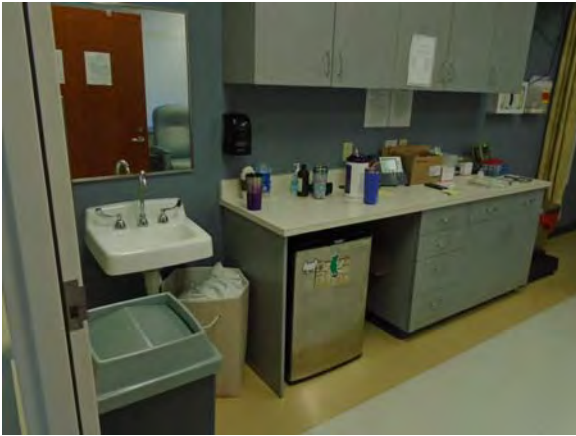
CARD100a 11/6/2018 Vinyl tile floor, painted walls, suspended ceiling, base and overhead cabinetry, and wall-mounted sink Second floor exam room
