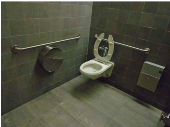
CARD158a 11/6/2018 Tiled floor and walls and accessible water closet Auditorium restroom
