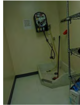
CARD107a 11/6/2018 Vinyl tile floor and custodial floor sink First floor
