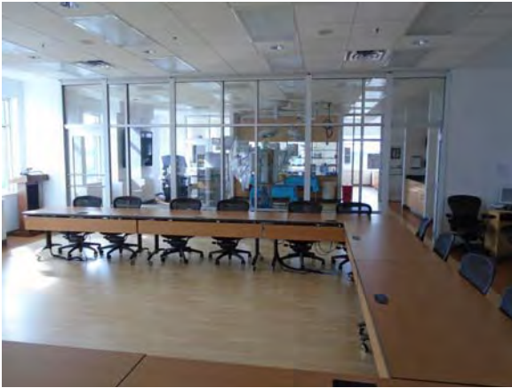
CARD014a 11/6/2018 Wood laminate flooring, suspended ceiling, and glazed interior wall partitions Fourth floor
