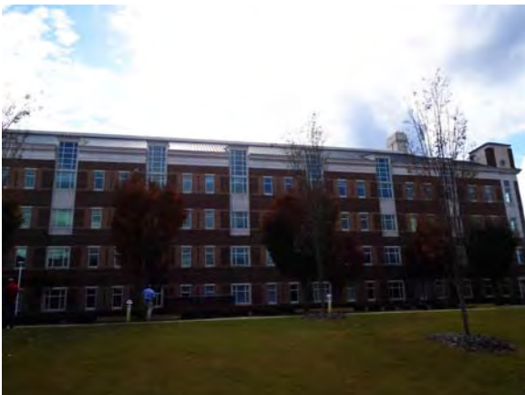
CARD164a 11/6/2018 Brick masonry exterior, dual-pane windows, and metal standing seam roof East exterior
