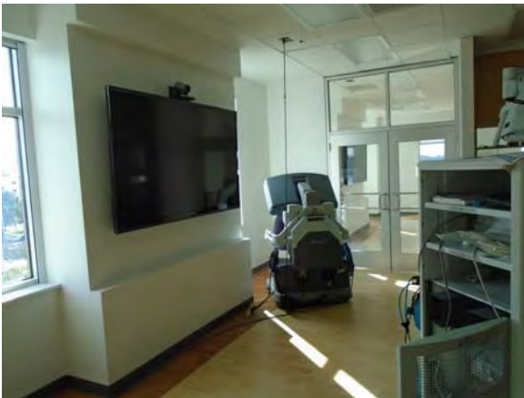
CARD015a 11/6/2018 Wood laminate flooring, suspended ceiling, and glazed interior doors Fourth floor
