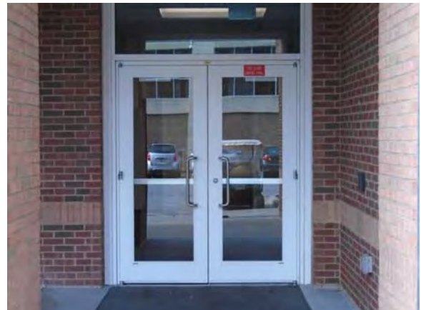
CARD181a 11/6/2018 Aluminum and glass exterior doors Southeast exterior
