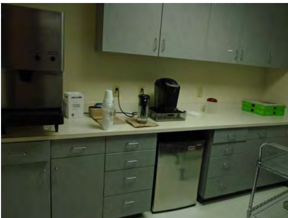
CARD102a 11/6/2018 Vinyl tile floor, painted walls, suspended ceiling, and base and overhead cabinetry Second floor
