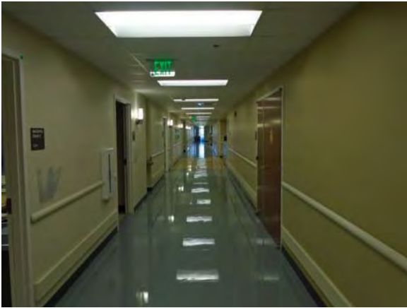
CARD130a 11/6/2018 Vinyl flooring, painted walls, and suspended grid ceiling First floor
