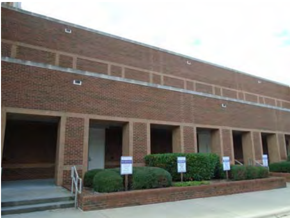
CARD182a 11/6/2018 Brick masonry exterior Southeast exterior
