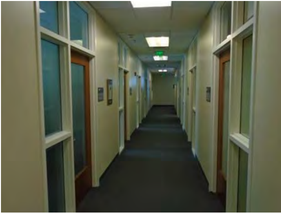
CARD061a 11/6/2018 Carpeting, glazed interior walls, and suspended grid ceiling Fourth floor corridor
