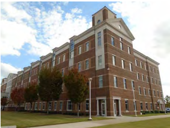
CARD170a 11/6/2018 Brick masonry exterior, dual-pane windows, and metal standing seam roof Northwest corner
