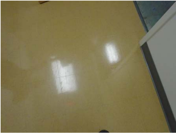
CARD010a 11/6/2018 Vinyl tile floor Fourth floor corridor
