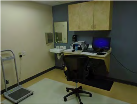
CARD101a 11/6/2018 Vinyl tile floor, painted walls, suspended ceiling, base and overhead cabinetry, and wall-mounted sink Second floor exam room
