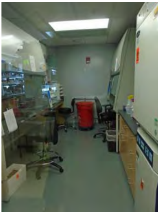
CARD042a 11/6/2018 Sheet vinyl flooring, painted walls, suspended grid ceiling, and wood and metal lab cabinetry Fourth floor
