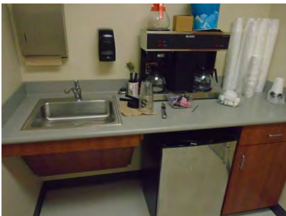
CARD075a 11/6/2018 Accessible sink Third floor
