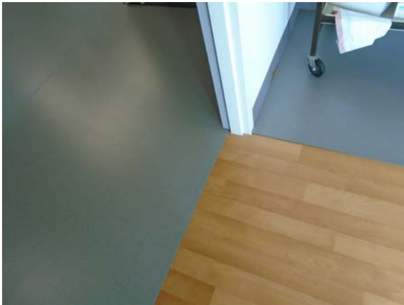
CARD020a 11/6/2018 Transition between laminate and sheet vinyl flooring Fourth floor
