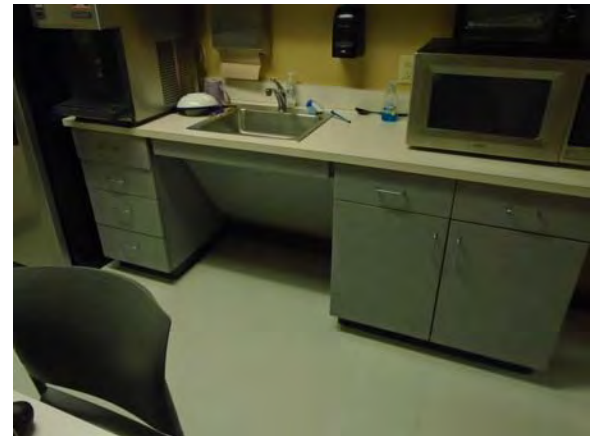
CARD111a 11/6/2018 Vinyl tile floor and accessible sink and cabinetry First floor
