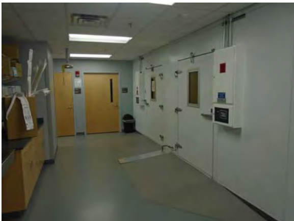
CARD021a 11/6/2018 Sheet vinyl flooring and suspended ceiling Fourth floor
