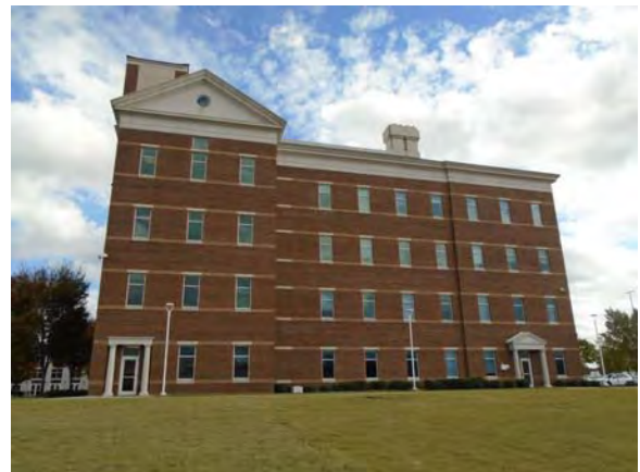
CARD171a 11/6/2018 Concrete exterior panels, dual-pane windows, and glass doors Northwest exterior
