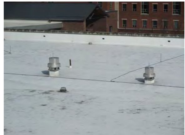
CARD039e 11/6/2018 Two centrifugal roof exhausters North roof
