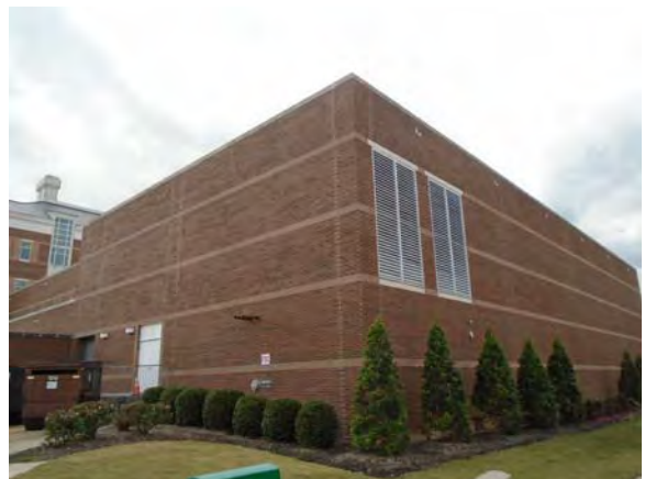
CARD187a 11/6/2018 Brick masonry exterior Southeast corner
