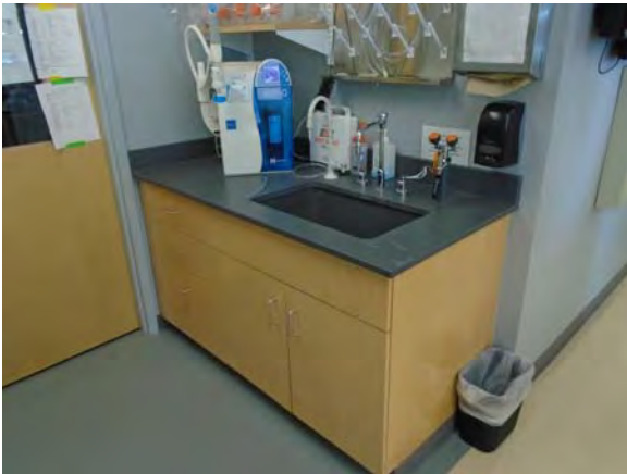
CARD044a 11/6/2018 Built-in wood lab cabinetry with sink Fourth floor
