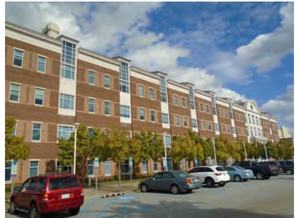
CARD175a 11/6/2018 Brick masonry exterior, dual-pane windows, and glass doors Southwest exterior
