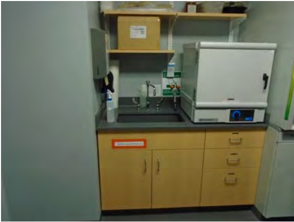
CARD043a 11/6/2018 Built-in wood lab cabinetry with sink Fourth floor
