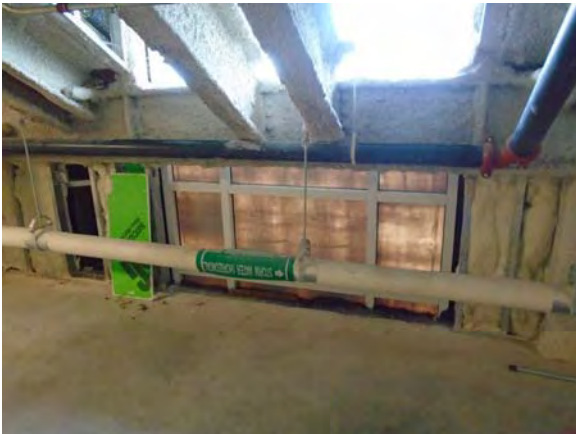
CARD002a 11/6/2018 Wall insulation and sprayed-on fireproofing Penthouse
