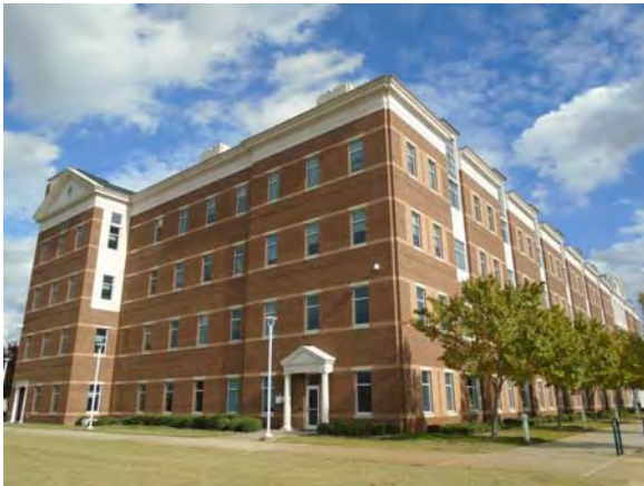
CARD174a 11/6/2018 Brick masonry exterior, dual-pane windows, and glass doors West corner
