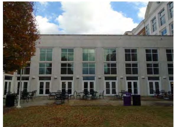
CARD165a 11/6/2018 Concrete exterior panels, dual-pane windows, and doors Northeast courtyard
