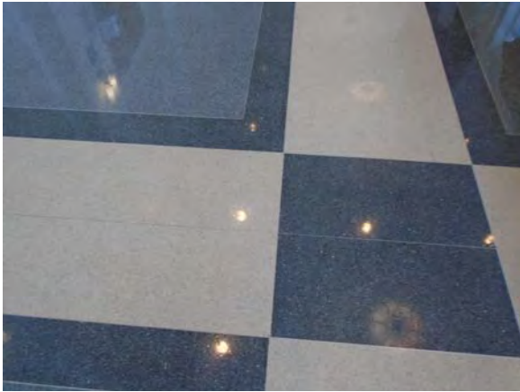
CARD154a 11/6/2018 Terrazzo flooring Prefunction space 1408
