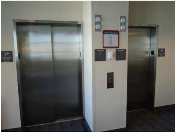
CARD073a 11/6/2018 Elevator lobby with accessible call buttons and signage Third floor
