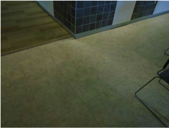
CARD052a 11/6/2018 Ceramic tile floor and painted and tiled walls Fourth floor break room
