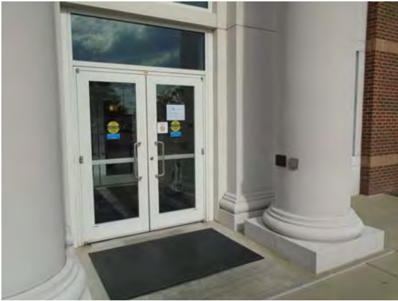
CARD178a 11/6/2018 Aluminum and glass exterior doors Main southwest entrance
