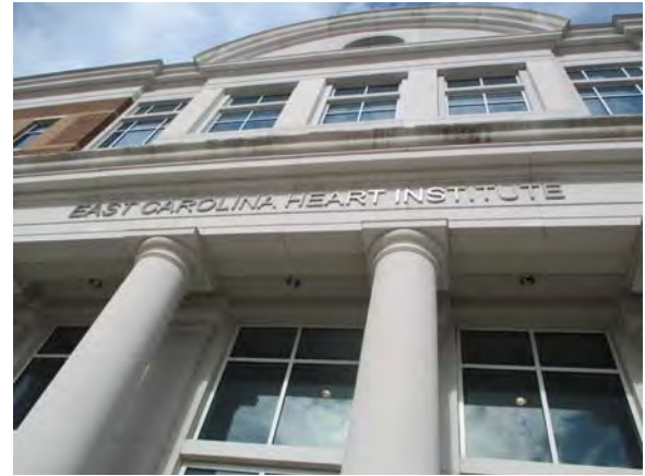
CARD101e 11/6/2018 Ceiling recessed CFL exterior lights South exterior
