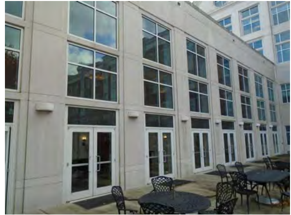
CARD167a 11/6/2018 Concrete exterior panels, dual-pane windows, and glass doors Northeast courtyard
