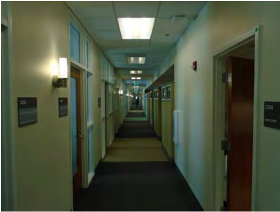
CARD088a 11/6/2018 Carpeting, painted walls, and suspended grid ceiling Second floor corridor
