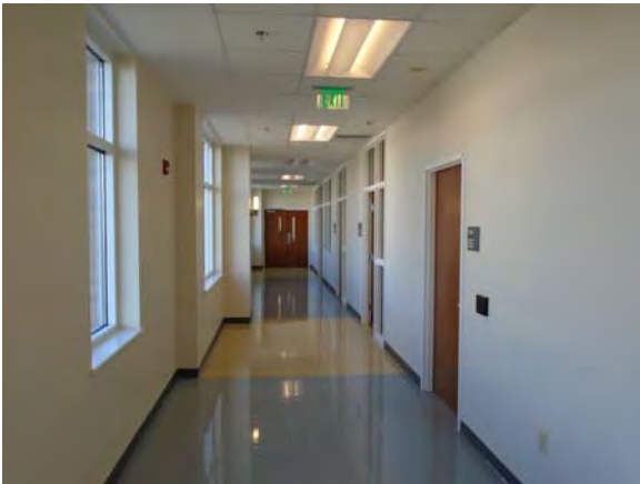
CARD071a 11/6/2018 Vinyl flooring, painted walls, and suspended grid ceiling Third floor outer corridor
