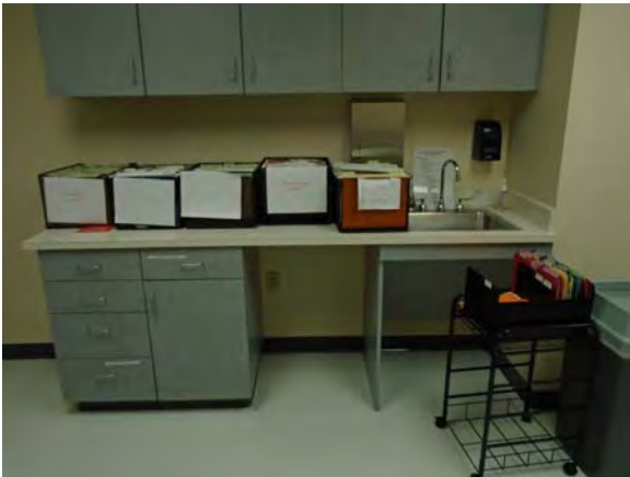
CARD098a 11/6/2018 Vinyl tile floor, painted walls, suspended ceiling, and base and overhead cabinetry with sink Second floor
