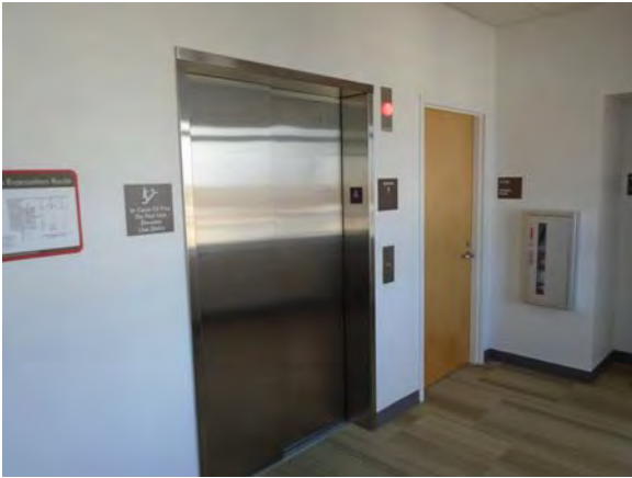
CARD056a 11/6/2018 Carpeting, lever hardware, and accessible signage Fourth floor
