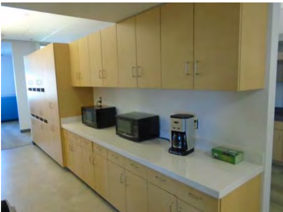
CARD054a 11/6/2018 Ceramic tile floor, painted walls, and wood cabinetry Fourth floor
