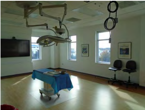
CARD017a 11/6/2018 Wood laminate flooring, suspended ceiling, and painted walls Fourth floor
