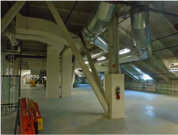
CARD004a 11/6/2018 Original sealed concrete slab floor Penthouse
