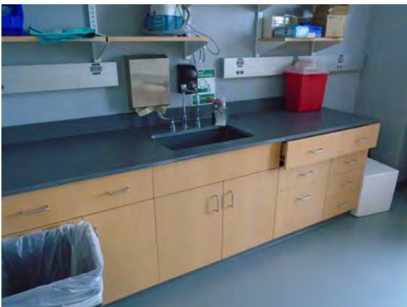
CARD024a 11/6/2018 Built-in wood lab cabinetry with sink Fourth floor
