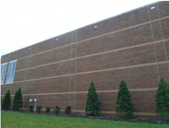
CARD162a 11/6/2018 Brick masonry exterior Northeast exterior
