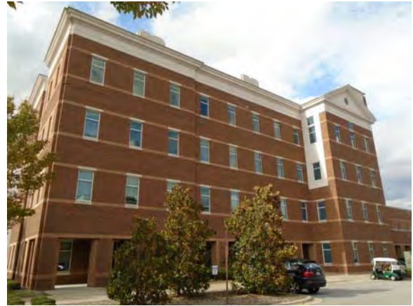
CARD179a 11/6/2018 Brick masonry exterior, dual-pane windows, and metal standing seam roof Southeast exterior
