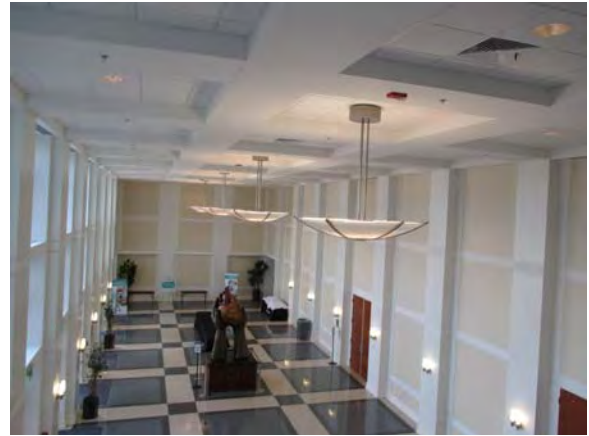
CARD068e 11/6/2018 Decorative pendant and wall sconce light fixtures Entrance lobby for auditorium
