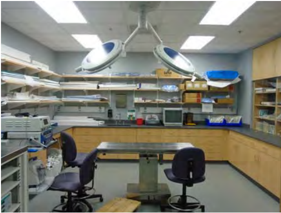
CARD025a 11/6/2018 Sheet vinyl flooring, painted walls, suspended grid ceiling, and wood cabinetry Fourth floor exam room
