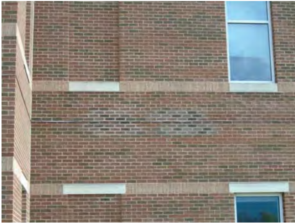
CARD172a 11/6/2018 Previous brick masonry repairs Northwest exterior
