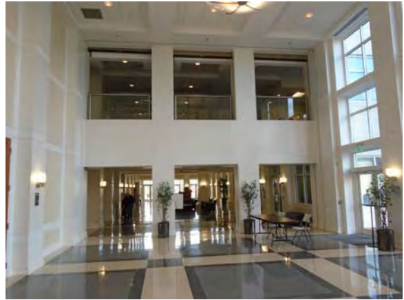
CARD155a 11/6/2018 Terrazzo flooring and painted walls Prefunction space 1408
