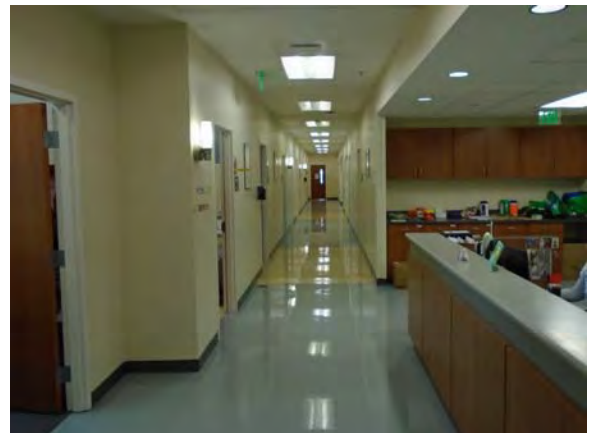
CARD117a 11/6/2018 Vinyl flooring, painted walls, and suspended grid ceiling First floor
