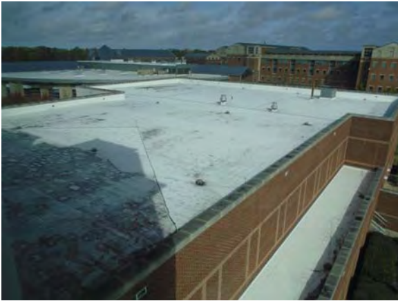
CARD007a 11/6/2018 Original membrane roof Lower northeast wing roof
