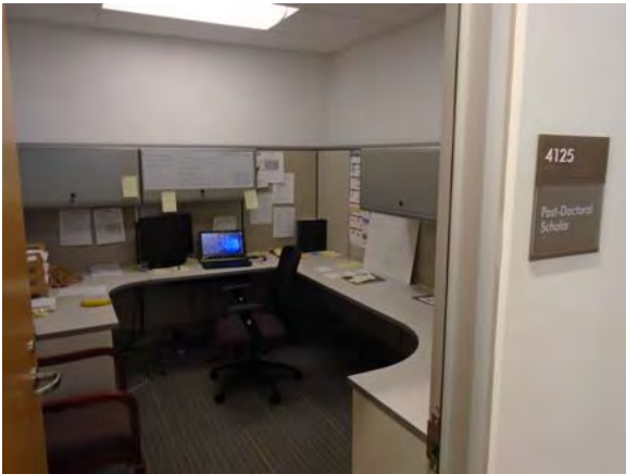
CARD059a 11/6/2018 Carpeting, painted walls, and suspended grid ceiling Fourth floor office
