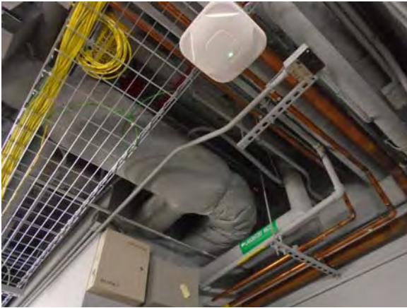
CARD034a 11/6/2018 Exposed ceiling areas for utility access Fourth floor
