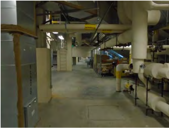
CARD001a 11/6/2018 Original sealed concrete slab floor Penthouse
