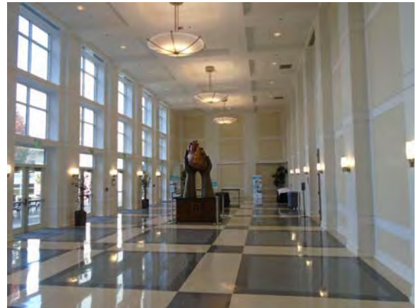
CARD139a 11/6/2018 Terrazzo flooring and painted walls Prefunction space 1408
