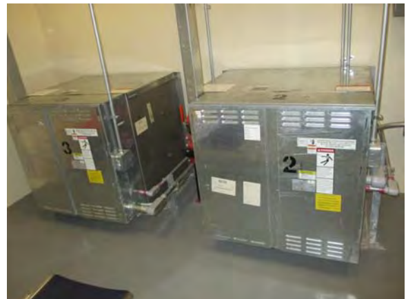
CARD033e 11/6/2018 50 hp and 40 hp Otis hydraulic pumps for elevators 2 and 3, respectively P104
