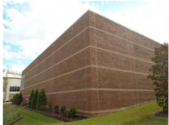
CARD163a 11/6/2018 Brick masonry exterior Northeast corner
