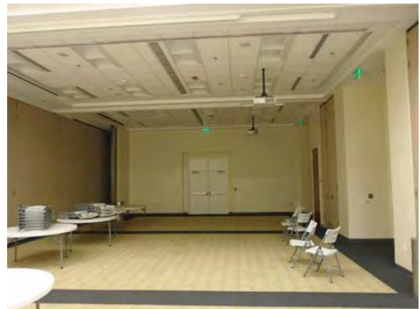
CARD141a 11/6/2018 Carpeting, painted walls, suspended grid ceiling, and room dividers Conference rooms 1410B, C, and D
