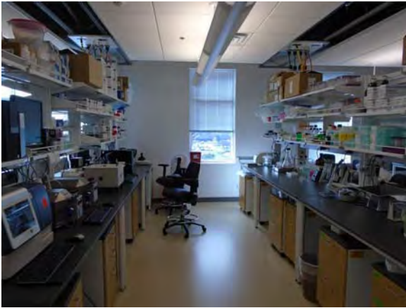
CARD040a 11/6/2018 Sheet vinyl flooring, painted walls, suspended grid ceiling, and wood and metal lab cabinetry Fourth floor lab
