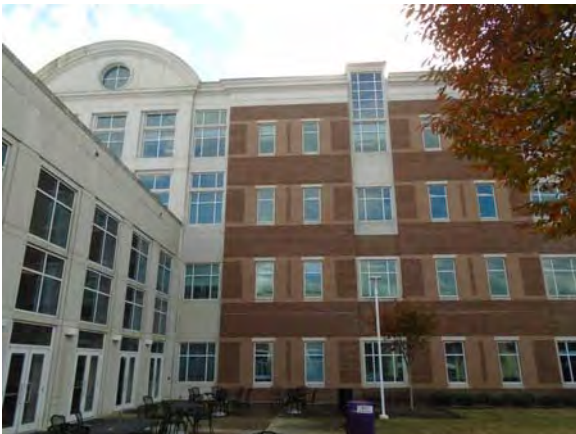
CARD168a 11/6/2018 Brick masonry and concrete panel exterior North exterior
