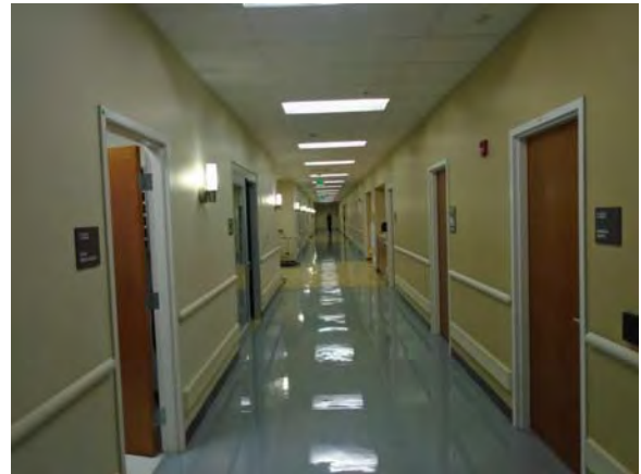
CARD127a 11/6/2018 Vinyl flooring, painted walls, and suspended grid ceiling First floor
