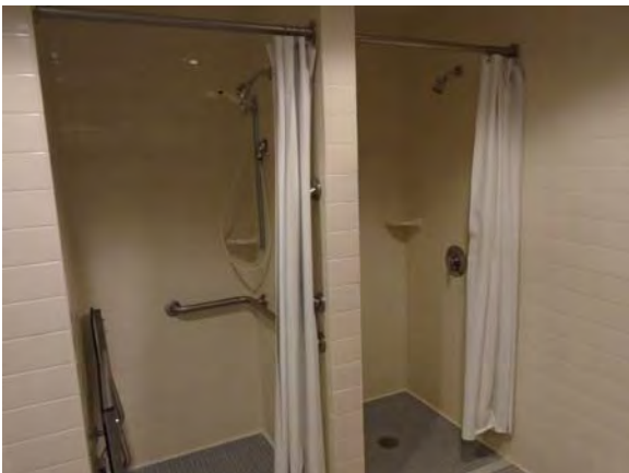
CARD081a 11/6/2018 Tiled floor and walls and accessible shower Third floor staff shower/restroom
