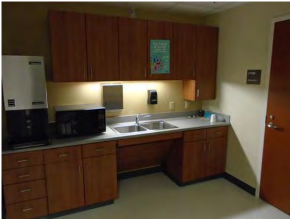
CARD074a 11/6/2018 Vinyl flooring, built-in wood cabinetry/sink, and suspended ceiling Third floor
