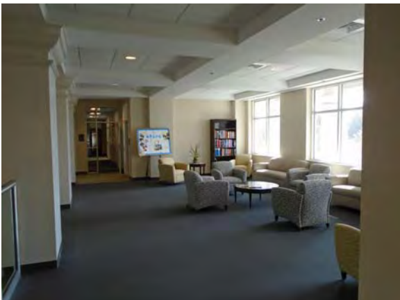
CARD087a 11/6/2018 Carpeting, painted walls, and suspended grid ceiling Second floor waiting area
