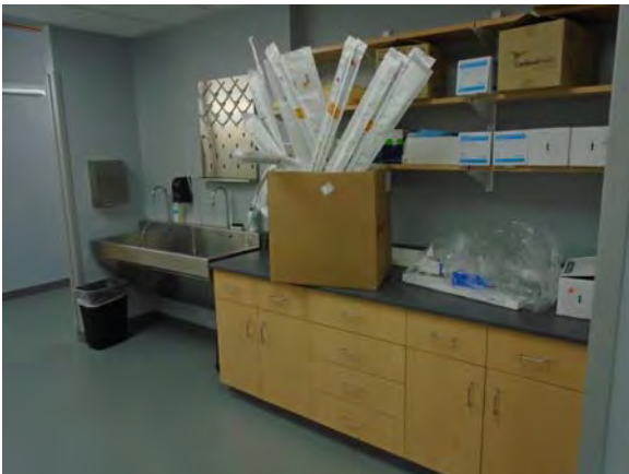
CARD029a 11/6/2018 Sheet vinyl flooring, painted walls, and stainless steel sink Fourth floor
