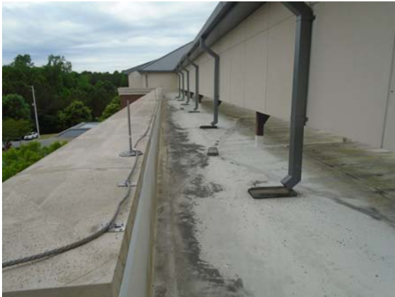
255010a 5/11/2021 Parapet wall and downspouts and drains Roof
