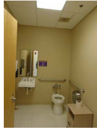
255095a 5/11/2021 Accessible fixtures and vinyl floor tile Single-user restroom
