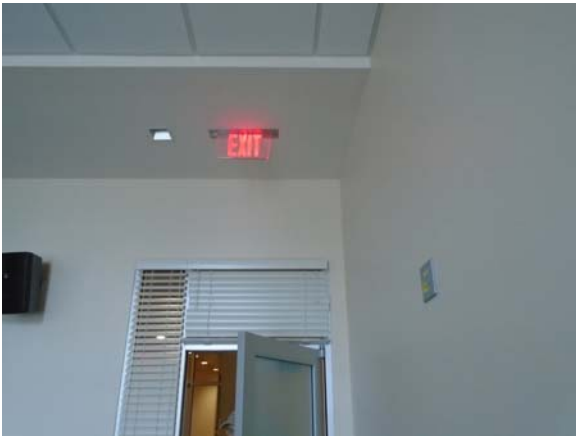
255044a 5/11/2021 Adequate exit signage Second floor classroom
