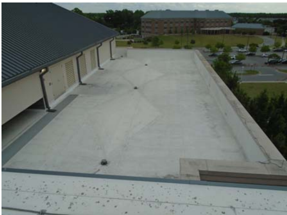
255003a 5/11/2021 Single-ply membrane roof Northeast roof
