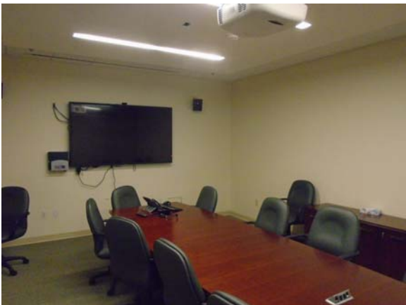
255042a 5/11/2021 Carpeting, painted walls, and suspended grid ceiling Conference room 2421C
