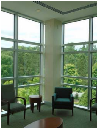
255051a 5/11/2021 Glazing at corner waiting areas Second floor
