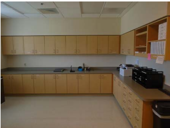
255033a 5/11/2021 Wood base and overhead cabinetry, vinyl floor tile Workroom 2408C
