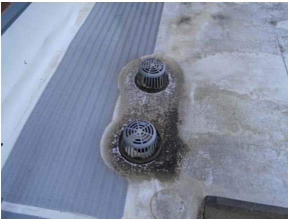
255006a 5/11/2021 Roof drains Roof
