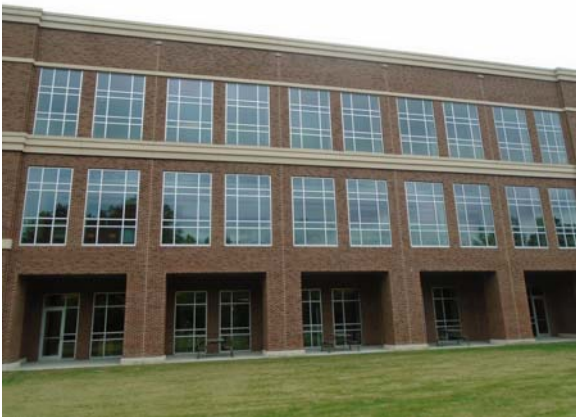
255126a 5/11/2021 Brick masonry, dual-pane windows, and EIFS accents West exterior
