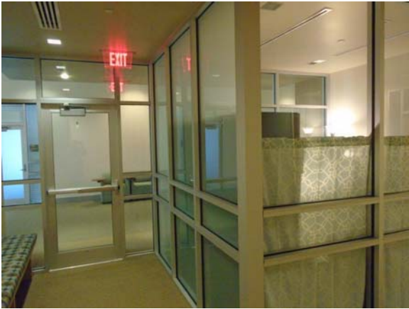
255040a 5/11/2021 Interior partition glazing Suite 2400
