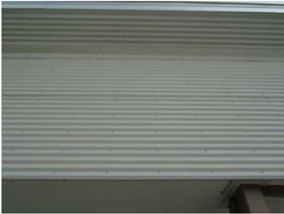
255007a 5/11/2021 Corrugated metal siding Mechanical penthouse
