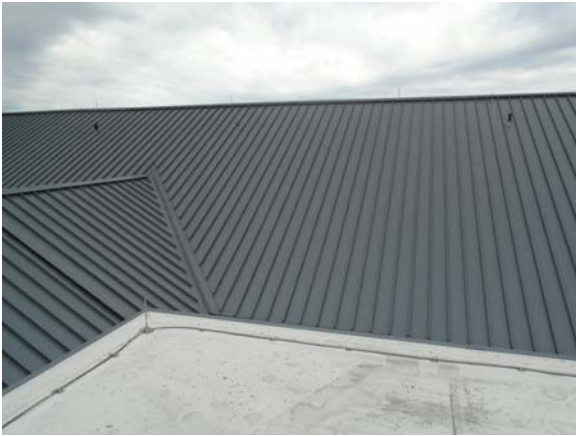
255004a 5/11/2021 Standing seam metal roof Pitched roof over mechanical penthouse
