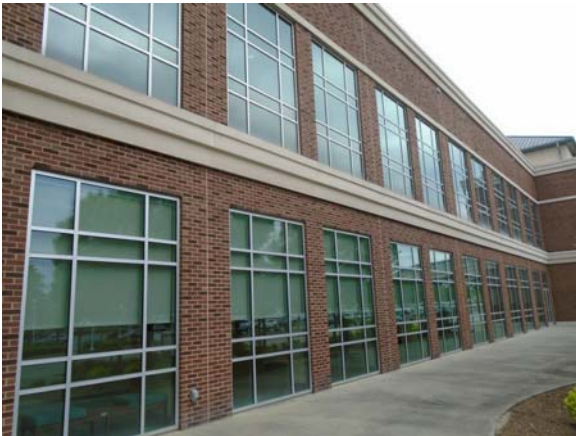
255132a 5/11/2021 Brick masonry, dual-pane windows, and EIFS accents South exterior
