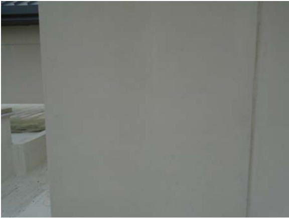
255013a 5/11/2021 Prefab exterior panels Mechanical penthouse
