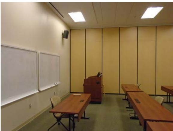
255030a 5/11/2021 Carpeting, painted and fabric walls, suspended grid ceiling, and accordion room divider Large meeting room 2610C
