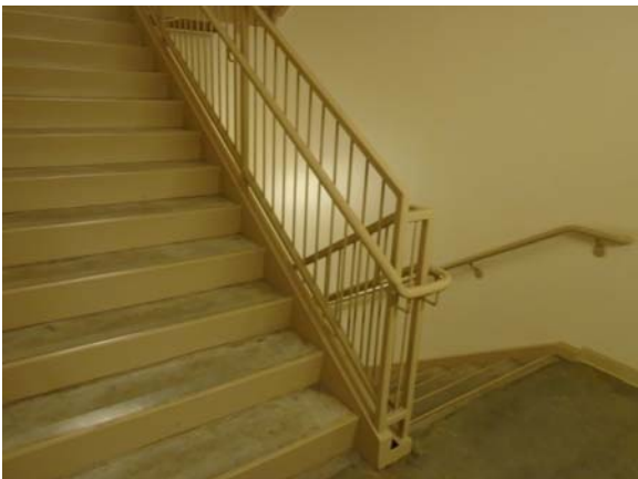
255024a 5/11/2021 Compliant stairwells with proper handrail Stairwell 3
