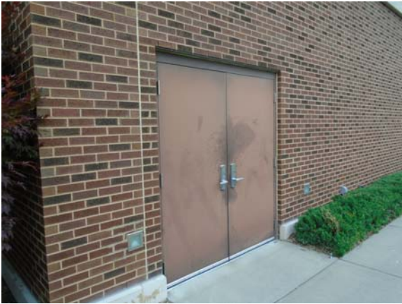
255136a 5/11/2021 Hollow metal service doors East exterior
