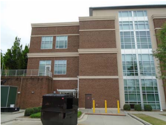
255120a 5/11/2021 Brick masonry, dual-pane windows, and EIFS accents North exterior
