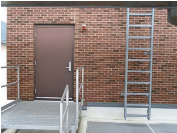
255002a 5/11/2021 Roof service door Center roof area
