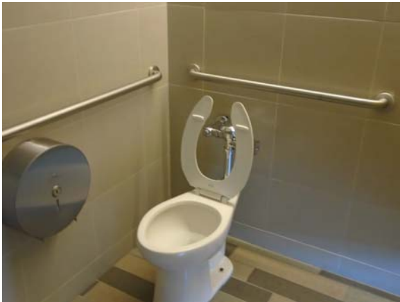
255056a 5/11/2021 Accessible toilet Restroom
