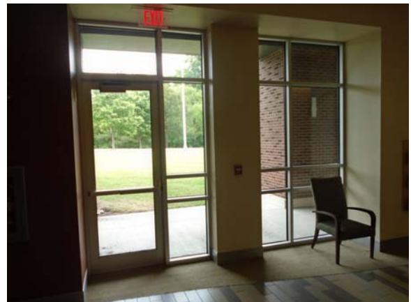
255111a 5/11/2021 Glazed storefront entry Lower level
