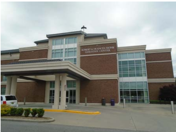
255134a 5/11/2021 Brick masonry, dual-pane windows, and EIFS accents Southeast corner
