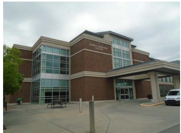
255129a 5/11/2021 Brick masonry, dual-pane windows, and EIFS accents Southwest corner
