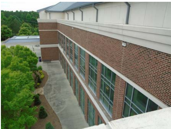
255012a 5/11/2021 Brick masonry exterior, dual-pane windows South exterior
