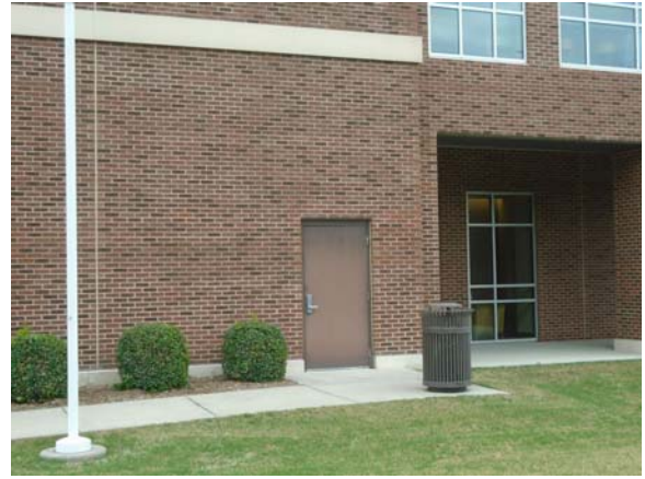
255125a 5/11/2021 Brick masonry, dual-pane windows, and EIFS accents West exterior
