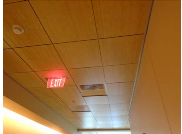
255109a 5/11/2021 Wood grid ceiling system Lower level elevator lobby
