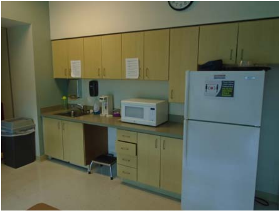
255067a 5/11/2021 Accessible base cabinetry with sink and overhead cabinetry Staff lounge 2411C
