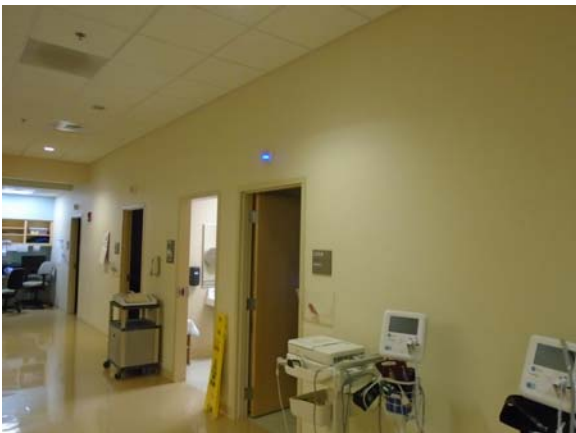
255116a 5/11/2021 Vinyl tile floor, painted walls, and suspended grid ceiling Lower level clinic
