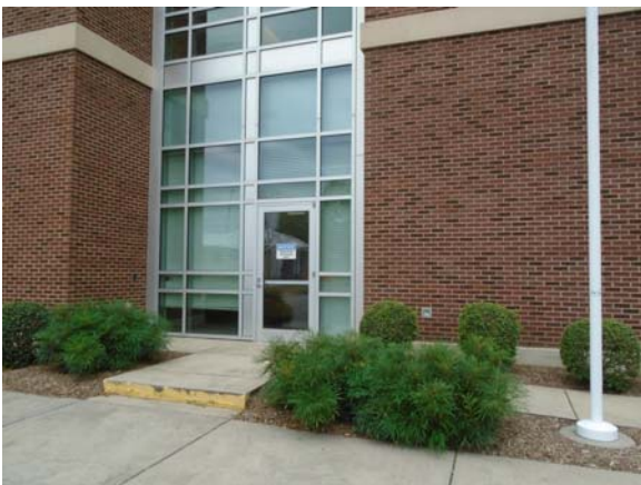
255122a 5/11/2021 Glass storefront entry North exterior
