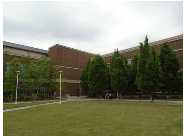
255139a 5/11/2021 Brick masonry, dual-pane windows, and EIFS accents East exterior
