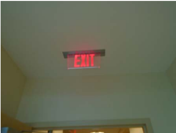
255071a 5/11/2021 Adequate exit signage First floor corridor
