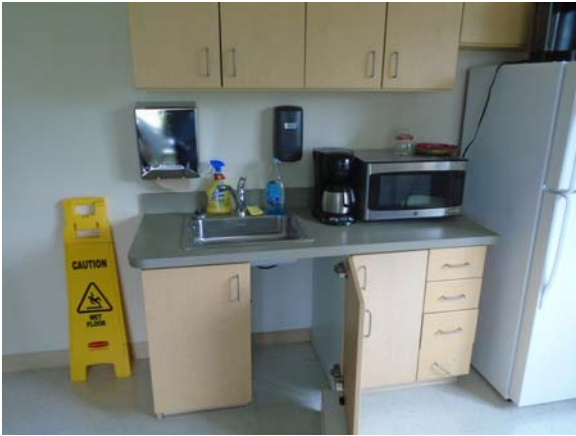
255037a 5/11/2021 Accessible base cabinetry with sink and overhead cabinetry Staff lounge 2411C
