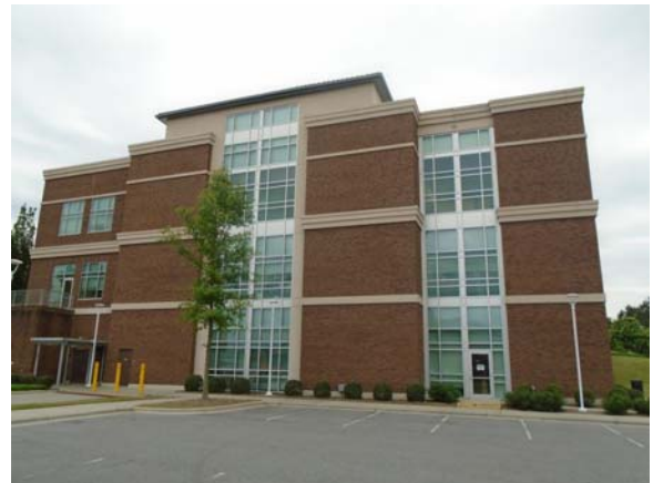
255121a 5/11/2021 Brick masonry, dual-pane windows, and EIFS accents North exterior
