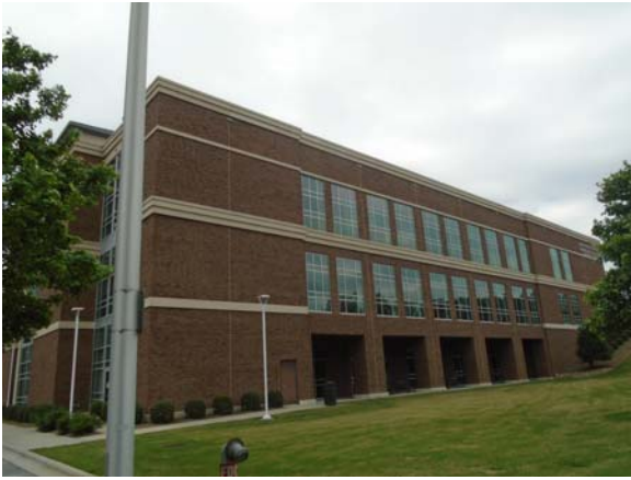
255124a 5/11/2021 Brick masonry, dual-pane windows, and EIFS accents West exterior
