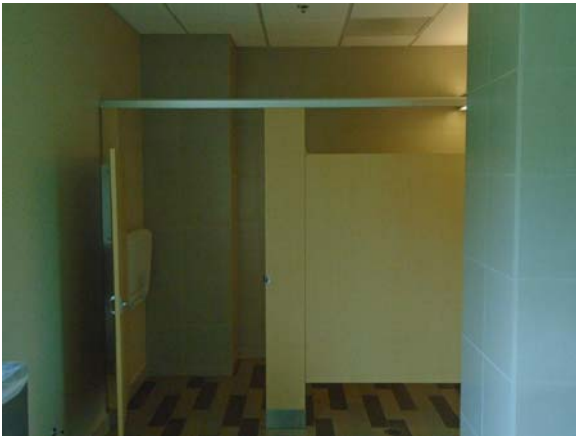
255053a 5/11/2021 Ceramic floor and wall tile, grid ceiling Restroom
