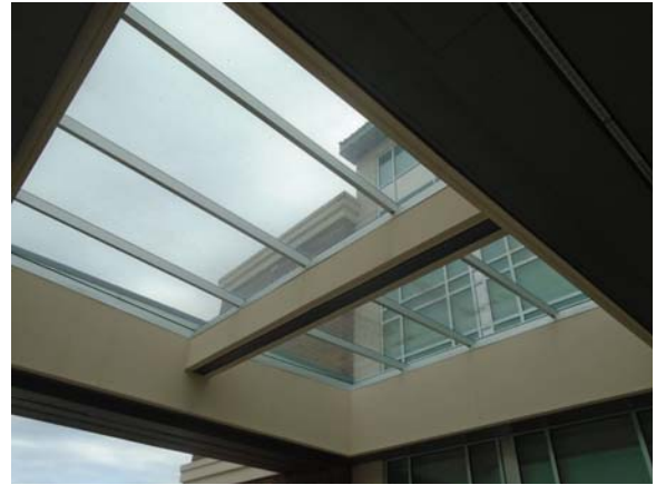
255131a 5/11/2021 Glassed skylights over entry canopies Ground level entries
