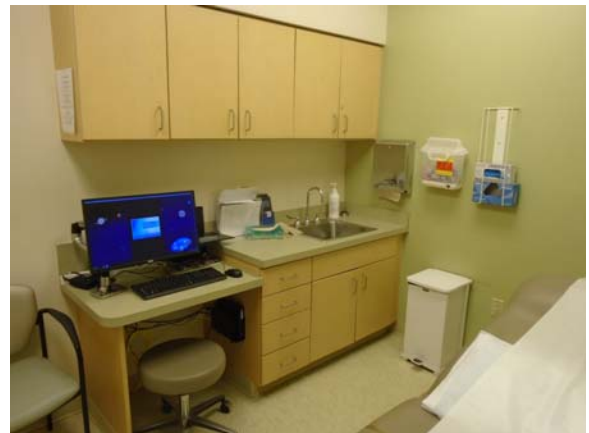
255093a 5/11/2021 Wood base cabinetry with sink and overhead cabinetry First floor exam room
