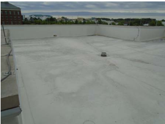
255021a 5/11/2021 Single-ply membrane roof Southeast roof
