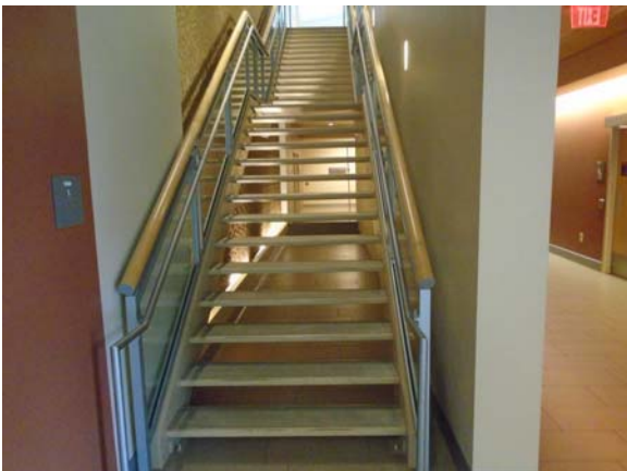
255110a 5/11/2021 Compliant stairwells with proper handrailing Stairwell 1
