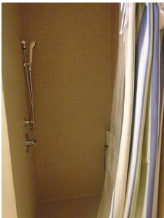
255104a 5/11/2021 Ceramic tiled accessible shower Staff locker room L104A
