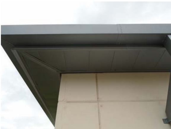
255018a 5/11/2021 Metal roof crown and fascia Roof
