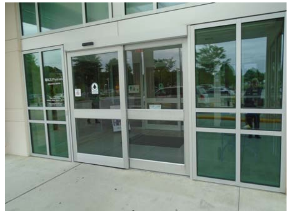
255135a 5/11/2021 Dual double glass airlock door system Southeast entry
