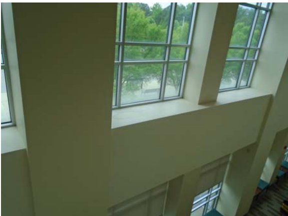
255045a 5/11/2021 Dual-pane windows Second floor, atrium
