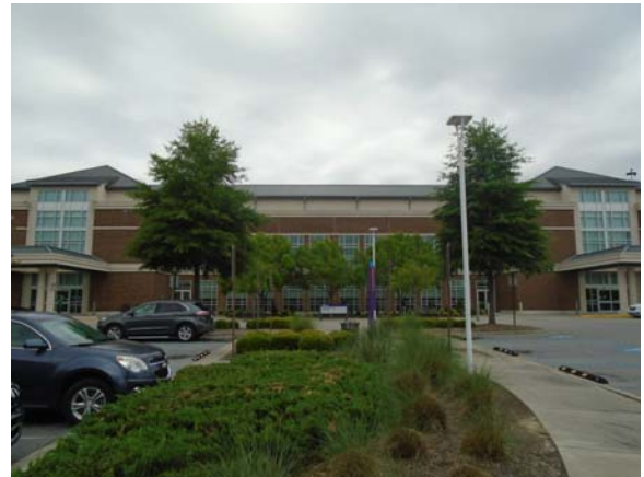
255133a 5/11/2021 Brick masonry, dual-pane windows, and EIFS accents South exterior
