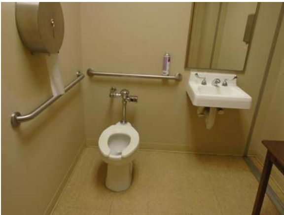
255069a 5/11/2021 Accessible fixtures and vinyl floor tile Single-user restroom
