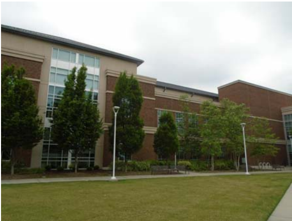
255138a 5/11/2021 Brick masonry, dual-pane windows, and EIFS accents East exterior
