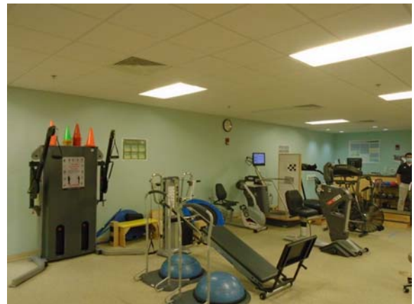
255117a 5/11/2021 Carpeting, painted walls, and suspended grid ceiling Lower level, physical therapy
