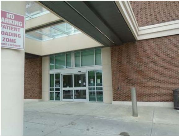
255130a 5/11/2021 Dual double glass airlock door system Southwest entry
