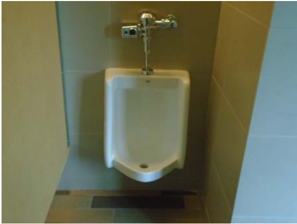
255055a 5/11/2021 Urinal Men's restroom
