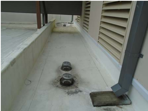
255008a 5/11/2021 Roof drains Roof
