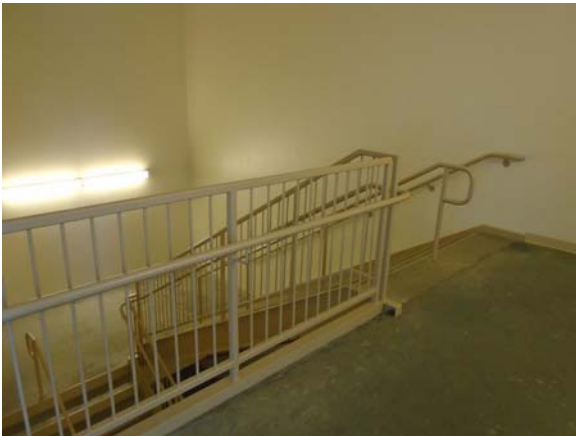
255041a 5/11/2021 Compliant stairwells with proper handrailing Stairwell 4
