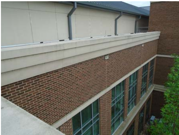
255017a 5/11/2021 Brick masonry, dual-pane windows, and paneled penthouse Northeast exterior
