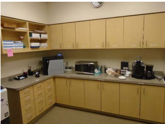
255063a 5/11/2021 Wood base and overhead cabinetry, vinyl floor tile Workroom 2505B
