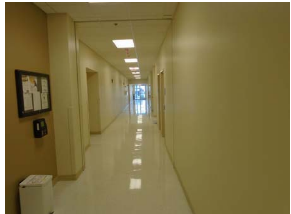
255105a 5/11/2021 Vinyl tile floor, painted walls, and suspended grid ceiling Lower level corridor
