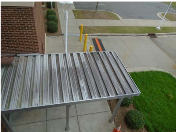
255140a 5/11/2021 Metal canopy North entry
