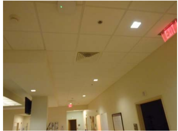
255079a 5/11/2021 Suspended grid ceiling Clinic
