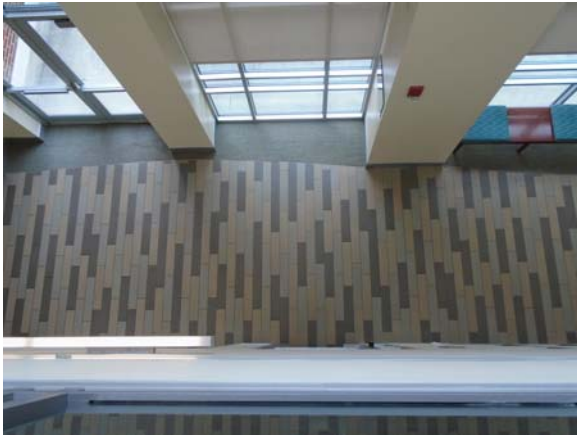
255046a 5/11/2021 Ceramic tile floor First floor
