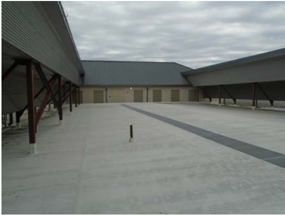
255001a 5/11/2021 Single-ply membrane roof Center roof area
