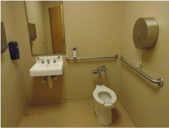
255068a 5/11/2021 Accessible fixtures and vinyl floor tile Single-user restroom
