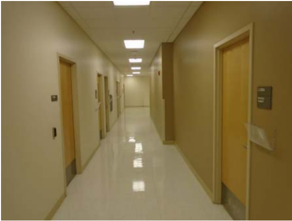
255106a 5/11/2021 Vinyl tile floor, painted walls, and suspended grid ceiling Lower level corridor
