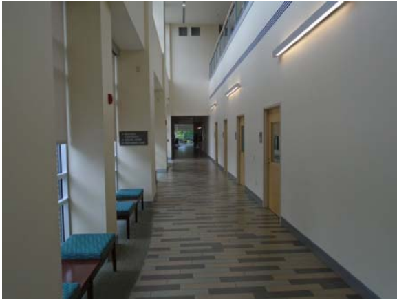
255082a 5/11/2021 Ceramic tile floor First floor
