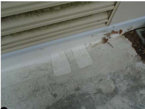
255009a 5/11/2021 Previous roof repair Roof
