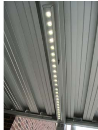
255069e 5/11/2021 String LED light fixture North exterior
