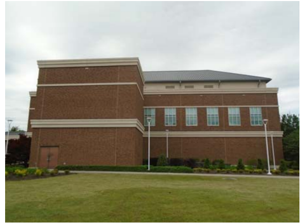
255137a 5/11/2021 Brick masonry, dual-pane windows, and EIFS accents East exterior
