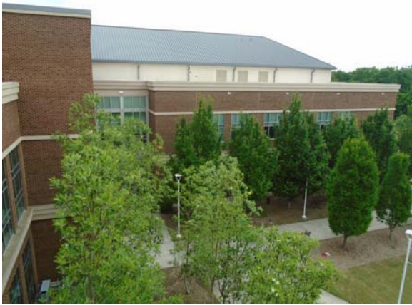
255016a 5/11/2021 Brick masonry, dual-pane windows, and paneled penthouse Northeast exterior
