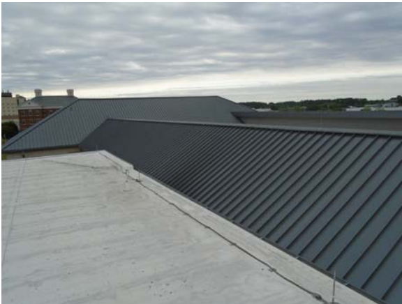
255005a 5/11/2021 Standing seam metal roof Pitched roof over mechanical penthouse
