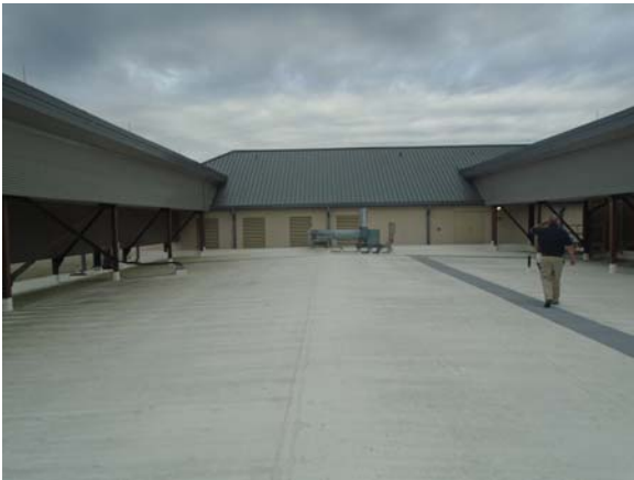
255023a 5/11/2021 Single-ply membrane roof Center roof area
