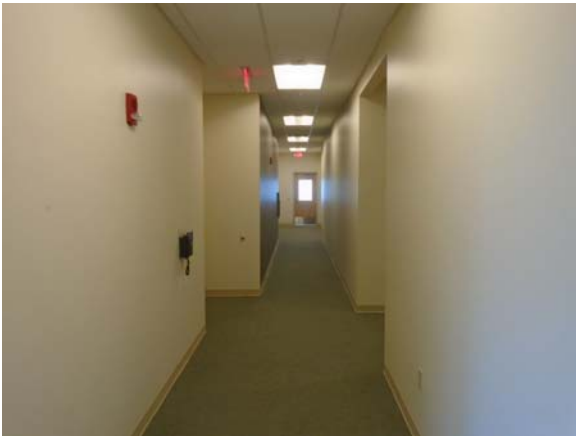
255026a 5/11/2021 Carpeting, painted walls, and suspended grid ceiling Second floor corridor
