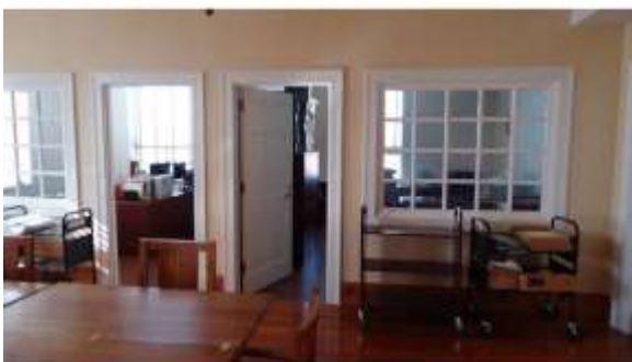
AHSB015a 4/20/2016 Heart of pine floors, painted walls, and fire rated glazing Historic Collections Reading room
