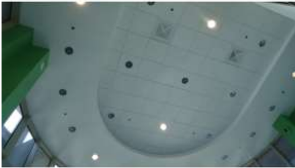
AHSB044a 4/20/2016 Painted and suspended ceilings First floor, snack bar
