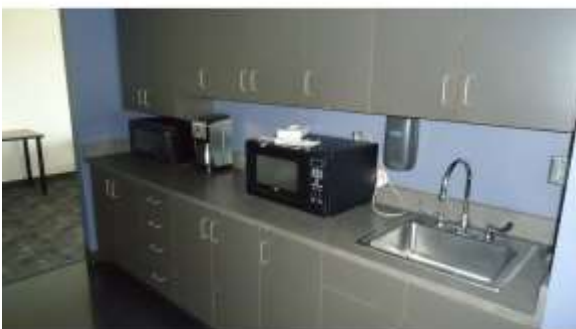
AHSB030a 4/20/2016 Built-in cabinetry Fourth floor, kitchen
