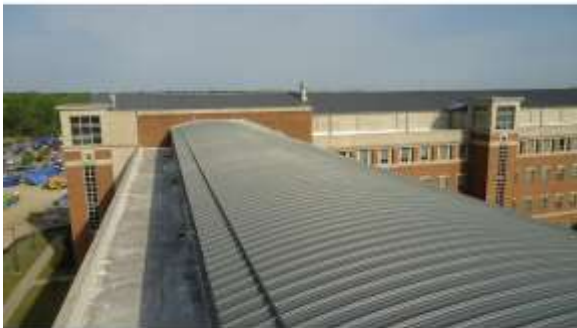
AHSB005a 4/20/2016 Pitched standing seam metal roof Upper level roof
