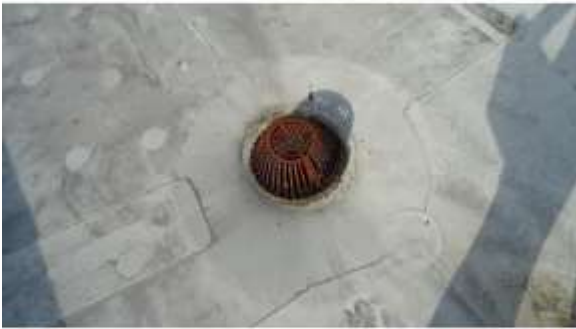
AHSB002a 4/20/2016 Single-ply TPO, flat roof with drain Mid level roof
