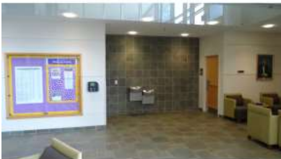
AHSB042a 4/20/2016 Slate floor tile and wall tile First floor, north
