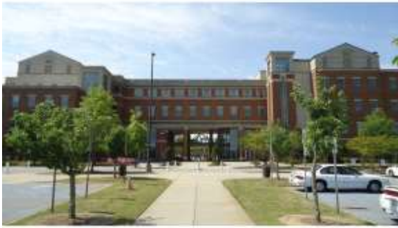
AHSB067a 4/20/2016 Brick masonry, dual-pane or tempered glazing, and standing seam metal roof North elevation, B and C wings
