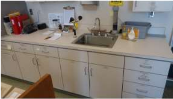
AHSB019a 4/20/2016 Laminated wooden lab cabinetry Preservation lab
