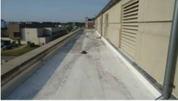
AHSB001a 4/20/2016 Single-ply TPO, flat roof Lower level roof
