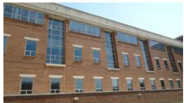
AHSB082a 4/20/2016 Brick masonry, dual-pane or tempered glazing, and concrete veneer crown South elevation, E wing
