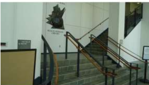
AHSB027a 4/20/2016 Slate tiled floor and staircase First floor, southern entrance
