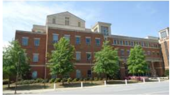
AHSB060a 4/20/2016 Brick masonry, dual-pane or tempered glazing, and standing seam metal roof North elevation, C wing
