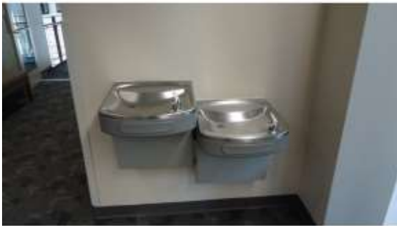
AHSB008a 4/20/2016 Compliant dual-level drinking fountain Fourth floor
