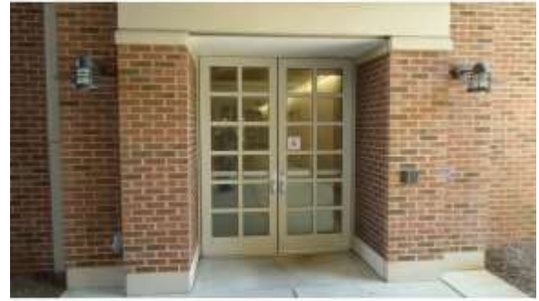
AHSB078a 4/20/2016 Aluminum-framed glass entrance doors Exterior envelope
