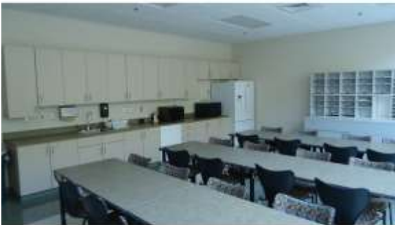
AHSB023a 4/20/2016 Vinyl tiled floors, suspended grid ceilings, and built-in cabinetry First floor, break room
