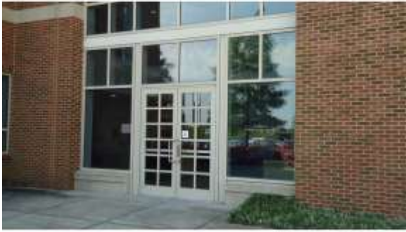
AHSB065a 4/20/2016 Aluminum-framed glass entrance doors Exterior envelope
