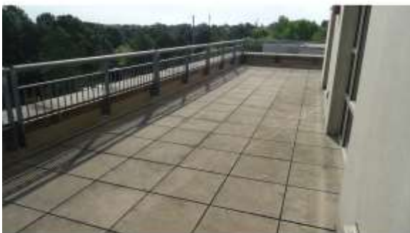
AHSB009a 4/20/2016 Exterior patio/roof Fourth floor
