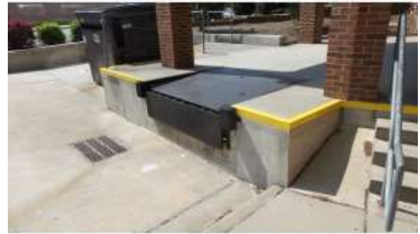
AHSB056e 4/20/2016 Hydraulic dock leveler Exterior, loading dock
