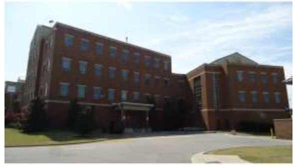
AHSB068a 4/20/2016 Brick masonry, dual-pane or tempered glazing, and standing seam metal roof East side A and B wings
