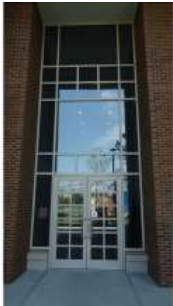
AHSB079a 4/20/2016 Aluminum-framed glass entrance doors Exterior envelope
