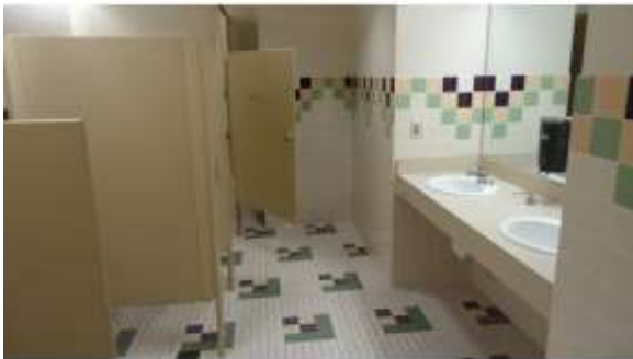
AHSB011a 4/20/2016 Ceramic tiled lower walls and floors and accessible fixtures Typical restrooms
