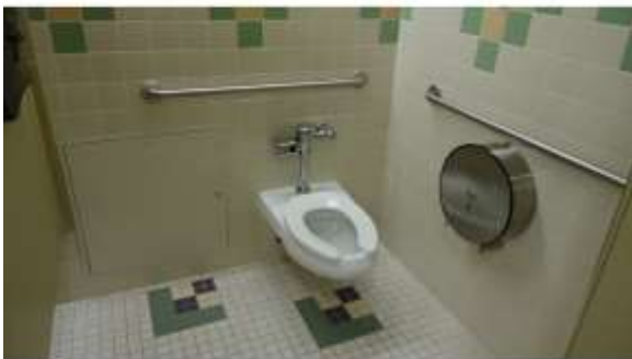
AHSB012a 4/20/2016 Ceramic tiled lower walls and floors and accessible fixtures Typical restrooms
