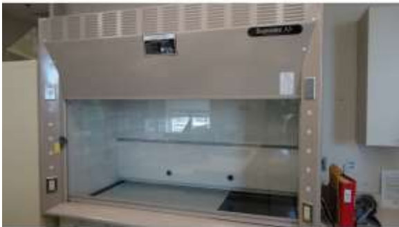
AHSB018a 4/20/2016 Exterior exhausted fume hood Preservation Lab
