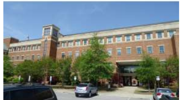
AHSB058a 4/20/2016 Brick masonry, dual-pane or tempered glazing, and standing seam metal roof East elevation, D wing
