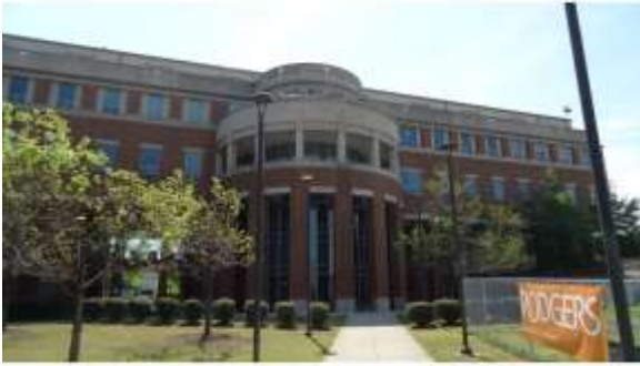
AHSB077a 4/20/2016 Brick masonry, dual-pane or tempered glazing, and standing seam metal roof West elevation, D wing
