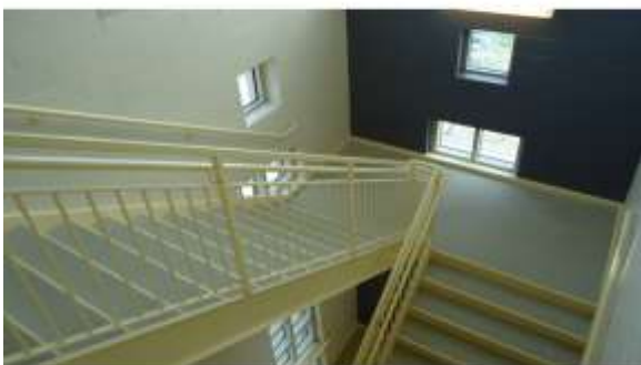
AHSB006a 4/20/2016 Typical stairwell with compliant handrails and guardrailing Stairwell
