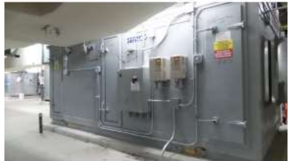
AHSB011e 4/20/2016 Energy recovery unit ERU-4 East Penthouse
