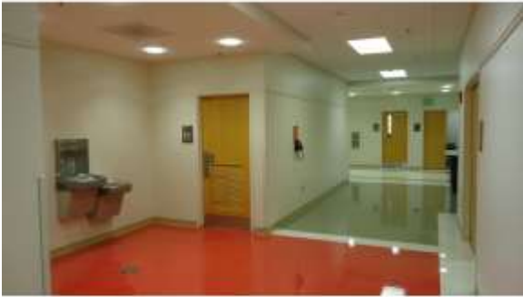
AHSB025a 4/20/2016 Vinyl tiled floors, suspended grid ceilings, and built-in cabinetry First floor
