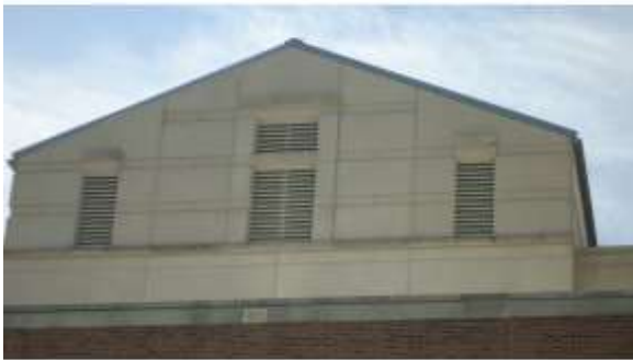
AHSB061a 4/20/2016 Concrete panel exterior veneer North elevation, C wing
