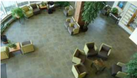
AHSB038a 4/20/2016 Slate tiled floor First floor, northwestern lobby
