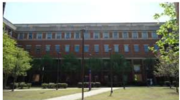
AHSB076a 4/20/2016 Brick masonry, dual-pane or tempered glazing, and standing seam metal roof West elevation, D wing
