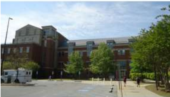
AHSB057a 4/20/2016 Brick masonry, dual-pane or tempered glazing, and standing seam metal roof North elevation, E wing
