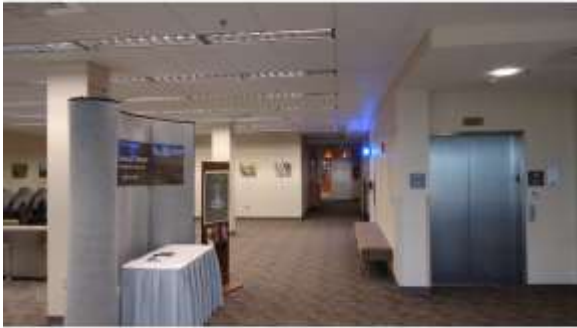
AHSB010a 4/20/2016 Suspended grid acoustical tile ceilings, painted walls, and carpeted floors Fourth floor
