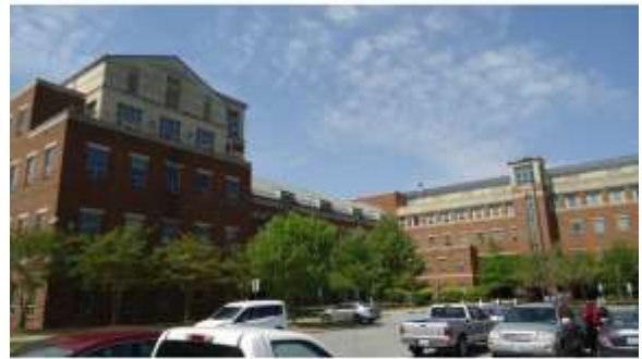
AHSB086a 4/20/2016 Brick masonry, dual-pane or tempered glazing, and standing seam metal roof Southeastern view
