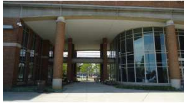
AHSB066a 4/20/2016 Brick masonry and dual-pane or tempered glazing North main entrance
