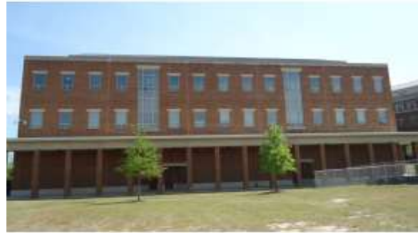
AHSB072a 4/20/2016 Brick masonry, dual-pane or tempered glazing, and standing seam metal roof West elevation, A wing
