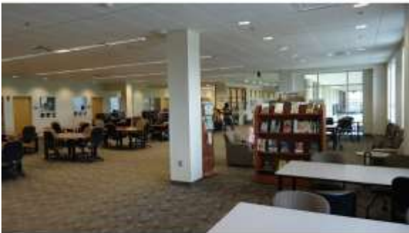
AHSB021a 4/20/2016 Suspended grid acoustical tile ceilings with painted walls and carpeted floors Third floor
