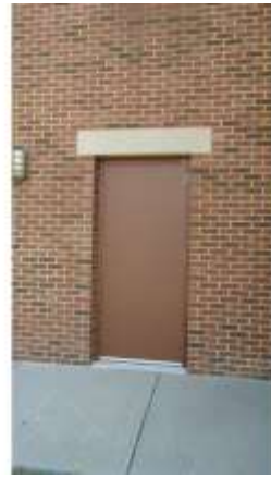
AHSB084a 4/20/2016 Hollow metal service door Exterior envelope
