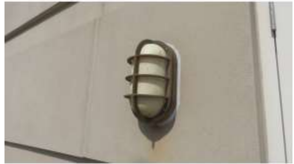
AHSB050e 4/20/2016 Surface-mounted exterior light fixture Roof
