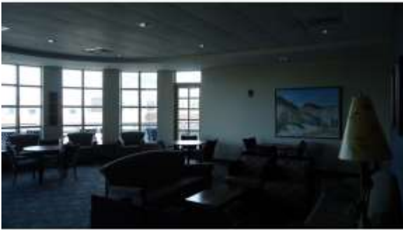
AHSB029a 4/20/2016 Suspended grid acoustical tile ceilings, painted walls, and carpeted floors Fourth floor, lounge
