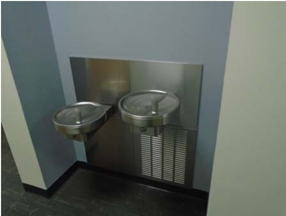
256061a 5/12/2021 Dual-level water fountain Fourth floor office suite corridor
