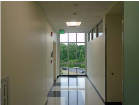
256044a 5/12/2021 Vinyl tile floor, painted walls, and suspended grid ceiling Fourth floor corridor
