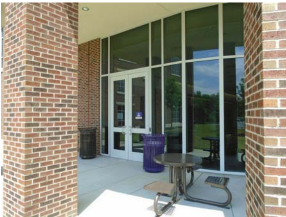
256021a 5/12/2021 Aluminum-framed glass entry doors and storefront glazing South exterior
