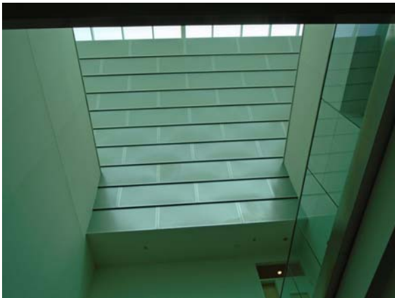
256085a 5/12/2021 Metal panel wall Atrium
