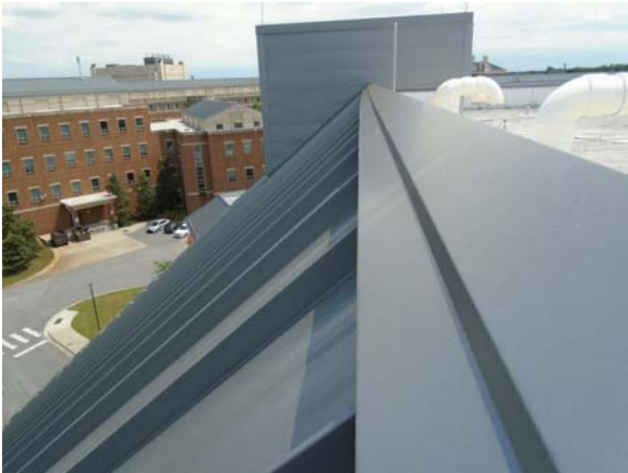
256031a 5/12/2021 Standing seam metal roof Perimeter pitched roof
