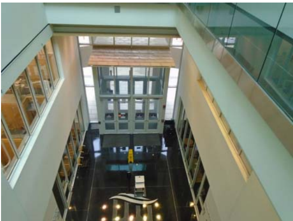
256089a 5/12/2021 Terrazzo floor and painted walls Center atrium area
