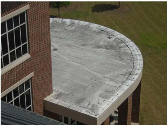
256036a 5/12/2021 Lower flat roof over the southern waiting area Lower roof
