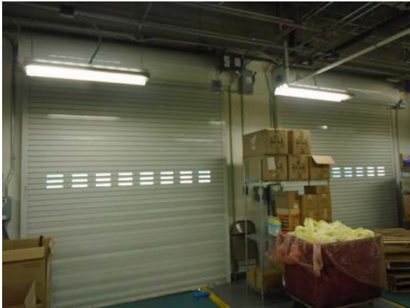
256118a 5/12/2021 Overhead garage doors Loading dock and receiving
