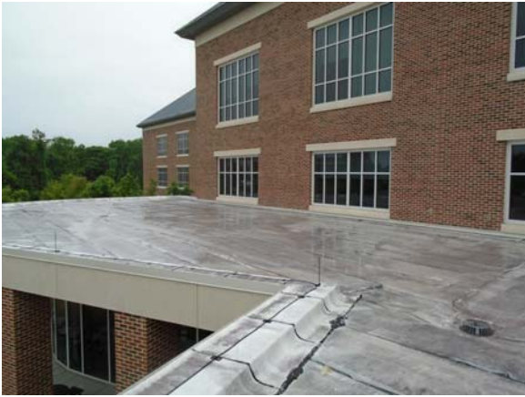
256127a 5/12/2021 Asphalt built-up roof over second floor South lower roof
