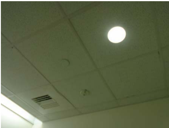
256040a 5/12/2021 Suspended grid ceiling system Fifth floor mechanical attic restroom
