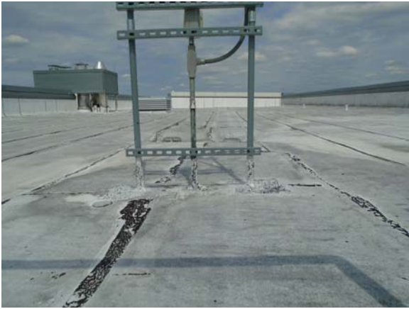
256038a 5/12/2021 Built-up asphalt roofing Central flat roof
