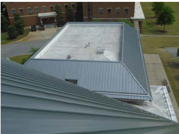
256033a 5/12/2021 Lower roof over the lecture halls Lower south roof
