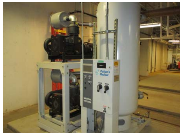
256114e 5/11/2021 Patton's Medical vacuum system with two 15 hp motors (WAGD) Room B0100
