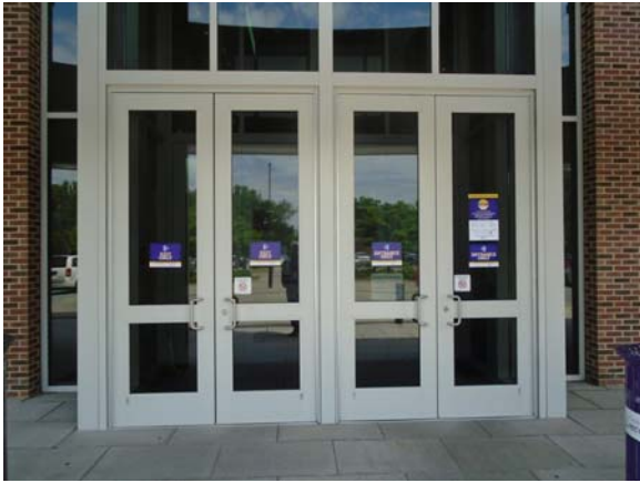
256008a 5/12/2021 Aluminum-framed glass entry doors North first floor entry
