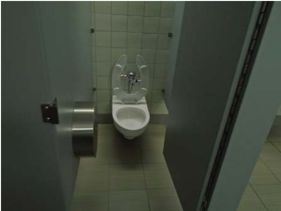
256070a 5/12/2021 Ceramic tile finishes and regular toilet stall Men's restroom 4170
