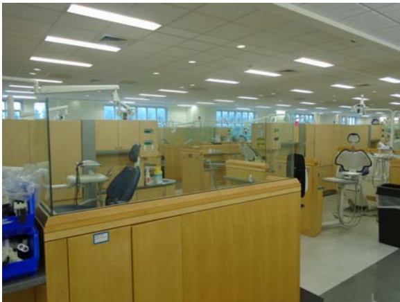
256098a 5/12/2021 Vinyl tile floor, painted walls, and suspended grid ceiling Second floor dental training area
