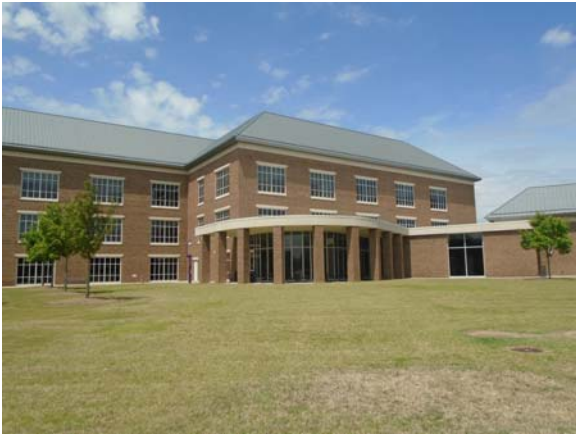
256019a 5/12/2021 Aluminum-framed dual-pane windows with stained cast concrete sills South exterior
