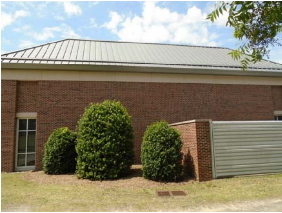
256025a 5/12/2021 Brick masonry exterior with cast concrete accents and dual-pane windows East exterior
