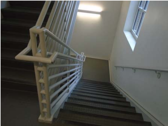
256088a 5/12/2021 Compliant handrails Stairwell 2
