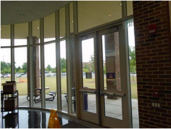
256106a 5/12/2021 Aluminum-framed glass entry doors Second floor
