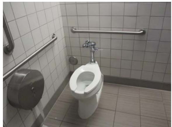
256090e 5/11/2021 Water closet in original restroom Third floor restroom
