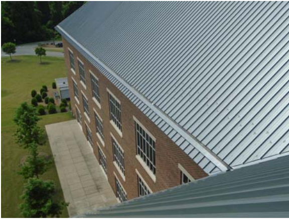
256034a 5/12/2021 Standing seam metal roof Perimeter pitched roof
