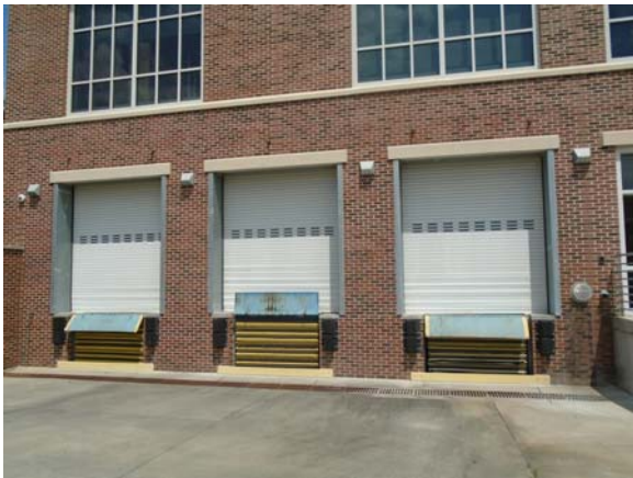
256014a 5/12/2021 Three docks and stormwater trench drain West exterior
