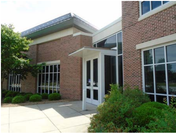
256005a 5/12/2021 Aluminum-framed glass entry doors with power openers Southeast entry to lecture halls
