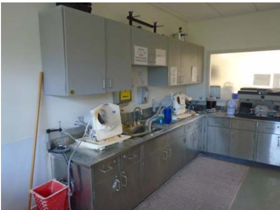
256093a 5/12/2021 Stainless steel lab cabinetry and sinks Lab suite 2225
