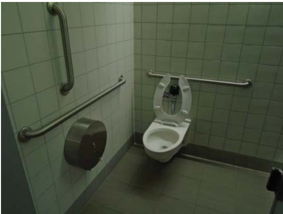
256071a 5/12/2021 Ceramic tile finishes and accessible toilet Men's restroom 4170
