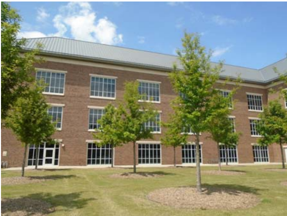
256018a 5/12/2021 Aluminum-framed dual-pane windows with stained cast concrete sills Southwest exterior
