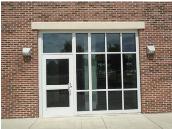
256024a 5/12/2021 Aluminum-framed glass entry doors and storefront glazing Southeast exterior
