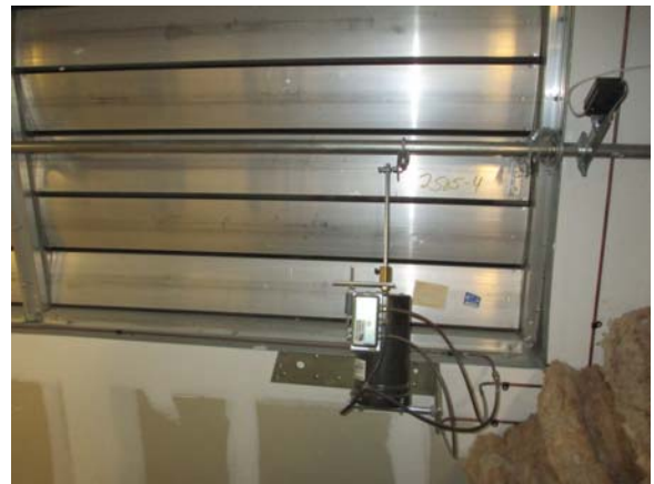
256021e 5/11/2021 Pneumatic actuator on outside air louvers Northwest corner of penthouse
