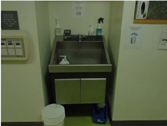
256115a 5/12/2021 Large stainless steel utility sink First floor lab area
