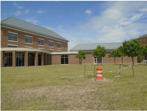
256020a 5/12/2021 Aluminum-framed dual-pane windows with stained cast concrete sills Southeast exterior
