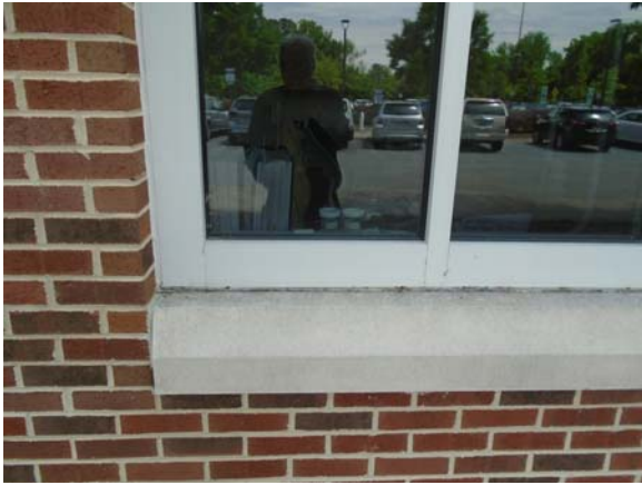
256007a 5/12/2021 Example of adequately caulked window East exterior
