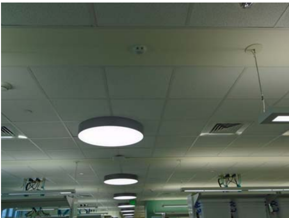
256053a 5/12/2021 Suspended grid ceiling Fourth floor lab
