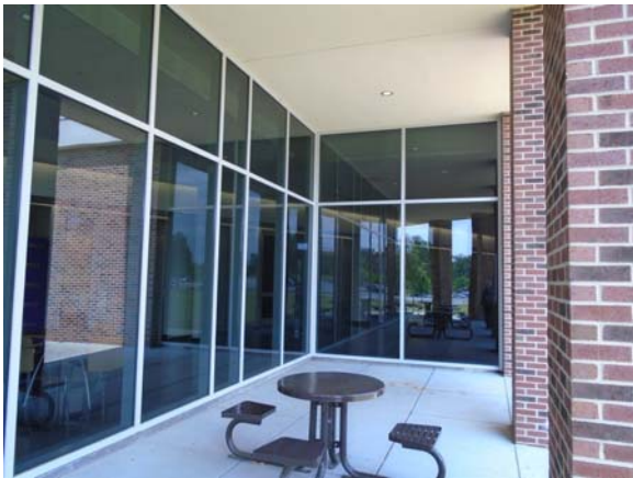
256023a 5/12/2021 Floor-to-ceiling glazing South exterior
