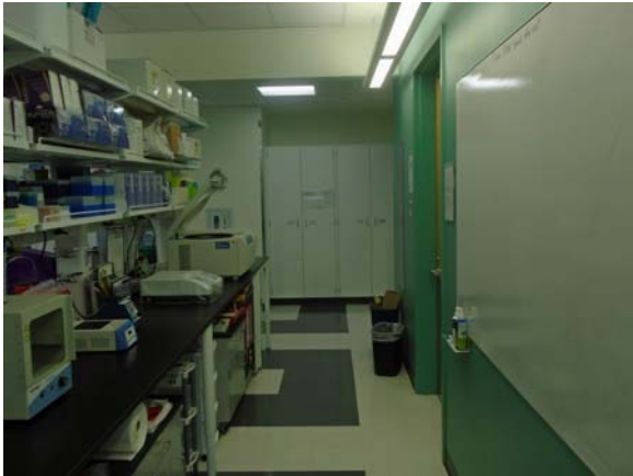
256050a 5/12/2021 Vinyl floor tile, suspended grid ceiling, and metal lab furniture Lab 4200
