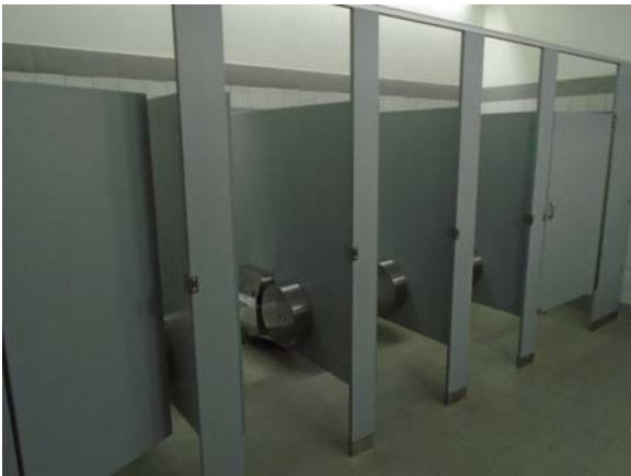
256074a 5/12/2021 Ceramic tile finishes and regular toilet stalls Women's restroom 4171
