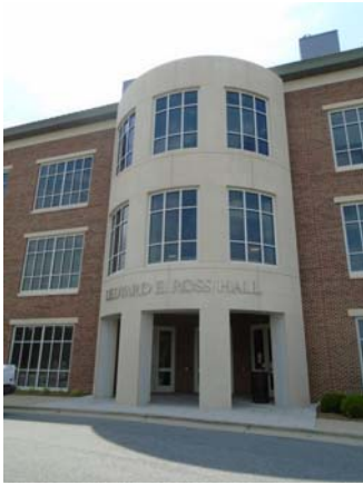
256001a 5/12/2021 Brick masonry exterior with cast concrete accents and dual-pane windows Second floor east entry
