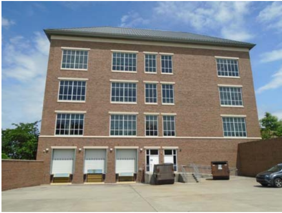
256013a 5/12/2021 Loading dock and receiving entrance West first floor entry
