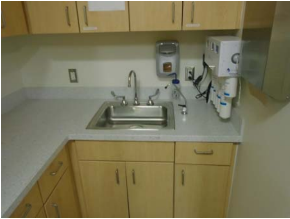
256103a 5/12/2021 Small lab sink with wood base and overhead cabinetry Second floor clinical research
