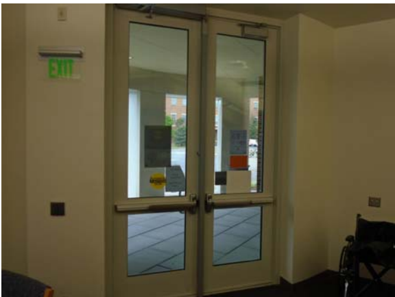
256102a 5/12/2021 Aluminum-framed glass entry doors Second floor
