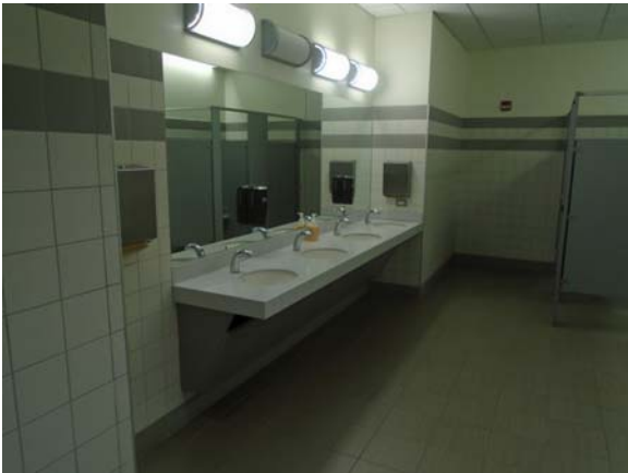
256068a 5/12/2021 Ceramic tile finishes and accessible sinks Men's restroom 4170
