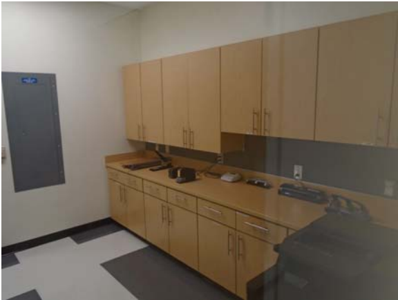
256043a 5/12/2021 Vinyl tile floor and wood base and overhead cabinetry Workroom 4282
