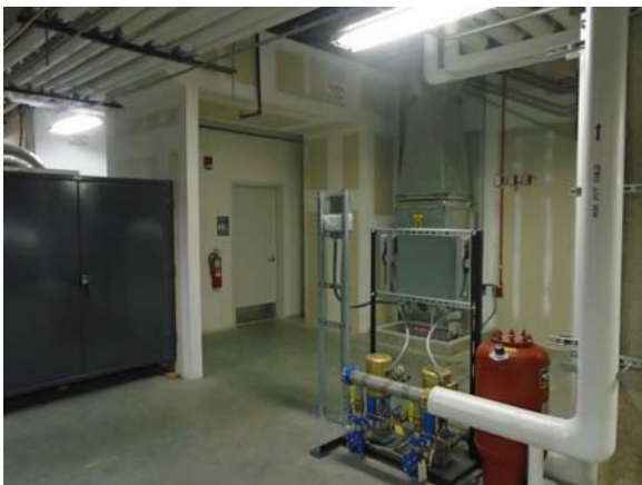
256042a 5/12/2021 Unfinished utilitarian space Fifth floor mechanical attic
