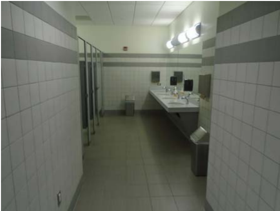
256073a 5/12/2021 Ceramic tile finishes and accessible sinks Women's restroom 4171
