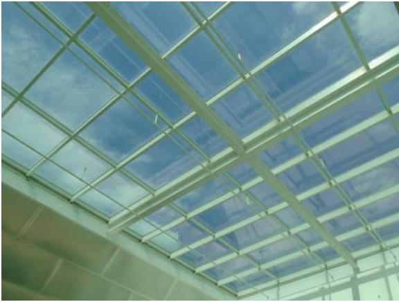
256037a 5/12/2021 Glass skylight system Central flat roof
