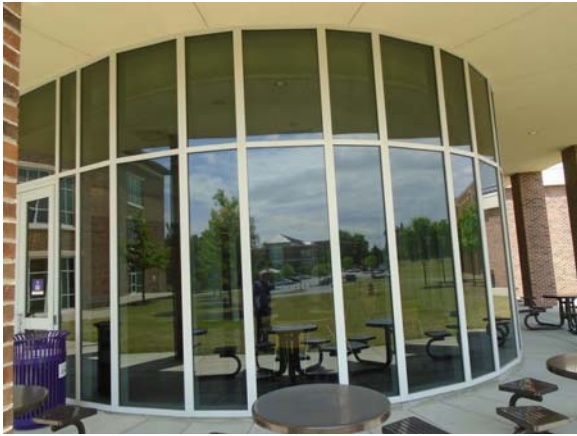
256022a 5/12/2021 Floor-to-ceiling glazing South exterior
