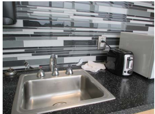
256075e 5/11/2021 Electrical outlet adjacent to kitchen sink has GFCI protection Fourth floor corridor (southeast end)
