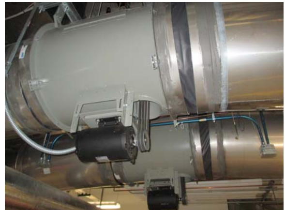
256053e 5/11/2021 Two 5 hp axial/mixed-air exhaust fans for fume hoods on the fourth floor Penthouse
