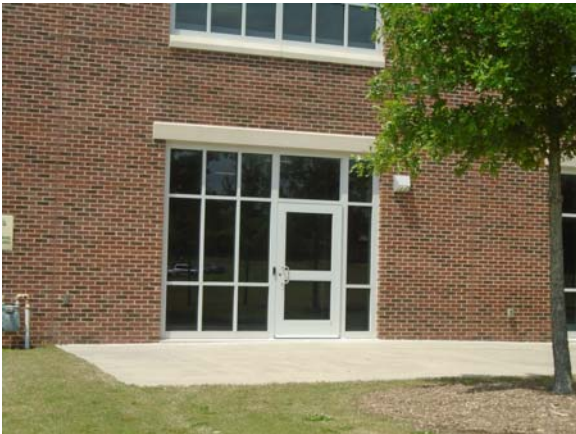
256017a 5/12/2021 Aluminum-framed glass entry doors and storefront glazing Southwest exterior
