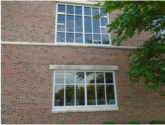
256010a 5/12/2021 Aluminum-framed dual-pane windows with stained cast concrete sills North exterior
