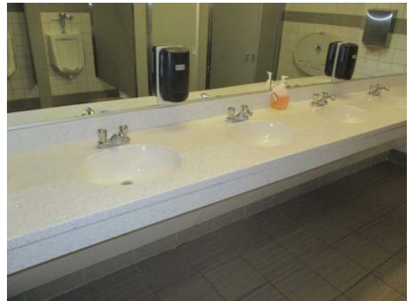
256089e 5/11/2021 Lavatories in original restroom Third floor restroom
