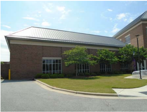
256026a 5/12/2021 Brick masonry exterior with cast concrete accents and dual-pane windows East exterior
