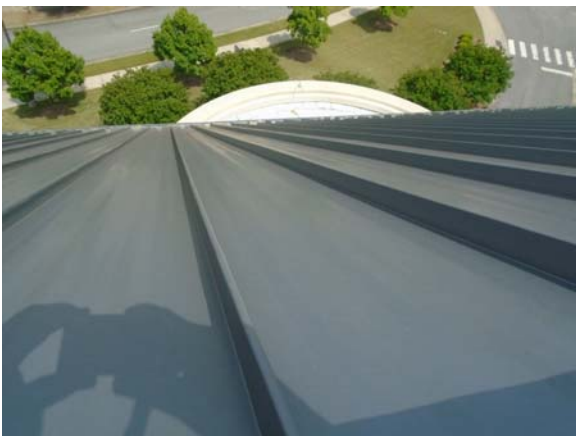
256030a 5/12/2021 Standing seam metal roof Perimeter pitched roof
