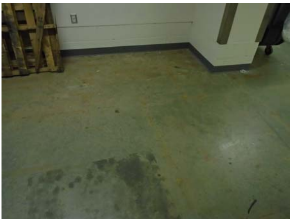
256120a 5/12/2021 Sealed concrete floor Basement
