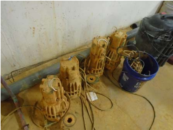
256124a 5/12/2021 Old groundwater pumps Basement
