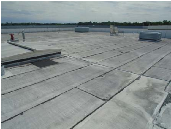
256029a 5/12/2021 Built-up asphalt roofing system Central flat roof
