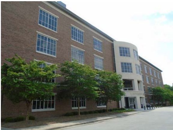
256006a 5/12/2021 Brick masonry exterior with cast concrete accents and dual-pane windows East exterior
