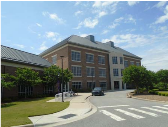
256027a 5/12/2021 Brick masonry exterior with cast concrete accents and dual-pane windows East exterior
