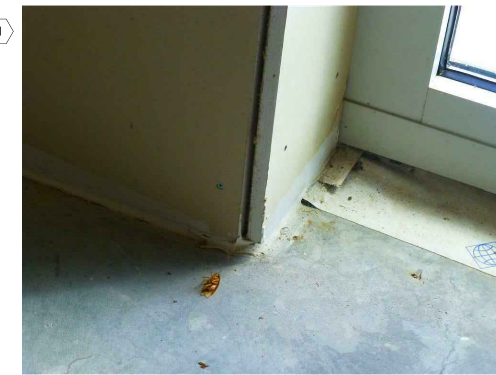
IMAGE A: TYPICAL CONDITION AT EXISTING WINDOW RETURN.
