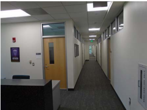
256075a 5/12/2021 Carpeting, painted walls, and suspended grid ceiling Office suite 4250
