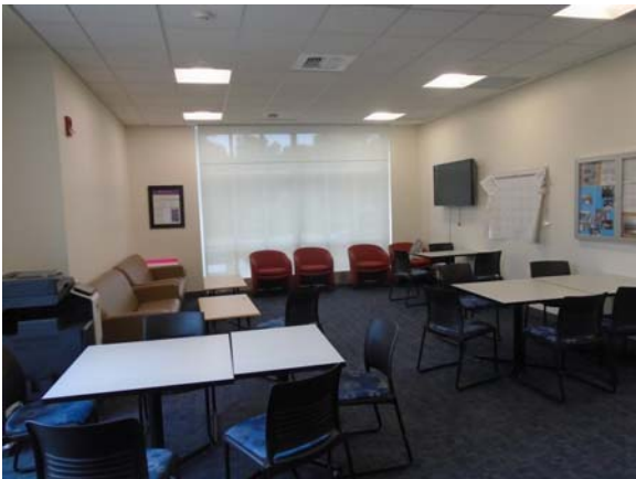
256096a 5/12/2021 Carpeting, painted walls, and suspended grid ceiling Second floor student lounge
