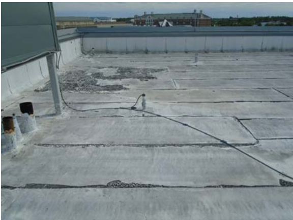
256032a 5/12/2021 Built-up asphalt roofing Central flat roof
