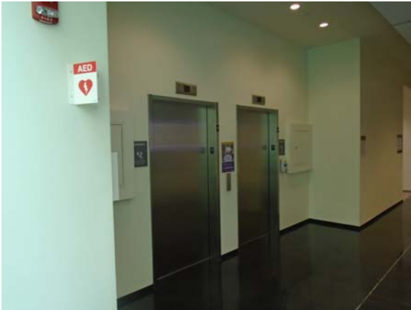
256058a 5/12/2021 Terrazzo floor and painted walls Fourth floor elevator lobby
