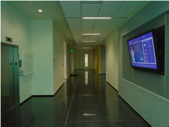
256059a 5/12/2021 Terrazzo floor and painted walls Fourth floor corridor
