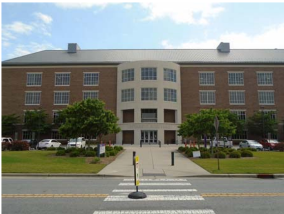
256009a 5/12/2021 Brick masonry exterior with cast concrete accents and dual-pane windows North exterior
