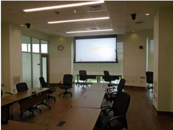
256056a 5/12/2021 Wood laminate flooring and suspended grid ceiling Conference room 4001
