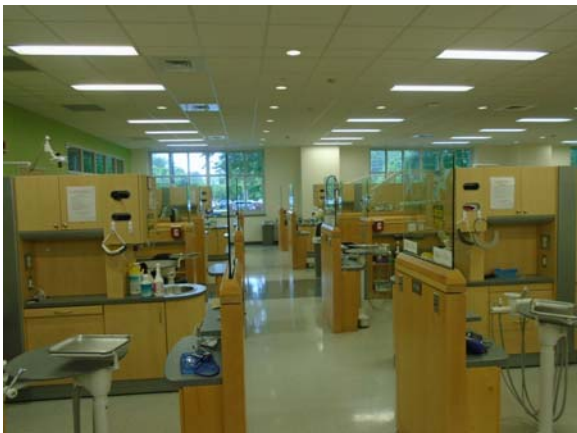
256111a 5/12/2021 Vinyl tile floor, painted walls, and suspended grid ceiling First floor dental training area
