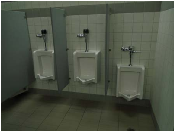
256069a 5/12/2021 Ceramic tile finishes and accessible urinals Men's restroom 4170
