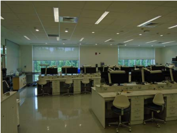
256079a 5/12/2021 Vinyl tile floor, painted walls, and suspended grid ceiling Third floor labs
