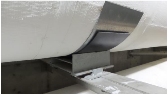
HSCW063e 4/18/2016 Pipe saddle Utility tunnel extension
