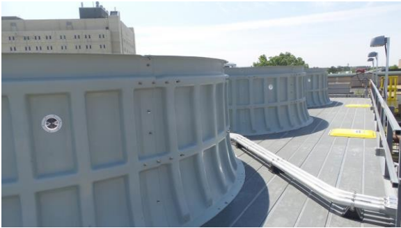
HSCW051e 4/18/2016 Three updated cooling tower cells CUP roof
