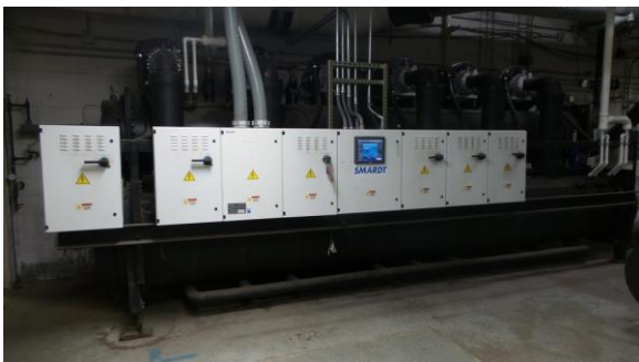
HSCW011e 4/18/2016 SMART Turbocor oil-free chiller CH-2 rated for 900 tons CUP, first floor
