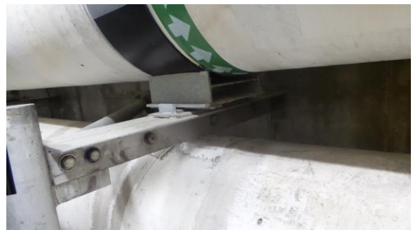
HSCW054e 4/18/2016 Pipe saddle Original utility tunnel
