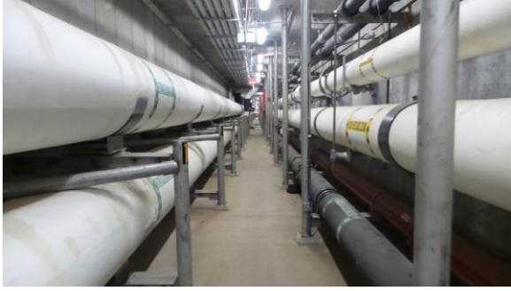
HSCW055e 4/18/2016 Utility pipe and tunnel overview Original utility tunnel
