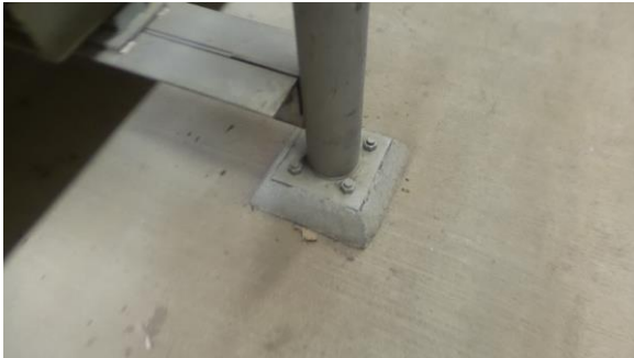
HSCW057e 4/18/2016 Pipe stanchion with stainless steel footer Original utility tunnel
