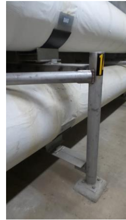
HSCW056e 4/18/2016 Pipe stanchion Original utility tunnel
