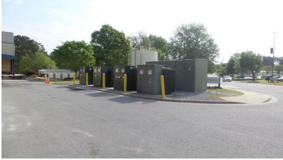
HSEL019e 4/21/2016 Oil-filled transformers and load interrupters CUP exterior
