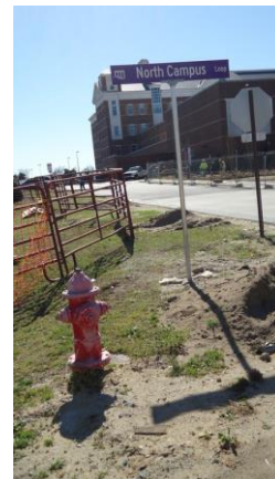
HSPWFP006e 3/8/2017 Older fire hydrant Campus grounds
