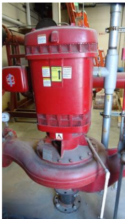
125 hp fire pump Central Plant
