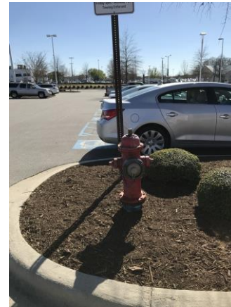
HSPWFP022e 3/8/2017 Other side of fire hydrant in photo 21e Campus grounds
