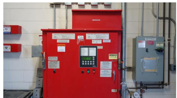
Electric fire pump controller Central Plant
