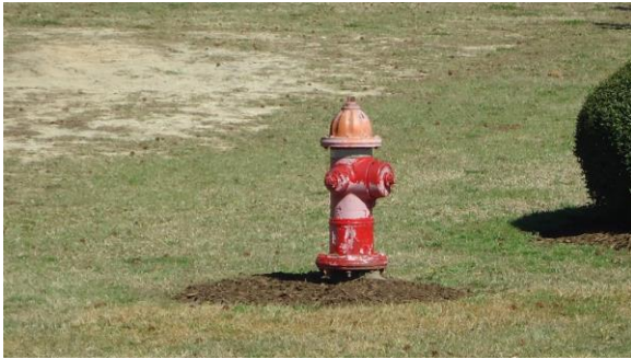
HSPWFP003e 3/8/2017 Older fire hydrant Campus grounds
