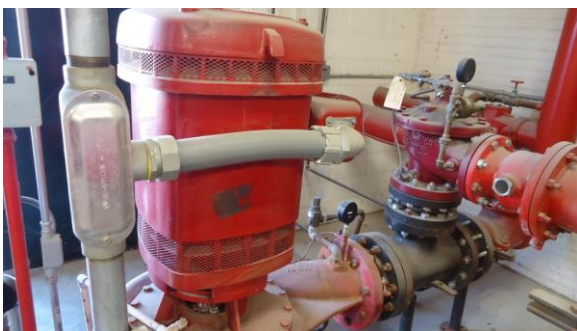
HSPWFP017e 3/8/2017 Older fire hydrant Campus grounds
