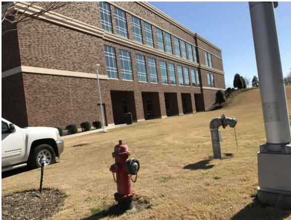
HSPWFP021e 3/8/2017 Older fire hydrant Campus grounds
