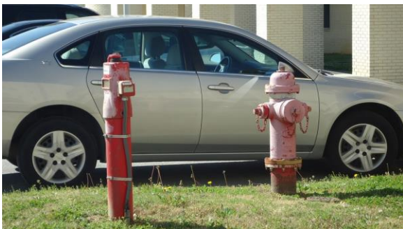
HSPWFP005e 3/8/2017 Older fire hydrant Campus grounds
