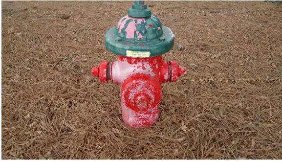
HSPWFP001e 3/8/2017 Older fire hydrant Campus grounds
