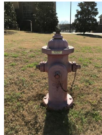
HSPWFP018e 3/8/2017 Older fire hydrant Campus grounds
