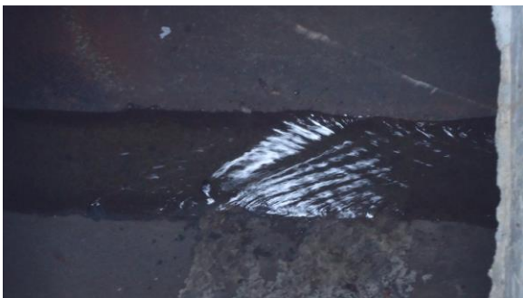
HSSANI005e 3/8/2017 Concrete manhole with flow from one inlet North Campus Drive by Biotechnology B1.2
