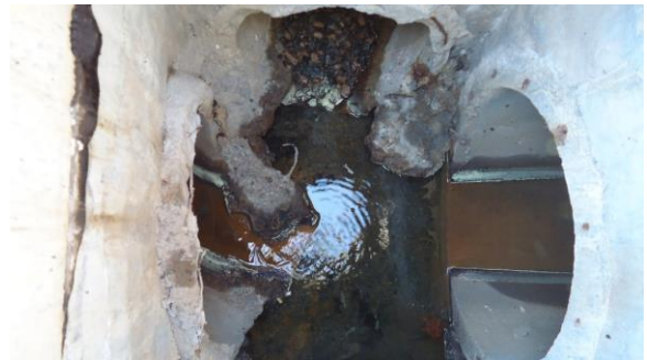
STRM064e 3/8/2017 Concrete stormwater manhole East of MacGregor Downs G2
