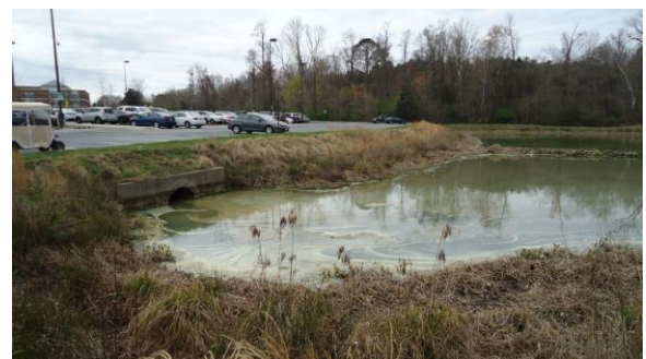
STRM024e 3/8/2017 Stormwater retention pond Dental sch. stormwater management pond
