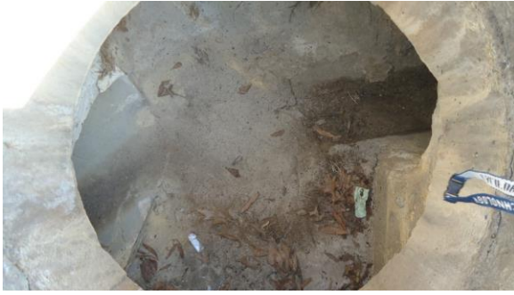
STRM061e 3/8/2017 Concrete stormwater manhole Off North Campus loop by Biotechnology
