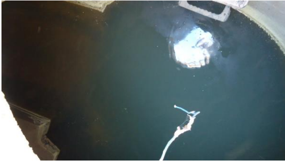
STRM067e 3/8/2017 Concrete stormwater manhole Parking lot by north Dental pond
