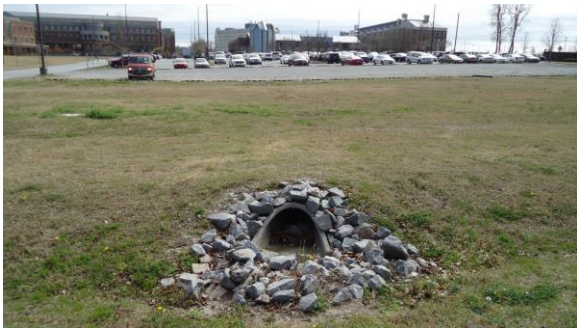
STRM033e 3/8/2017 Riprap-armored slope around pipe outlet Along MacGregor Downs Road
