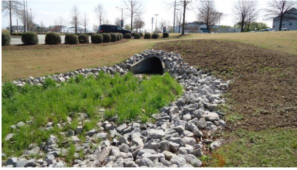
STRM043e 3/8/2017 Riprap-armored slope around 36 inch pipe outlet Northeast corner of Heart Dr and W Arlington
