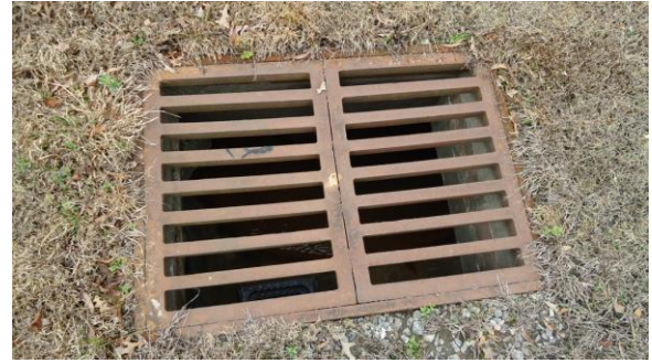
STRM020e 3/8/2017 Drainage inlet Planter island in north Dental parking lot
