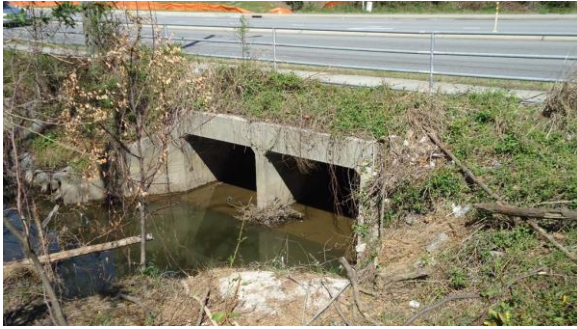
STRM055e 3/8/2017 Twin 4'x6' concrete box culverts to carry flow under road Under W 5th St to the north
