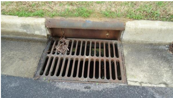
STRM015e 3/8/2017 Drainage inlet HSB south parking
