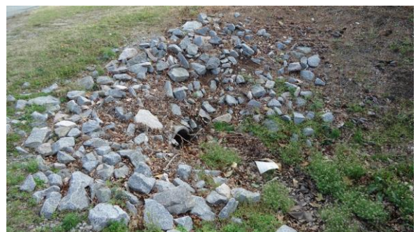
STRM036e 3/8/2017 Riprap-armored slope around pipe outlet Along MacGregor Downs Road
