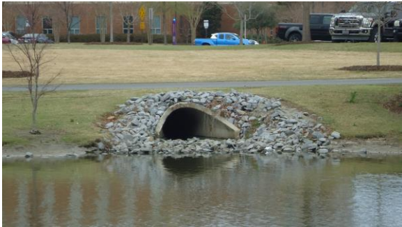
STRM009e 3/8/2017 Riprap-armored slope around pipe outlet Lake Laupus west side
