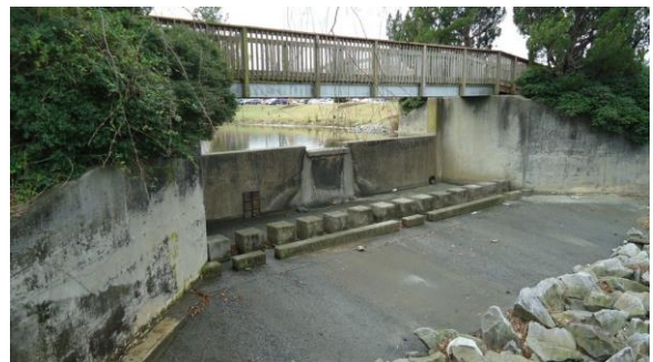
STRM012e 3/8/2017 Concrete dam and overflow weir Lake Laupus
