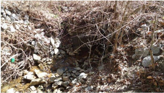
STRM039e 3/8/2017 Riprap-armored slope around pipe outlet Along MacGregor Downs Road
