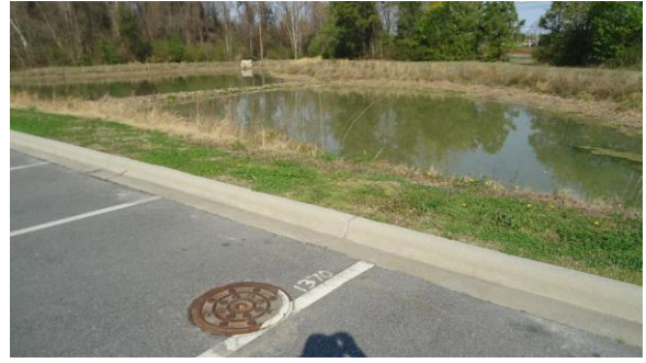
STRM068e 3/8/2017 Concrete stormwater manhole Parking lot by north Dental pond
