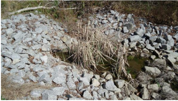
STRM049e 3/8/2017 Riprap-armored slope around pipe outlet Grounds stormwater management pond
