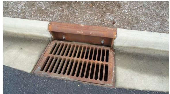
STRM022e 3/8/2017 Drainage inlet North Dental parking lot
