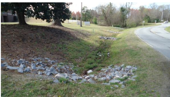
STRM035e 3/8/2017 Riprap-armored slope and small check dam Along MacGregor Downs Road
