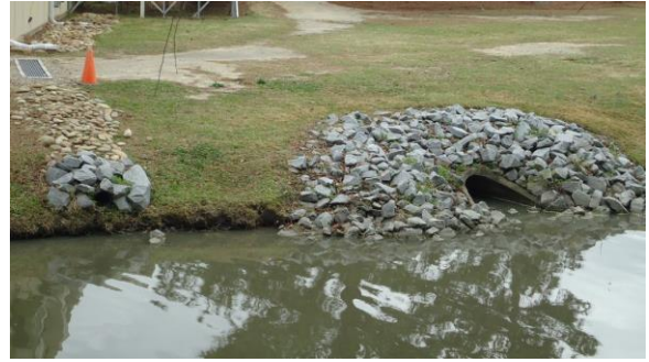
STRM008e 3/8/2017 Riprap-armored slope around pipe outlet Lake Laupus west side
