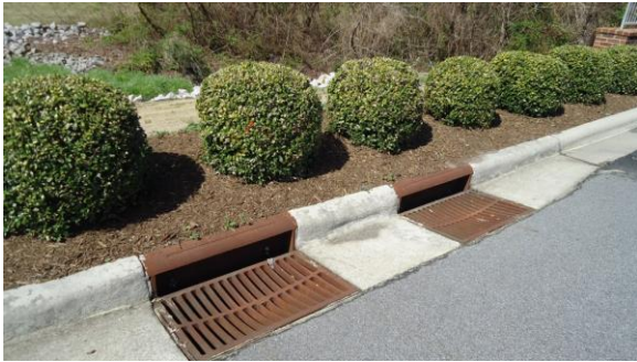
STRM045e 3/8/2017 Drainage inlets Southwest corner of Fam Med parking
