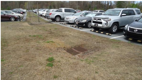
STRM021e 3/8/2017 Drainage inlet Planter island in north Dental parking lot
