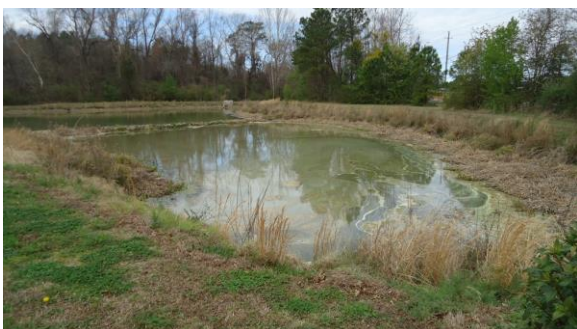
STRM023e 3/8/2017 Stormwater retention pond Dental sch. stormwater management pond
