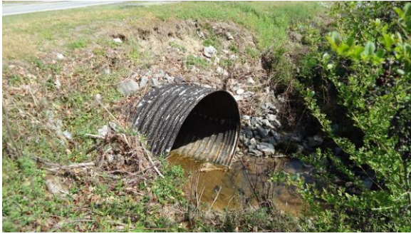
STRM037e 3/8/2017 72 inch corrugated metal pipe Under MacGregor Downs Road
