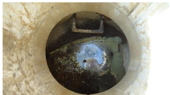
STRM066e 3/8/2017 Concrete stormwater manhole Parking lot by north Dental pond
