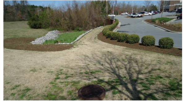
STRM044e 3/8/2017 Riprap-armored slope Northeast corner of Heart Dr and W Arlington
