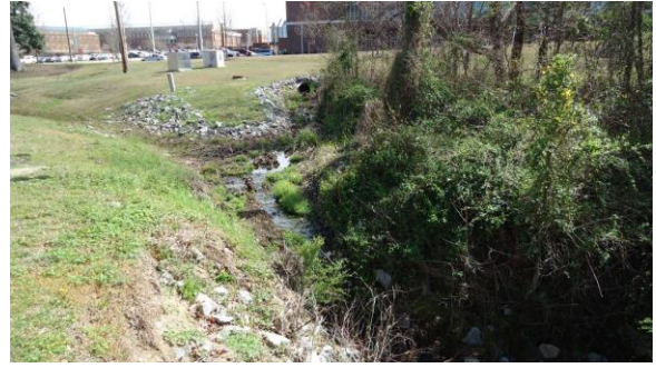
STRM038e 3/8/2017 Riprap-armored slope around pipe outlet Along MacGregor Downs Road
