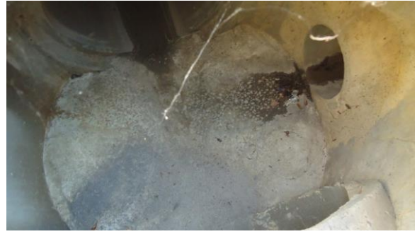
STRM062e 3/8/2017 Concrete stormwater manhole East of HSB in Health Sciences Dr
