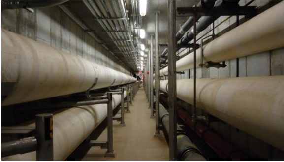
UTUN001e 4/21/2016 Poured-in-place reinforced concrete utility tunnel Beginning of tunnel by plant
