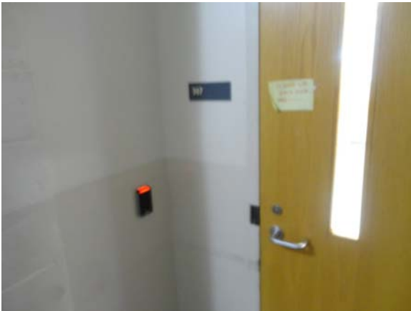
AUST023a 5/11/2021 Newer corridor doors and lever hardware Third floor
