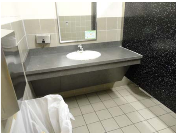
AUST033a 5/11/2021 Accessible counter lavatory First floor, men's restroom
