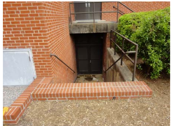
AUST052a 5/11/2021 Hollow-metal service doors at areaway Southwest elevation
