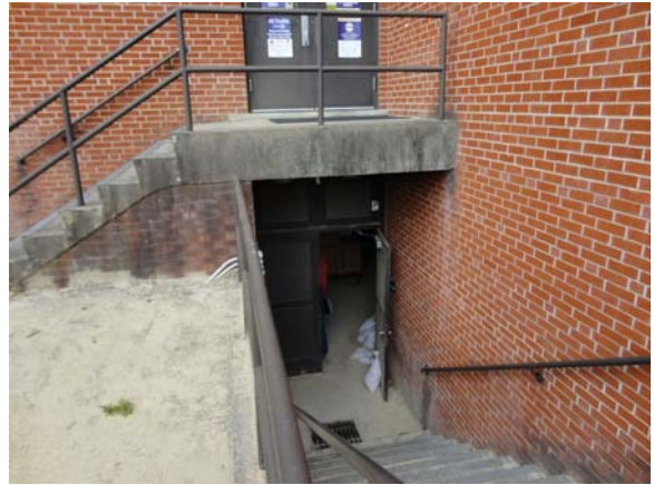
AUST054a 5/11/2021 Hollow-metal service doors at areaway Southeast elevation
