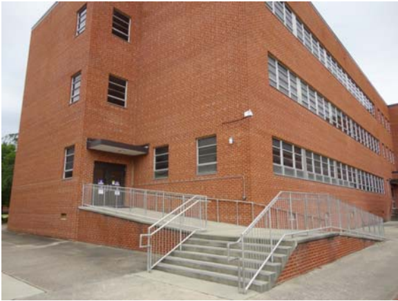
AUST053a 5/11/2021 Ramped access to first floor South end elevation
