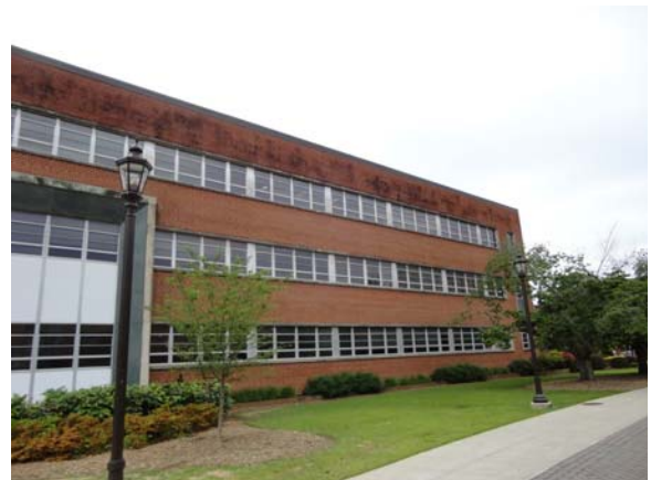
AUST046a 5/11/2021 Bands of original single-pane glazing North elevation
