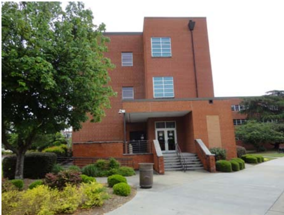
AUST049a 5/11/2021 Newer glass entry doors and newer tower windows West elevation
