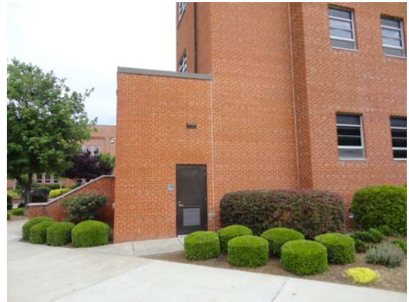
AUST050a 5/11/2021 Newer hollow-metal service door West elevation
