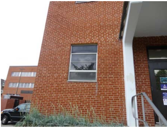
AUST043a 5/11/2021 Original single-pane, metal-framed glazing East end elevation
