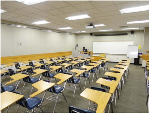
AUST022a 5/11/2021 Broadloom carpeting and lay-in acoustical ceiling Third floor, classroom
