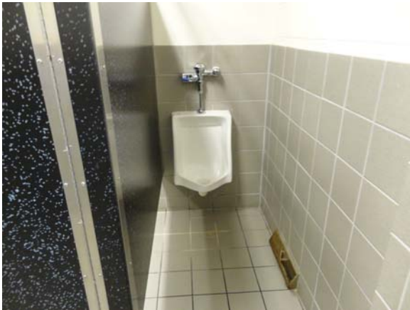
AUST035a 5/11/2021 Urinal area First floor, men's restroom
