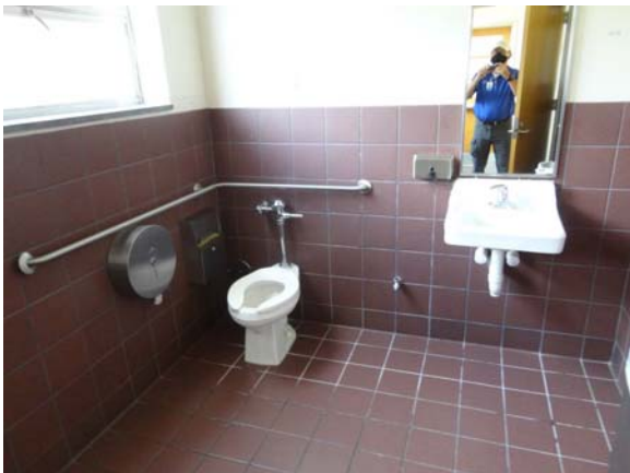
AUST012a 5/11/2021 Accessible two-fixture restroom Third floor, all-gender restroom
