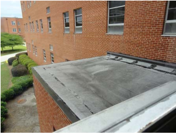
AUST031a 5/11/2021 Lower built-up roof South center of building
