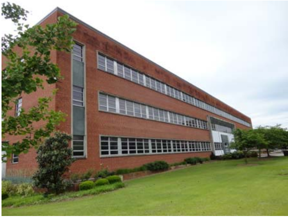
AUST044a 5/11/2021 Brick and glazing Northeast corner elevation
