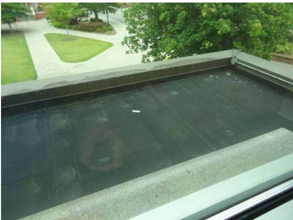
AUST027a 5/11/2021 Unballasted membrane roof Third floor, west elevator tower addition
