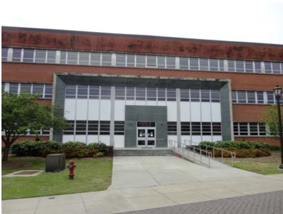
AUST045a 5/11/2021 Newer entry doors and stone accents North elevation
