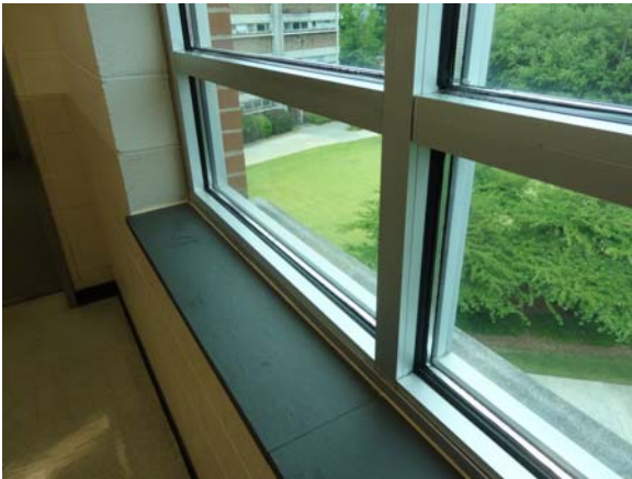
AUST026a 5/11/2021 Newer thermal-pane fixed glazing Third floor, west elevator tower addition
