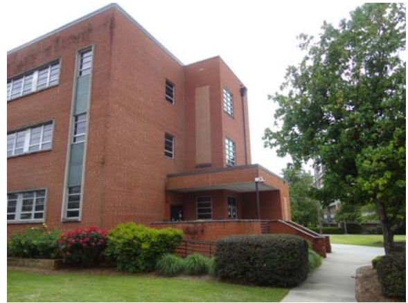
AUST048a 5/11/2021 Elevator tower addition West elevation
