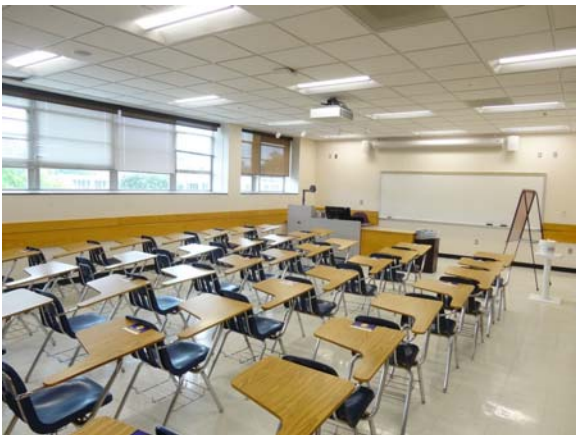
AUST024a 5/11/2021 Vinyl composite floor tile and lay-in acoustical ceiling Third floor, classroom
