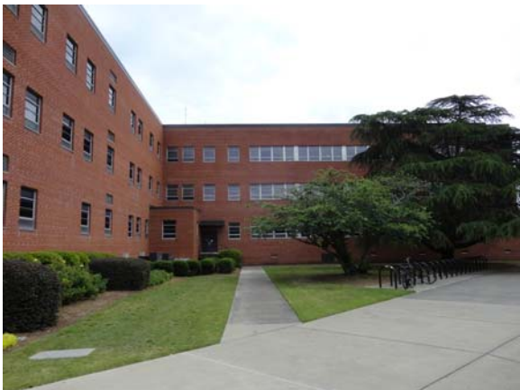
AUST051a 5/11/2021 Brick finishes and glazing Southwest elevation
