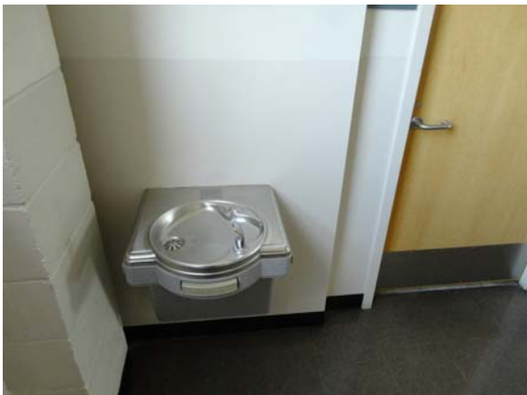
AUST006a 5/11/2021 Newer single-level water fountain Third floor corridor
