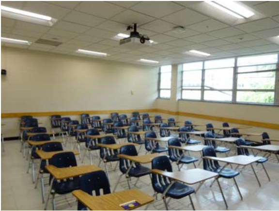
AUST016a 5/11/2021 Older vinyl composite floor tile and lay-in acoustical ceiling Third floor, classroom
