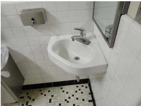
AUST021a 5/11/2021 Standard corner wall-hung lavatory Third floor, men's restroom
