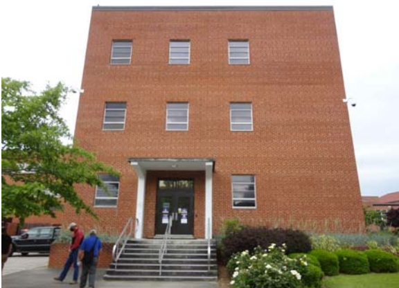
AUST042a 5/11/2021 Hollow-metal doors at end elevation East end elevation
