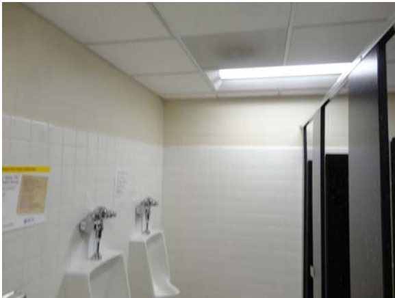
AUST011a 5/11/2021 Ceramic tile wainscot and acoustical ceiling Third floor, men's restroom
