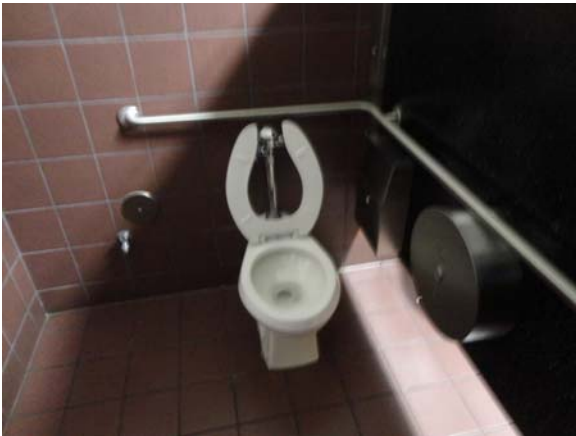
AUST038a 5/11/2021 Accessible toilet stall First floor, women's restroom
