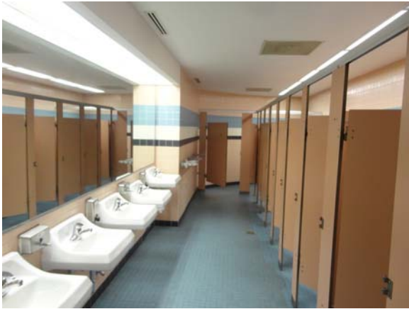
BATE040a 5/11/2021 Typical wall-hung lavatories Second floor, main women's restroom
