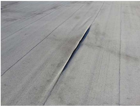
BATE004a 5/11/2021 Minor issue with cap sheet Main roof
