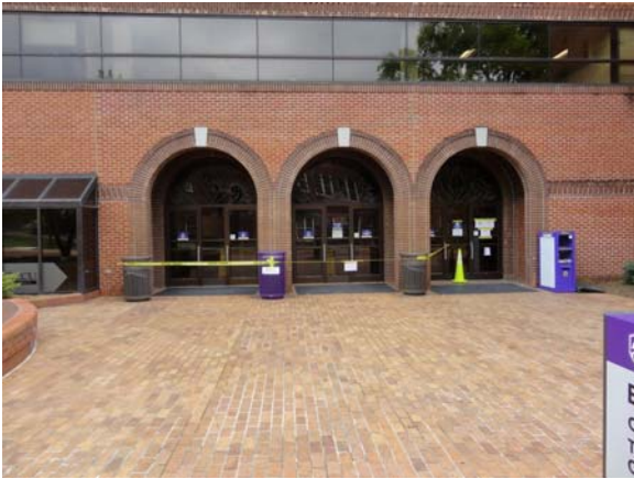
BATE067a 5/11/2021 Glass entry doors Northwest corner elevation
