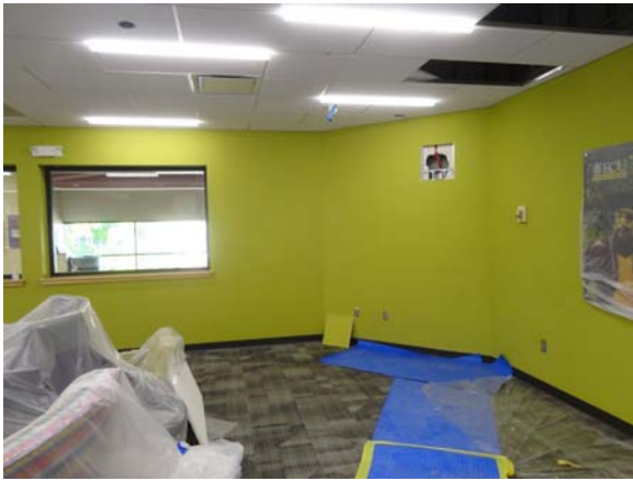
BATE008a 5/11/2021 Newer carpet tile and acoustical ceilings Third floor, select offices
