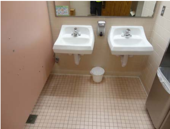
BATE023a 5/11/2021 Wall-hung lavatories Third floor, women's SE restroom
