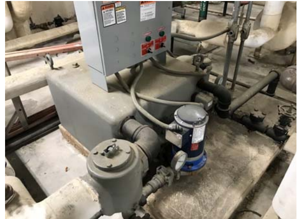
BATE022e 5/11/2021 Condensate receiver Room 1040A
