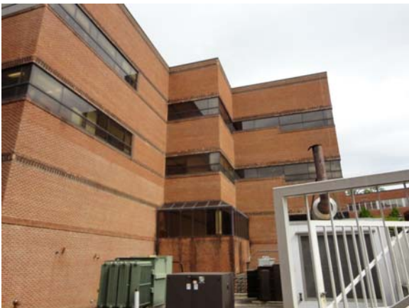
BATE059a 5/11/2021 Brick facades with bands of glazing Southeast corner elevation
