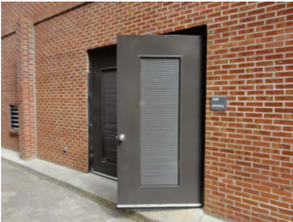
BATE057a 5/11/2021 Hollow-metal service doors First floor, mechanical area
