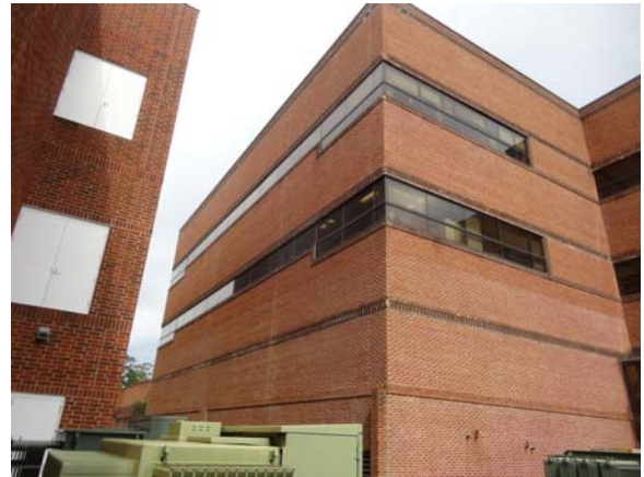
BATE058a 5/11/2021 Brick facades with bands of glazing Corner elevation
