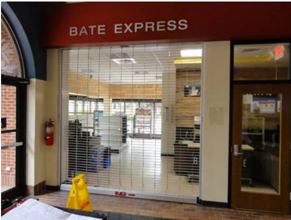
BATE051a 5/11/2021 Roll down shutter for food service area First floor, Bate Express
