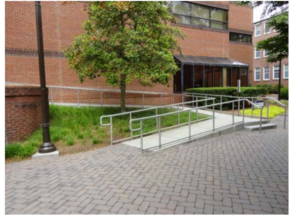
BATE062a 5/11/2021 Ramped access to building Northeast elevation
