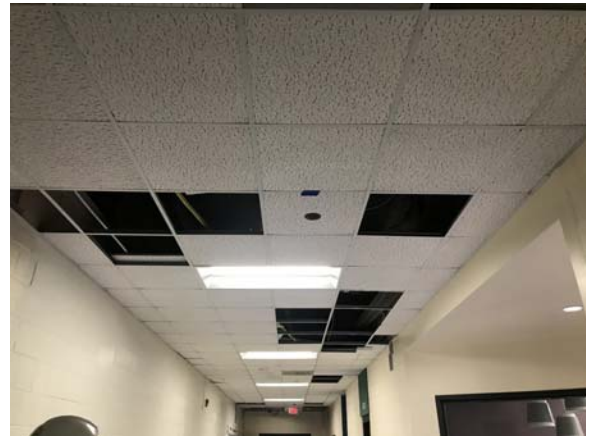
BATE005e 5/11/2021 Recessed LED lighting fixtures Third floor corridor
