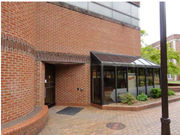
BATE065a 5/11/2021 On-grade building entry with power door assist Northwest elevation
