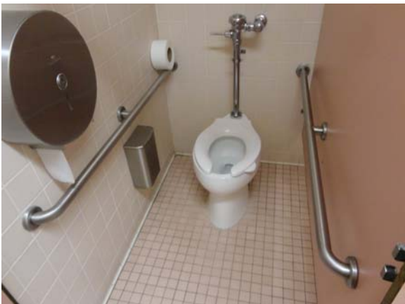
BATE024a 5/11/2021 Partially accessible toilet stall Third floor, women's SE restroom
