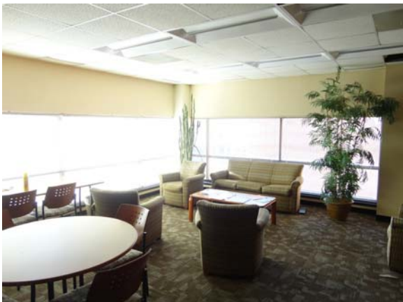
BATE018a 5/11/2021 Newer carpet tile and acoustical ceiling Third floor, staff lounge
