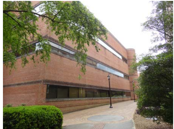
BATE064a 5/11/2021 Brick facades with bands of glazing North elevation
