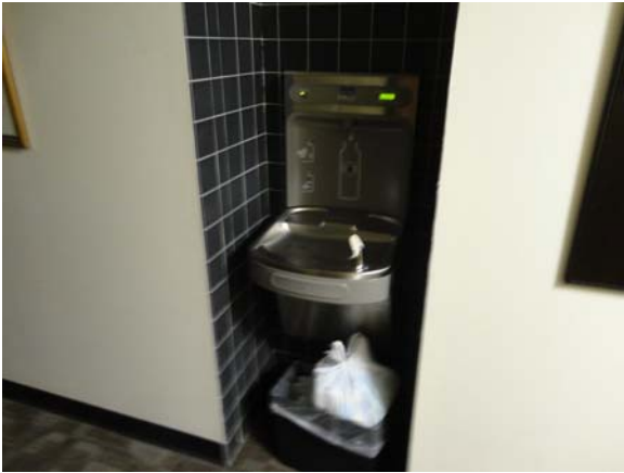
BATE028a 5/11/2021 Newer single-level water fountain with bottle filler Third floor corridor
