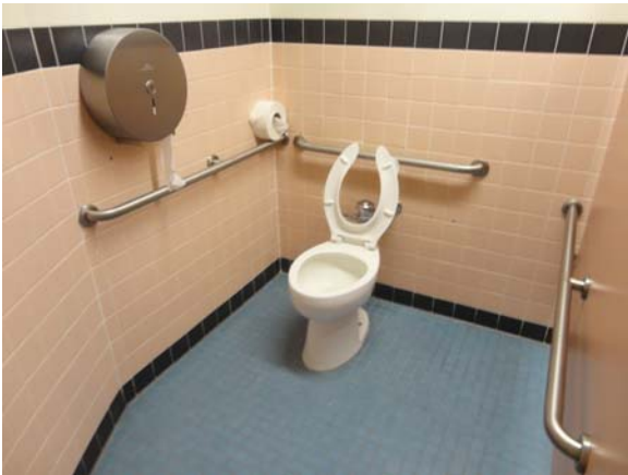
BATE032a 5/11/2021 Accessible toilet stall Third floor, main women's restroom
