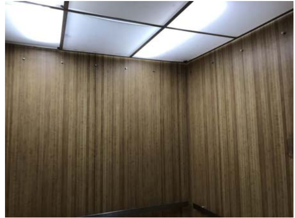
BATE013e 5/11/2021 Elevator interior Elevator 1
