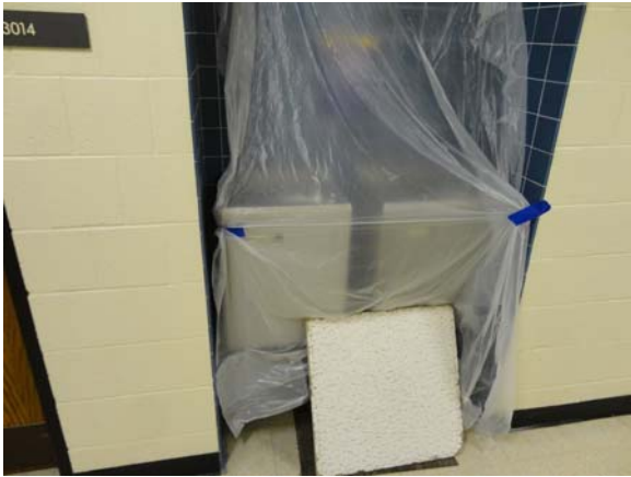
BATE025a 5/11/2021 Two water fountains mounted as same height Third floor corridor
