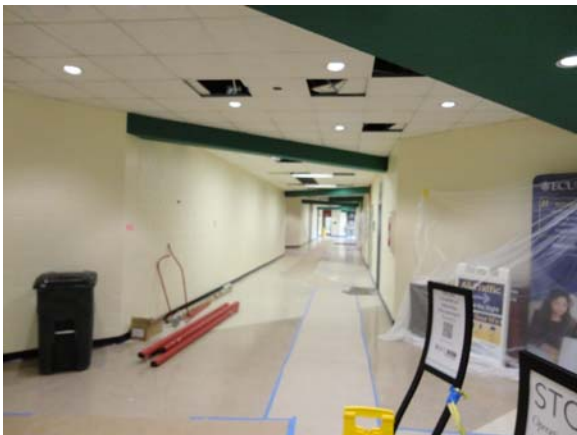
BATE039a 5/11/2021 Older vinyl flooring and acoustical ceiling Second floor corridor
