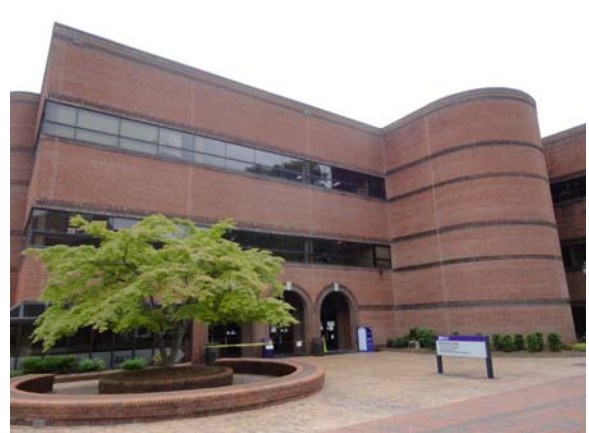
BATE066a 5/11/2021 Main plaza entry Northwest elevation
