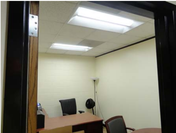
BATE014a 5/11/2021 Older acoustical ceiling Third floor, office
