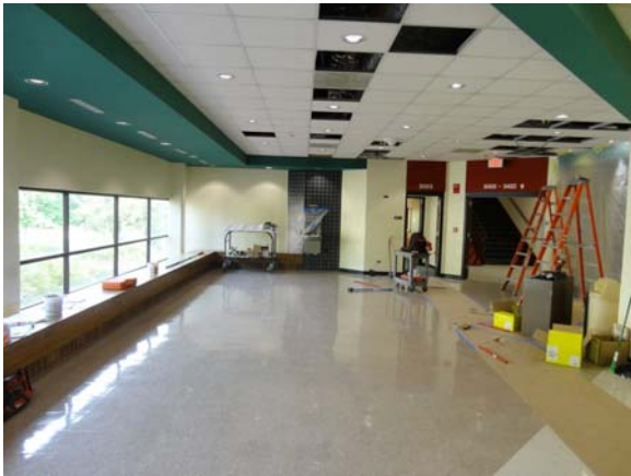
BATE041a 5/11/2021 Older vinyl flooring and acoustical ceiling Second floor, commons
