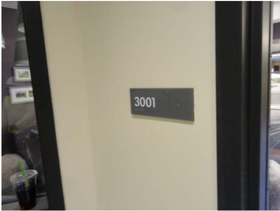
BATE007a 5/11/2021 Accessible wall-mounted room signage Third floor corridor
