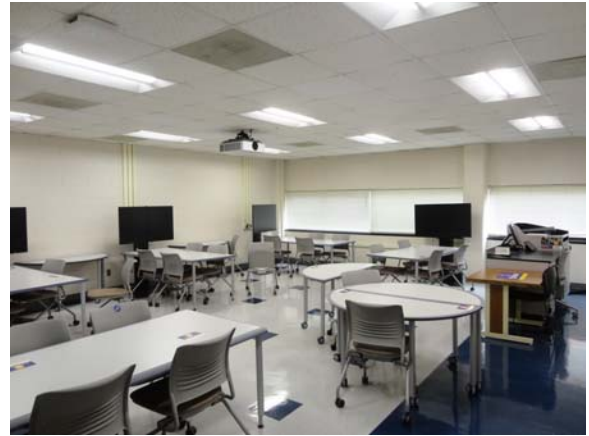
BATE044a 5/11/2021 Older VCT and acoustical ceiling Second floor, class lab
