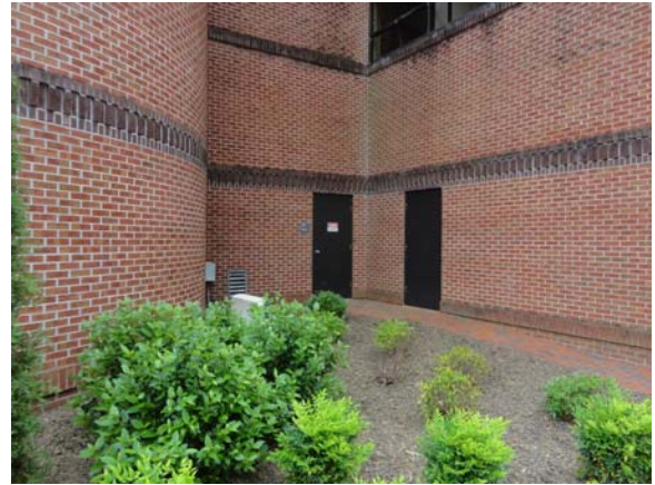
BATE068a 5/11/2021 Hollow-metal service doors West elevation
