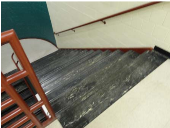
BATE027a 5/11/2021 Upgraded rubber stair treads Third floor, stair tower
