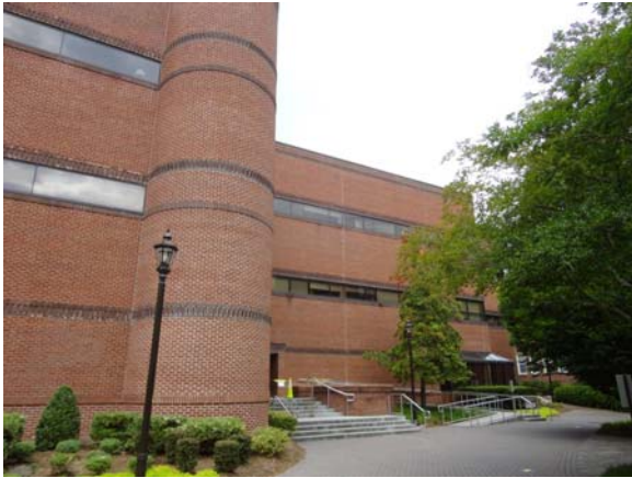
BATE061a 5/11/2021 Brick facades with bands of glazing Northeast elevation
