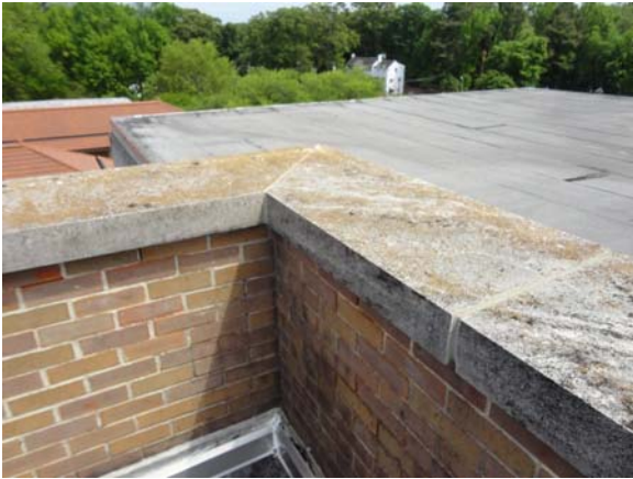
BREW010a 5/12/2021 Cut stone parapet cap Breezeway roof
