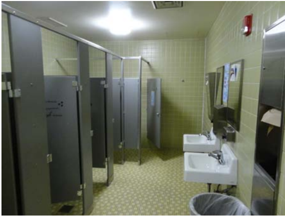
BREW040a 5/12/2021 Standard wall-hung lavatories and toilet stalls D Wing, first floor women's restroom
