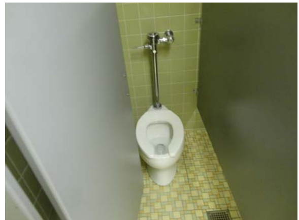
BREW078a 5/12/2021 Older standard toilet stall A Wing, first floor women's restroom
