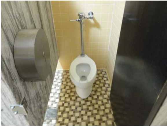
BREW019a 5/12/2021 Standard tankless water closet B Wing, third floor men's restroom
