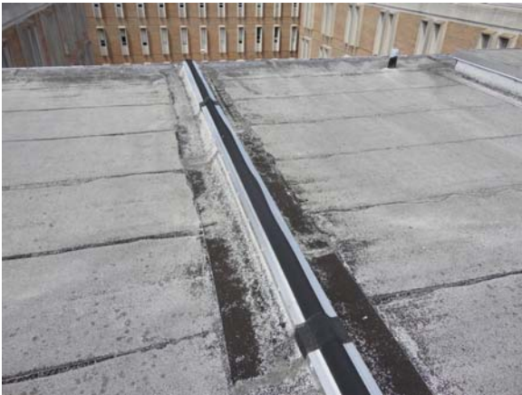
BREW005a 5/12/2021 Roof expansion joint A Wing roof
