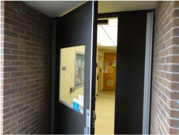
BREW070a 5/12/2021 Newer 1-1/2 exterior entry door A Wing, fourth floor
