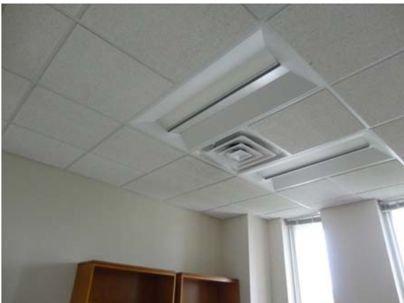
BREW060a 5/12/2021 Newer acoustical ceiling D Wing, third floor office
