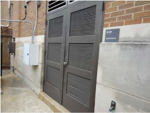
BREW091a 5/12/2021 Two louvered hollow-metal service doors Wing B, west mechanical area
