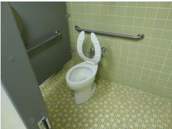
BREW077a 5/12/2021 Accessible toilet stall A Wing, first floor women's restroom
