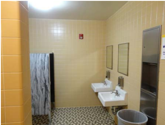
BREW020a 5/12/2021 Ceramic floor and wall tile and painted ceiling B Wing, third floor men's restroom
