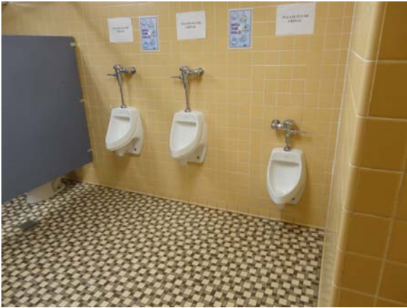
BREW046a 5/12/2021 Accessible newer urinals D Wing, first floor men's restroom
