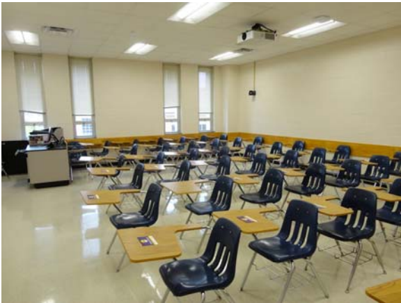
BREW053a 5/12/2021 Older vinyl flooring and acoustical ceiling D Wing, third floor classroom
