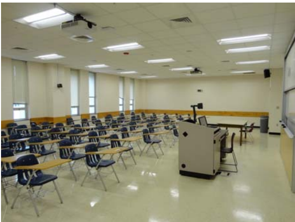
BREW048a 5/12/2021 Older vinyl floor tile and acoustical ceiling D Wing, second floor classroom
