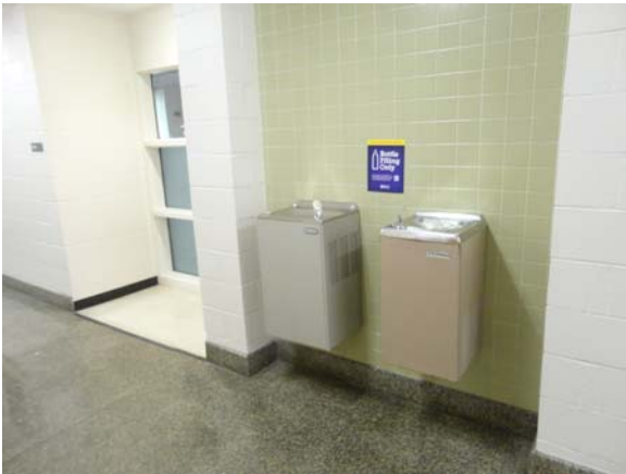
BREW023a 5/12/2021 Two older partially accessible water fountains B Wing, third floor corridor
