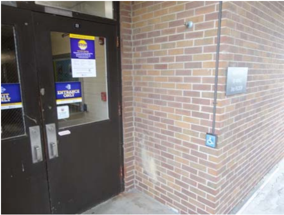
BREW025a 5/12/2021 Older, power-assisted door operator B Wing, third floor entry
