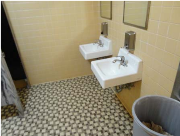
BREW017a 5/12/2021 Older wall-hung lavatories B Wing, third floor men's restroom
