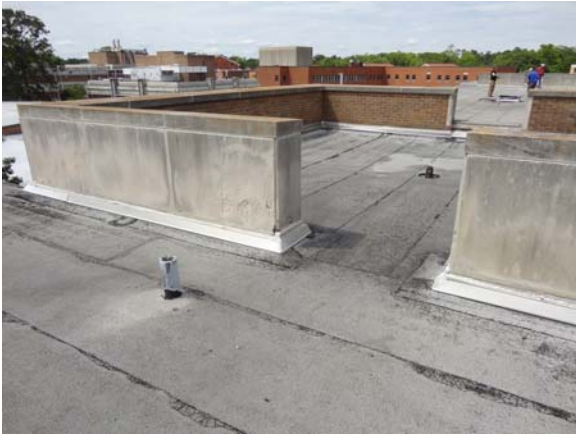
BREW011a 5/12/2021 Localized cut stone weathering Breezeway roof
