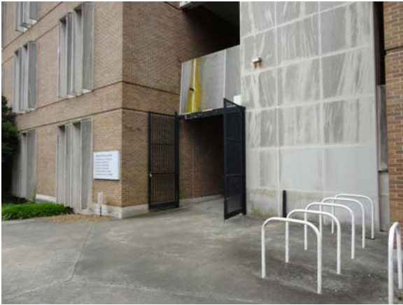
BREW085a 5/12/2021 Metal gate at each courtyard entry West courtyard entry
