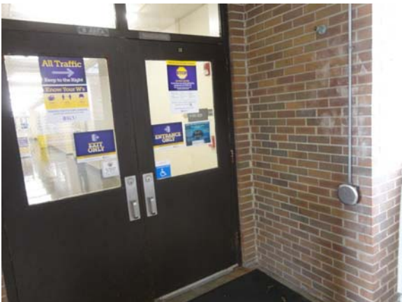
BREW015a 5/12/2021 Hollow-metal entry doors with power assist B Wing, third floor entry
