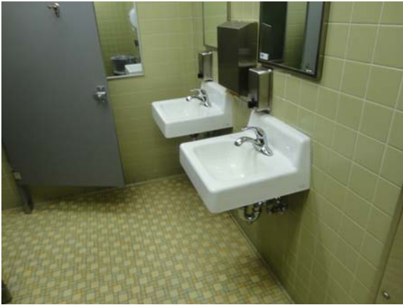
BREW079a 5/12/2021 Partially accessible wall-hung lavatories A Wing, first floor women's restroom
