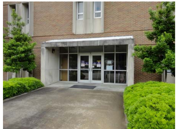
BREW090a 5/12/2021 Glass entry doors A Wing, main south entry
