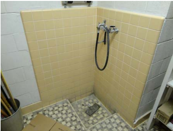
BREW002a 5/12/2021 Original ceramic tile floor service sink B Wing, janitor's closet
