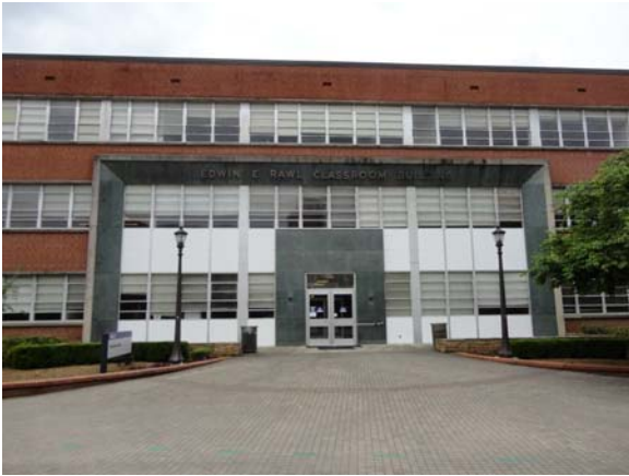
RAWL061a 5/10/2021 On-grade access to main entry Main north building entry
