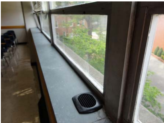
RAWL009a 5/10/2021 Original single-pane glazing Third floor glazing
