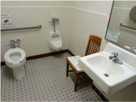
RAWL013a 5/10/2021 Three-fixture accessible restroom Third floor all-gender restroom
