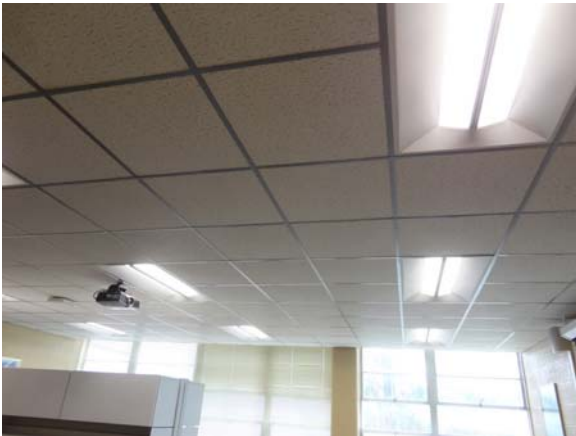
RAWL026a 5/10/2021 Acoustical lay-in ceiling Second floor classroom
