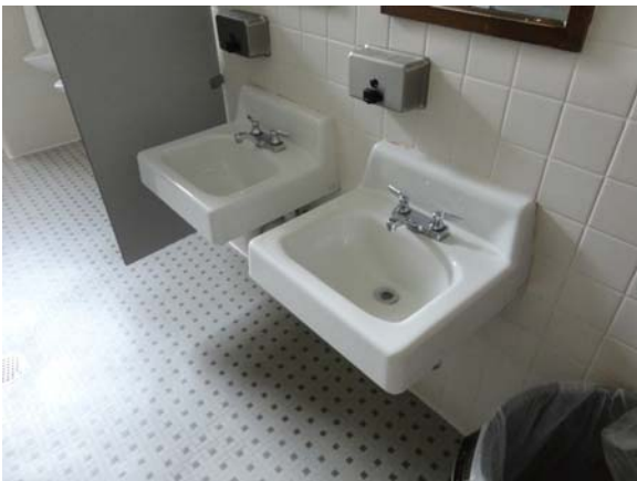
RAWL015a 5/10/2021 Two older wall-mounted sinks Third floor men's restroom
