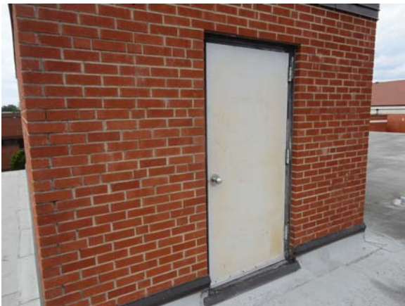
RAWL003a 5/10/2021 Hollow metal roof access door Main roof
