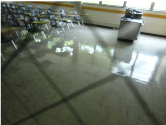
RAWL027a 5/10/2021 9x9 vinyl flooring Second floor classroom
