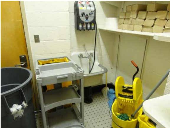
RAWL020a 5/10/2021 Typical original wall-mounted service sink Second floor janitors closet
