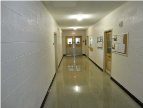
RAWL031a 5/10/2021 9x9 vinyl flooring and textured ceiling First floor corridor
