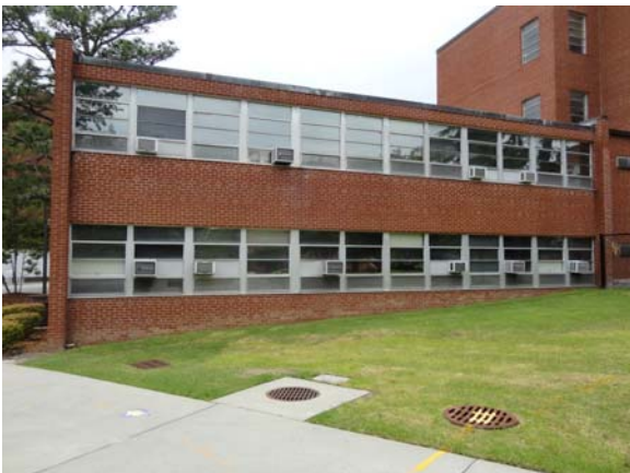
RAWL053a 5/10/2021 Exterior finishes East elevation of south annex wing
