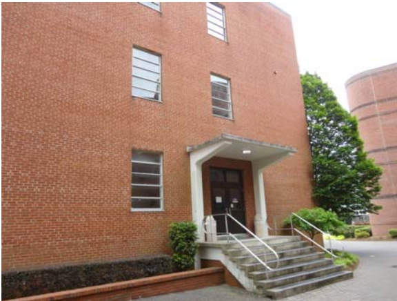
RAWL063a 5/10/2021 Secondary entry/egress with accessible handrails West entry
