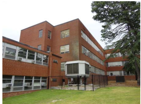
RAWL054a 5/10/2021 Exterior finishes Southeast corner of main building
