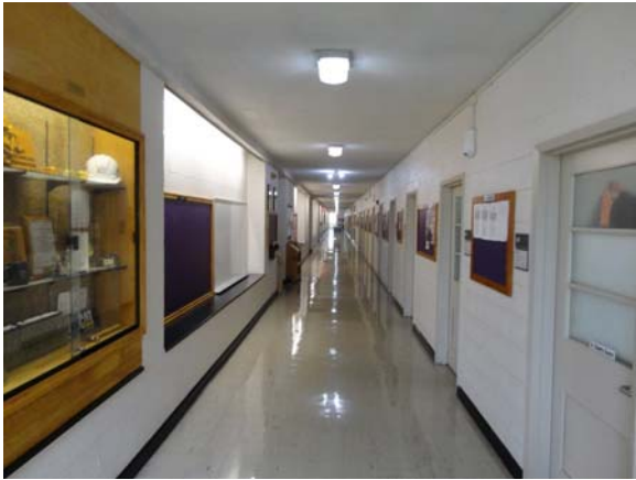
RAWL005a 5/10/2021 9x9 vinyl floor tile and textured ceiling Third floor corridor
