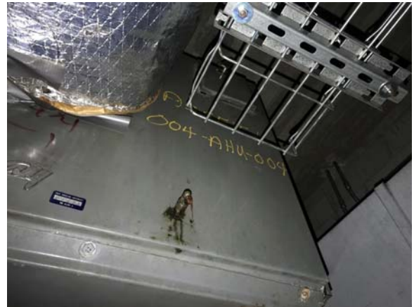
RAWL029e 5/10/2021 Fan coil unit AHU-004 Room 009
