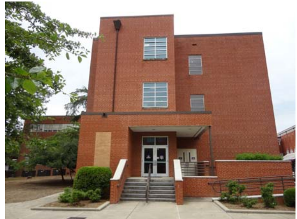
RAWL058a 5/10/2021 End elevation, noting new glazing on elevator tower East elevation
