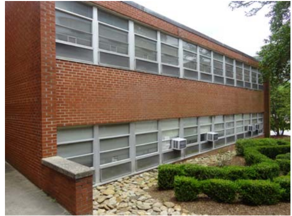
RAWL050a 5/10/2021 Exterior finishes West elevation of south annex wing
