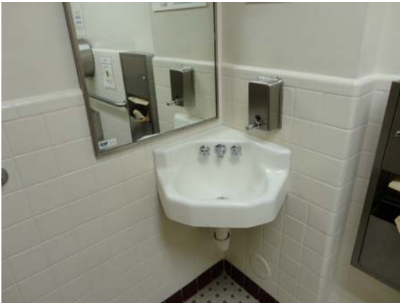
RAWL011a 5/10/2021 Nonaccessible corner wall sink Third floor all-gender restroom
