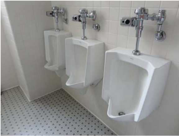
RAWL016a 5/10/2021 Three newer wall-mounted urinals Third floor men's restroom
