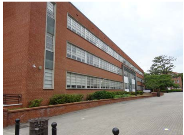
RAWL060a 5/10/2021 Exterior corner elevation Northeast corner elevation
