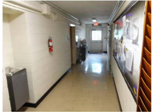
RAWL044a 5/10/2021 9x9 vinyl floor tile and textured ceiling Annex basement corridor
