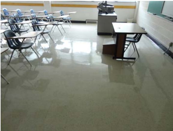
RAWL029a 5/10/2021 Newer vinyl composite floor tile First floor classroom
