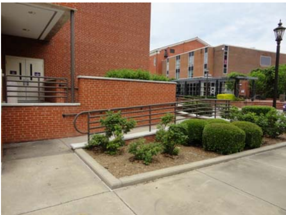
RAWL059a 5/10/2021 Accessible entry ramp East elevation
