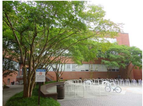
RAWL064a 5/10/2021 Exterior finishes West elevation of south main building
