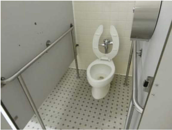
RAWL034a 5/10/2021 Partially accessible toilet stall First floor men's restroom
