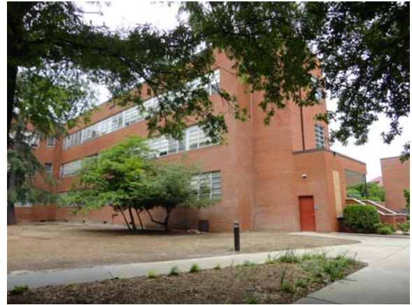
RAWL056a 5/10/2021 Hollow metal service door East elevator tower mechanical room
