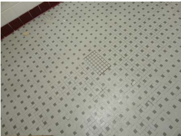
RAWL012a 5/10/2021 Dissimilar ceramic tile floor repair Third floor all-gender restroom
