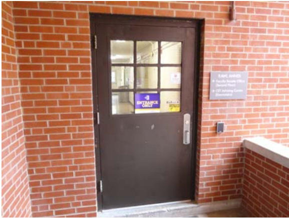
RAWL043a 5/10/2021 Hollow metal entry door Annex first floor north entry
