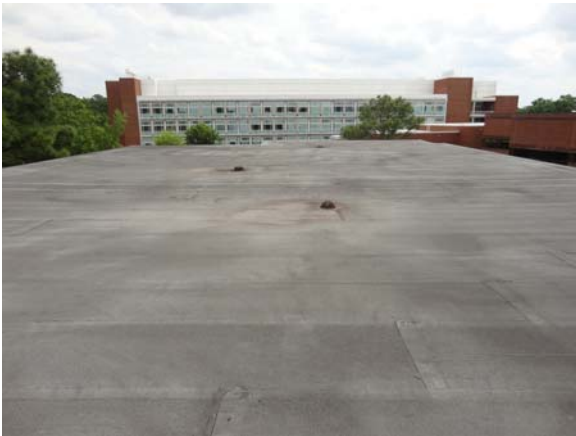
RAWL002a 5/10/2021 Main built-up roof Main roof
