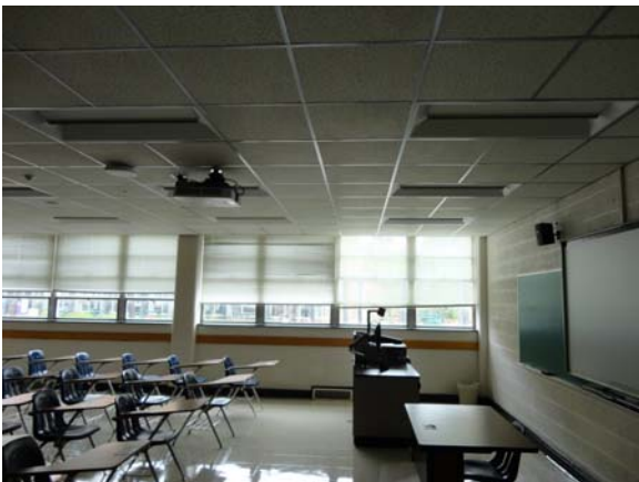
RAWL030a 5/10/2021 Newer lay-in acoustical ceiling First floor classroom
