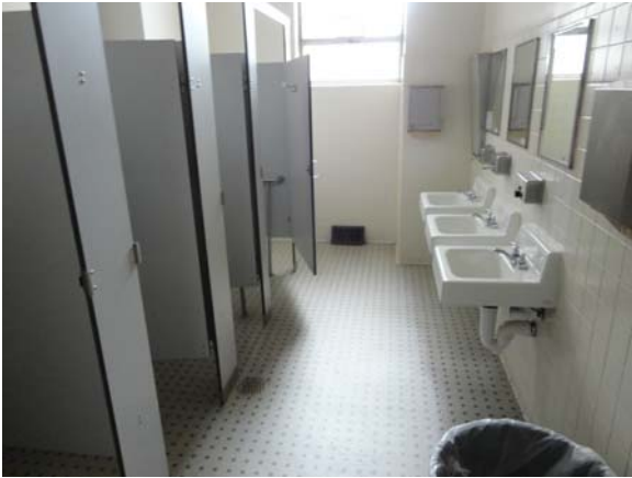
RAWL037a 5/10/2021 Typical finishes in restroom First floor women's restroom
