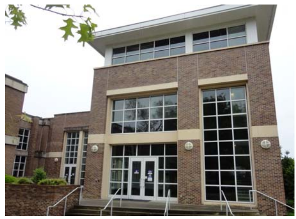
RIVW037a 5/12/2021 Brick veneer and cast stone accents West end of north elevation
