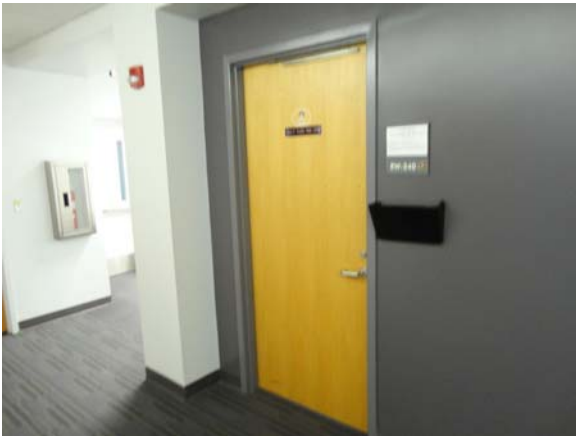
RIVW008a 5/12/2021 Flush wood door with lever hardware and accessible signage Third floor corridor
