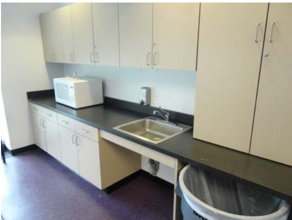
RIVW030a 5/12/2021 Casework First floor, student lounge
