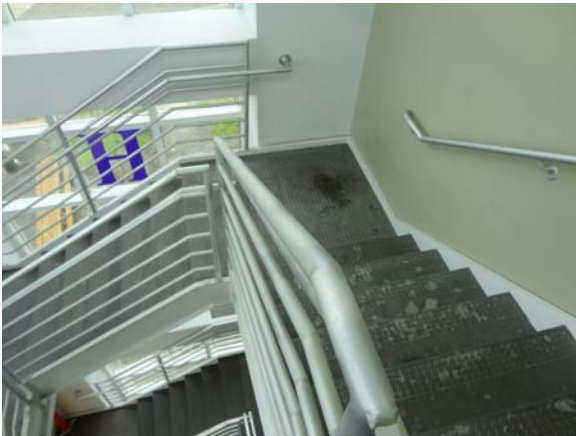
RIVW005a 5/12/2021 Stair tread finishes and painted walls Stair tower
