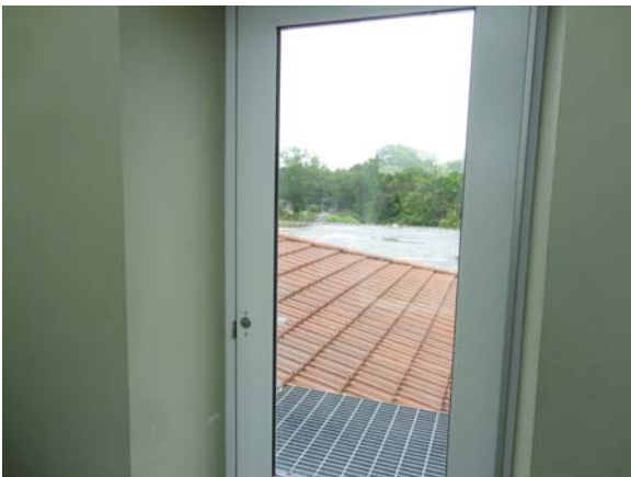
RIVW006a 5/12/2021 Glass roof access door Corner stair tower
