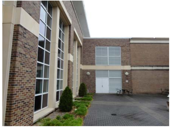
RIVW047a 5/12/2021 Double hollow-metal service doors Southeast corner elevation
