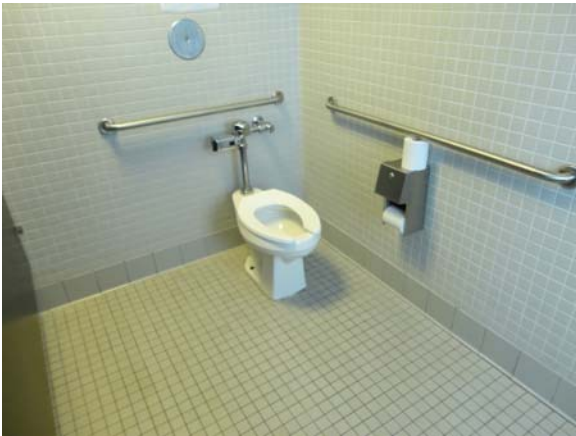
RIVW014a 5/12/2021 Accessible toilet stall Third floor, women's restroom
