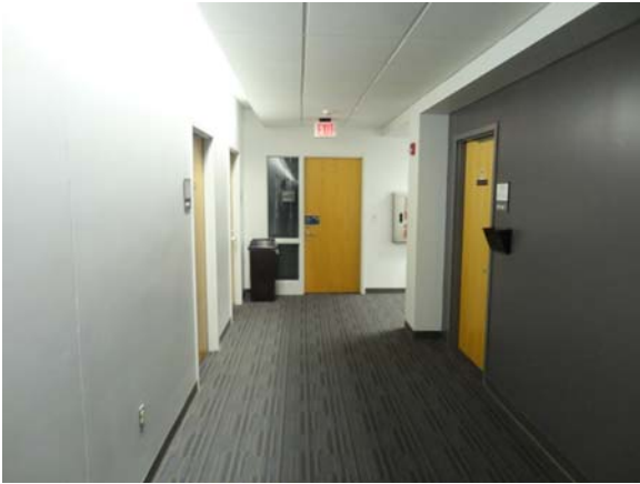
RIVW007a 5/12/2021 Broadloom carpet and acoustical ceiling Third floor corridor
