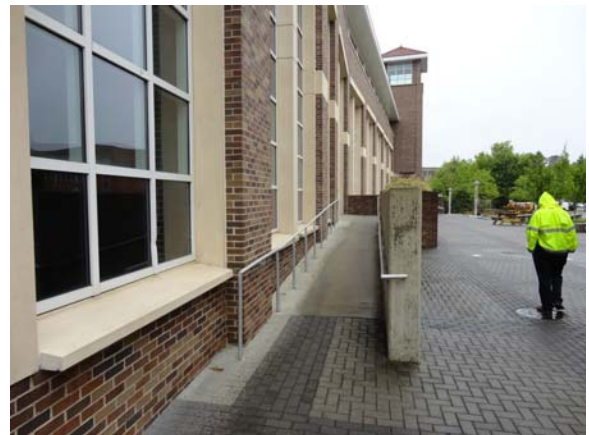
RIVW039a 5/12/2021 Ramped access to building West elevation
