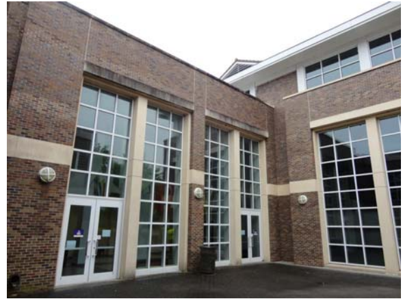
RIVW035a 5/12/2021 Glass doors and fixed glazing East end of north elevation
