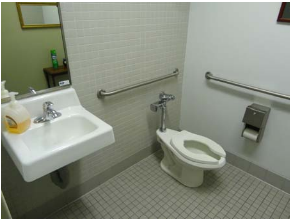
RIVW026a 5/12/2021 Accessible two-fixture restroom Second floor, Dean's suite office
