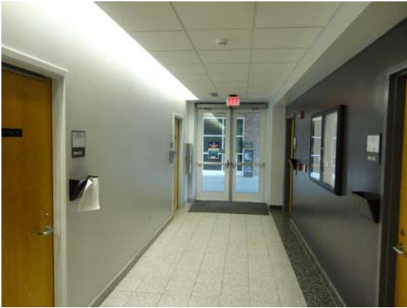
RIVW031a 5/12/2021 Terrazzo floor tile and acoustical ceiling First floor corridor
