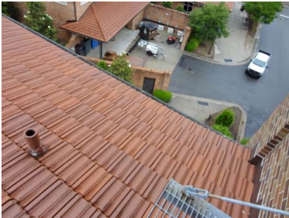
RIVW002a 5/12/2021 Clay tile roof Main roof
