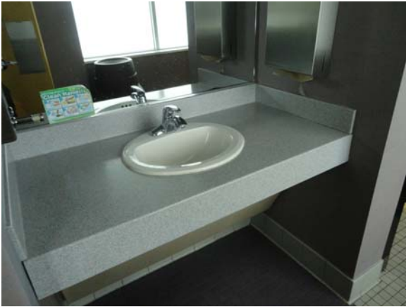
RIVW013a 5/12/2021 Counter lavatory Third floor, women's restroom
