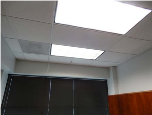
RIVW016a 5/12/2021 Acoustical lay-in ceiling Third floor, office
