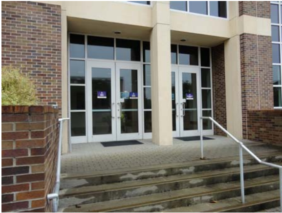
RIVW040a 5/12/2021 Glass entry doors West elevation
