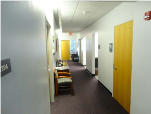
RIVW028a 5/12/2021 Carpeting and acoustical ceiling Second floor, Dean's suite office
