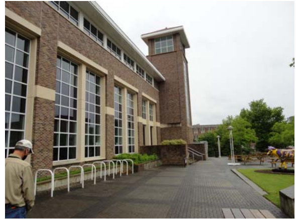
RIVW041a 5/12/2021 Stair tower Southwest elevation
