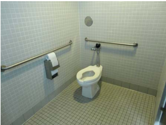
RIVW012a 5/12/2021 Accessible toilet stall Third floor, men's restroom
