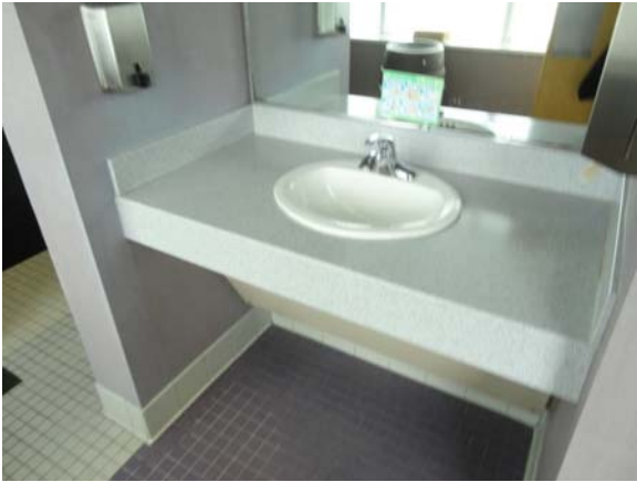
RIVW010a 5/12/2021 Counter lavatory Third floor, men's restroom
