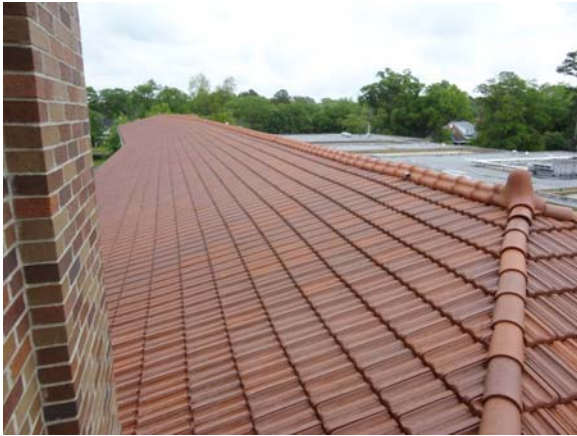
RIVW001a 5/12/2021 Clay tile roof ridge line Main roof
