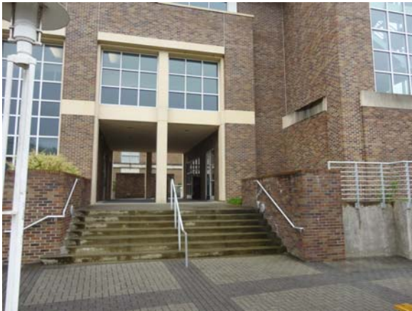
RIVW042a 5/12/2021 Accessible rails on breezeway passage South end of west elevation
