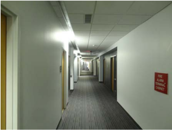
RIVW019a 5/12/2021 Broadloom carpeting and acoustical ceiling Second floor corridor
