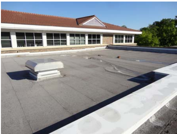
RIVW003a 5/12/2021 Lower built-up roof Lower east roof
