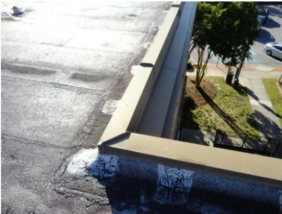
RIVE002a 5/13/2021 Low parapet with continuous metal cap Main roof
