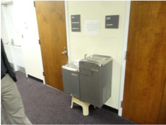
RIVE052a 5/13/2021 Older two-level water fountain First floor, south daycare area
