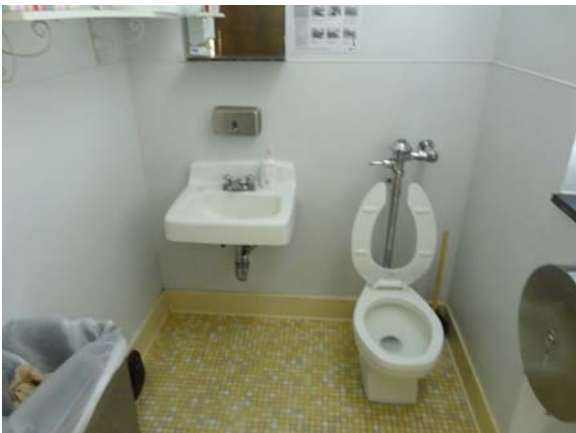
RIVE042a 5/13/2021 Older standard fixtures First floor, south unisex restroom
