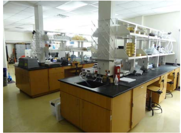
RIVE068a 5/13/2021 Standard wood lab cabinetry with vinyl floor tile First floor, engineering lab
