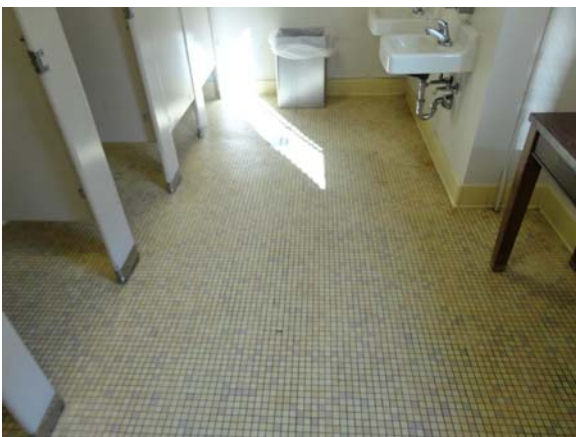
RIVE015a 5/13/2021 Older 1x1 ceramic floor tile Second floor, south women's restroom
