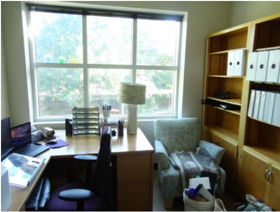
RIVE040a 5/13/2021 Newer exterior glazing in select areas Second floor, office
