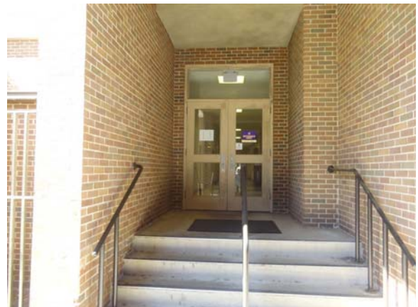
RIVE078a 5/13/2021 Typical metal and glass corridor egress doors First floor, entry/egress
