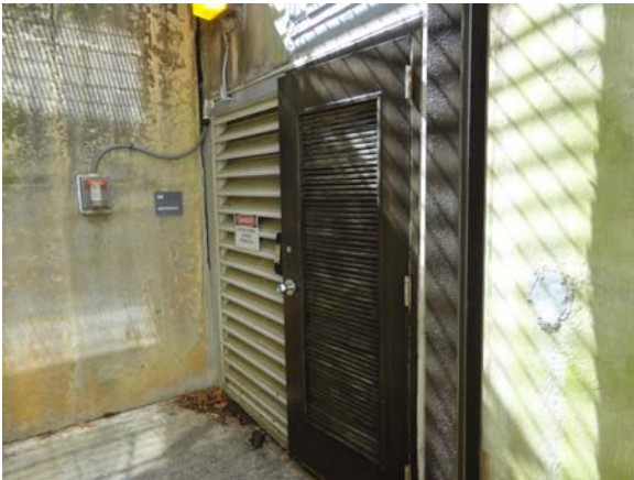
RIVE075a 5/13/2021 Hollow-metal louvered service door Courtyard areaway
