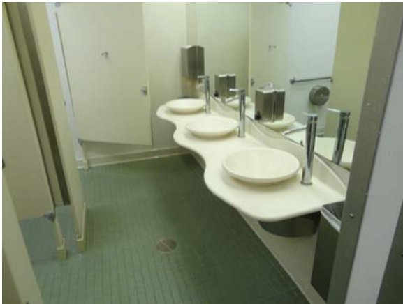
RIVE053a 5/13/2021 Three new accessible counter lavatories First floor, central women's restroom
