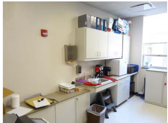
RIVE072a 5/13/2021 Older casework and sink First floor, north office area
