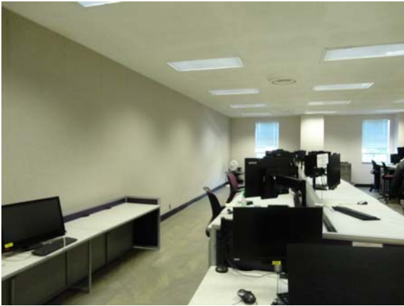
RIVE025a 5/13/2021 Newer LVT flooring but original textured ceiling Second floor, south computer labs
