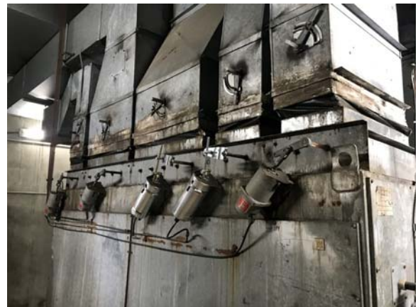
RIVE039e 5/13/2021 Zoned deck for air handling unit AHU-001 Room 02
