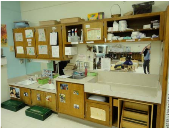
RIVE044a 5/13/2021 Older casework in toddler's dayroom First floor, south daycare area
