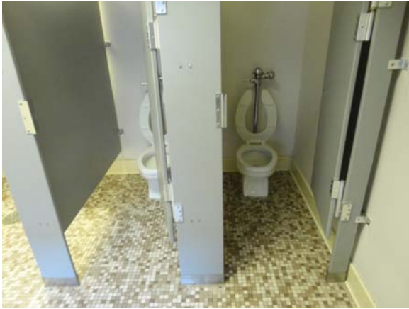
RIVE037a 5/13/2021 Older standard toilet stalls Second floor, central women's restroom
