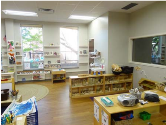
RIVE049a 5/13/2021 Newer sheet vinyl flooring First floor, south daycare area
