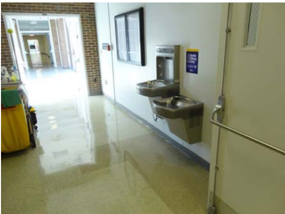
RIVE012a 5/13/2021 Older vinyl floor tile but newer dual-level water fountain Second floor corridor
