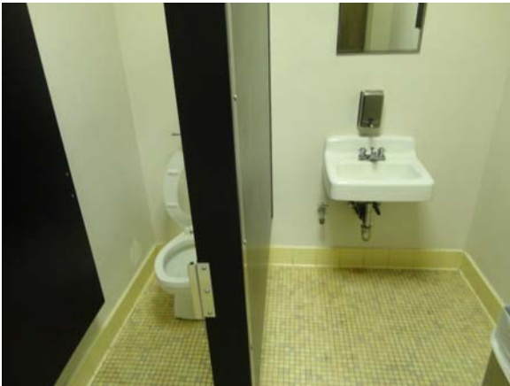
RIVE032a 5/13/2021 Older standard fixtures Second floor, central men's restroom
