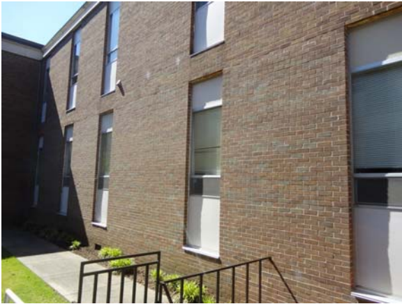
RIVE079a 5/13/2021 Single-pane glazing Courtyard
