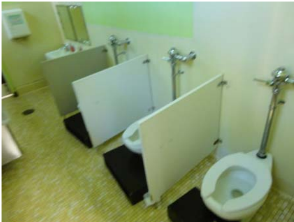
RIVE050a 5/13/2021 Three children's water closets and two wall-hung lavatories First floor, south daycare area
