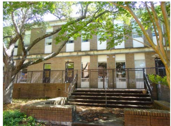
RIVE084a 5/13/2021 Brick, precast banding, and single-pane glazing South elevation
