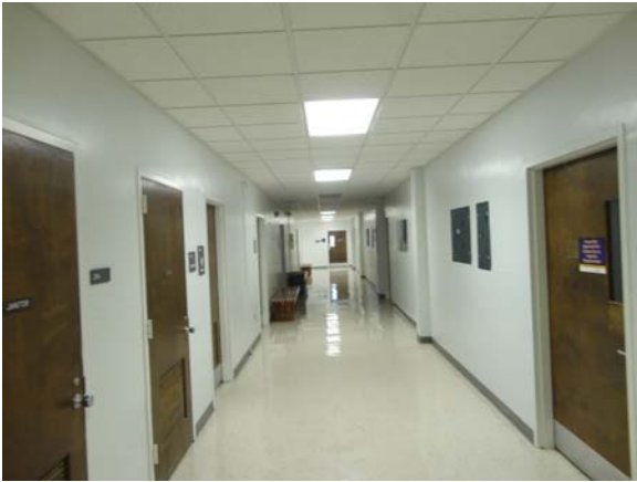
RIVE013a 5/13/2021 Older vinyl tile and suspected ACM above acoustical ceiling Second floor, south corridor
