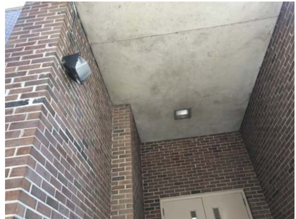
RIVE053e 5/13/2021 HID wallpack and recessed can exterior fixtures Entry
