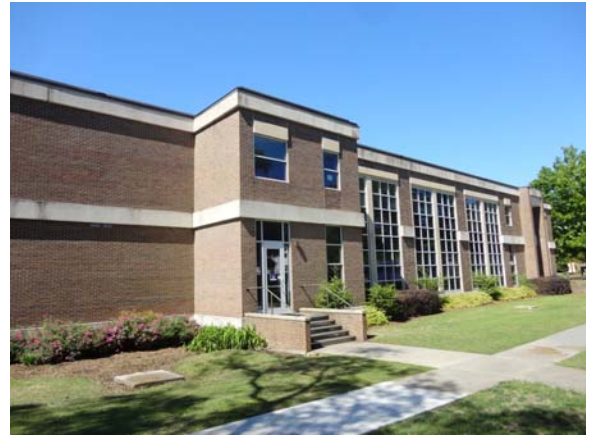
RIVE086a 5/13/2021 Brick, precast banding, and single-pane glazing East end elevation
