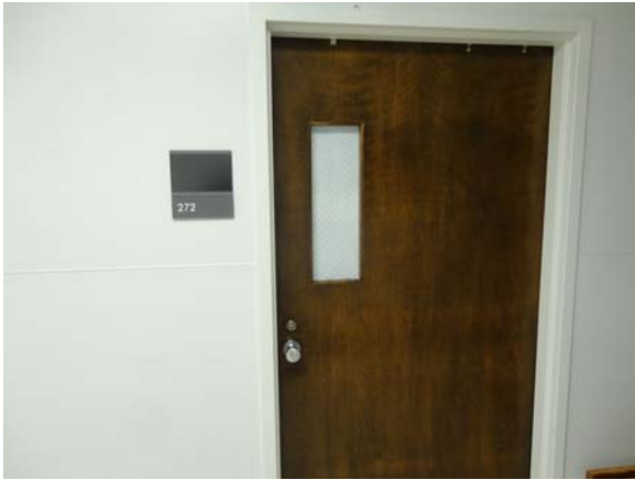
RIVE022a 5/13/2021 Original doors with knob hardware Second floor corridor
