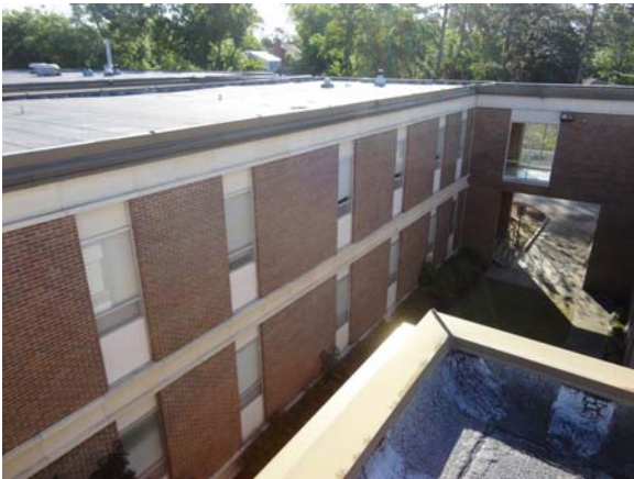
RIVE005a 5/13/2021 Brick facade and original single-pane glazing Typical courtyard exterior
