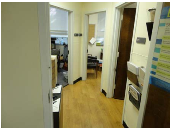
RIVE051a 5/13/2021 Newer sheet vinyl flooring in offices First floor, south daycare area
