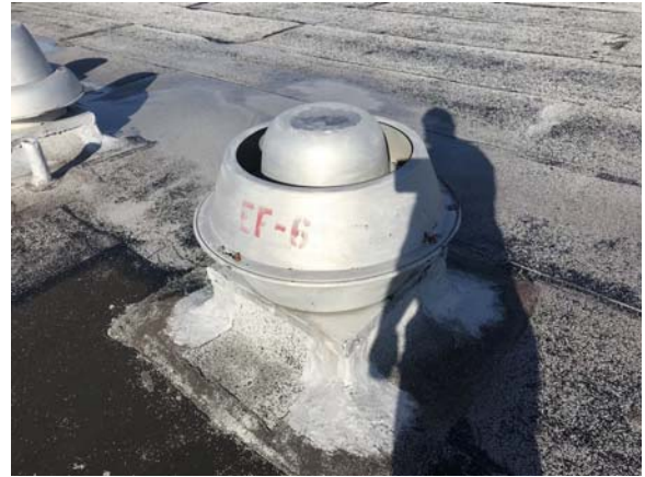
RIVE004e 5/13/2021 Centrifugal rooftop exhaust fan Roof
