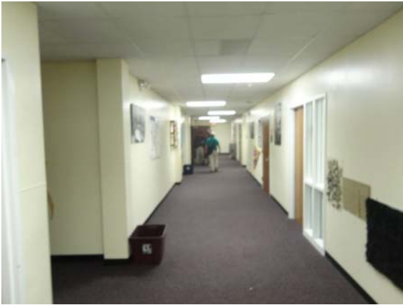
RIVE043a 5/13/2021 Broadloom carpeting and acoustical ceiling First floor, south daycare area
