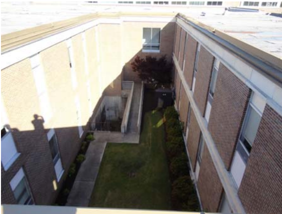
RIVE008a 5/13/2021 View of areaway in one of the courtyards Exterior courtyard
