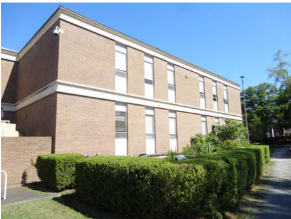
RIVE077a 5/13/2021 Brick, precast banding, and single-pane glazing Northeast corner elevation
