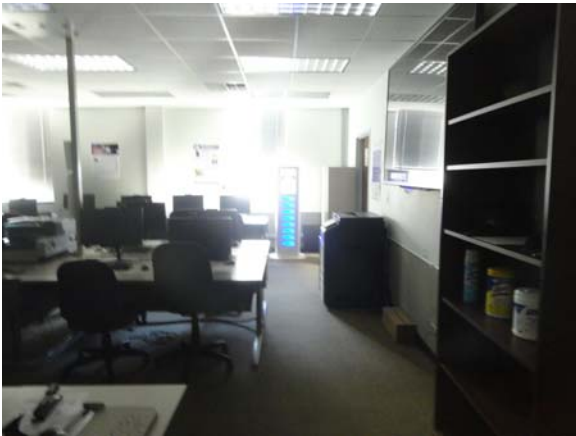
RIVE026a 5/13/2021 Older broadloom carpeting and 2x2 acoustical ceiling Second floor, computer lab
