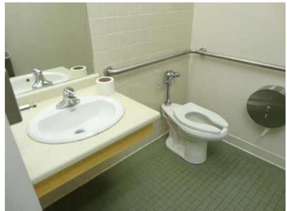
RIVE090a 5/13/2021 New accessible two-fixture unisex restroom First floor, restroom upgrade
