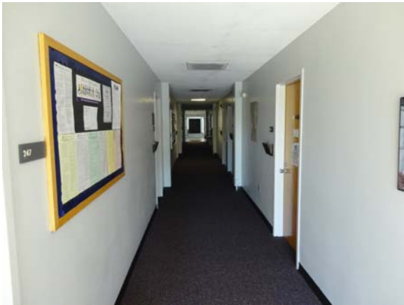
RIVE035a 5/13/2021 Older broadloom carpeting and textured ceiling Second floor, north office corridor
