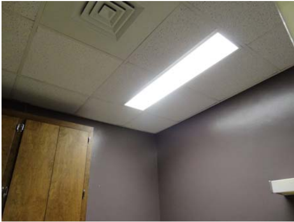
RIVE046a 5/13/2021 Acoustical ceiling First floor, south daycare area
