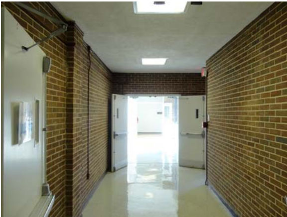
RIVE011a 5/13/2021 Exterior doors to breezeway link Second floor corridor
