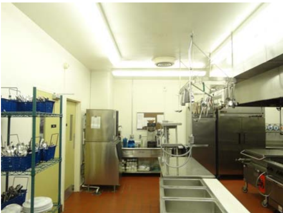
RIVE057a 5/13/2021 Quarry tile floor and painted ceiling First floor, east Culinary area
