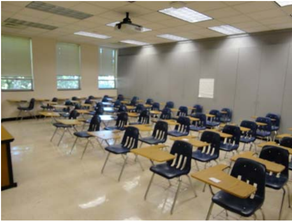
RIVE019a 5/13/2021 Older vinyl floor tile and older acoustical ceiling Second floor, classroom
