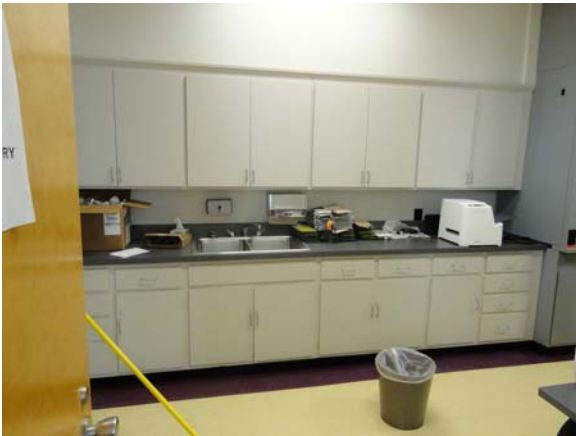
RIVE069a 5/13/2021 New casework and sink First floor, office area
