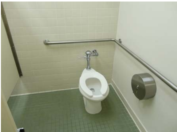
RIVE054a 5/13/2021 Accessible toilet stall First floor, central women's restroom
