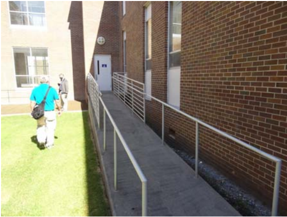
RIVE073a 5/13/2021 Ramp and railing to secondary egress Courtyard
