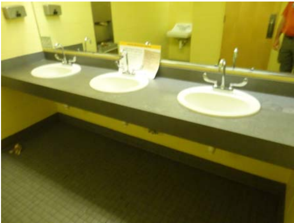
SCIT071a 5/10/2021 Counter lavatories North classroom wing men's restroom
