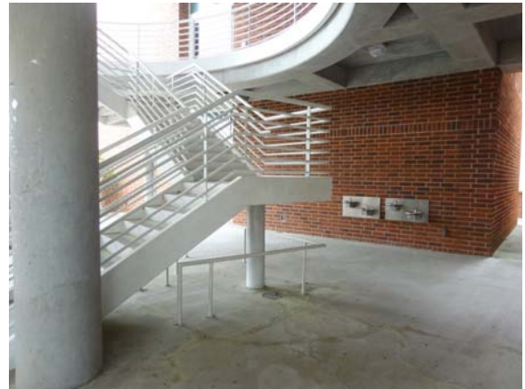
SCIT086a 5/10/2021 Cane guard at breezeway stair Breezeway link to classroom building
