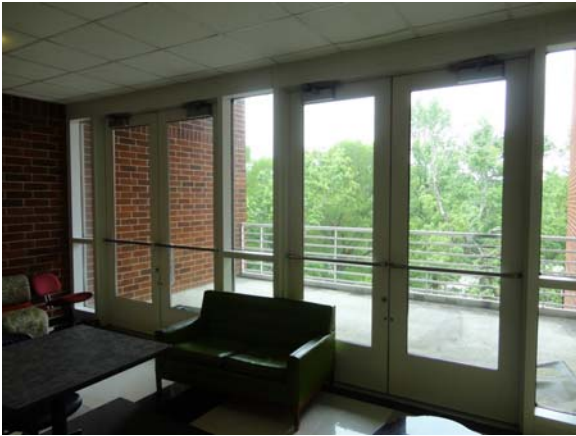
SCIT034a 5/10/2021 Exterior glass door off balcony area Fifth floor, southwest balcony
