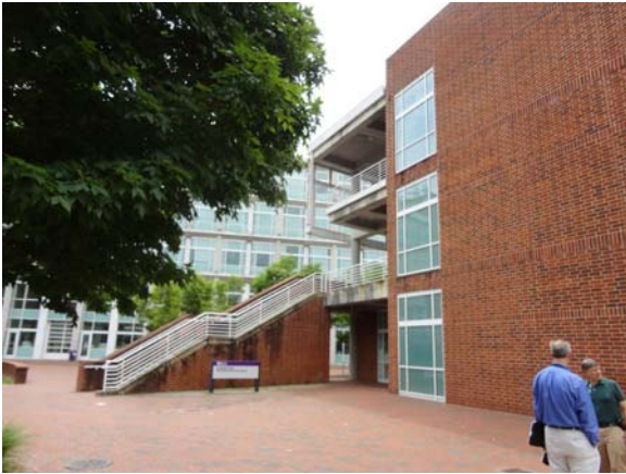
SCIT095a 5/10/2021 Exterior brick facade East elevation of north wing
