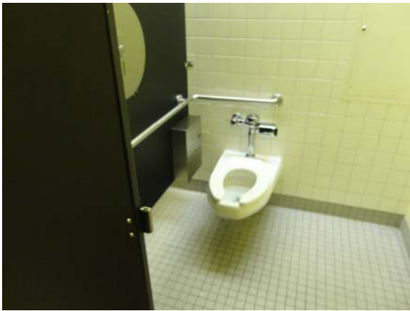
SCIT019a 5/10/2021 Accessible toilet stall Fifth floor, west women's restroom
