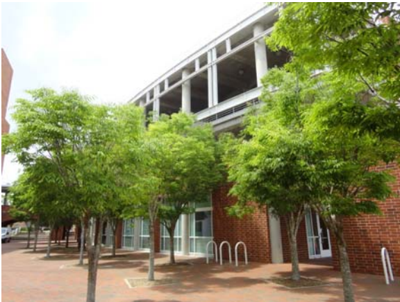
SCIT097a 5/10/2021 Curved exterior masonry facade South elevation of north wing
