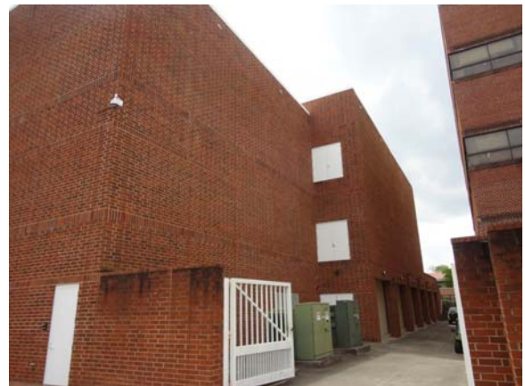
SCIT094a 5/10/2021 Exterior brick facade North elevation of north wing
