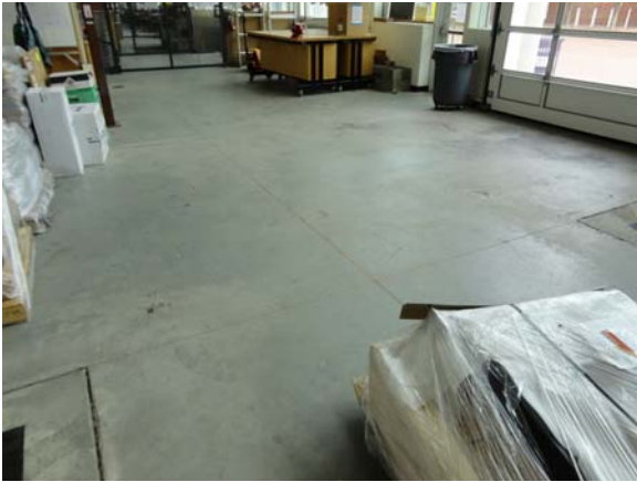
SCIT058a 5/10/2021 Concrete floor in high bay First floor, ITEC high bay
