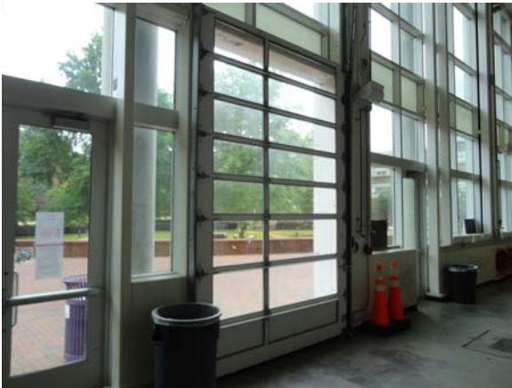
SCIT059a 5/10/2021 Sectional overhead door First floor, ITEC high bay
