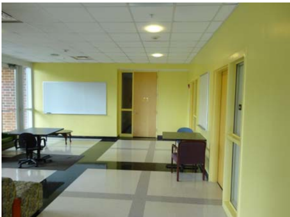
SCIT015a 5/10/2021 Vinyl floor tile, painted walls, and acoustical ceiling Fifth floor, commons
