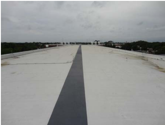
SCIT002a 5/10/2021 Newer upper membrane roof Penthouse roof
