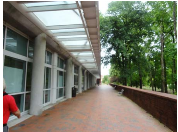
SCIT104a 5/10/2021 Brick paved walkway South end of site
