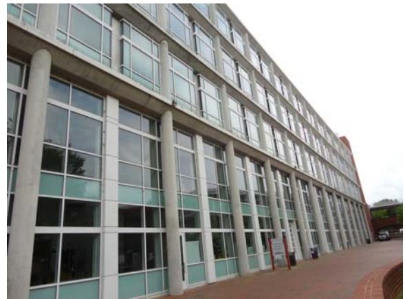
SCIT106a 5/10/2021 Glazing Partial north elevation of south wing
