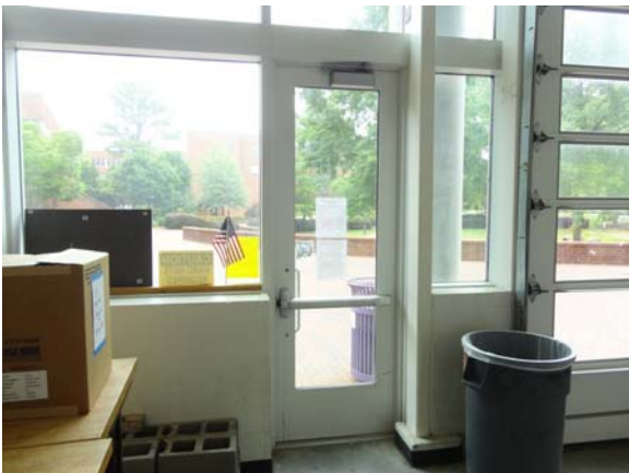
SCIT060a 5/10/2021 Oversized glass entry/egress door First floor, ITEC high bay
