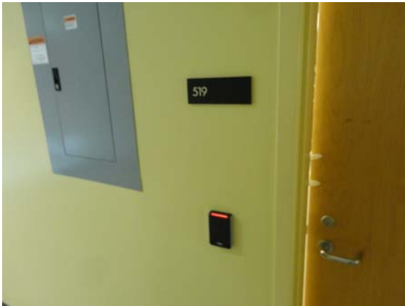
SCIT017a 5/10/2021 Lever hardware, smart card lock, and ADA room signage Fifth floor, commons
