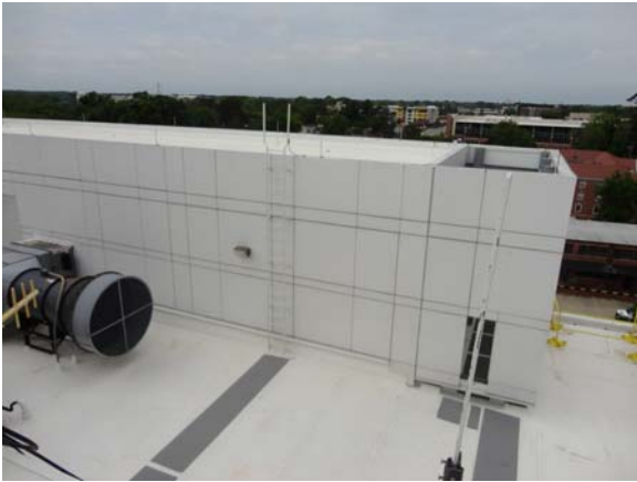
SCIT007a 5/10/2021 Prefinished metal panel facade Upper penthouse exterior
