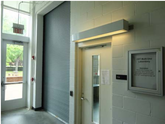
SCIT062a 5/10/2021 Coil overhead interior door First floor, former paint booth area
