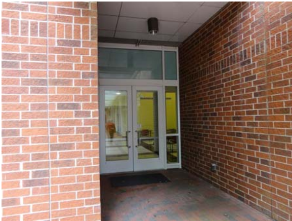
SCIT103a 5/10/2021 Exterior glass entry/egress doors First floor, south wing
