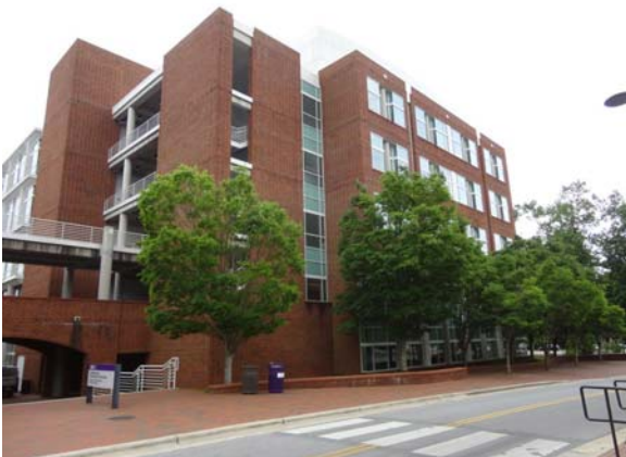
SCIT099a 5/10/2021 Exterior brick facade and glazing West elevation of south wing
