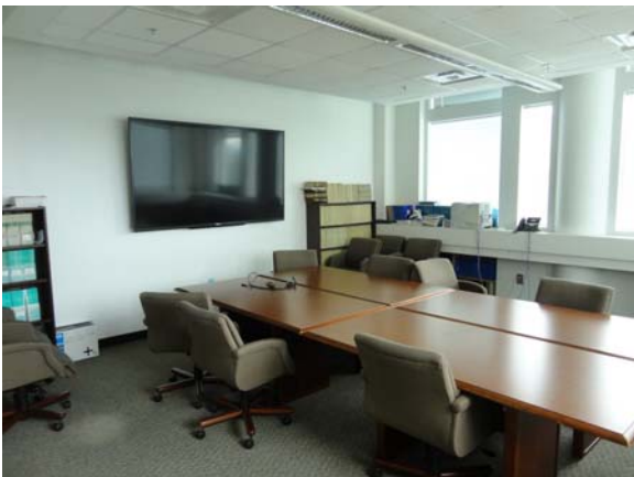
SCIT033a 5/10/2021 Broadloom carpeting and acoustical ceiling Fifth floor, west conference room
