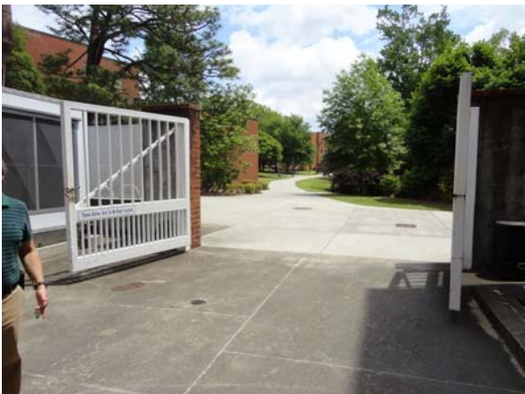
SCIT093a 5/10/2021 Metal service gates First floor, northeast service yard
