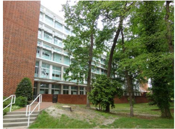
SCIT102a 5/10/2021 Brick facade and glazing South elevation of south wing
