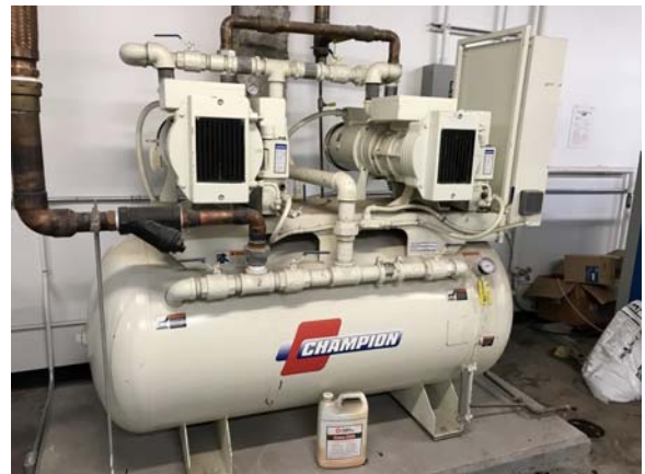
SCIT009e 5/10/2021 Laboratory vacuum pump Room P01
