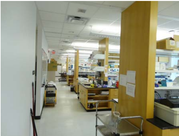
SCIT029a 5/10/2021 Vinyl flooring, acoustical ceiling, and wood lab cabinetry Fifth floor, lab
