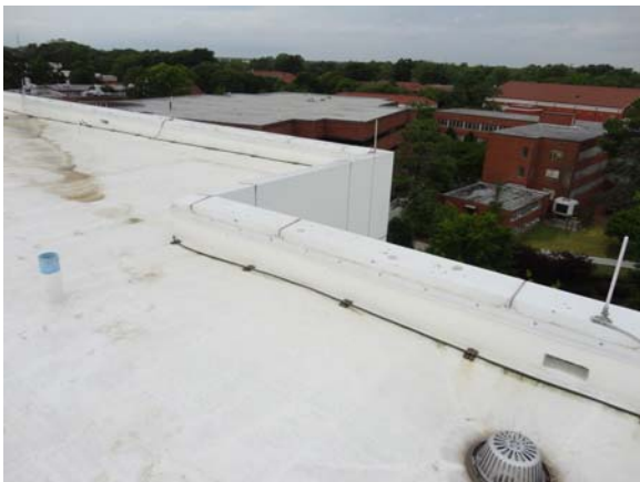
SCIT003a 5/10/2021 Low parapet cap Penthouse roof
