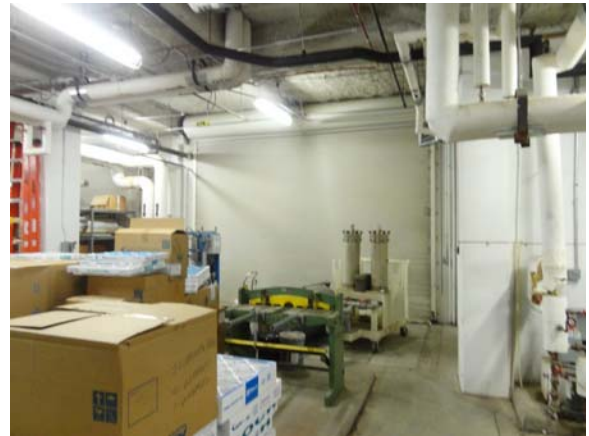
SCIT092a 5/10/2021 Utilitarian finishes First floor, central plant
