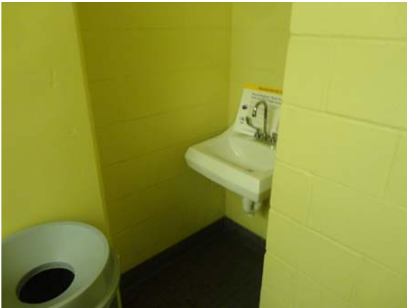
SCIT074a 5/10/2021 Accessible wall-hung lavatory North classroom wing women's restroom
