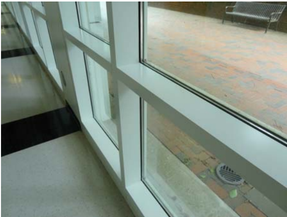
SCIT053a 5/10/2021 Thermal-pane storefront First floor, south perimeter corridor
