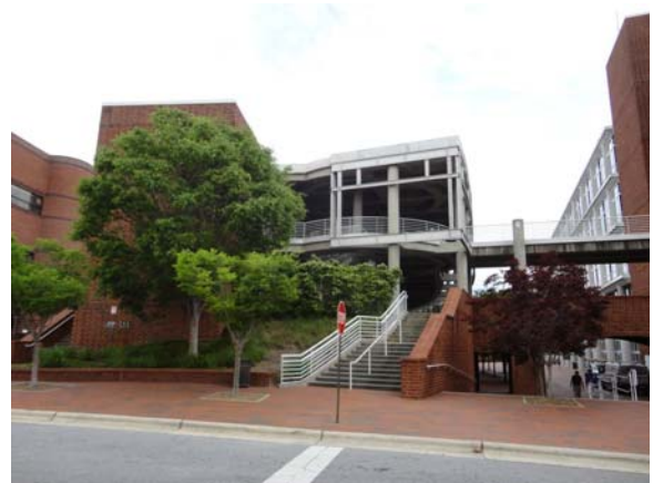
SCIT098a 5/10/2021 Exterior brick facade and glazing West elevation of north wing
