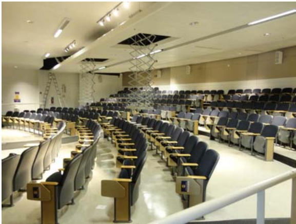
SCIT085a 5/10/2021 Lecture hall under partial renovation Second floor, north lecture hall
