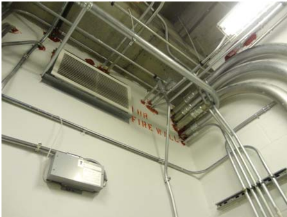
SCIT026a 5/10/2021 Firestopping in electrical closet Fifth floor
