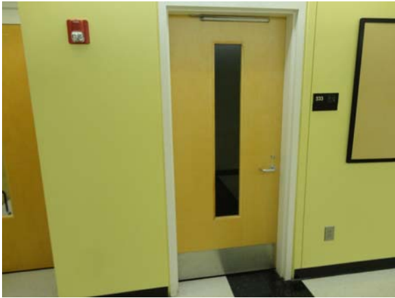
SCIT025a 5/10/2021 Typical corridor wood door with lever hardware Fifth floor corridor
