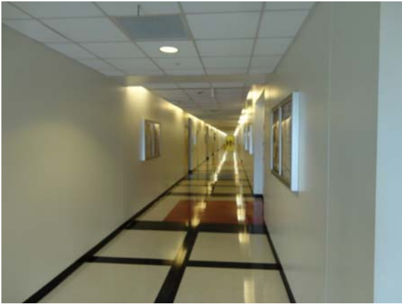
SCIT049a 5/10/2021 Vinyl floor tile, painted walls, and acoustical ceiling Second floor corridor
