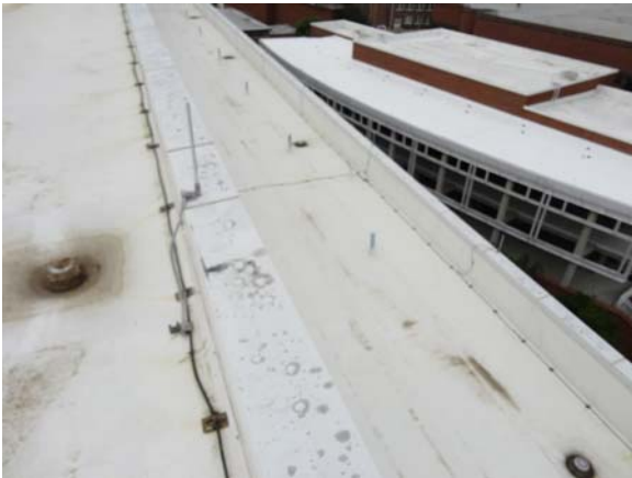
SCIT005a 5/10/2021 Lower membrane roof Lower roof
