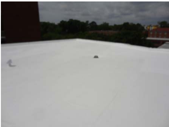
SCIT066a 5/10/2021 Coated membrane roof on breezeway Breezeway link to classroom building
