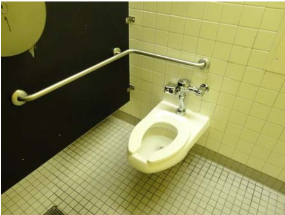
SCIT023a 5/10/2021 Accessible toilet stall Fifth floor, west men's restroom
