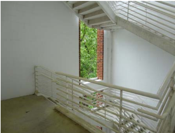
SCIT044a 5/10/2021 Accessible handrails Fourth floor, exterior stair tower
