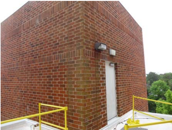
SCIT008a 5/10/2021 Brick veneer Upper stair tower exterior
