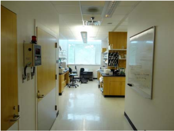
SCIT028a 5/10/2021 Vinyl flooring, acoustical ceiling, and wood lab cabinetry Fifth floor, lab
