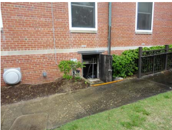
SLAY036a 5/12/2021 Cut down hollow-metal crawl space access door North elevation
