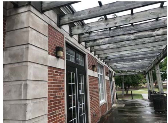
SLAY033e 5/12/2021 HID wallpacks Exterior
