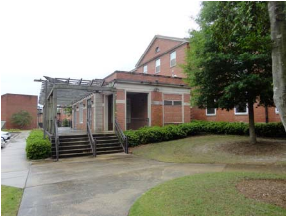
SLAY038a 5/12/2021 Adequate handrails at main entry steps North elevation
