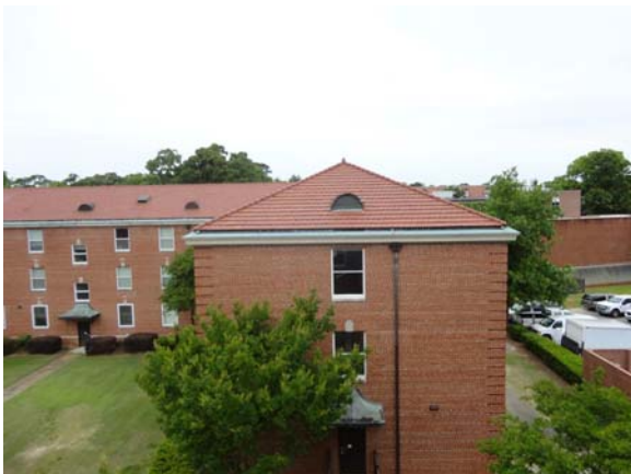
SLAY048a 5/12/2021 Main pitched clay tile roof with integral guttering Pitched roof
