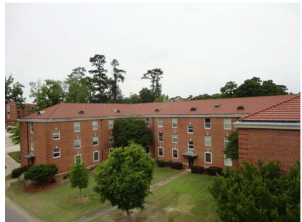
SLAY049a 5/12/2021 Main pitched clay tile roof with integral guttering Pitched roof
