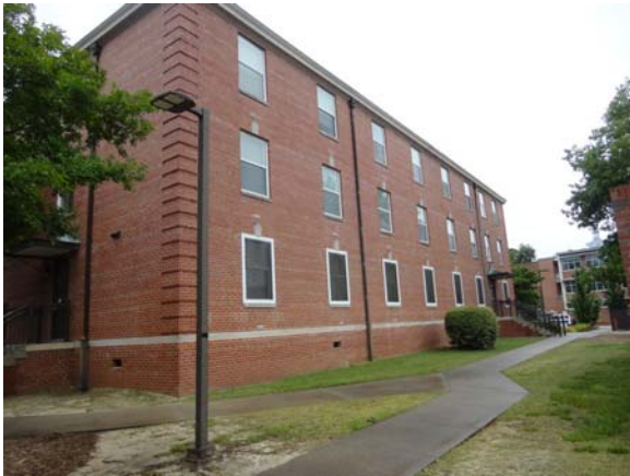
SLAY046a 5/12/2021 Brick facade East elevation
