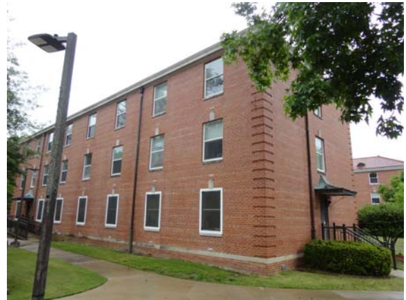
SLAY041a 5/12/2021 Exterior brick facade Southwest corner elevation
