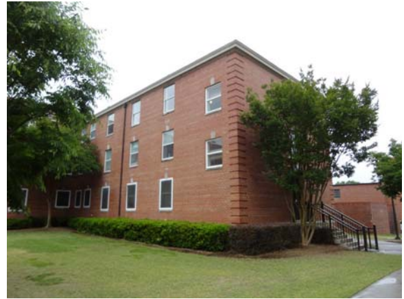
SLAY045a 5/12/2021 Brick facade Southeast corner elevation
