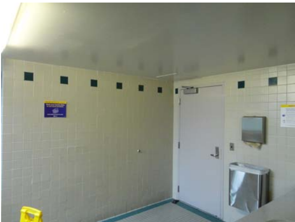
SLAY015a 5/12/2021 Ceramic wall tile Third floor, hall bath
