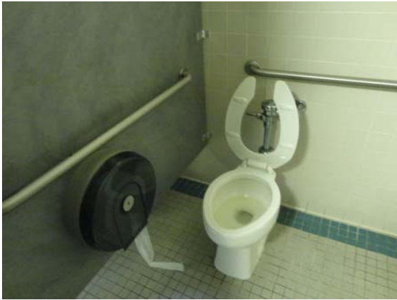
SLAY016a 5/12/2021 Accessible toilet stall Third floor, hall bath
