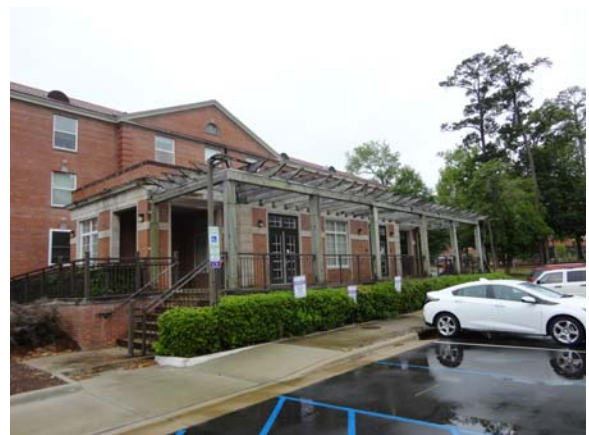
SLAY037a 5/12/2021 Wood trellis above entry porch North elevation
