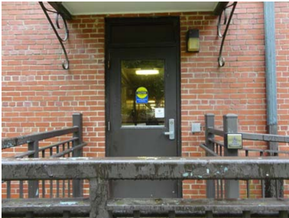
SLAY040a 5/12/2021 Hollow-metal exterior door with power door assist Northwest corner elevation
