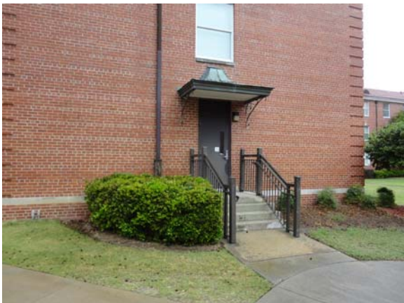
SLAY042a 5/12/2021 Hollow-metal secondary egress doors with adequate railings Southwest corner elevation
