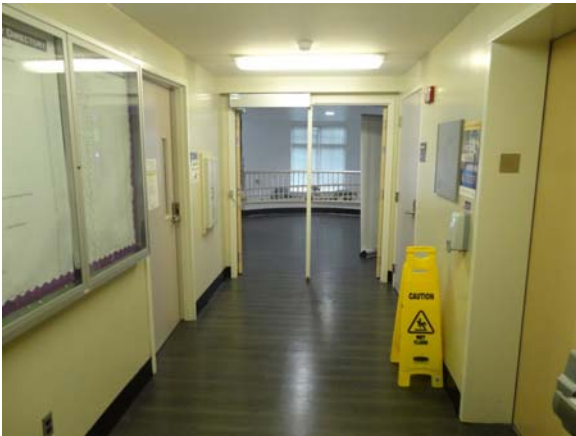
SLAY029a 5/12/2021 LVT flooring First floor, north entry lobby
