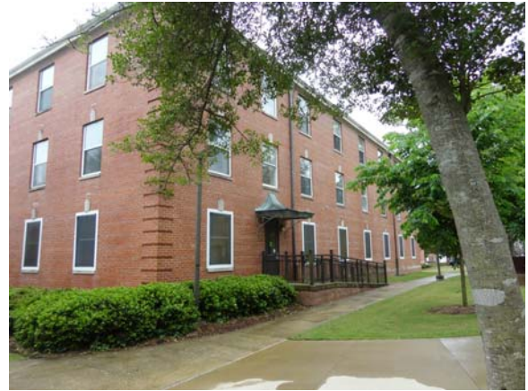
SLAY039a 5/12/2021 Ramped secondary entry/egress point Northwest corner elevation
