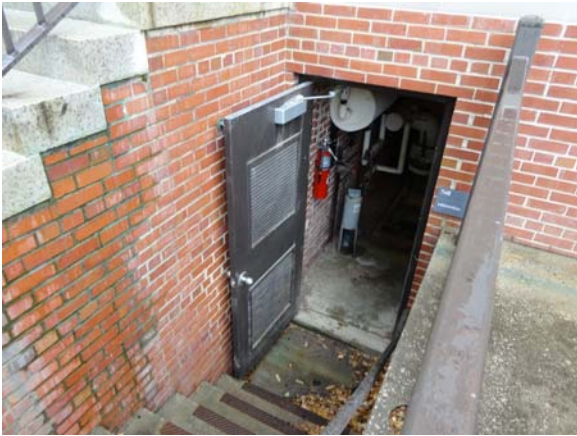
SLAY034a 5/12/2021 Hollow-metal exterior service door Northeast mechanical areaway
