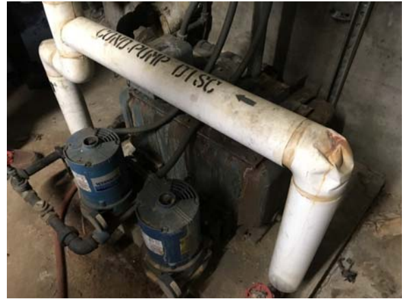
SLAY022e 5/12/2021 Condensate receiver Room 114E
