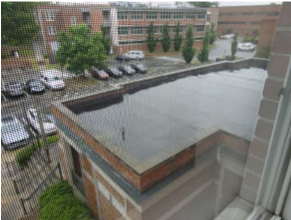
SLAY020a 5/12/2021 View of older membrane roof Roof over entry lobby
