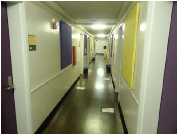
SLAY026a 5/12/2021 Newer LVT flooring Second floor corridor
