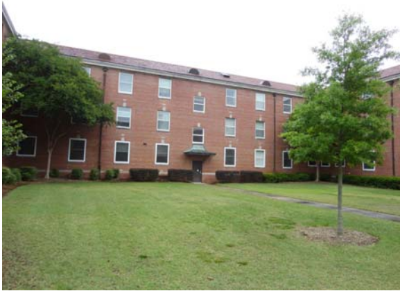
SLAY044a 5/12/2021 Brick facade Center of south elevation
