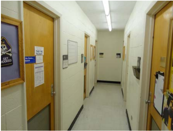
SPEI022a 5/11/2021 Aging original doors with knob hardware Second floor corridor
