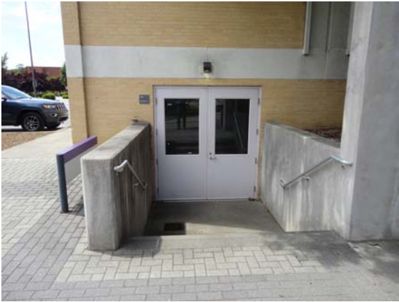
SPEI057a 5/11/2021 Newer hollow-metal service doors Southeast elevation
