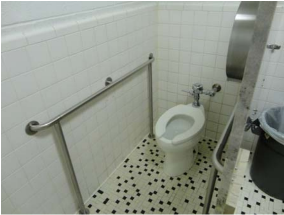
SPEI040a 5/11/2021 Partially accessible toilet stall First floor, all-gender restroom
