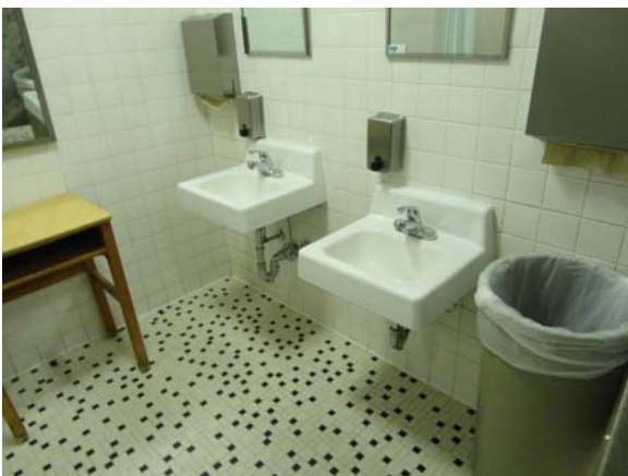
SPEI042a 5/11/2021 Two older wall-hung lavatories First floor, restroom
