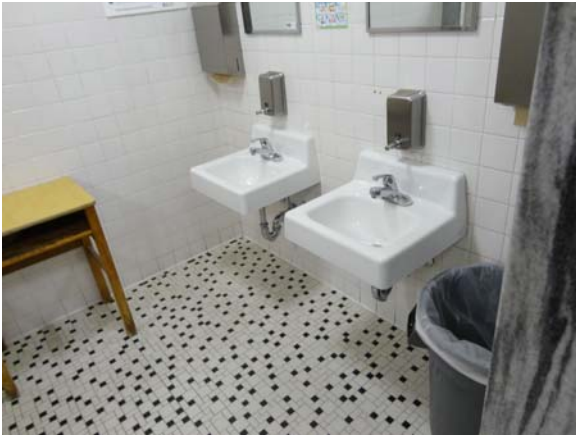
SPEI028a 5/11/2021 Partially accessible lavatories Second floor, women's restroom
