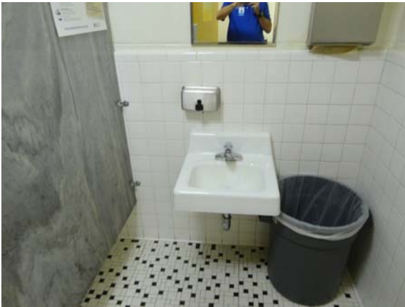
SPEI014a 5/11/2021 Older standard wall-hung lavatory Third floor, all-gender restroom
