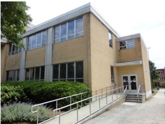
SPEI045a 5/11/2021 Ramped access and newer egress doors First floor, northwest stair tower
