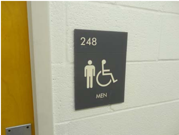
SPEI023a 5/11/2021 Nonaccessible restroom with ADA signage Second floor, men's restroom
