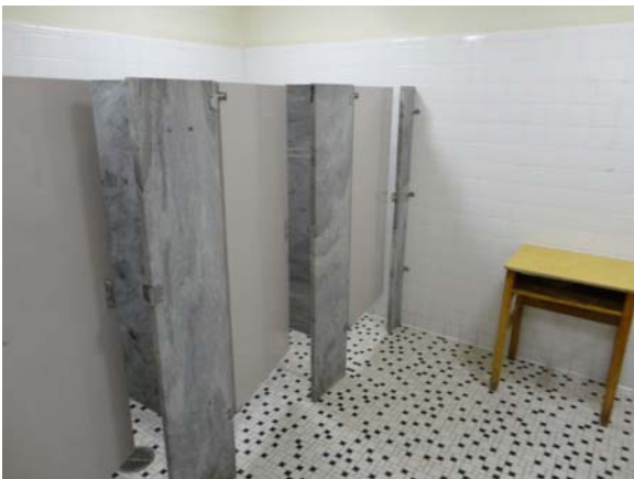
SPEI030a 5/11/2021 Ceramic floor tile and wainscot Second floor, women's restroom
