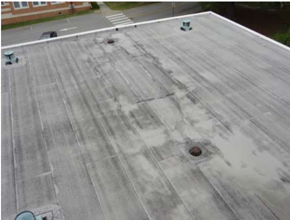
SPEI005a 5/11/2021 One of four lower built up roofs Lower roof
