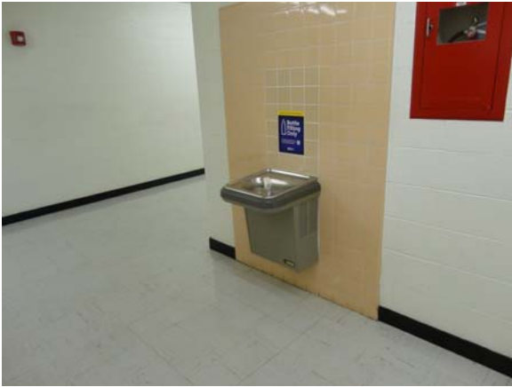
SPEI016a 5/11/2021 Newer, partially accessible, single-level water fountain Third floor corridor
