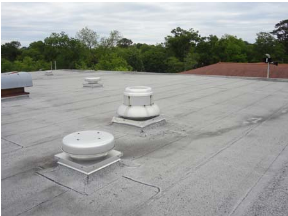
SPEI003a 5/11/2021 Upper built-up roof with cap sheet Upper main roof
