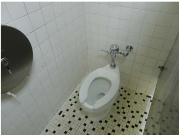
SPEI015a 5/11/2021 Older standard tankless water closet Third floor, all-gender restroom
