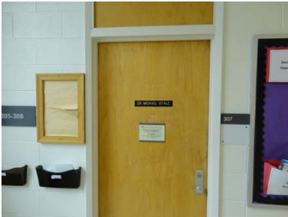
SPEI011a 5/11/2021 Nonrated corridor door with knob hardware Third floor corridor
