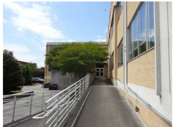
SPEI056a 5/11/2021 Updated ramp with flanking handrails Southeast elevation
