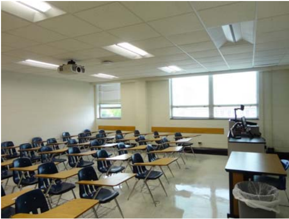
SPEI013a 5/11/2021 Original 9x9 vinyl flooring and newer acoustical ceiling Third floor, classroom
