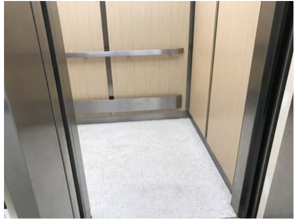
SPEI010e 5/11/2021 Elevator interior Elevator
