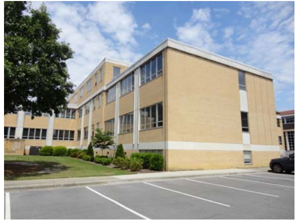
SPEI058a 5/11/2021 Brick facades and glazing Southwest corner elevation
