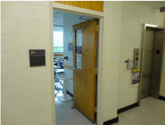
SPEI020a 5/11/2021 Aging original nonrated door Third floor corridor
