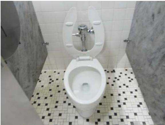
SPEI029a 5/11/2021 Standard narrow toilet stall Second floor, women's restroom
