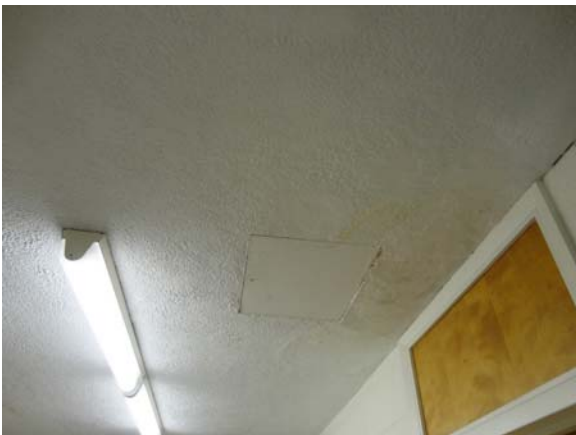
SPEI039a 5/11/2021 Original textured ceiling First floor corridor
