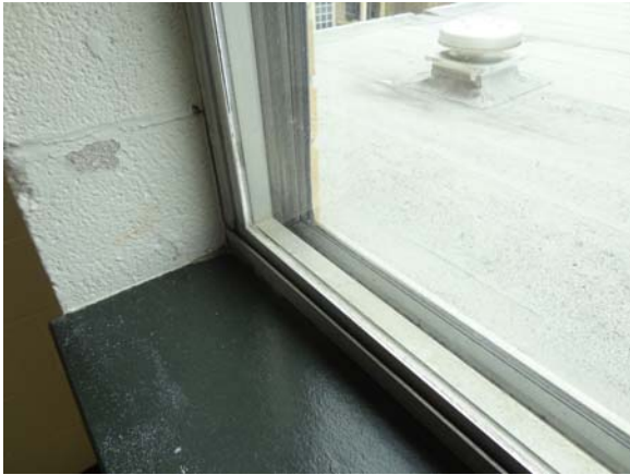
SPEI010a 5/11/2021 Windows with added outer storm window Third floor
