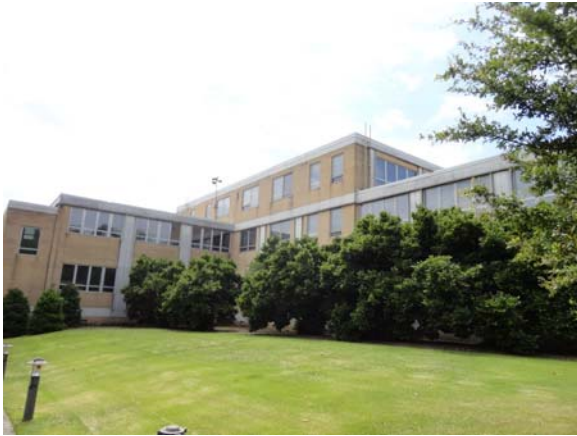
SPEI051a 5/11/2021 Brick facades and glazing Northeast corner elevation
