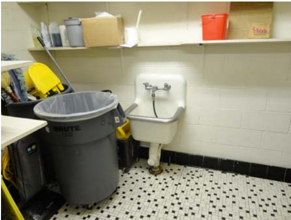
SPEI032a 5/11/2021 Original wall-mounted service sink Second floor, janitor's closet
