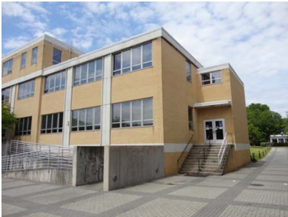
SPEI053a 5/11/2021 Brick facades and glazing Southeast corner elevation
