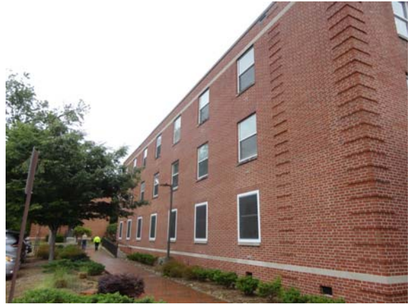
UMST056a 5/12/2021 Brick exterior and glazing West elevation
