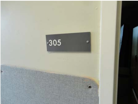
UMST011a 5/12/2021 Accessible wall-mounted room signage with Braille Third floor corridor
