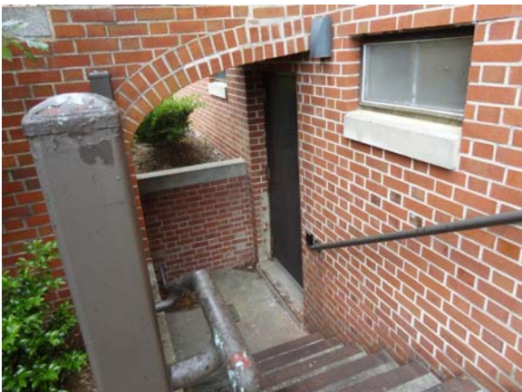
UMST047a 5/12/2021 Hollow-metal entry door Southeast corner basement entry
