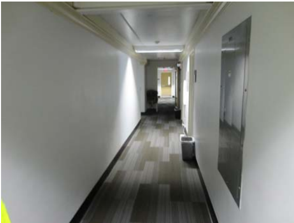
UMST039a 5/12/2021 Carpet tile and painted walls and ceiling First floor, counseling corridor
