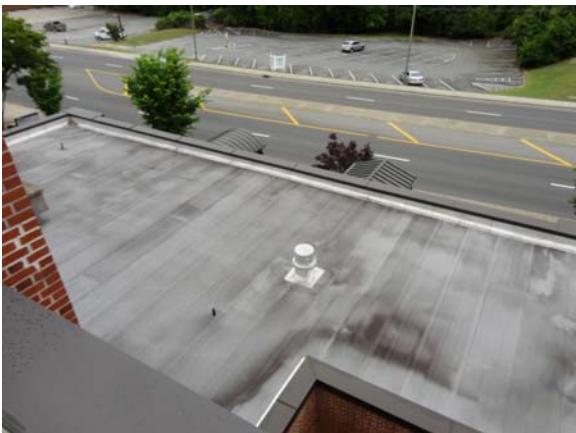
UMST006a 5/12/2021 Lower built-up roof with cap sheet Lobby roof
