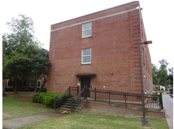
UMST058a 5/12/2021 Brick exterior and glazing Northwest corner elevation
