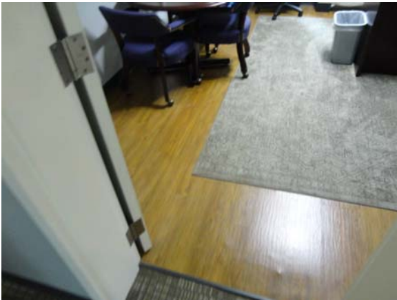
UMST045a 5/12/2021 Sheet vinyl flooring in some offices First floor, northeast offices
