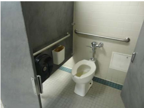
UMST033a 5/12/2021 Accessible toilet stall Second floor, women's hall bath
