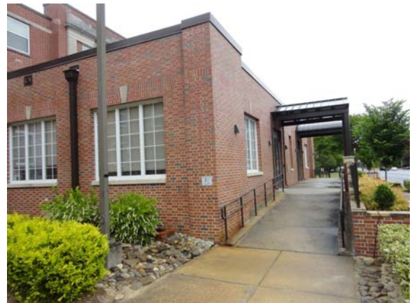
UMST054a 5/12/2021 Ramped access to main entry South elevation
