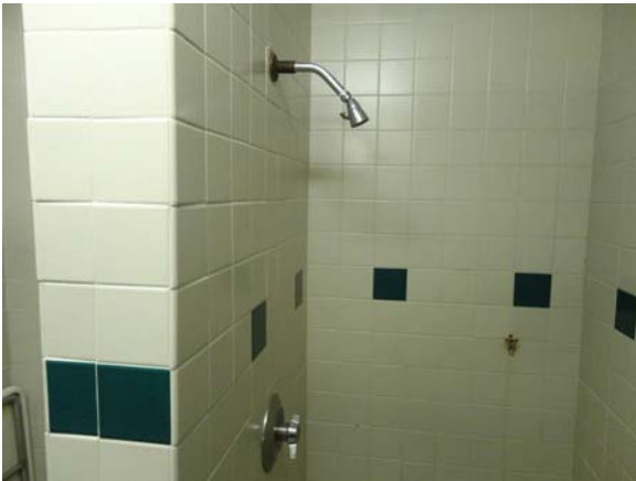
UMST017a 5/12/2021 Standard tiled shower Third floor, men's central hall bath
