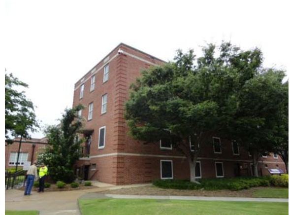
UMST046a 5/12/2021 Exterior brick facade Southeast corner elevation
