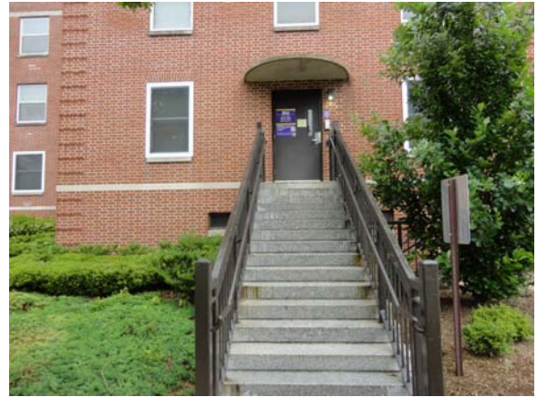
UMST050a 5/12/2021 Flanking handrails on egress stair Southeast wing
