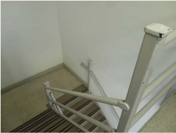
UMST010a 5/12/2021 Accessible inner handrails Third floor, stair tower
