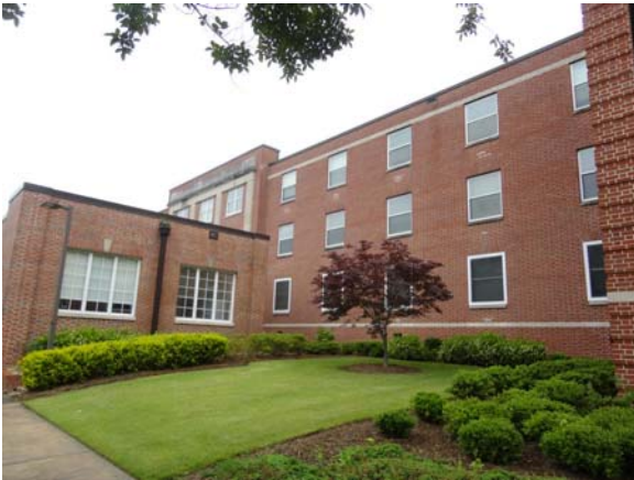
UMST051a 5/12/2021 Exterior brick facade East end of south main elevation
