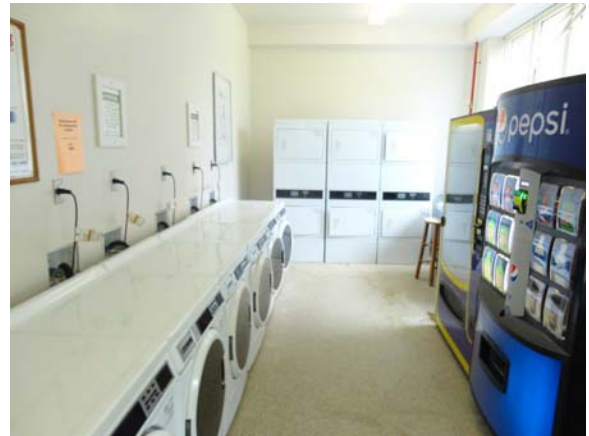
UMST064a 5/12/2021 Epoxy floor First floor, south laundry
