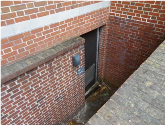
UMST061a 5/12/2021 Hollow-metal areaway door East basement service entry
