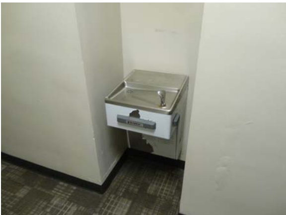
UMST030a 5/12/2021 Older single-level water fountain Third floor corridor
