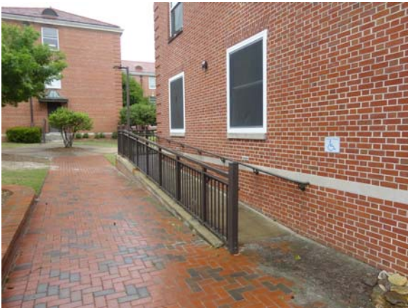
UMST057a 5/12/2021 Ramped access to secondary entry/egress point Northwest wing
