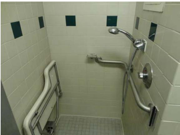
UMST018a 5/12/2021 Accessible roll-in shower Third floor, men's central hall bath
