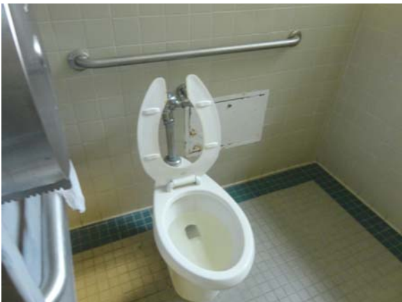
UMST036a 5/12/2021 Accessible toilet stall Second floor, men's hall bath
