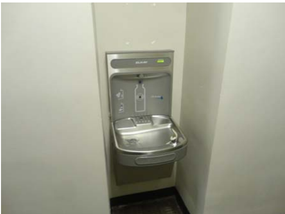
UMST027a 5/12/2021 New, partially accessible, single-level water fountain and bottle filler Third floor corridor
