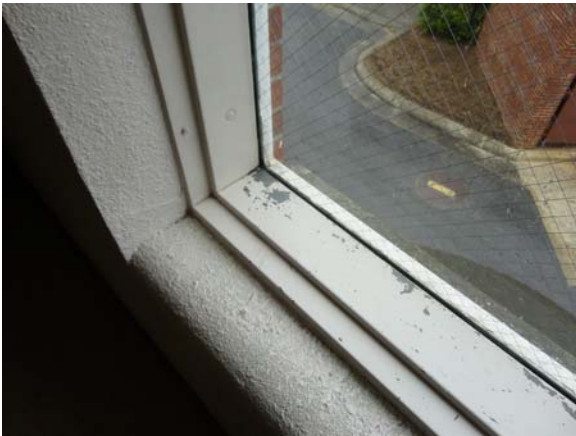
UMST032a 5/12/2021 Original single-pane wire glass Third floor, stair tower
