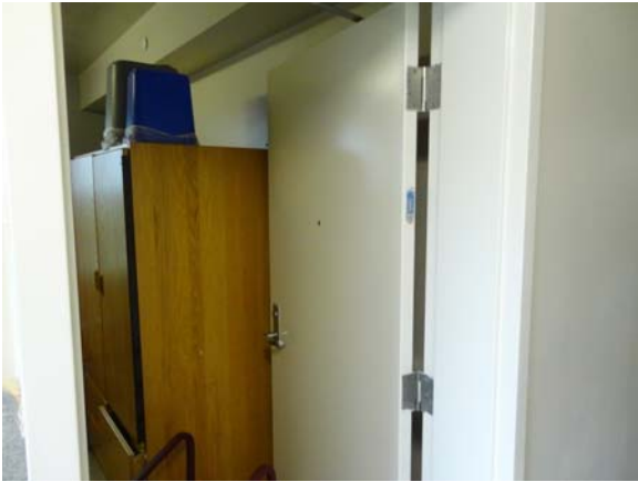
UMST013a 5/12/2021 Newer fire-rated corridor door with lever hardware Third floor corridor
