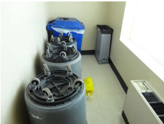
UMST021a 5/12/2021 Older VCT flooring Third floor, trash room
