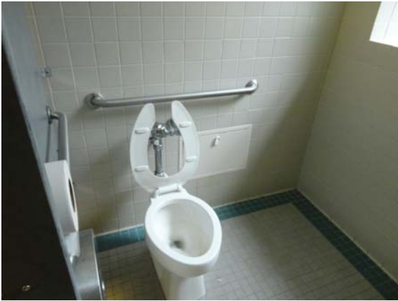
UMST016a 5/12/2021 Accessible toilet stall Third floor, men's central hall bath
