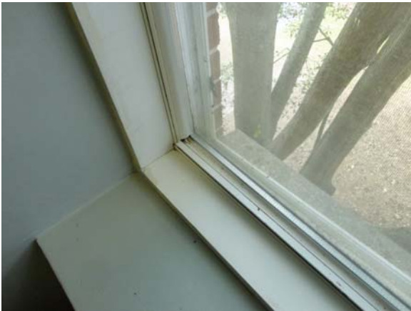
UMST014a 5/12/2021 Older thermal-pane, metal-framed glazing Third floor
