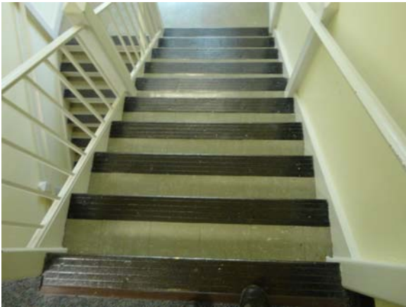
WHIC029a 5/10/2021 9x9 vinyl flooring on stair treads Second floor, original stair tower
