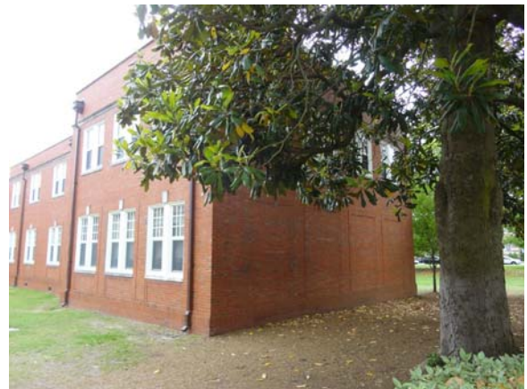
WHIC054a 5/10/2021 Brick facade and glazing Northeast corner of annex
