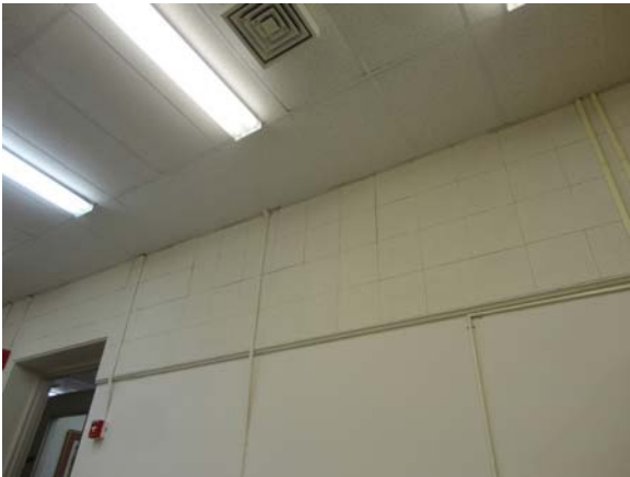
WHIC035a 5/10/2021 Upper adhesive wall tiles First floor, east wing addition
