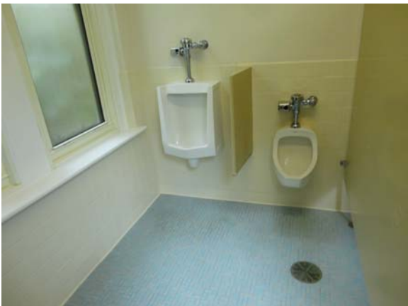
WHIC036a 5/10/2021 One old and one newer wall-hung urinal First floor, men's restroom
