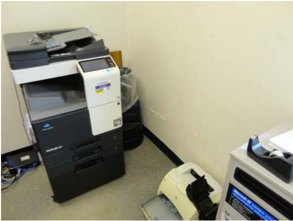
WHIC013a 5/10/2021 Signs of possible localized water infiltration Second floor, perimeter wall
