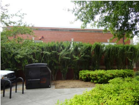
WHIC063a 5/10/2021 Brick facade East elevation of east wing
