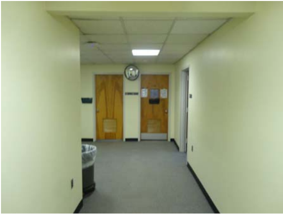
WHIC010a 5/10/2021 Older carpeting and acoustical ceiling Second floor, annex corridor
