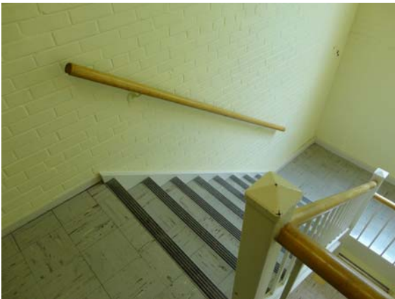
WHIC006a 5/10/2021 9x9 vinyl floor tile and nonaccessible handrails Second floor, annex stair tower
