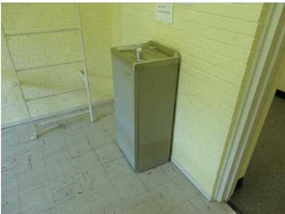
WHIC009a 5/10/2021 Poorly located, nonaccessible, aging water fountain Second floor, stair tower
