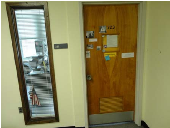
WHIC011a 5/10/2021 Nonrated corridor door with knob hardware Second floor, annex corridor
