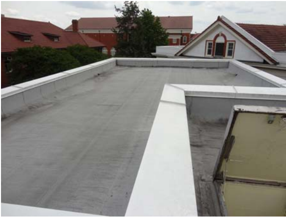
WHIC001a 5/10/2021 Newer built-up roof and cap sheet Annex roof
