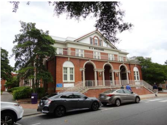
WHIC059a 5/10/2021 Brick facade and glazing South elevation of original building
