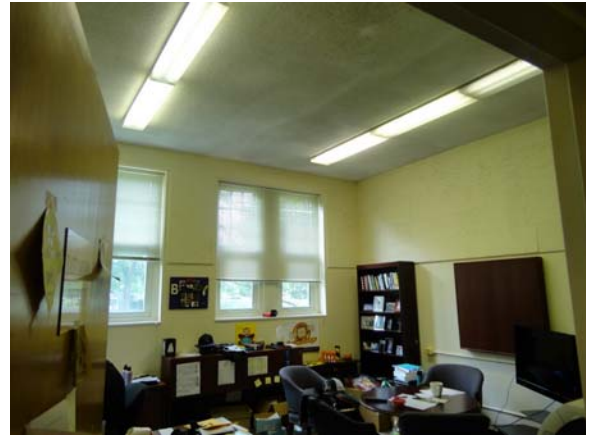
WHIC050a 5/10/2021 Textured ceilings First floor, north annex
