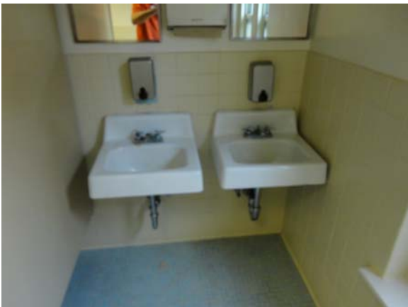
WHIC021a 5/10/2021 Older wall-hung lavatories Second floor, men's restroom
