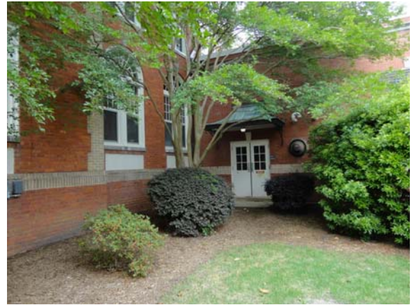
WHIC062a 5/10/2021 Older hollow-metal service doors South elevation of east wing addition
