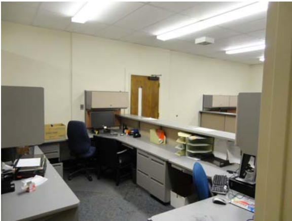
WHIC032a 5/10/2021 Typical carpeting and acoustical ceiling First floor, original building office
