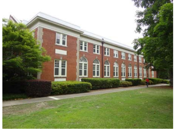
WHIC056a 5/10/2021 Brick facade and glazing West elevation of original building
