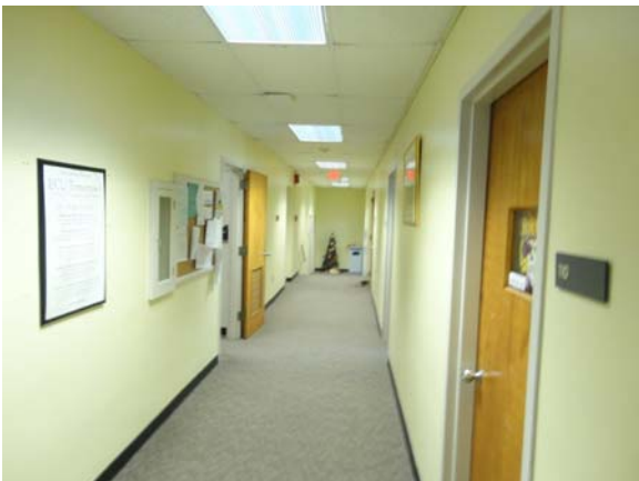
WHIC047a 5/10/2021 Carpeting and acoustical ceiling First floor, annex corridor
