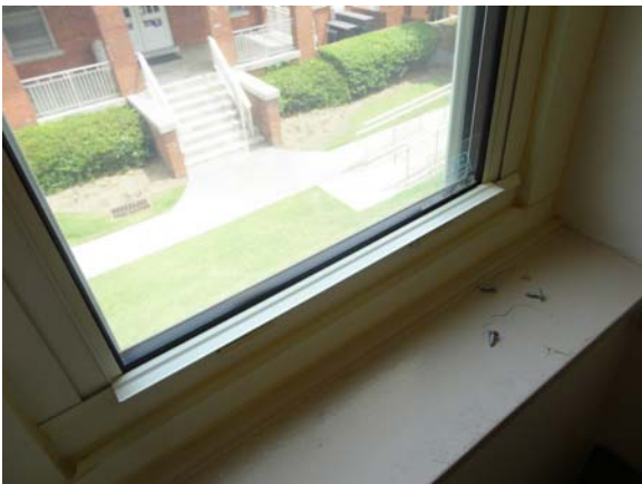
WHIC015a 5/10/2021 Updated exterior glazing Second floor, annex
