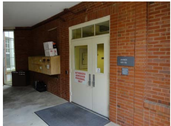
WHIC066a 5/10/2021 Newer hollow-metal doors South entry to first floor annex
