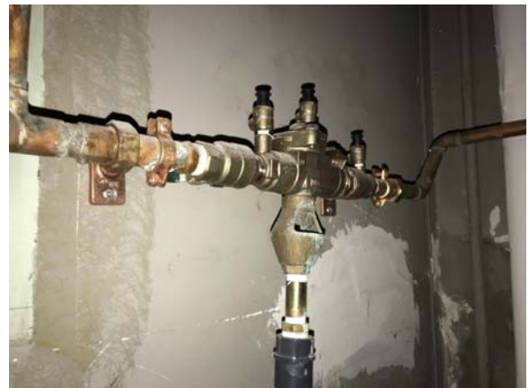
WHIC027e 5/10/2021 Backflow preventer for heating hot water makeup Room 117D
