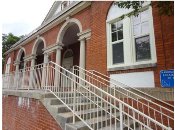
WHIC068a 5/10/2021 Accessible handrails on main south entry steps South elevation of original building
