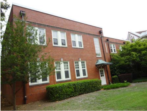
WHIC055a 5/10/2021 Metal egress door at stair tower West elevation of annex
