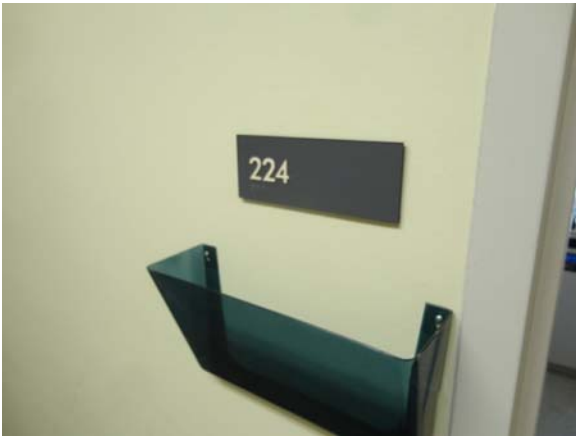
WHIC014a 5/10/2021 Upgraded accessible room signage Second floor corridor
