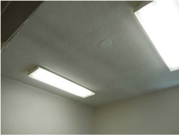
WHIC016a 5/10/2021 Textured ceilings Second floor, annex office
