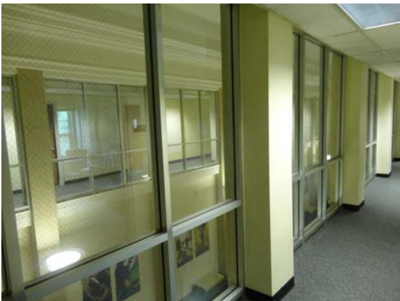
WHIC027a 5/10/2021 Wire glass glazing in central atrium Second floor, original building
