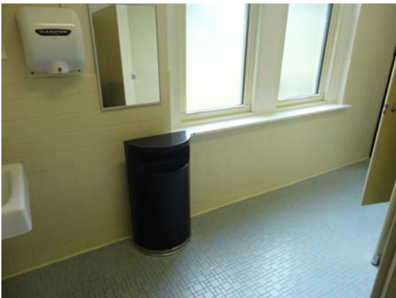
WHIC039a 5/10/2021 Ceramic floor tile and wainscoting First floor, men's restroom
