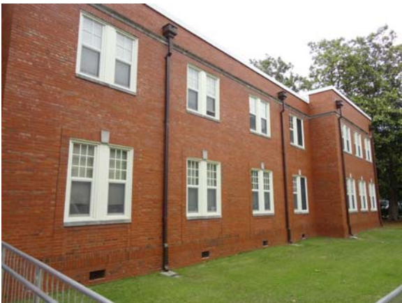
WHIC053a 5/10/2021 Brick facade and glazing East elevation of annex
