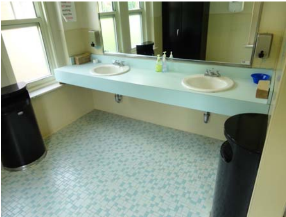
WHIC023a 5/10/2021 Older counter lavatories Second floor, women's restroom
