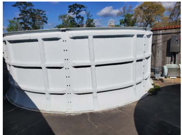
MCCP1060e 4/6/2022 Re-epoxied cooling tower shell CCP#1 Cooling Tower roof
