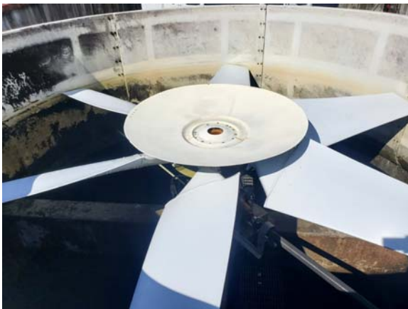
MCCP1053e 4/6/2022 Re-epoxied cooling tower CT-1 fan assembly CCP#1 Cooling Tower roof
