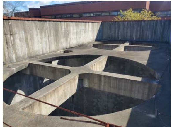
MCCP1062e 4/6/2022 Area for cooling tower expansion CCP#1 Cooling Tower roof
