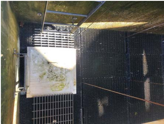
MCCP1061e 4/6/2022 Cooling tower infill CCP#1 Cooling Tower roof
