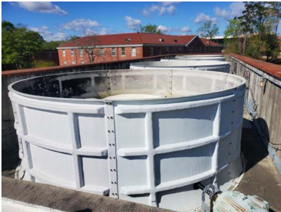
MCCP1051e 4/6/2022 Overview of tower fan assemblies CT-1 to CT-4 CCP#1 Cooling Tower roof
