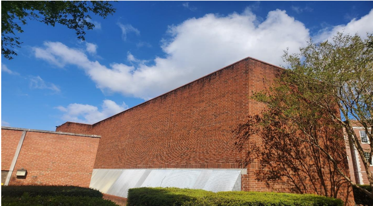
Image 4: Cooling Tower Building
