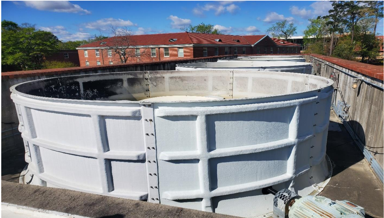
Image 5: Cooling Tower cells 1-4 with new epoxy exterior finish
