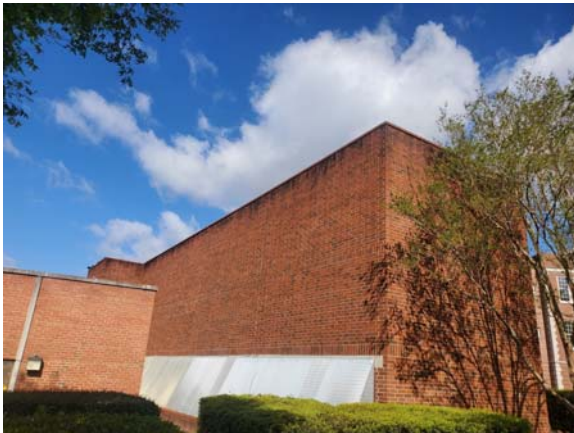
MCCP1027e 4/6/2022 Overview of cooling tower facility CCP#1 Cooling Tower
