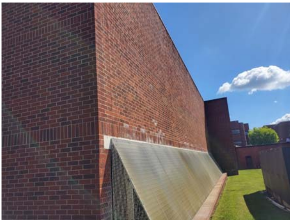
MCCP1065e 4/6/2022 Exterior brick facade CCP#1 Cooling Tower
