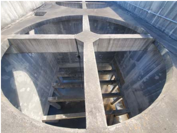
MCCP1063e 4/6/2022 Area for cooling tower expansion CCP#1 Cooling Tower roof
