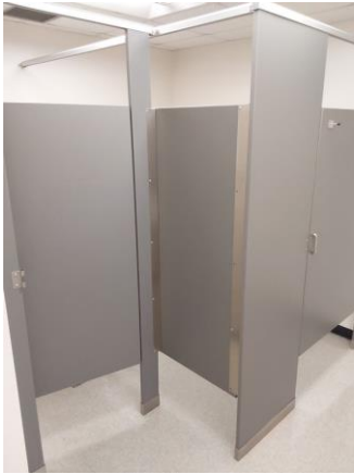
059014a 1/11/2023 Toilet partitions Women's restroom 114
