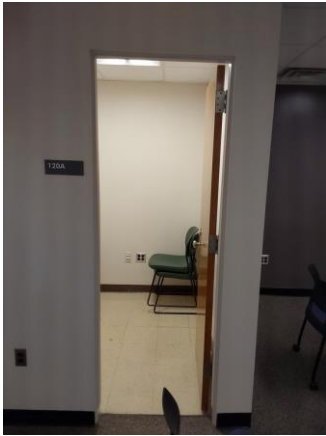
059020a 1/11/2023 Vinyl tile floor Room 120A
