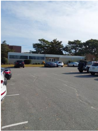
059023a 1/11/2023 Concrete panel facade and glazing West elevation
