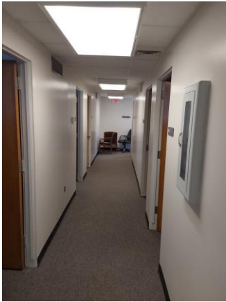
059007a 1/11/2023 Typical corridor, with painted walls, carpeting, lay-in acoustical tile ceiling Corridor
