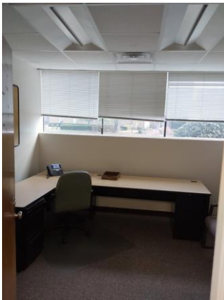
059008a 1/11/2023 Typical office, with painted walls, carpeting, lay-in acoustical tile ceiling Room 107
