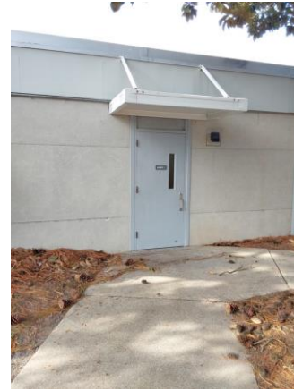
059026a 1/11/2023 Painted metal door and canopy East elevation
