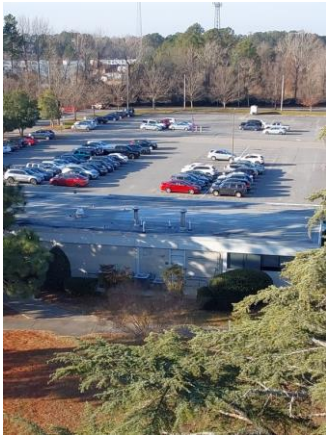
059001a 1/11/2023 Modified bitumen roof Roof
