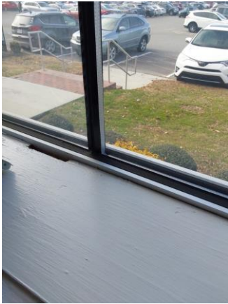
059005a 1/11/2023 Exterior window Room 101
