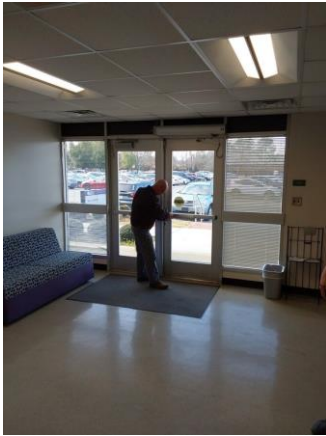
059002a 1/11/2023 Anodized aluminum door with operator Waiting room
