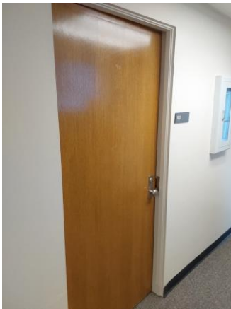
059006a 1/11/2023 Nonrated wood door with knob hardware Room 102
