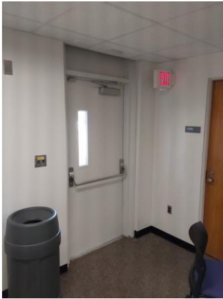
059019a 1/11/2023 Exit door with signage and panic hardware North exit
