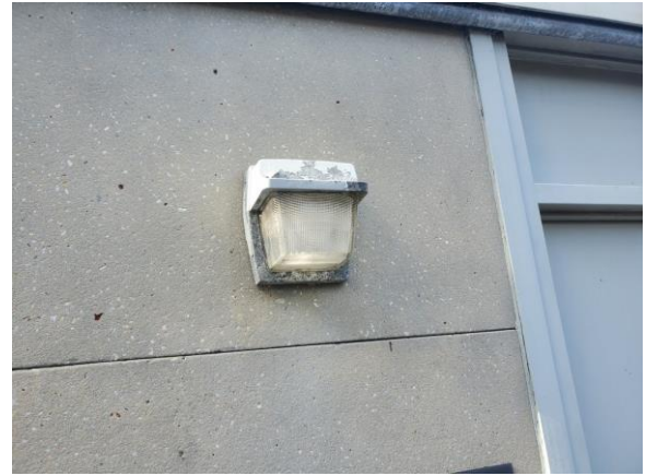
059022e 1/11/2023 Aged surface-mounted exterior light with HID lamp Exterior
