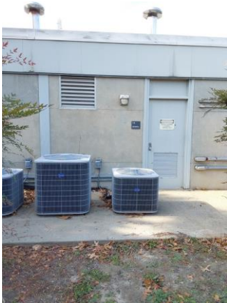
059027a 1/11/2023 Painted metal door and louver East elevation
