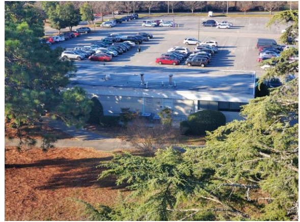
059001e 1/11/2023 Furnace vent stack and rooftop exhaust fan Roof
