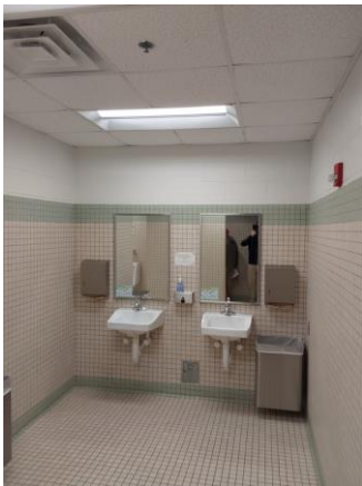
013009a 1/11/2023 Restroom lavatories Room 3601
