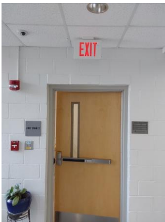
013012a 1/11/2023 Typical exit stair door with signage Stair 2
