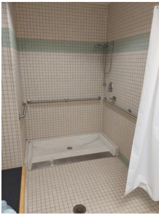
013029a 1/11/2023 Women's restroom roll-in shower Room 2702
