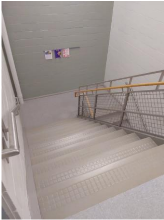
013013a 1/11/2023 Stairs with compliant handrails and guardrail Stair 2
