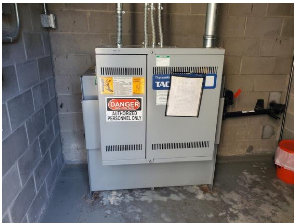
013075e 1/11/2023 Hydraulic elevator machine Room 1701
