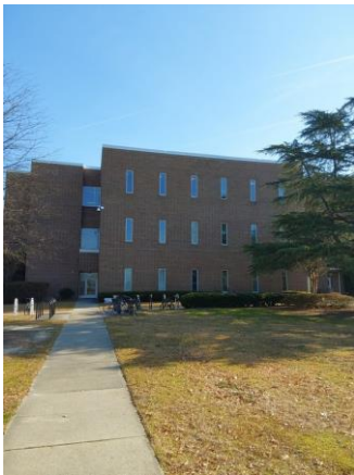
013051a 1/11/2023 Exterior brick and walk West elevation
