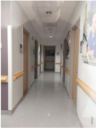
013031a 1/11/2023 Corridor with finishes shown Room 2018
