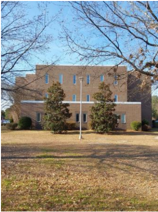
013056a 1/11/2023 Exterior brick and glazing with trees East elevation
