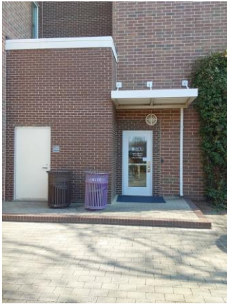
013050a 1/11/2023 Painted exit doors West elevation
