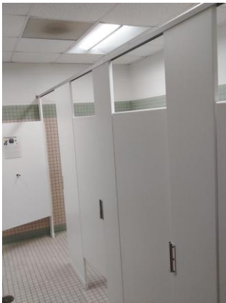
013015a 1/11/2023 Partitions in women's restroom Room 3602
