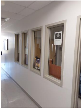
013014a 1/11/2023 Interior tempered glass along corridor Room 3006
