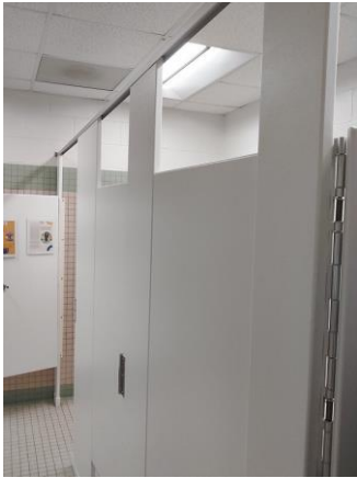
013028a 1/11/2023 Women's restroom partitions Room 2702
