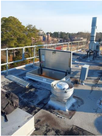
013001a 1/11/2023 Roof hatch with fall protection Roof
