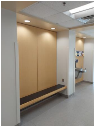
013048a 1/11/2023 Typical alcove wall with wood laminate Room 1003
