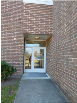
013052a 1/11/2023 Painted exit door with power operator West elevation
