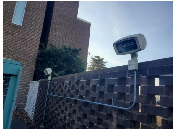
013051e 1/11/2023 Flood type light fixtures Site
