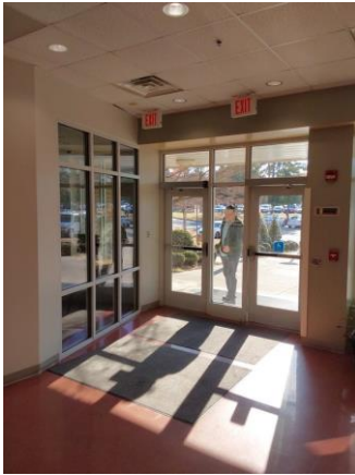
013046a 1/11/2023 Anodized aluminum main entrance door Room 1001
