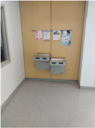
013026a 1/11/2023 Typical water fountain and wall finish Room 3003
