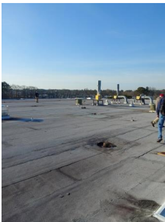
013006a 1/11/2023 Overall roof photo Roof
