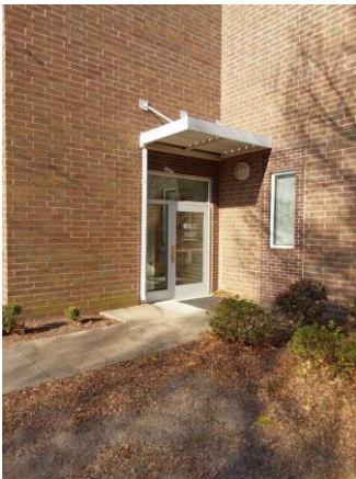
013057a 1/11/2023 Entrance with painted door Southeast elevation
