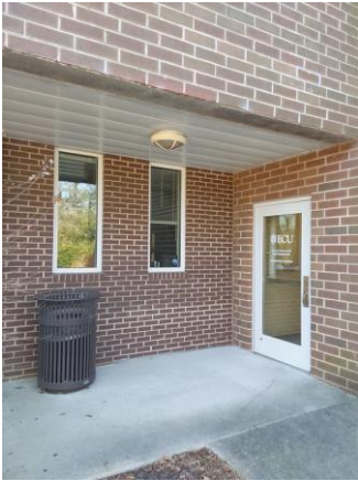
013055a 1/11/2023 Entrance with metal soffit Northeast elevation
