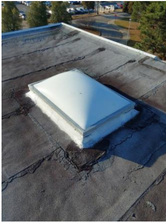
013004a 1/11/2023 Fiberglass skylight Roof over stair 1
