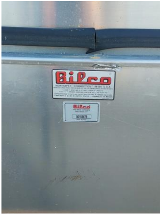
013007a 1/11/2023 Roof hatch nameplate Roof
