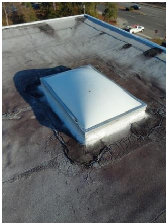
013005a 1/11/2023 Fiberglass skylight Roof over stair 2
