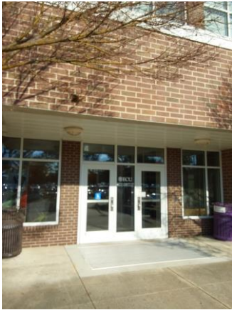
013049a 1/11/2023 Metal panel entrance soffit South elevation
