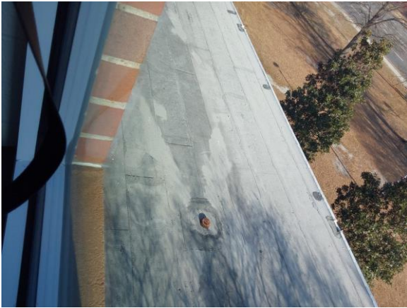
013061a 1/11/2023 Modified bitumen build-out roof Roof
