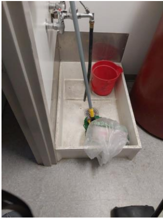
013035a 1/11/2023 Mop sink Room 2311
