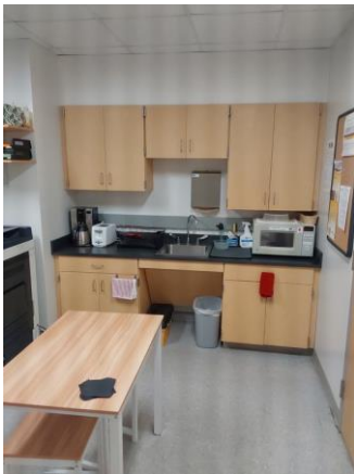
013039a 1/11/2023 Break room casework with accessible sink Room 1417
