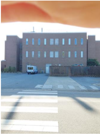
013053a 1/11/2023 Exterior brick and glazing with mechanical yard North elevation
