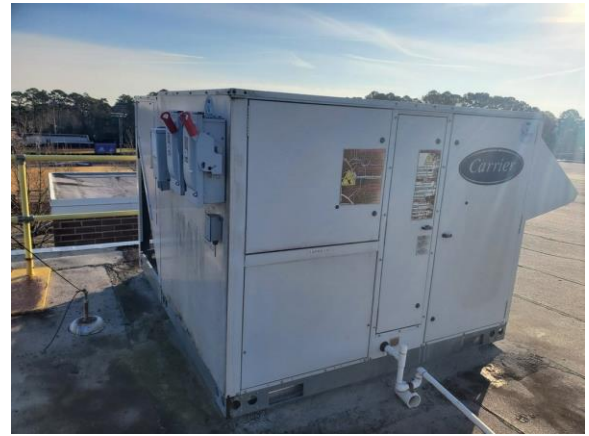
013004e 1/11/2023 Rooftop package unit RTU-3-1 Roof
