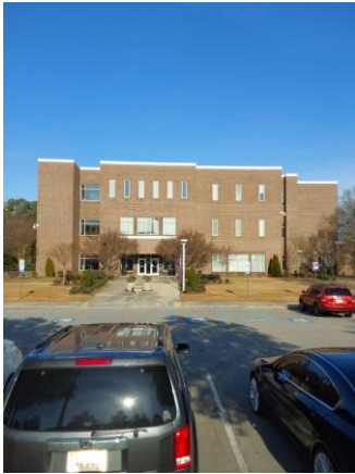
013058a 1/11/2023 Exterior brick and glazing at entry South elevation
