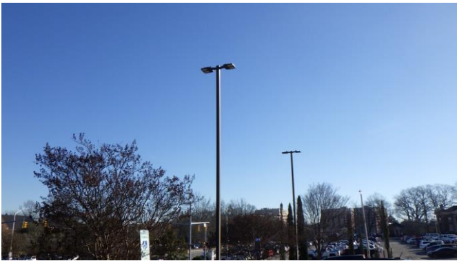
164078e 1/25/2023 Parking lot lighting South elevation
