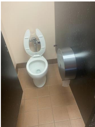
164009a 1/25/2023 Tile flooring, finished walls, and water closet Restroom
