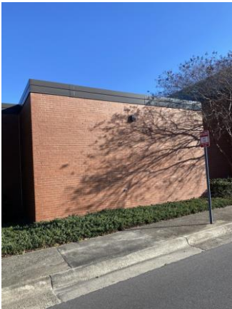
164026a 1/25/2023 Brick exterior Exterior
