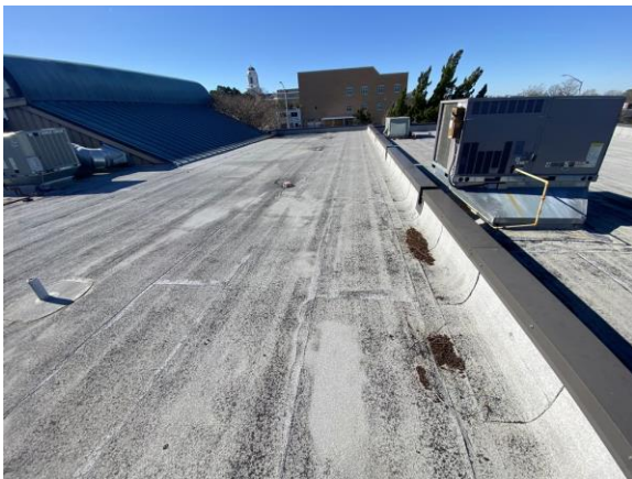
164003a 1/25/2023 Modified bitumen roof Roof
