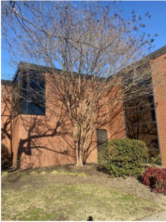
164028a 1/25/2023 Brick exterior, metal door, and glazing Exterior
