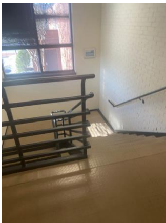
164015a 1/25/2023 Vinyl treads and landings, metal railing, and finished walls Stairwell
