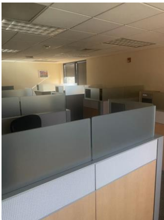
164012a 1/25/2023 ACT, carpet, and finished walls Work area
