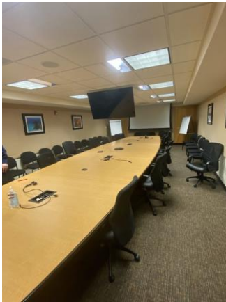
164019a 1/25/2023 Finished walls, tile ACT, and carpet Conference room
