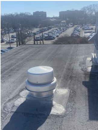
164005a 1/25/2023 Modified bitumen roof Roof
