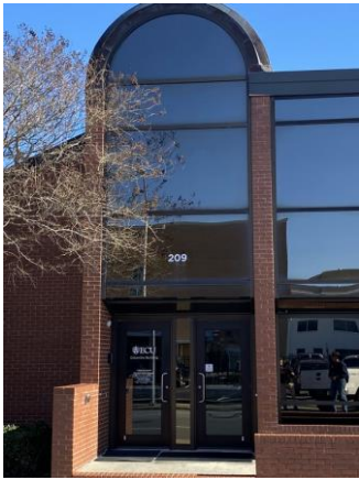
164001a 1/25/2023 Brick and glazing Entrance
