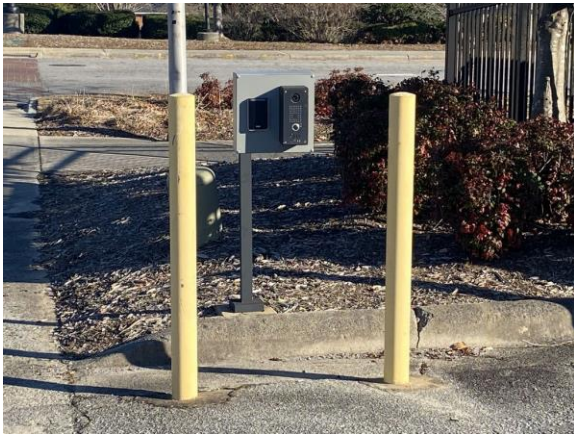
164031a 1/25/2023 Gate system Exterior
