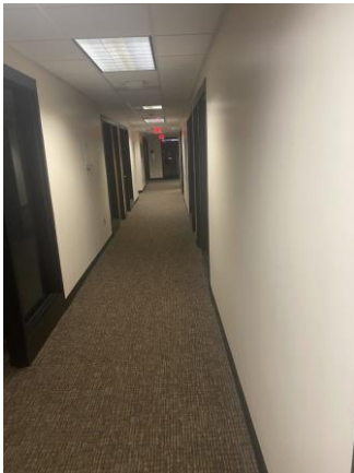
164014a 1/25/2023 ACT, carpet, and finished walls Corridor
