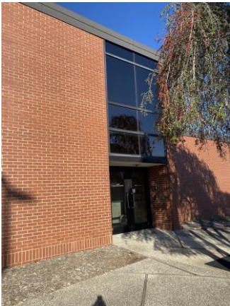
164029a 1/25/2023 Brick exterior, glass doors, and glazing Exterior
