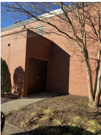
164027a 1/25/2023 Brick exterior and metal doors Exterior
