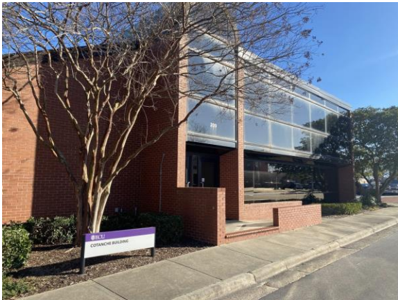
164032a 1/25/2023 Ramp lacking handrail Entrance
