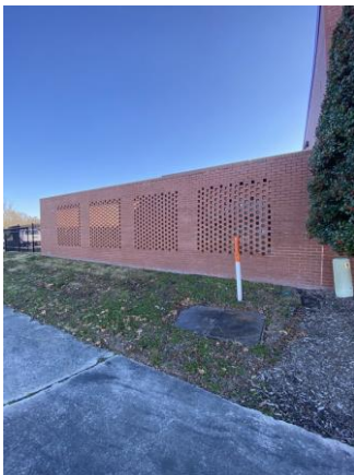
164024a 1/25/2023 Brick exterior Exterior
