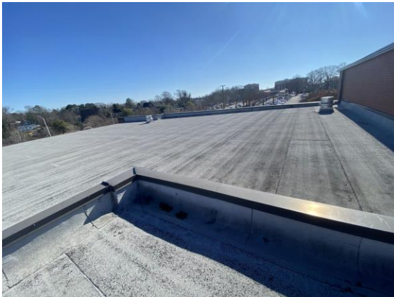
164002a 1/25/2023 Modified bitumen roof Roof
