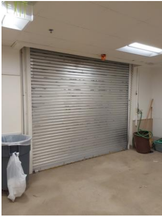
002094a 1/9/2023 Loading dock overhead door Room 107
