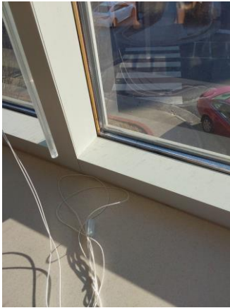
002070a 1/9/2023 Exterior windows and joints Room 2221
