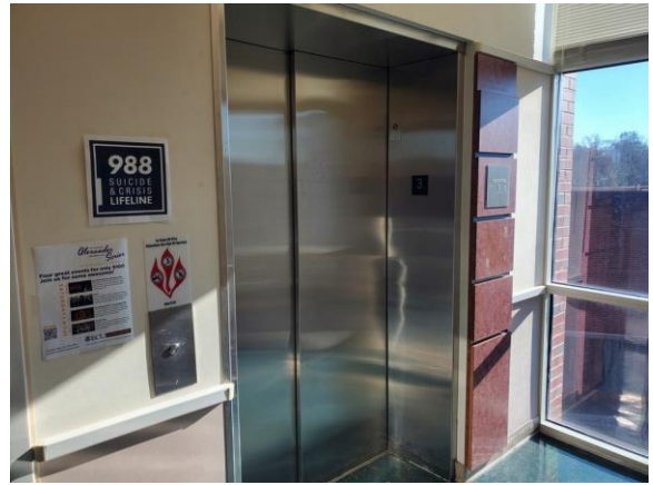
002044e 1/9/2023 Elevator B passenger car doors Lobby 394
