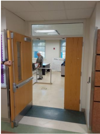
002035a 1/9/2023 Rated door with side panel and vision glass Room 349
