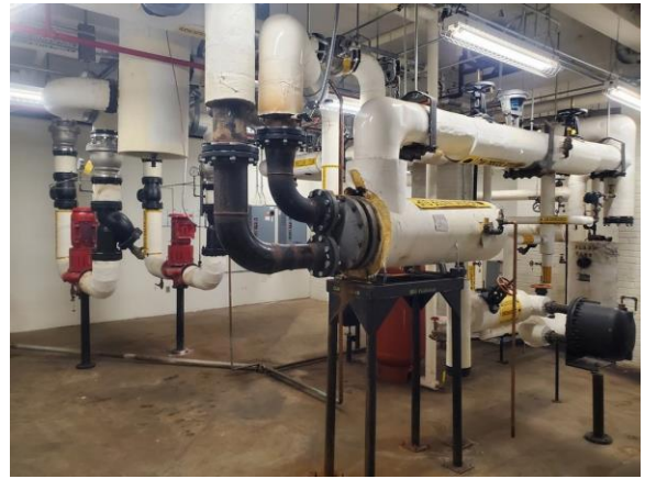
002056e 1/9/2023 Overview of mechanical room Room 153
