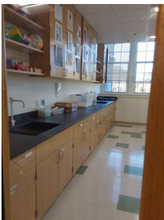
002042a 1/9/2023 Solid surface lab counter with casework Room 355
