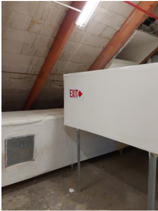
002019a 1/9/2023 Exit signage and roof attic Roof attic
