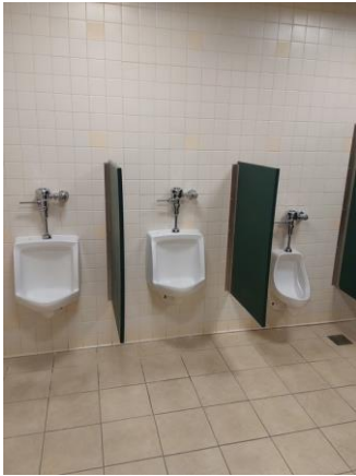
002028a 1/9/2023 Typical urinals with ADA height Room 334
