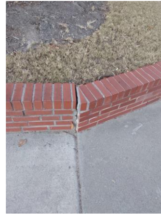
Damaged brick knee wall South elevation
