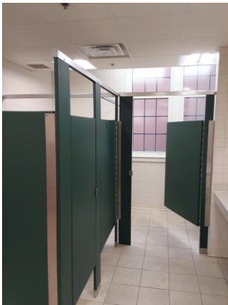
002030a 1/9/2023 Typical toilet partitions Room 334
