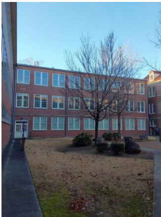
002098a 1/9/2023 Exterior brick and windows with exterior door Inside west wing
