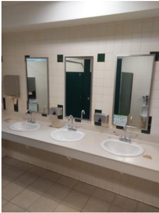
002029a 1/9/2023 Solid surface sink counter Room 334
