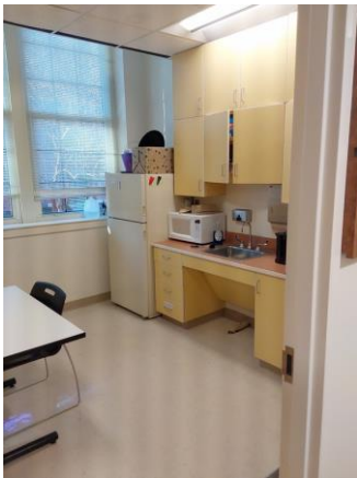
002066a 1/9/2023 Laminate casework and countertop Room 227
