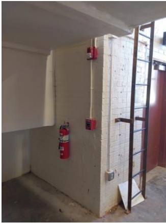
002020a 1/9/2023 Roof ladder and extinguisher Roof attic
