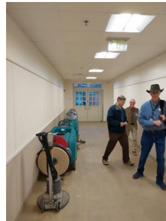
002093a 1/9/2023 Epoxy floor with acoustic wall covering Room 1202
