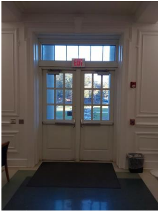
002079a 1/9/2023 Exterior doors with panic hardware Room 245
