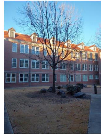
002097a 1/9/2023 Exterior brick and windows with lower Inside north wing
