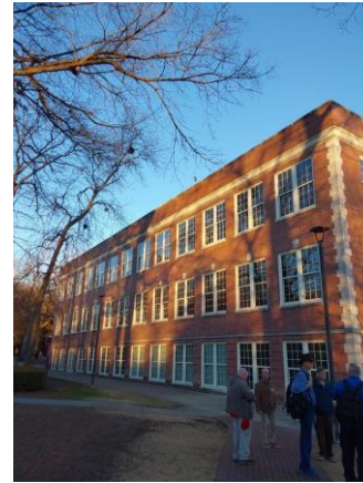
002103a 1/9/2023 Exterior brick and windows with adjacent walk West elevation
