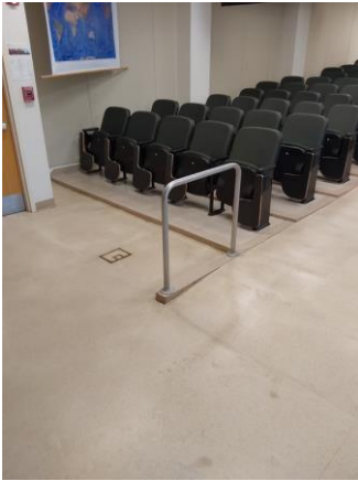
002037a 1/9/2023 Ramp railing separating ADA wheelchair spot Room 349
