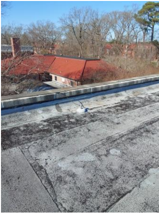
002001a 1/9/2023 Low parapet wall with lightning protection Roof
