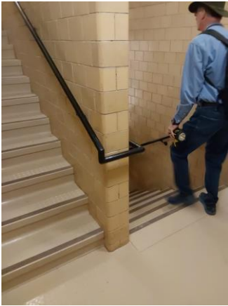
002022a 1/9/2023 Stair tower handrails Stair 3
