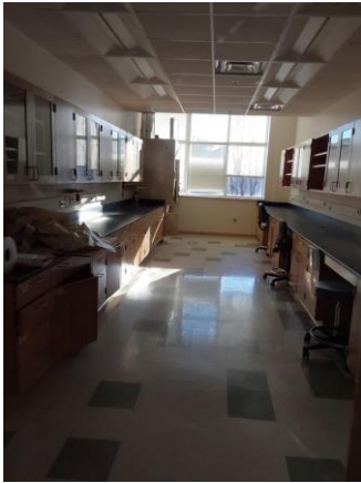
002073a 1/9/2023 Solid surface lab wall countertop Room 2213
