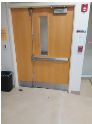
002040a 1/9/2023 Panic hardware of assembly area Room 349
