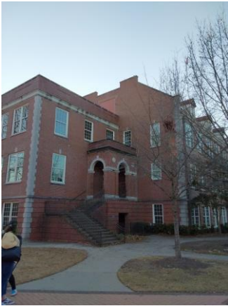
002108a 1/9/2023 Exterior brick and stone entry Northeast elevation
