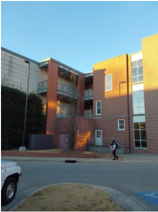
002106a 1/9/2023 Exterior brick and concrete panel Southeast elevation
