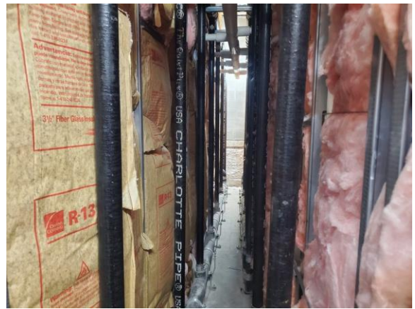
002033e 1/9/2023 Waste piping Plumbing chase 336
