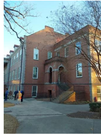
002101a 1/9/2023 Exterior brick and glazing Northwest elevation
