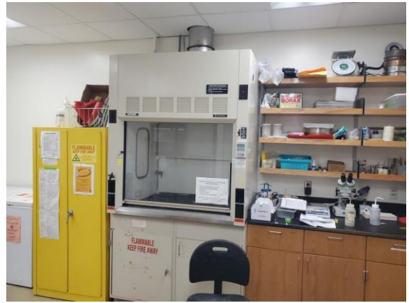
002043e 1/9/2023 Fume hood Room 384
