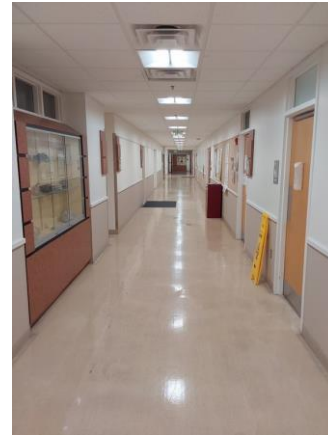
002083a 1/9/2023 Corridors with welded seam vinyl flooring Room 140
