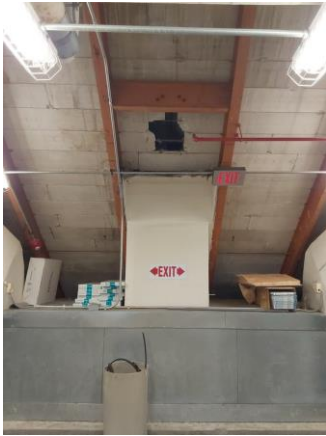
002013a 1/9/2023 Exit signage and roof attic Roof attic
