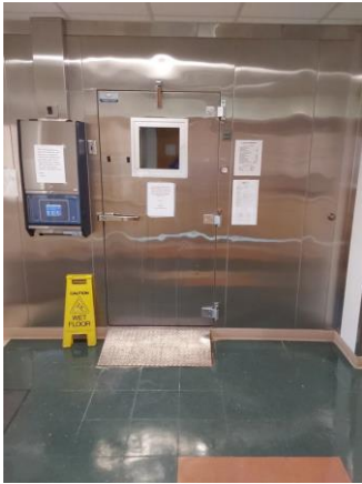
002061a 1/9/2023 Freezer with adjacent finishes Room 3202
