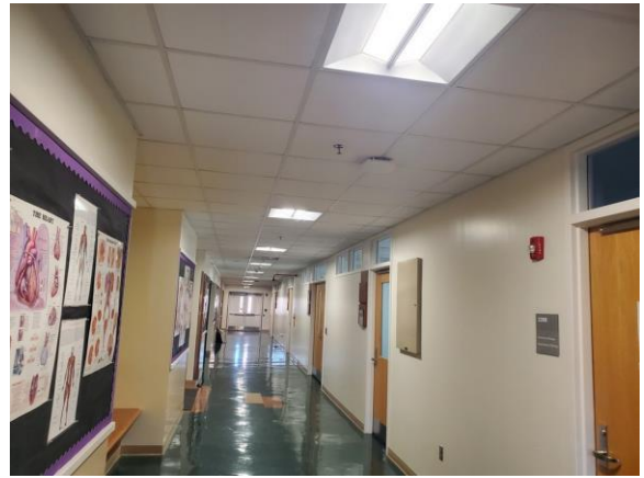
002046e 1/9/2023 Overview of corridor systems in 2008 addition Corridor 3202
