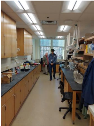
002049a 1/9/2023 Solid surface lab counter and laminate cabinets Room 382
