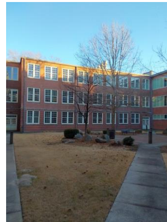
002099a 1/9/2023 Exterior brick and gutters Inside east wing
