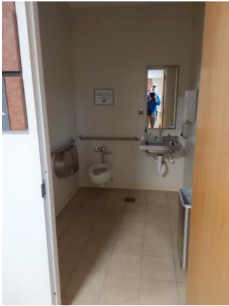
002074a 1/9/2023 Typical single-user restroom Room 204
