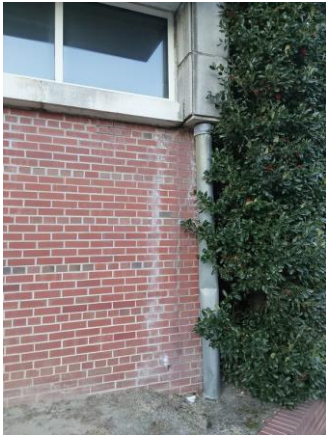
Water deposits on brick South elevation
