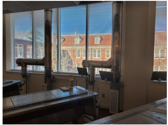
002047e 1/9/2023 Ductwork from AHU DDU-1 Room 3212
