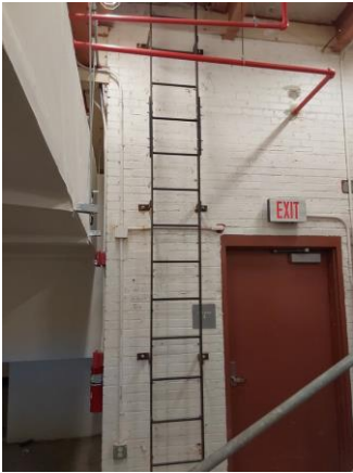
002017a 1/9/2023 Roof ladder to flat portion of tile roof Roof attic
