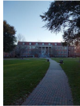
002109a 1/9/2023 Front approach to main entry North elevation
