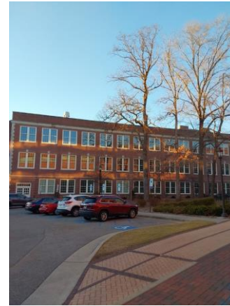
002107a 1/9/2023 Exterior brick, windows, and ADA entry East elevation
