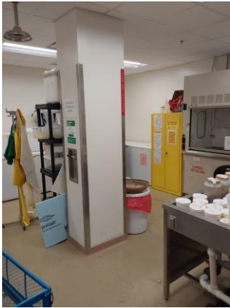
002050a 1/9/2023 Lab storage with epoxy flooring and ACT ceiling Room 384
