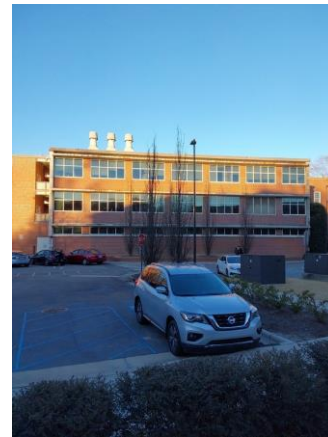
002105a 1/9/2023 Exterior brick and storefront glazing South elevation
