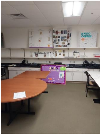
002067a 1/9/2023 Solid surface counter with wood casework Room 214
