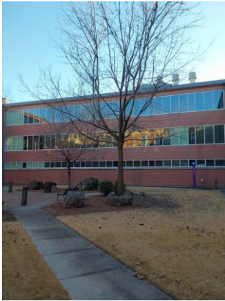
002096a 1/9/2023 Exterior brick and ribbon glazing Inside South wing
