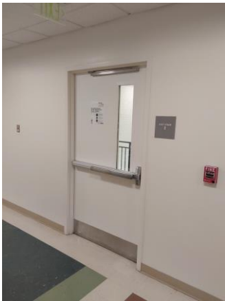
002057a 1/9/2023 Typical panic hardware Stair 2
