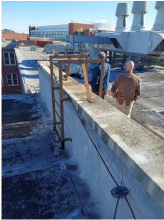
002005a 1/9/2023 Transfer ladder of parapet Roof
