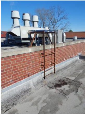
002008a 1/9/2023 Parapet transfer ladder Roof
