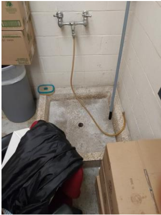
009007a 1/10/2023 Typical mop sink Room OA380
