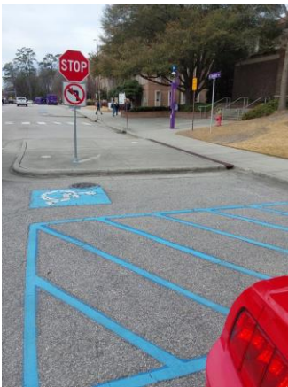
009118a 1/10/2023 Missing ADA curb cut South elevation
