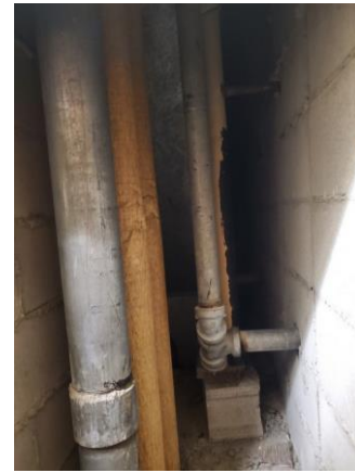
009014e 1/10/2023 Original supply and waste piping systems Third floor pipe chase
