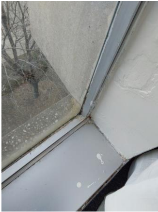
009023a 1/10/2023 Typical single-pane window Room OA304
