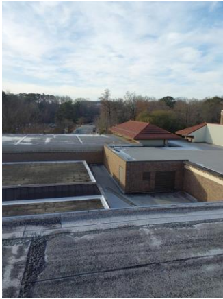
009004a 1/10/2023 Overall view of roofs Roof
