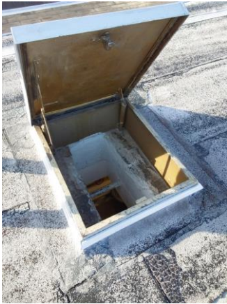
009005a 1/10/2023 Roof hatch with very small access Roof
