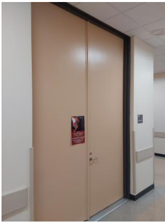
009056a 1/10/2023 Full height doors Room OB115
