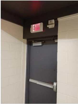
009035a 1/10/2023 Exit doors with appropriate signage and hardware Corridor B131
