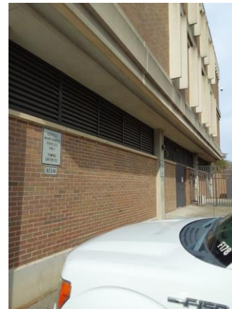
009125a 1/10/2023 Louvers and exterior hollow-metal door East elevation
