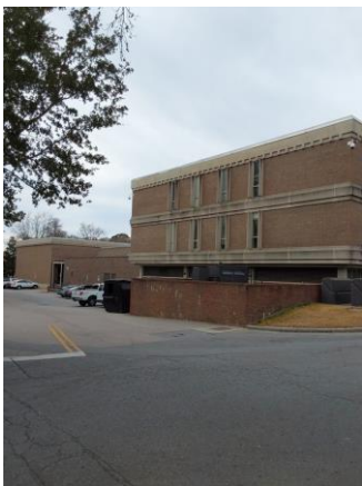
009100a 1/10/2023 Exterior brick, stone, and glazing East elevation
