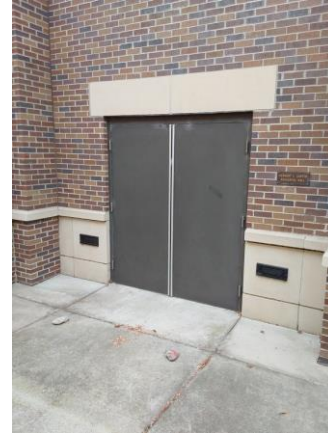
009109a 1/10/2023 Hollow-metal door West elevation
