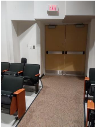
009084a 1/10/2023 Auditorium exit doors Room OC107
