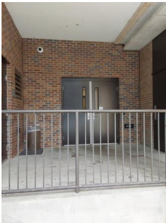
009124a 1/10/2023 Exterior hollow-metal doors East elevation
