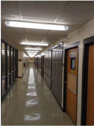
009022a 1/10/2023 Wall of lockers North corridor
