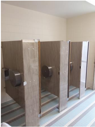
009026a 1/10/2023 Women's restroom partitions Room OA370B
