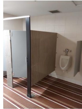
009081a 1/10/2023 Men's restroom fixtures Room OC108
