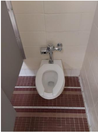
009010a 1/10/2023 Typical water closet Room OA381
