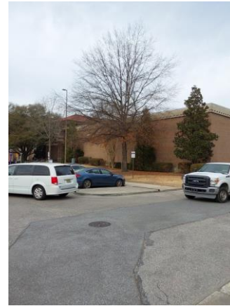
009117a 1/10/2023 Exterior brick and stone South elevation
