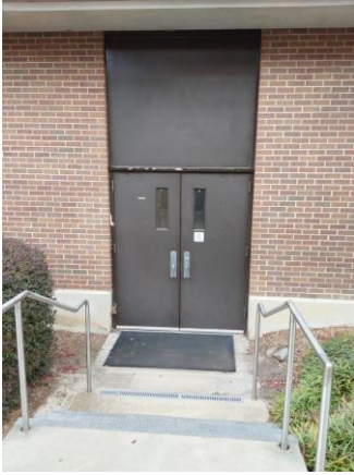
009108a 1/10/2023 Hollow-metal door the safety glass West elevation
