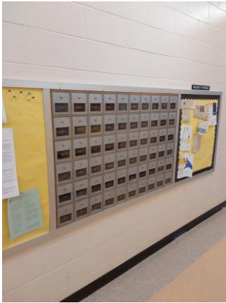
009044a 1/10/2023 Pass through mailboxes on corridor wall Room OA118
