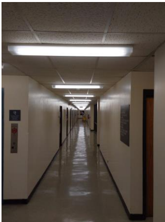
009006a 1/10/2023 Typical corridor with 9x9 ACT ceiling South corridor
