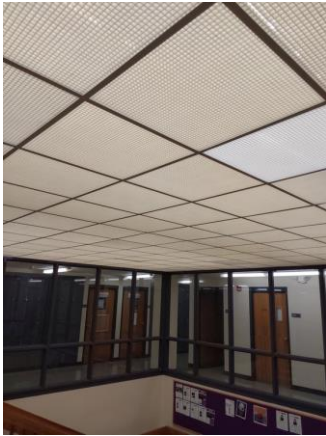
009017a 1/10/2023 Honeycomb light diffusers above central stair Central stair
