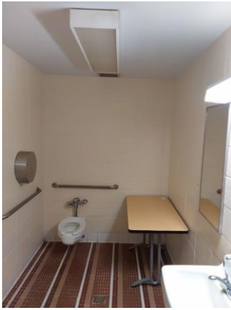
009049a 1/10/2023 Typical single-user restroom Room OC116A
