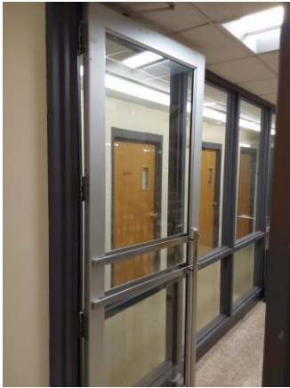
009034a 1/10/2023 Typical central stair doors Central stair
