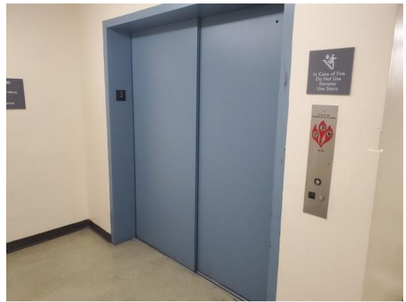
009003e 1/10/2023 Passenger elevator car doors Elevator
