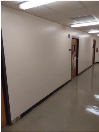
009029a 1/10/2023 Offices on east wall Second floor, room OA264
