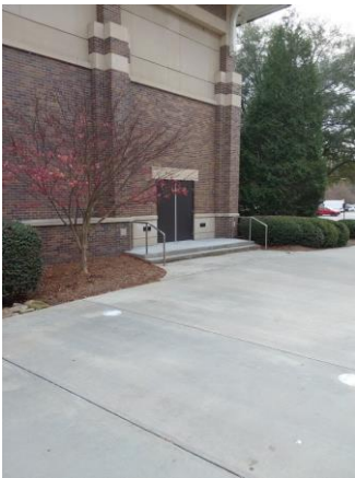
009112a 1/10/2023 Hollow-metal door west elevation West elevation
