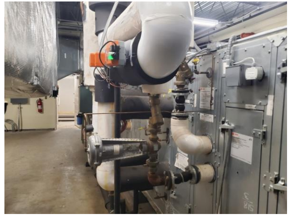
009032e 1/10/2023 Updated electronic Belimo actuating damper Mechanical B201
