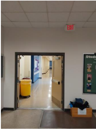
009050a 1/10/2023 Fire exit door with inset panic hardware Room 101
