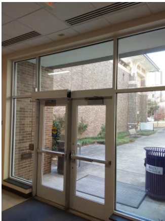
009054a 1/10/2023 Exterior entry doors with power door opener Room OB117
