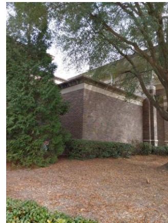
009113a 1/10/2023 Northwest corner brick and eave Southwest elevation
