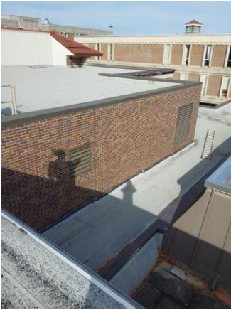
009077a 1/10/2023 Painted louvers West roof, mechanical room addition
