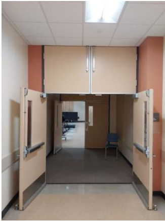
009055a 1/10/2023 Double egress doors with panic hardware Room OB110
