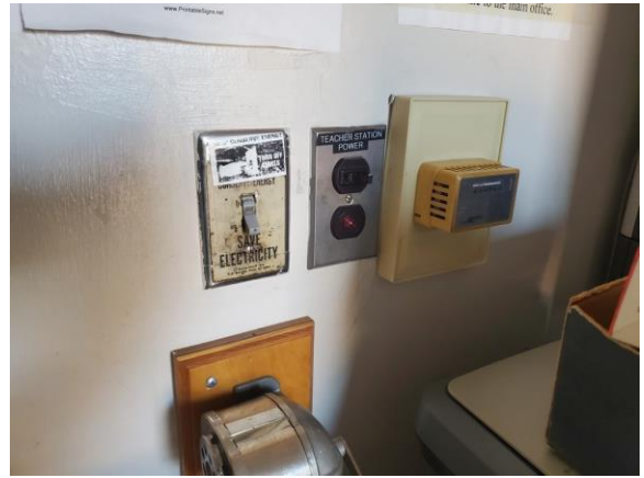
009011e 1/10/2023 Original light switch, outlet, and aged thermostat Room A300
