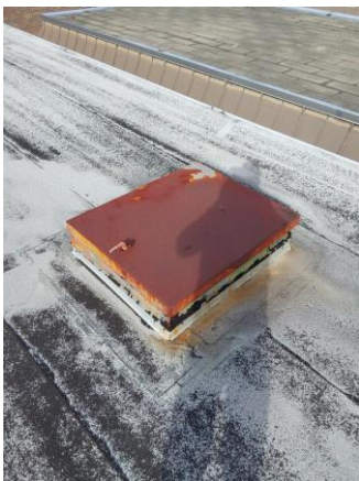
009075a 1/10/2023 Roof hatch South roof
