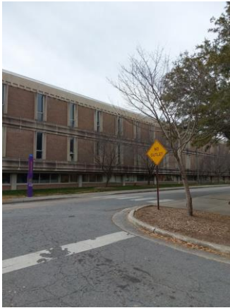
009102a 1/10/2023 Exterior brick, stone, and glazing North elevation
