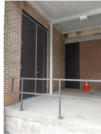
009123a 1/10/2023 Hollow-metal doors at loading dock East elevation
