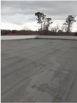
001A029a 1/12/2023 Southeast roof with parapet wall Roof
