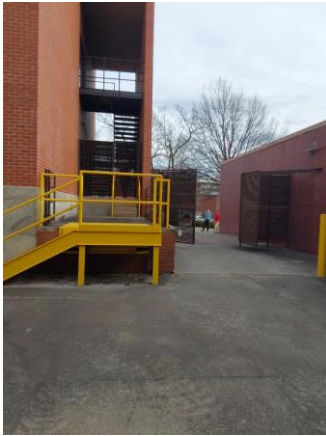
001A013a 1/12/2023 Exterior gates and stair South elevation
