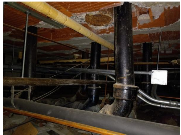
001A030e 1/12/2023 Overview of waste pipe and potable water pipe Crawlspace
