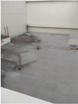
001A022a 1/12/2023 Basement roof Roof
