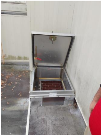
001A020a 1/12/2023 Roof hatch Roof
