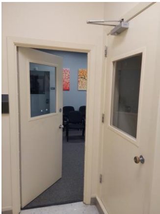
001A045a 1/12/2023 Doors with knob hardware and vision glass Room 205C
