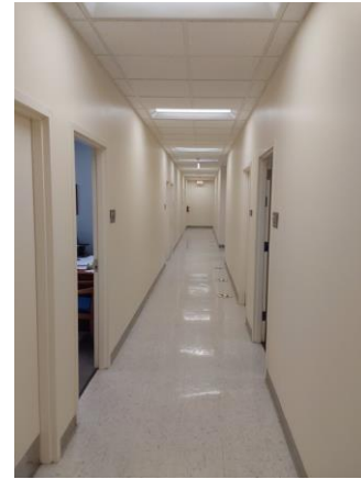
001A073a 1/12/2023 Lever hardware First floor south corridor
