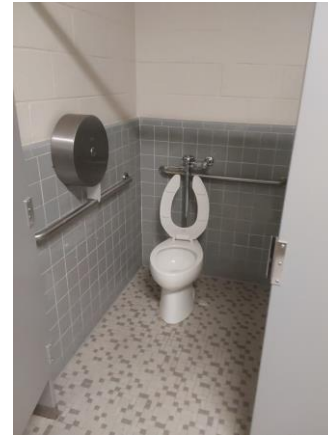
001A063a 1/12/2023 Typical water closet with grab bars Room 109a
