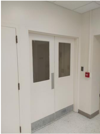
001A038a 1/12/2023 Stair tower doors Second floor south corridor
