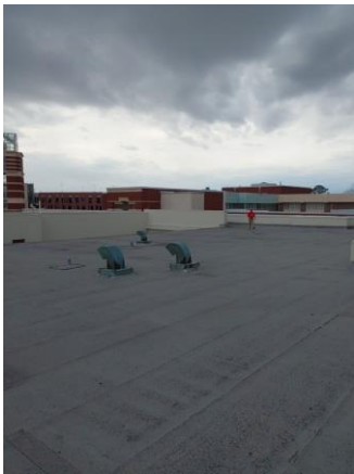
001A024a 1/12/2023 North roof with parapets Roof
