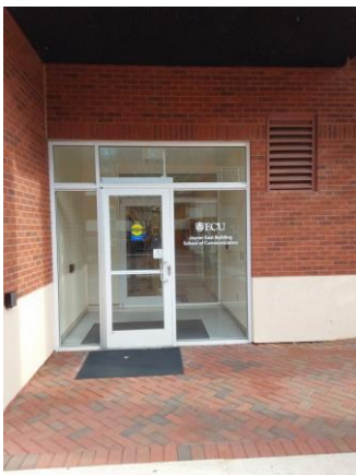
001A003a 1/12/2023 Exterior door power operator West elevation
