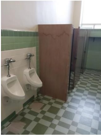
001A066a 1/12/2023 Urinals, partitions, and ceramic wall and floor finishes Room 108a
