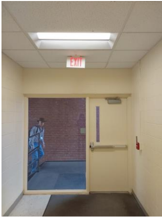
001A032a 1/12/2023 South corridor entrance Stair 2200
