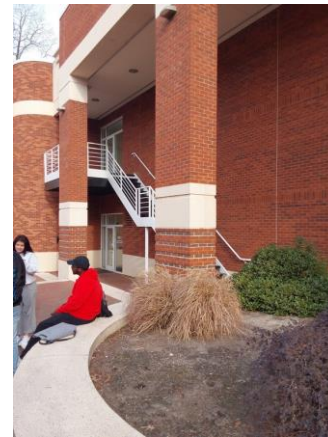
001A077a 1/12/2023 Exterior egress stair West elevation
