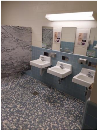
001A041a 1/12/2023 Ceramic wall and floor tile, painted upper wall, and wall-hung lavatories Room 206B
