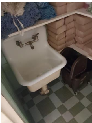
001A064a 1/12/2023 Mop sink Room 110
