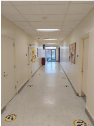
001A046a 1/12/2023 Corridor finishes Second floor west corridor
