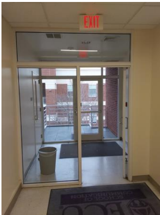
001A051a 1/12/2023 West second floor entrance Room 2097
