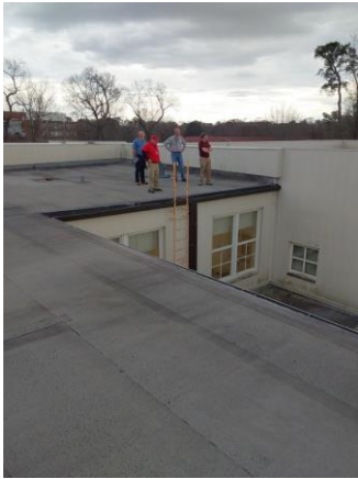
001A025a 1/12/2023 Gutter with downspout Roof
