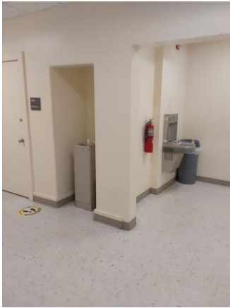
001A047a 1/12/2023 Two single height water fountains Second floor west corridor
