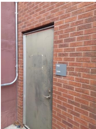
001A012a 1/12/2023 Exterior tunnel door South elevation
