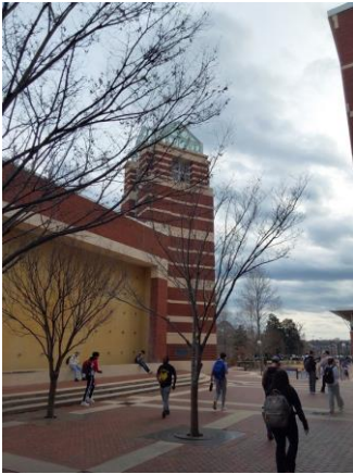
001A016a 1/12/2023 Clock tower glazing and brick Northwest elevation
