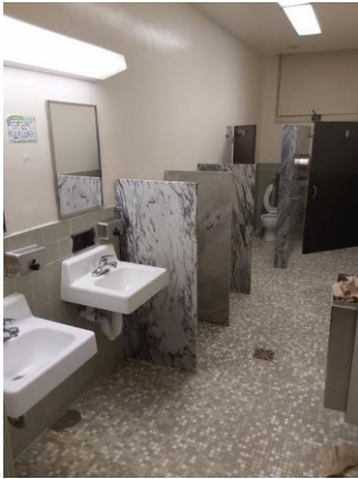
001A040a 1/12/2023 Wall-hung lavatories and partitions Room 206A
