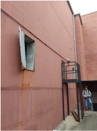
001A017a 1/12/2023 Replace water wall doors West wall
