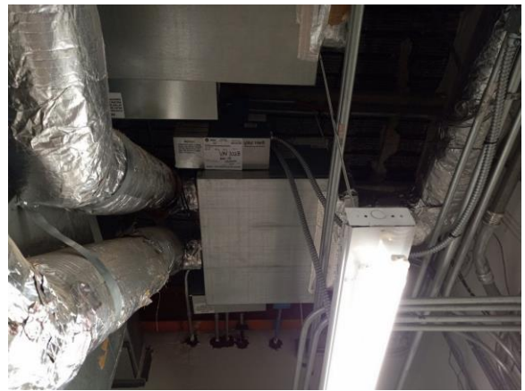
001A045e 1/12/2023 Variable air volume terminal assembly Mechanical 098
