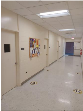
001A037a 1/12/2023 Knob hardware Second floor south corridor
