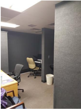
001A058a 1/12/2023 Typical sound booth with acoustic wall finish Room 105H
