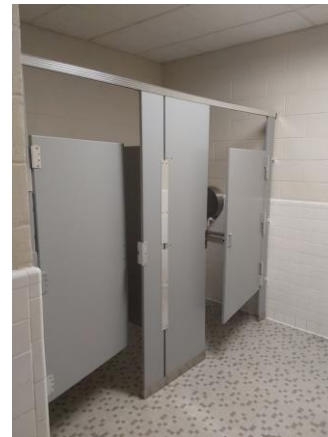
001A071a 1/12/2023 Plastic partitions Room 109B
