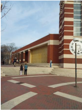
001A001a 1/12/2023 Water wall and brick pavers West elevation
