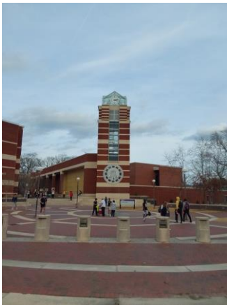
001A015a 1/12/2023 Clock tower glazing and brick Southwest elevation
