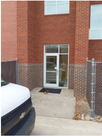
001A007a 1/12/2023 Exterior powder-coated aluminum door East elevation
