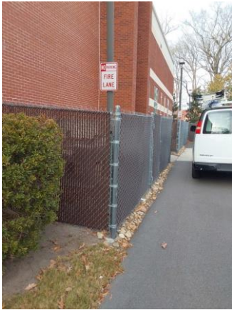
001A008a 1/12/2023 Exterior chain link fence East elevation
