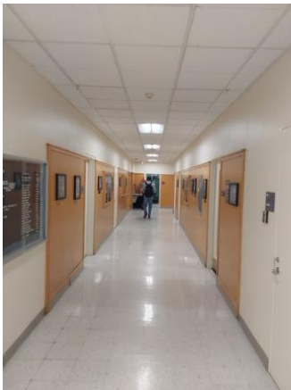
001A054a 1/12/2023 Corridor finishes First floor west corridor
