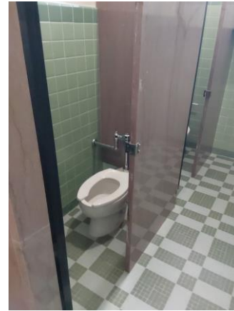
001A067a 1/12/2023 Side mounted water closets Room 108a
