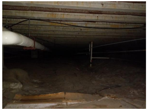
001A057e 1/12/2023 Overview of piping systems Crawlspace
