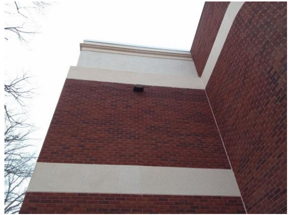
001A059e 1/12/2023 Surface mounted light fixture with LED lamps Exterior
