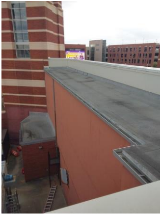
001A028a 1/12/2023 Gutter with downspouts Roof
