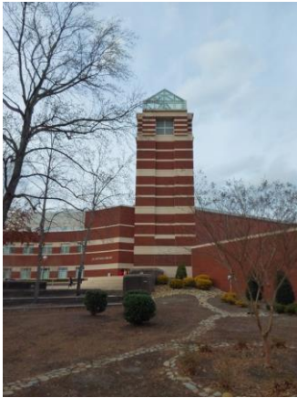
001A014a 1/12/2023 Clock tower with glazing and brick Southeast elevation
