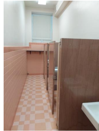
001A069a 1/12/2023 Toilet partitions and pink ceramic finishes Room 108B
