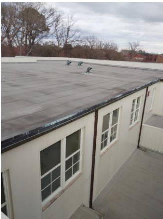
001A030a 1/12/2023 Roof with downspouts Roof
