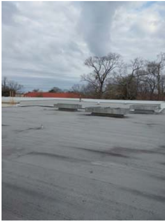
001058a 1/12/2023 Modified bitumen with parapet wall Northeast roof
