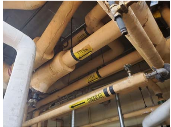
Original steam and condensate pipe Mechanical B909
