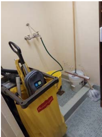
001075a 1/12/2023 Mop sink Room 2902
