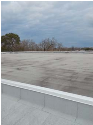
001009a 1/12/2023 Roof showing parapet Northwest roof
