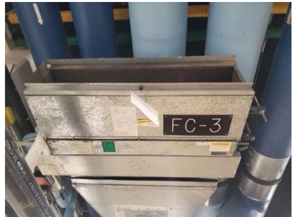
Fan coil FC-3 Mechanical B901
