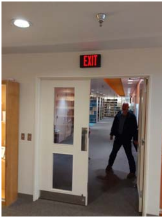
001035a 1/12/2023 Exit doors Room 3048
