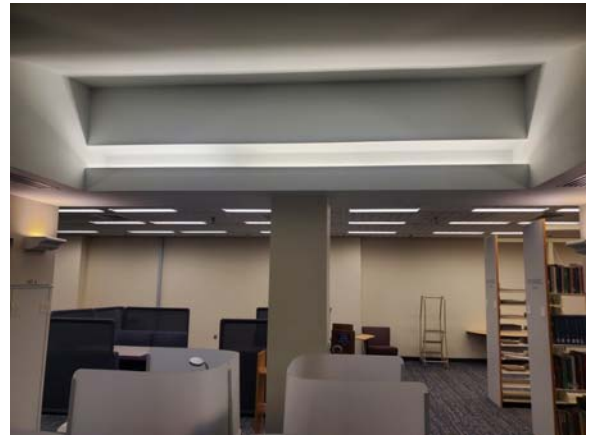
001044e 1/12/2023 Overview of stack systems and lighting Stacks 3023
