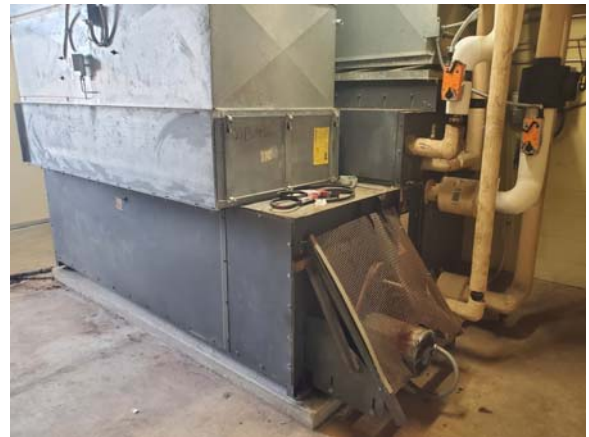
001054e 1/12/2023 AHU-5 with original motor and shaft Mechanical 2900
