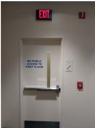
001030a 1/12/2023 Typical fire stair door Room 4002
