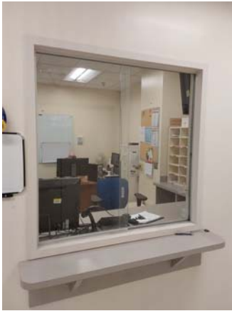
001082a 1/12/2023 Pass through window Room 1080
