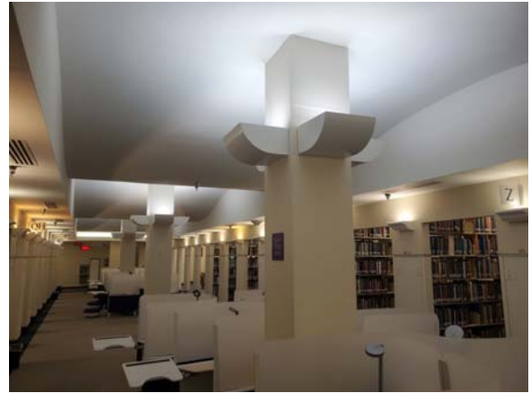
001043e 1/12/2023 Overview of stack systems and lighting Stacks 3023
