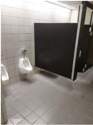
001047a 1/12/2023 Urinals and toilet partitions Room 3008
