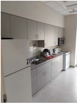
001068a 1/12/2023 Break room casework with sink Room 2408
