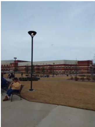
001126a 1/12/2023 Brick and stone exterior with glazing South elevation
