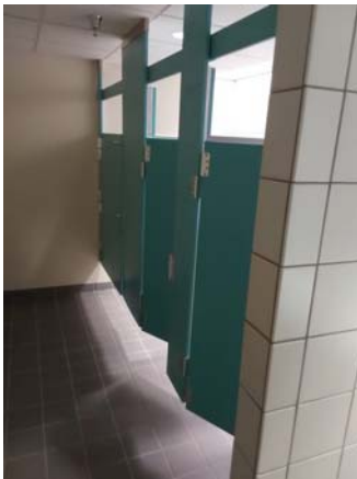
001018a 1/12/2023 Restroom partitions Room 4004
