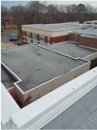
001010a 1/12/2023 Lower portion of roof Middle roof
