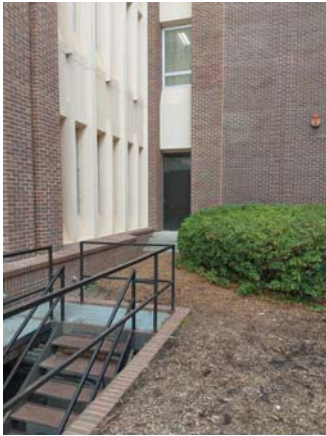
001141a 1/12/2023 Exterior hollow-metal door North elevation
