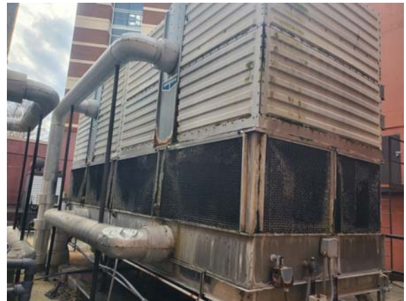
001120e 1/12/2023 Aged cooling tower CT2 cells A and B Site
