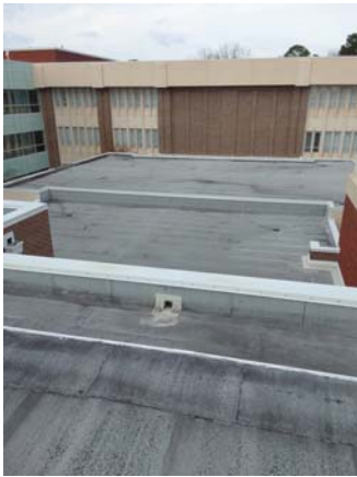
001059a 1/12/2023 Modified bitumen roof Lower middle roof
