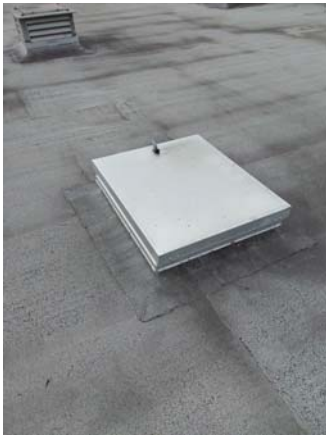
001008a 1/12/2023 Roof hatch Northwest roof
