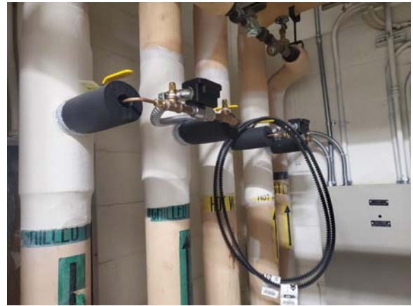
001041e 1/12/2023 Updated controls for hydronic distribution Mechanical 3903
