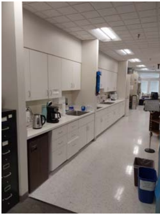
001080a 1/12/2023 Casework with three sinks Room 1200
