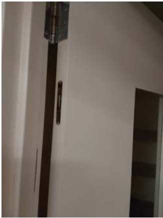
001056a 1/12/2023 Rated stack room doors with safety glass Room 3115
