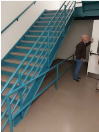
001031a 1/12/2023 Cane rail Stair 2
