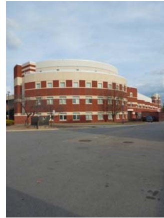
001142a 1/12/2023 Exterior brick and glazing Southwest elevation
