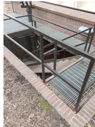
001140a 1/12/2023 Mechanical well with painted hollow-metal door North elevation
