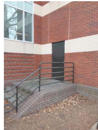
001134a 1/12/2023 Exterior hollow-metal door North elevation
