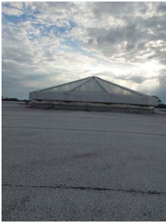
001002a 1/12/2023 Glass skylight Rotunda roof
