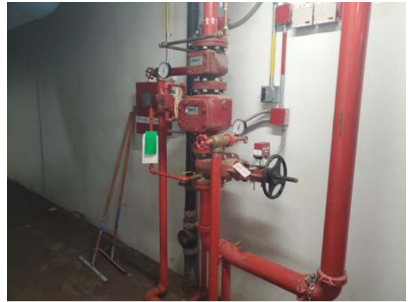
Preaction fire suppression system for Media Center Mechanical B901
