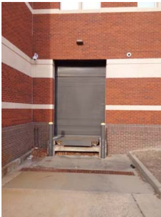
001145a 1/12/2023 Exterior overhead roll up door South elevation
