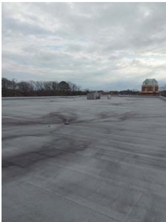
001006a 10/12/2023 Lower portion of south roof Rotunda roof
