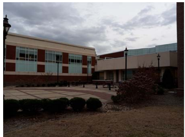
001129e 1/12/2023 Pole-mounted exterior light fixtures Site
