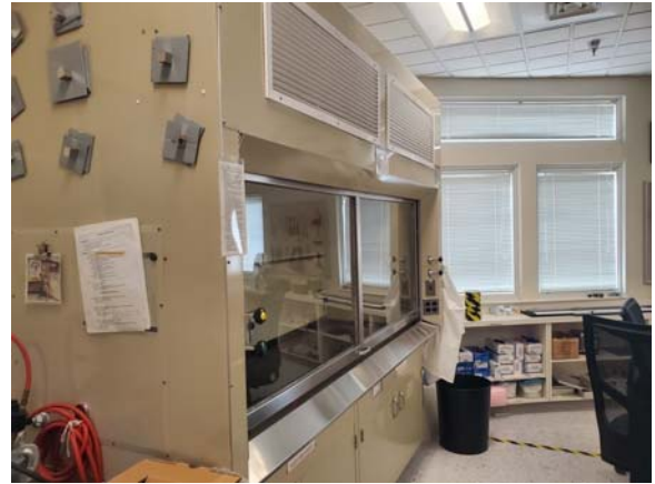
001058e 1/12/2023 Fume hood Tech Services 1300
