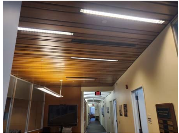
001067e 1/12/2023 Renovated space with updated lighting Office suite 1001
