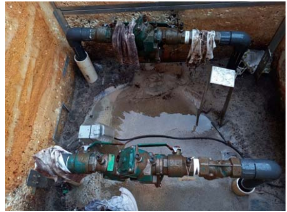
001127e 1/12/2023 Aged backflow devices Exterior
