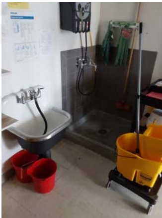
001045a 1/12/2023 Two mop sinks and ACM vinyl tile Room 3908
