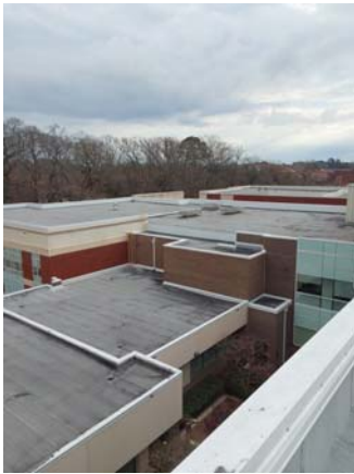
001011a 1/12/2023 East roof overall Northeast roof
