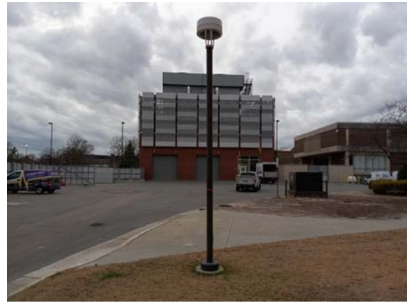
001125e 1/12/2023 Pole mounted exterior light fixture Site
