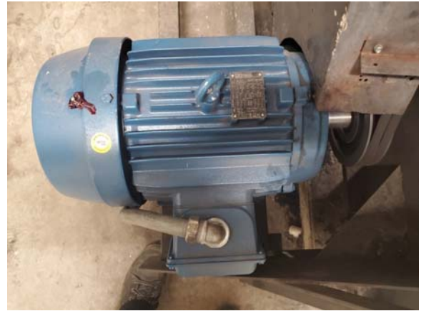
001040e 1/12/2023 Updated motor and shaft assembly on AHU-8 Mechanical 3903
