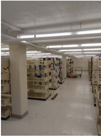
001127a 1/12/2023 Basement record storage showing finishes Room B001
