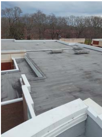
001012a 1/12/2023 East roof smoke hatches Northeast roof
