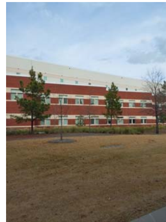
001146a 1/12/2023 South sawtooth exterior brick and glazing South elevation
