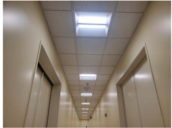
001061e 1/12/2023 Overview of corridor systems Corridor 1092
