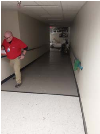
001123a 1/12/2023 Large service ramp with vinyl sheet Room B004
