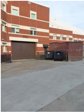
001143a 1/12/2023 Overhead exterior roll-up door and brick South elevation
