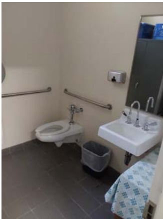
001105a 1/12/2023 Single-use restroom Room 1047
