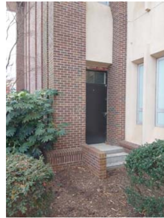
001138a 1/12/2023 Exterior hollow-metal door North elevation
