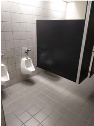
001016a 1/12/2023 Men's restroom with fixtures and partition shown Room 4005
