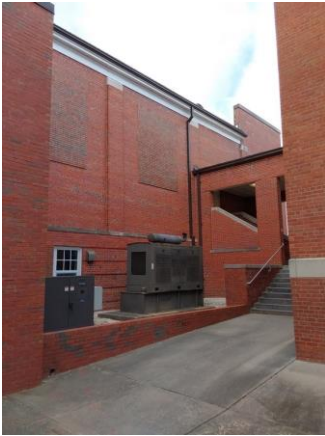
033087a 1/10/2023 Exterior brick and glazing East elevation
