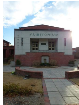
033084a 1/10/2023 Exterior brick, stone, and glazing North elevation
