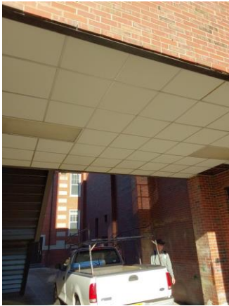
033034a 1/10/2023 Portico soffit 2-E-1
