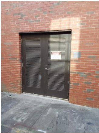
033041a 1/10/2023 Exterior electrical room to shop Room 127
