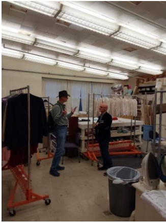
033061a 1/10/2023 Asbestos acoustic ceiling tile and 9x9 tile Room 112
