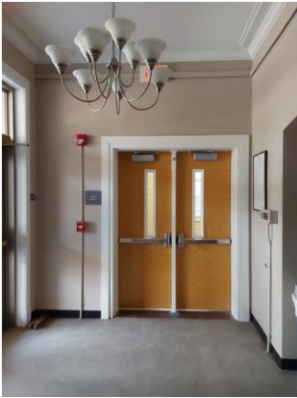
033020a 1/10/2023 Stairwell doors with panic hardware and safety glass Room 201
