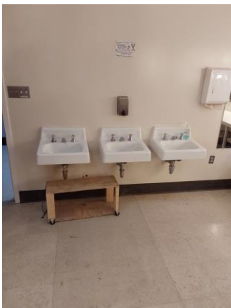
033048a 1/10/2023 Dressing room sinks Room 125
