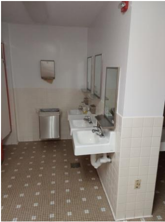
033068a 1/10/2023 Wall-hung lavatories and ceramic tile Room 108
