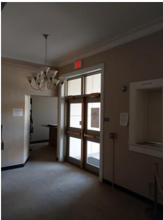
033018a 1/10/2023 Auditorium entrance doors with panic hardware Room 201
