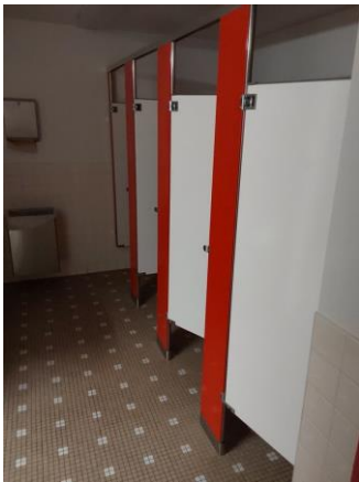
033066a Toilet partitions Room 108 1/10/2023
