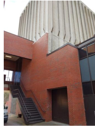
033090a 1/10/2023 Exterior brick, glazing, and doors East elevation
