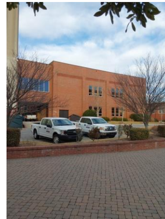
033092a 1/10/2023 Exterior brick and glazing with drive Shop south elevation
