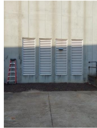
033076a 1/10/2023 Exterior mechanical louvers South elevation
