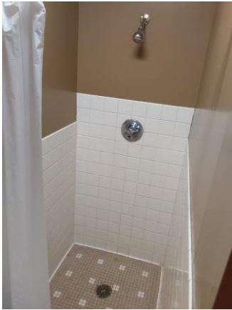
033056a 1/10/2023 Shower Room 129
