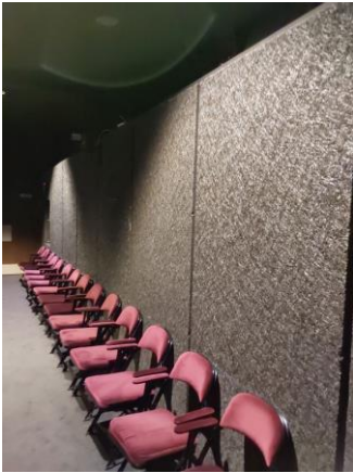
033016a 1/10/2023 Acoustic panel wall Room 209
