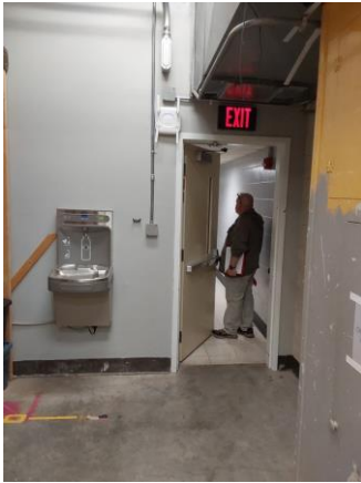
033047a 1/10/2023 Exit door with panic hardware, exit signage, and single height water fountain Room 131
