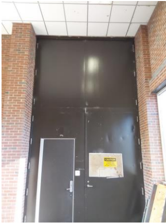
033023a 1/10/2023 Painted exterior shop door 2-E-1
