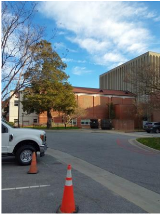
033081a 1/10/2023 Exterior brick, stone, and glazing West elevation
