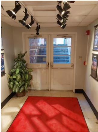
033062a 1/10/2023 Exterior door with old panic hardware Room 106
