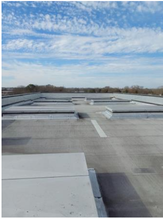
033002a 1/10/2023 Roof photo showing smoke vents Stage roof
