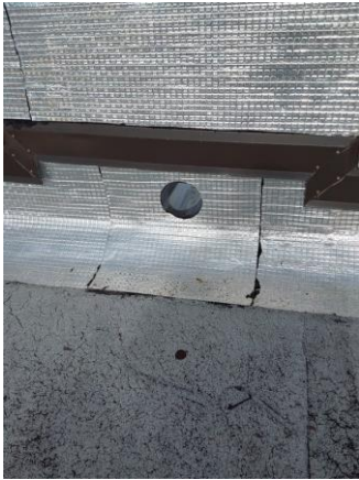
033001a 1/10/2023 Overflow scupper of stage roof Stage roof
