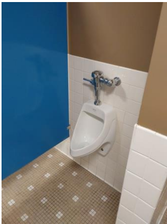
033057a 1/10/2023 Urinal and ceramic finishes Room 129
