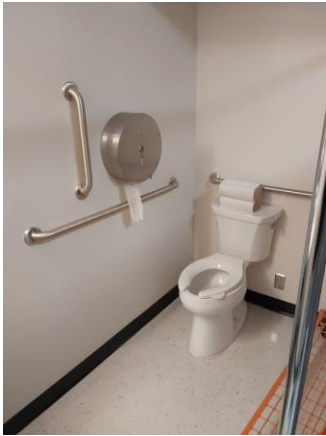
033007a 1/10/2023 Dressing room water closet Room 210
