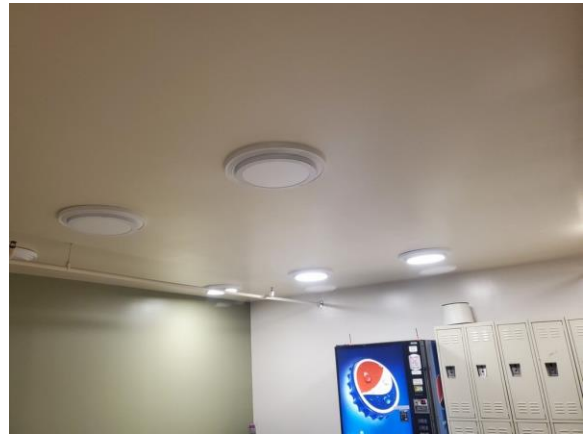
033050e 1/10/2023 Updated LED lighting Room 115
