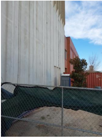
033077a 1/10/2023 Exterior concrete wall South elevation
