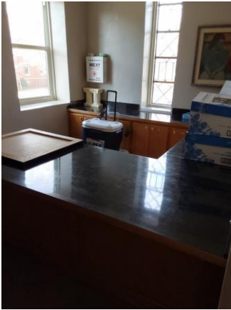
033019a 1/10/2023 Large laminate case work inside Room 202
