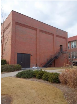
033093a 1/10/2023 Exterior brick and hollow-metal doors Shop east elevation
