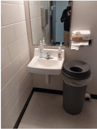
033008a 1/10/2023 Dressing room sink Room 213
