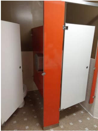
033052a 1/10/2023 Toilet partitions Room 128
