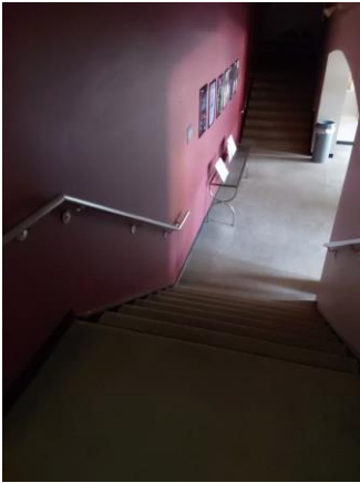
033017a 1/10/2023 Auditorium entry stair Room 204
