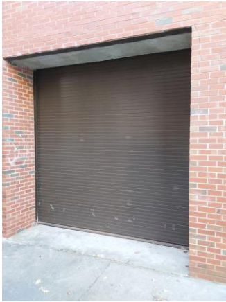
033044a 1/10/2023 Overhead coiling door Room 131
