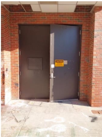
033036a 1/10/2023 Exterior shop door 2-E-1
