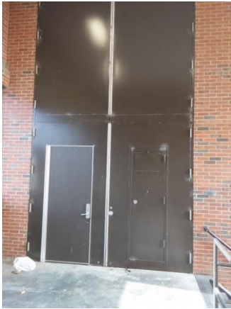
033022a 1/10/2023 Painted exterior stage door 2-E-1
