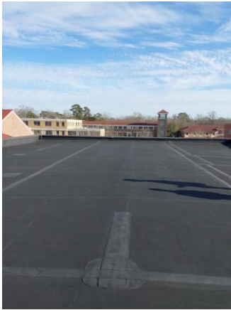
033029a 1/10/2023 EPDM roof with parapet wall 2-E-1
