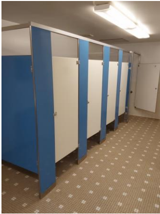
033064a Toilet partitions Room 105 1/10/2023
