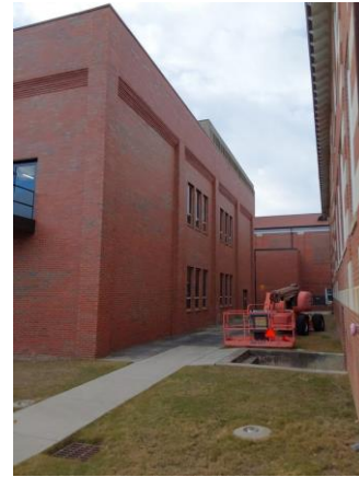
033094a 1/10/2023 Exterior brick and glazing Shop north elevation
