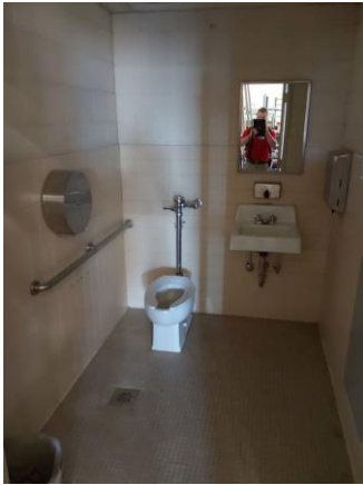
033025a 1/10/2023 Shop restroom 2-E-1
