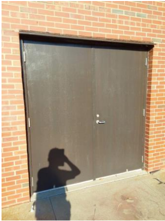
033040a 1/10/2023 Exterior shop door with inset Room 101
