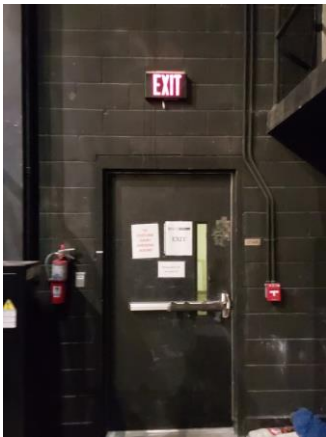
033009a 1/10/2023 Exit door with signage, panic hardware, and safety glass Room 209
