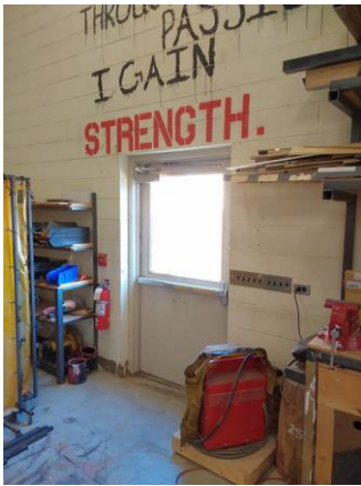
033032a 1/10/2023 Exit door with panic hardware 2-E-1
