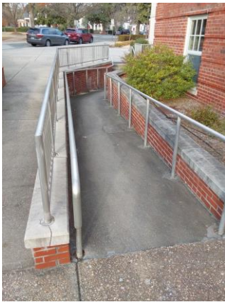
033083a 1/10/2023 ADA ramp West elevation
