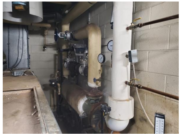
033054e 1/10/2023 Updated isolation valves on heat exchanger Mechanical 126
