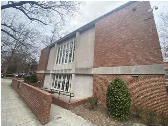
047031a 1/26/2023 Brick facade, glazing, glass entry doors Exterior
