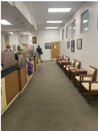
047005a 1/26/2023 Acoustical tile ceiling, painted walls, carpeting, counter Work area
