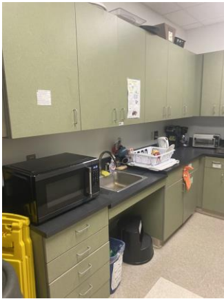
047007a 1/26/2023 Casework with a sink, vinyl tile floor, acoustical tile ceiling Break area
