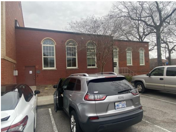
047033a 1/26/2023 Brick facade, glazing, hollow metal doors Exterior
