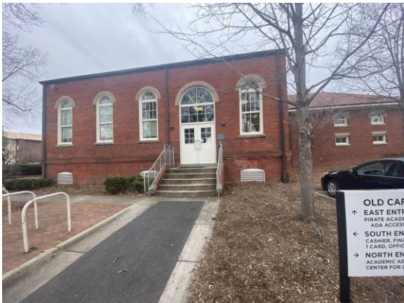
047035a 1/26/2023 Brick facade, glazing, metal and glass doors Exterior
