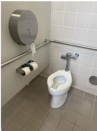
047020a 1/26/2023 Tile walls and floor, accessible water closet Restroom
