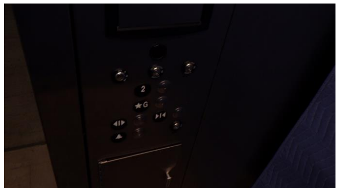
047015e 1/26/2023 Elevator controls Elevator 1 cab
