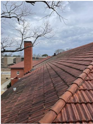
047043a 1/26/2023 Clay tile roof Roof
