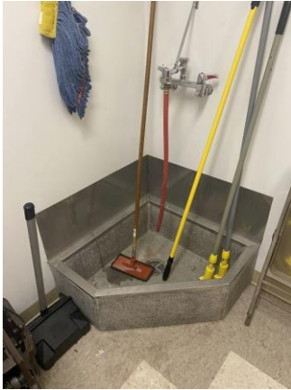
047025a 1/26/2023 Concrete utility sink Custodial closet
