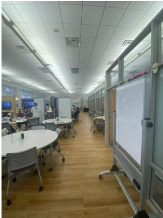
047017a 1/26/2023 Acoustical tile ceiling, wood flooring Tutor room
