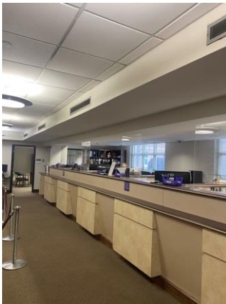
047030a 1/26/2023 Acoustical tile ceiling, carpeting, counter Work area
