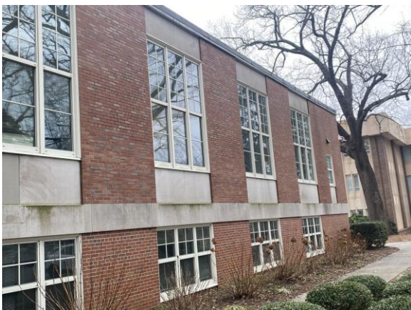
047039a 1/26/2023 Brick facade, glazing Exterior
