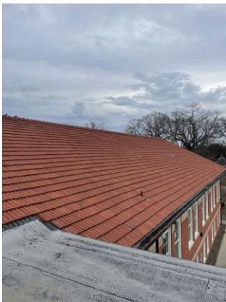
047042a 1/26/2023 Clay tile roof Roof
