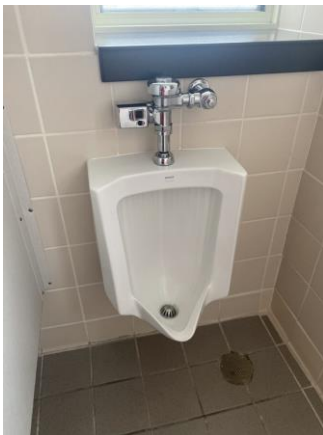
047021a 1/26/2023 Tile walls and floor, urinal Restroom
