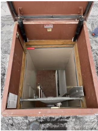
047044a 1/26/2023 Roof hatch Roof
