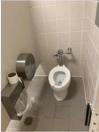
047019a 1/26/2023 Tile walls and floor, toilet with hands-free flush valve Restroom
