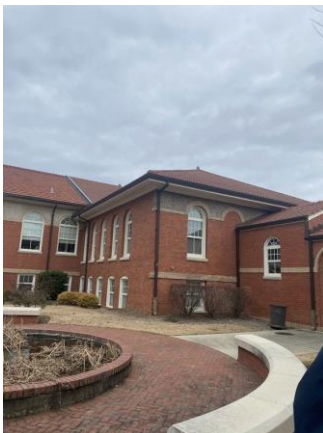
047027a 1/26/2023 Brick facade, clay tile roof, glazing Courtyard
