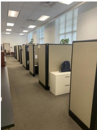
047006a 1/26/2023 Acoustical tile ceiling, painted walls, carpeting Work area
