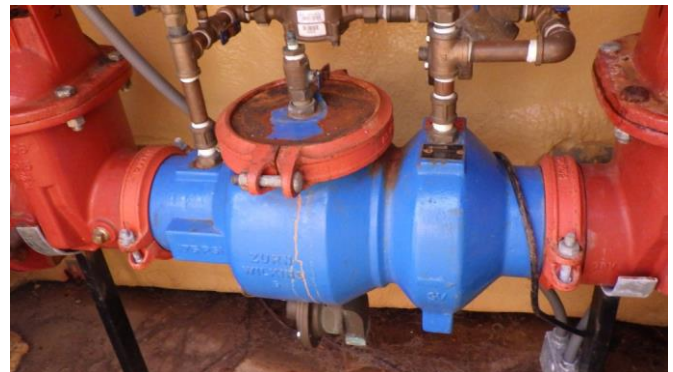
047024e 1/26/2023 Fire suppression system backflow preventer North side
