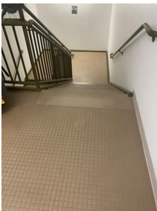
047012a 1/26/2023 Vinyl treads and landings, metal railings Stairwell
