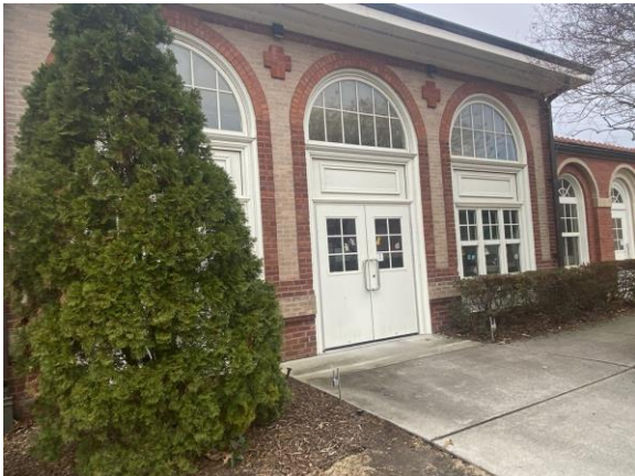
047037a 1/26/2023 Brick facade, glazing, metal and glass doors Exterior
