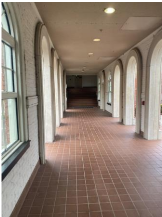
047023a 1/26/2023 Painted brick, quarry tile Breezeway
