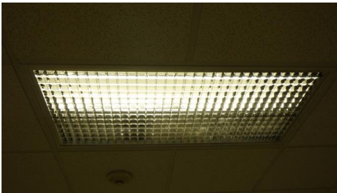
047073e 1/26/2023 Open parabolic lay-in fluorescent interior light fixture Corridor G100A
