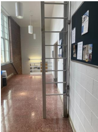
047002a 1/26/2023 CMU walls, terrazzo floor, roof ladder Corridor
