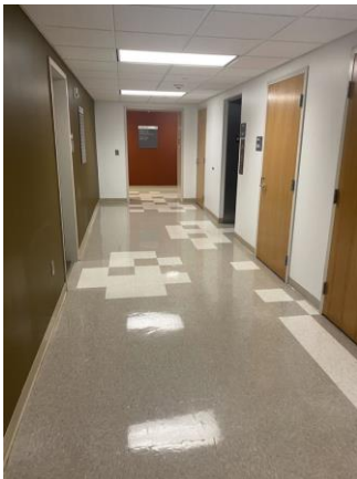
047029a 1/26/2023 Acoustical tile ceiling, vinyl tile floor, wood doors Corridor
