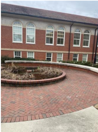
047026a 1/26/2023 Brick facade, clay tile roof, glazing Courtyard
