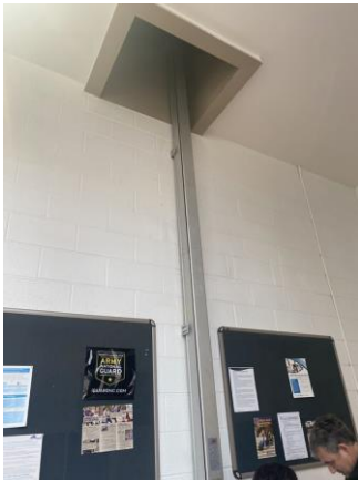
047001a 1/26/2023 Painted CMU wall and painted ceiling, roof ladder Corridor
