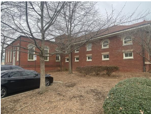
047036a 1/26/2023 Brick facade, glazing Exterior
