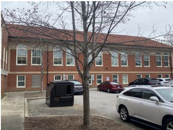
047032a 1/26/2023 Brick facade, glazing, mission tile roof Exterior
