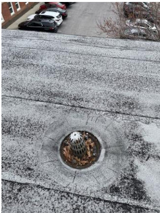
047041a 1/26/2023 Modified bitumen roof Roof
