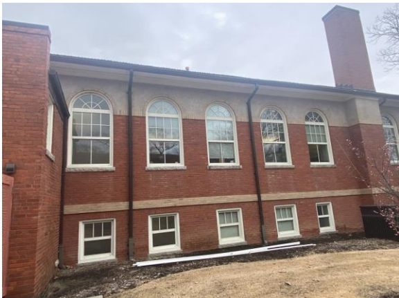
047038a 1/26/2023 Brick facade, glazing, tile roof, gutters and downspouts Exterior
