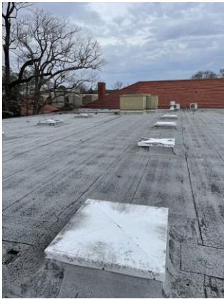
047040a 1/26/2023 Modified bitumen roof Roof
