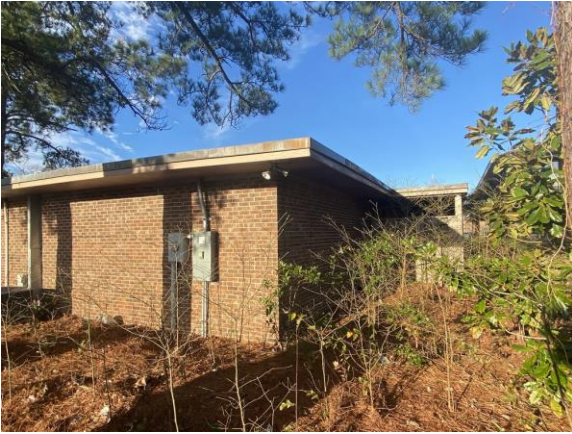
118022a 1/26/2023 Brick exterior and glazing Exterior
