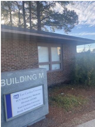
118016a 1/26/2023 Brick exterior, glazing, and signage Exterior
