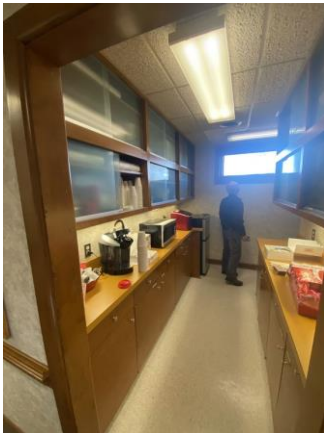
118005a 1/26/2023 VCT, ACT, and casework Break area
