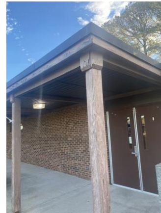
118017a 1/26/2023 Brick exterior, hollow-metal doors, and wood posts Exterior
