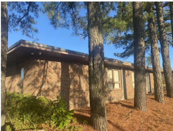
118020a 1/26/2023 Brick exterior and glazing Exterior
