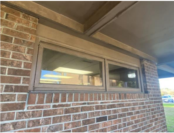
118024a 1/26/2023 Wood-framed, single-pane windows Exterior
