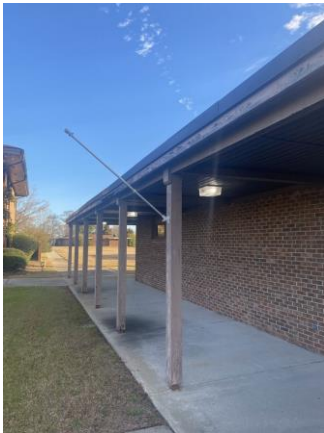
118018a 1/26/2023 Brick exterior, wood posts, and extended roof awning Exterior
