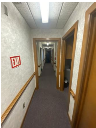
118003a 1/26/2023 ACT, wall covering, and carpet Corridor
