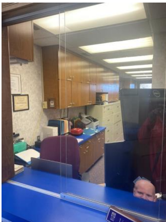
118015a 1/26/2023 Countertop and casework Reception window
