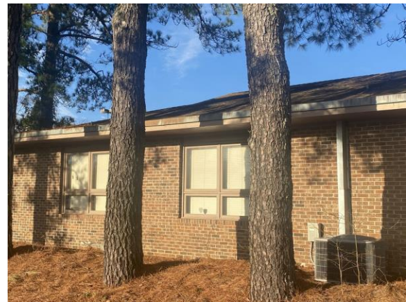
118021a 1/26/2023 Brick exterior and glazing Exterior
