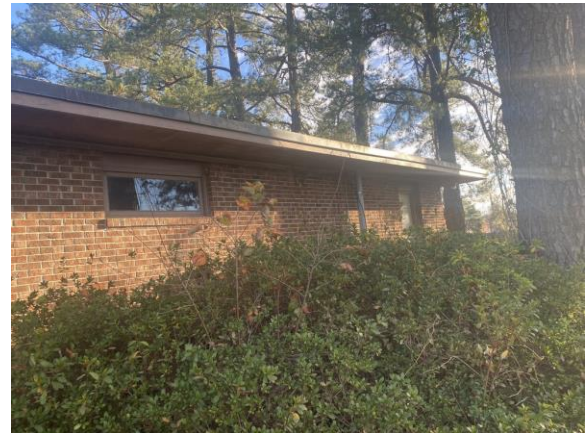
118019a 1/26/2023 Brick exterior and glazing Exterior
