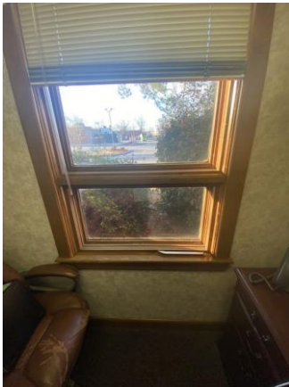
118004a 1/26/2023 Wood-framed, single-pane window Office
