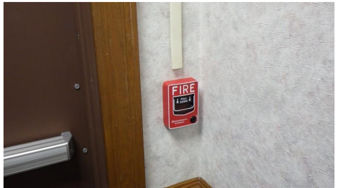
118011e 1/26/2023 Manual fire alarm device Side exit door
