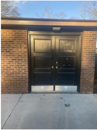
119018a 1/26/2023 Brick exterior, wood doors with knob hardware Exterior
