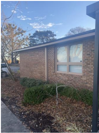
119014a 1/26/2023 Brick exterior and glazing Exterior
