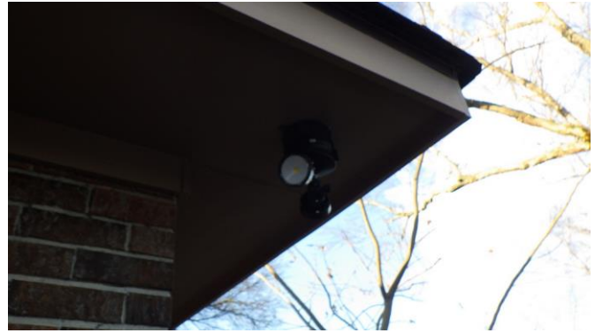
119004e 1/26/2023 Incandescent floodlight Exterior corner soffit
