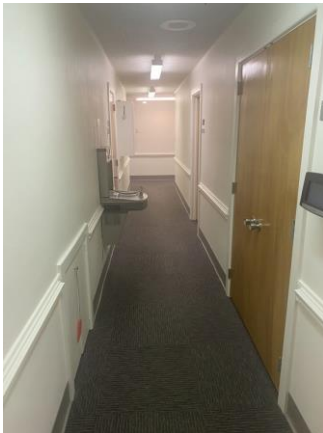
119005a 1/26/2023 Painted walls and ceiling, carpeting, wood doors with knob Corridor
