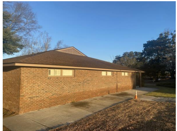
119017a 1/26/2023 Brick exterior, glazing, asphalt shingle roof Exterior
