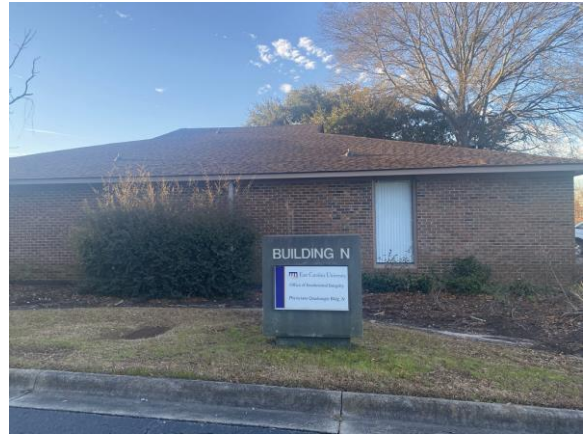
119019a 1/26/2023 Brick exterior, glazing, asphalt shingle roof Exterior
