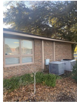
119015a 1/26/2023 Brick exterior and glazing Exterior
