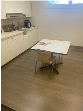
119007a 1/26/2023 Painted walls, glazing, casework, vinyl plank floor Break room
