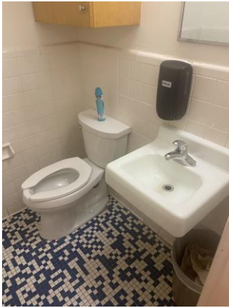
119001a 1/26/2023 Tile walls and floor, wall-hung lavatory and tank-type toilet Restroom
