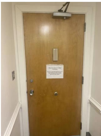
119012a 1/26/2023 Wood door with knob hardware Corridor
