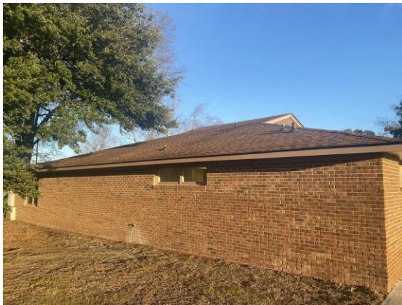
119016a 1/26/2023 Brick exterior, glazing, asphalt shingle roof Exterior
