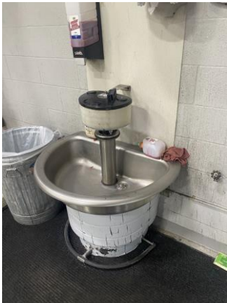
258029a 1/25/2023 Gang lavatory Wash bay
