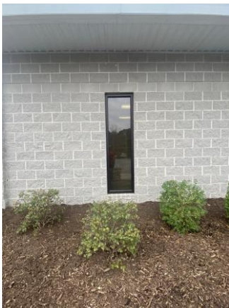
258021a 1/25/2023 Aluminum and glass glazing Exterior of office
