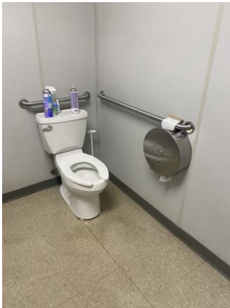
258010a 1/25/2023 Fiberglass reinforced panels Restroom
