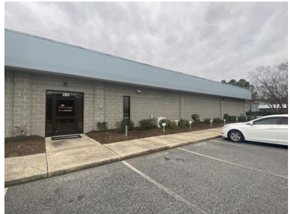
258030a 1/25/2023 Split faced cement block exterior wall Entrance
