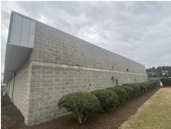
258020a 1/25/2023 Split faced cement block exterior wall Exterior of office
