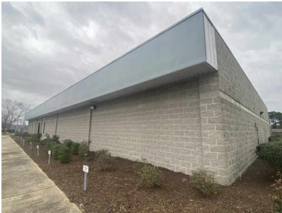
258022a 1/25/2023 Metal panel facades Exterior of office
