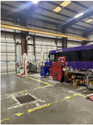
258007a 1/25/2023 Sealed concrete floor Wash bay
