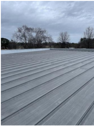
258001a 1/25/2023 Standing-seam metal roofing Office roof
