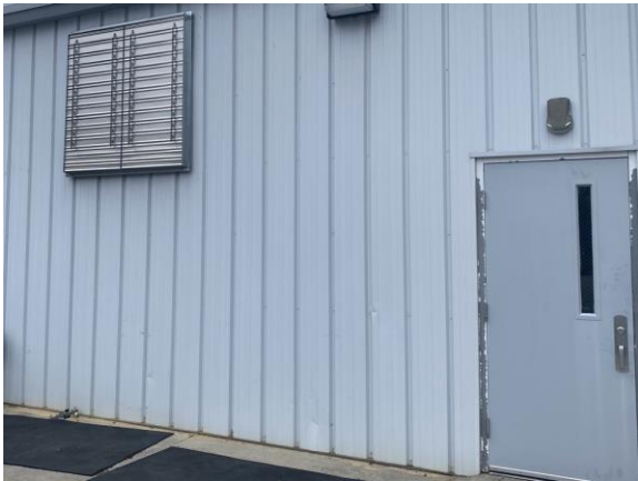
258023a 1/25/2023 Corrugated metal siding Wash bay
