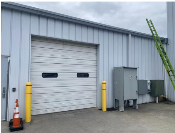
258018a 1/25/2023 Metal panel garage door Warehouse
