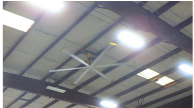
258011e 1/25/2023 Ceiling fan Warehouse parts area
