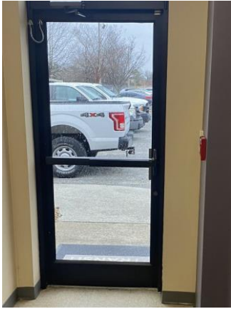
258016a 1/25/2023 Aluminum and glass exterior door Secondary office exit
