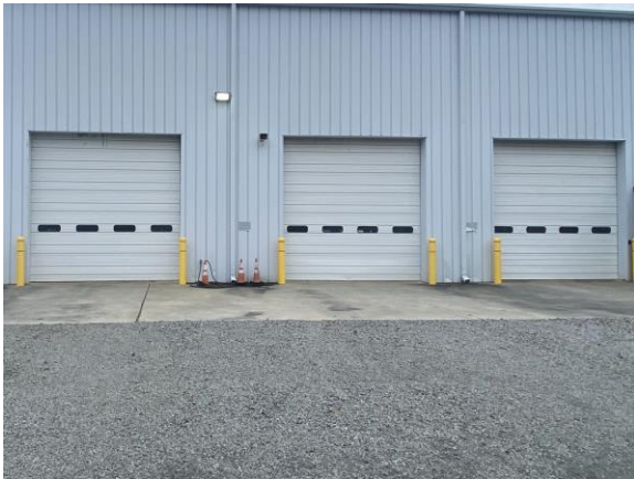
258019a 1/25/2023 Metal panel garage doors Wash bay
