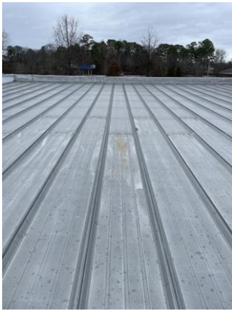
258002a 1/25/2023 Standing-seam metal roofing Wash bay roof
