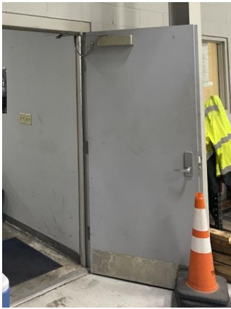
258013a 1/25/2023 Hollow-metal rated door Office to wash bay
