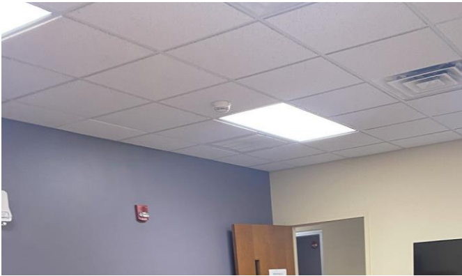
258008a 1/25/2023 Suspended acoustical tile ceiling Office area
