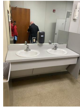
258028a 1/25/2023 Counter lavatories Restroom
