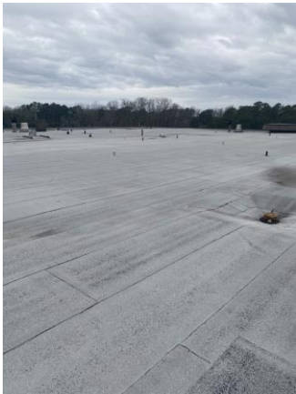
097005a 1/24/2023 Modified bitumen roof Roof
