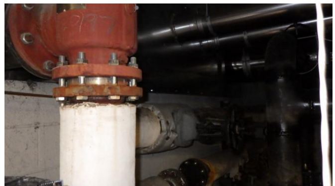
097039e 1/25/2023 Original steam utility entrance (being replaced during inspection) Mechanical 02
