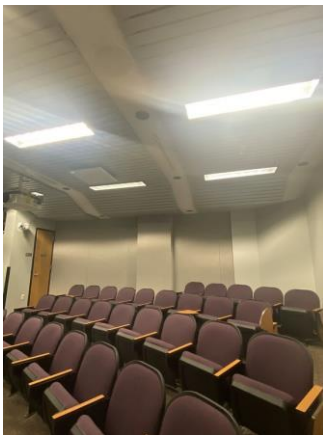
097024a 1/24/2023 Panel ceiling, finished walls, and fixed seating Classroom
