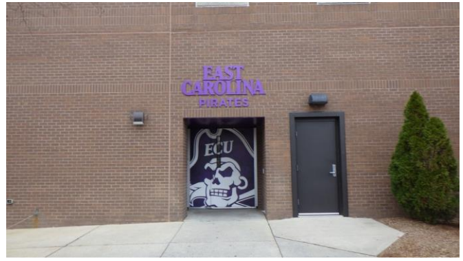
097073e 1/25/2023 LED and HID exterior wall pack light fixtures South elevation
