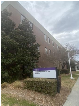
097041a 1/24/2023 Brick and stone exterior with glazing Exterior
