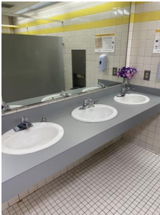
097008a 1/24/2023 Tile walls and floor and countertop lavatories Restroom
