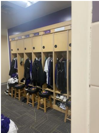
097025a 1/24/2023 ACT, finished walls, carpet, and lockers Locker Room
