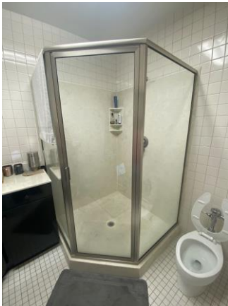
097020a 1/24/2023 Fiberglass shower stall Bathroom
