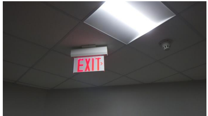
097035e 1/25/2023 Upgraded emergency exit sign Study room 237
