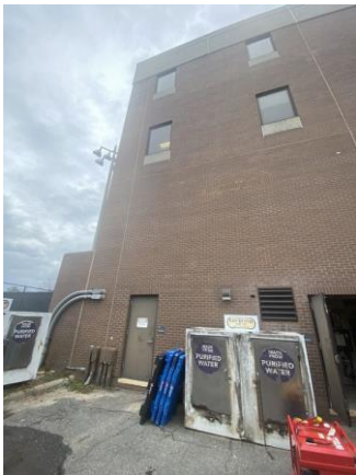
097039a 1/24/2023 Brick and stone exterior with glazing Exterior
