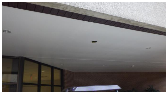
097003e 1/25/2023 Original recessed exterior light fixtures North elevation
