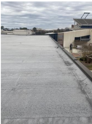
097003a 1/24/2023 Modified bitumen roof Roof
