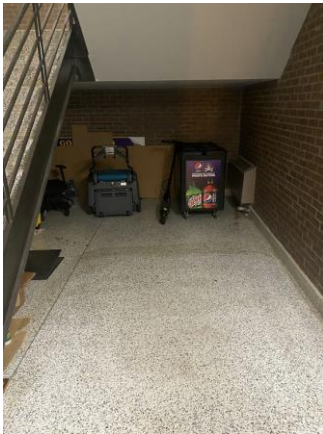
097028a 1/24/2023 Terrazzo landing, metal railings, and under stair clearance Stairwell
