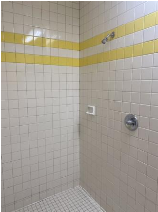
097014a 1/24/2023 Tile walls and floor and shower fixtures Bathroom
