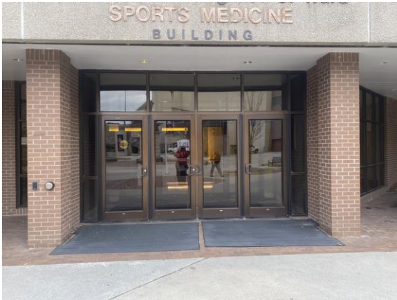
097043a 1/24/2023 Storefront door with power-operated assistance Entrance
