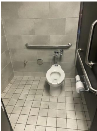
097033a 1/24/2023 Tile walls and floor and accessible water closet Restroom
