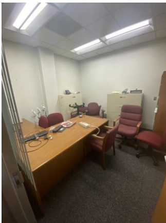
097012a 1/24/2023 ACT, finished wall, and carpet Office
