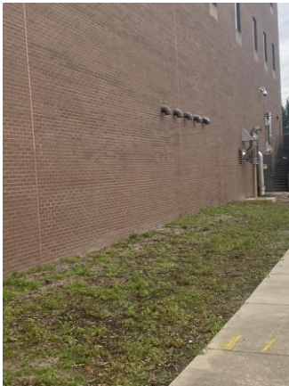
097038a 1/24/2023 Brick and stone exterior Exterior
