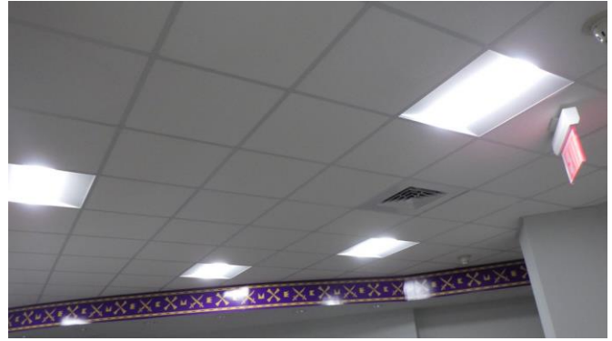
097034e 1/25/2023 Upgrade LED interior light fixtures Study room 237
