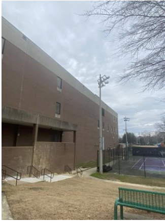
097037a 1/24/2023 Brick and stone exterior with glazing Exterior
