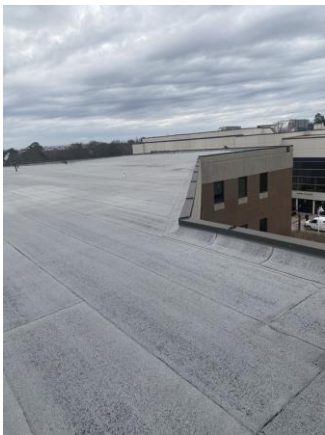
097006a 1/24/2023 Modified bitumen roof Roof
