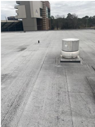
097002a 1/24/2023 Modified bitumen roof Roof
