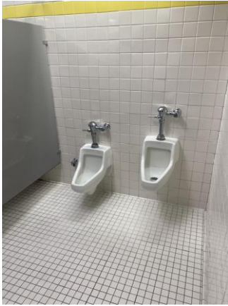
097010a 1/24/2023 Tile walls and floor and urinals Restroom
