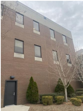
097040a 1/24/2023 Brick and stone exterior with glazing Exterior
