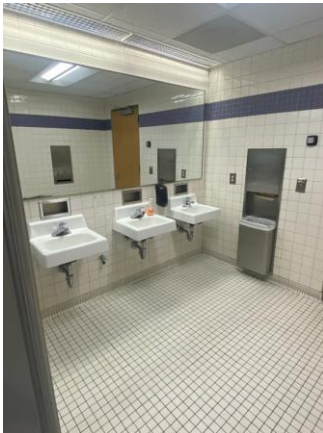
097023a 1/24/2023 Tile walls and floor and wall-hung lavatories Restroom
