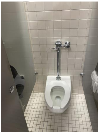
097009a 1/24/2023 Tile walls and floor and water closet Restroom
