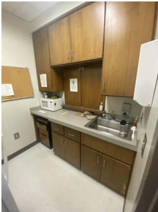
097013a 1/24/2023 ACT, finished wall, VCT, and casework with a sink Break room
