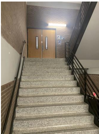
097027a 1/24/2023 Terrazzo treads and landings and metal railings Stairwell
