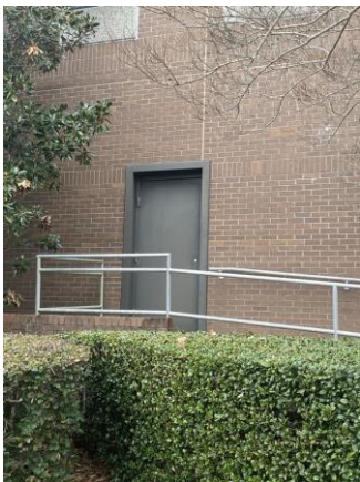
097042a 1/24/2023 Brick and stone exterior, hollow-metal door, and ramp Exterior
