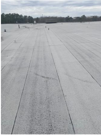
097004a 1/24/2023 Modified bitumen roof Roof
