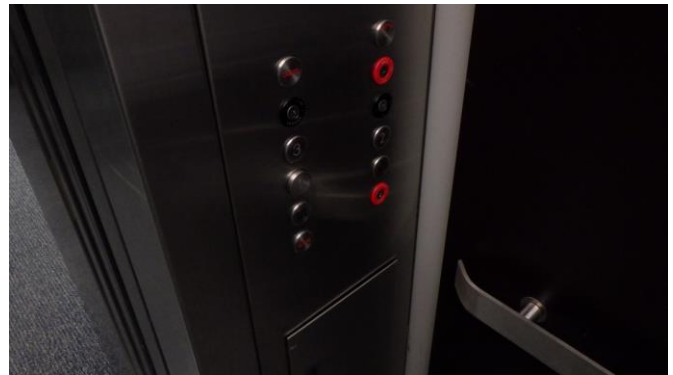
097005e 1/25/2023 Elevator controls Elevator A cab
