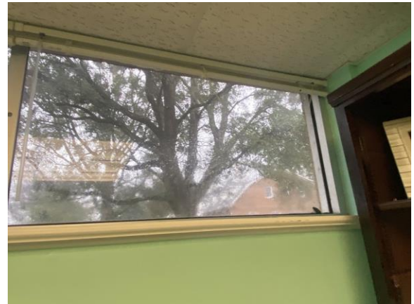
098019a 1/25/2023 Single-pane, metal-framed glazing Office
