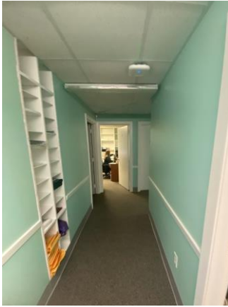
098016a 1/25/2023 Finished walls, carpet, and ACT Corridor
