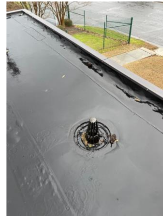
Black EPDM roof Roof
