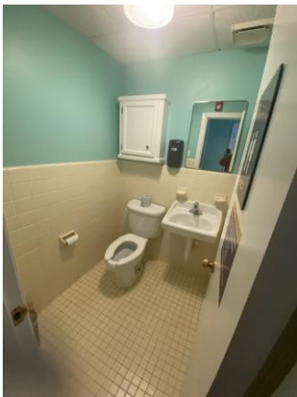
098006a 1/25/2023 Tile walls and floor, ACT, tank water closet, and wall-hung lavatory Restroom
