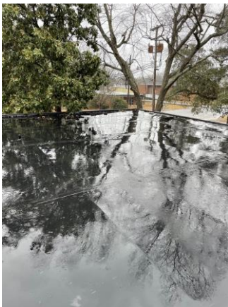
098020a 1/25/2023 Black EPDM roof Roof
