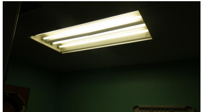
098002e 1/25/2023 Fluorescent light Storage room
