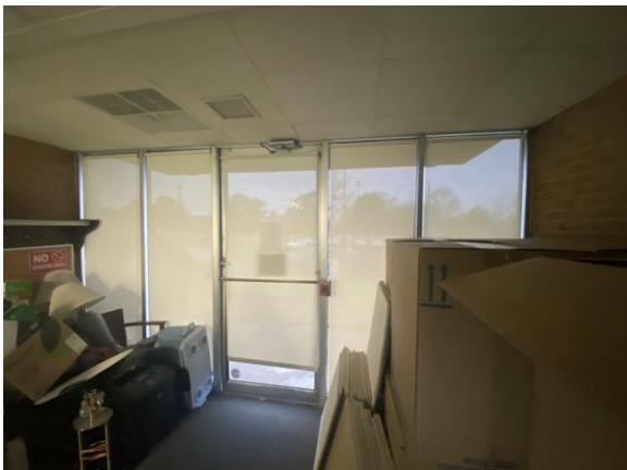
098015a 1/25/2023 ACT, brick walls, storefront glazing, and carpet Lobby
