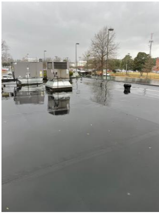
Black EPDM roof Roof
