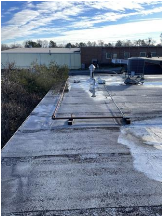
099029a 1/26/2023 Modified bitumen roof Roof
