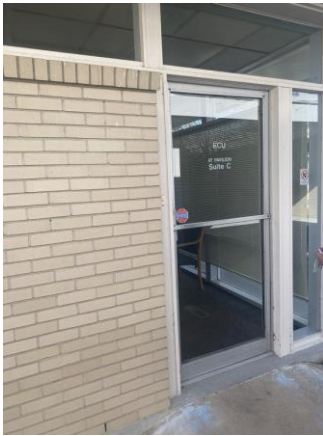
099020a 1/26/2023 Metal and glass storefront door Entrance
