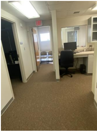
099008a 1/26/2023 Acoustical tile ceiling, carpet, painted walls Work area
