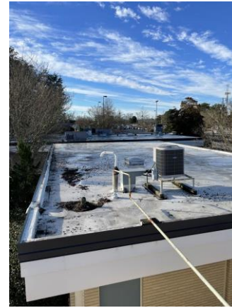
099024a 1/26/2023 EPDM roof Roof
