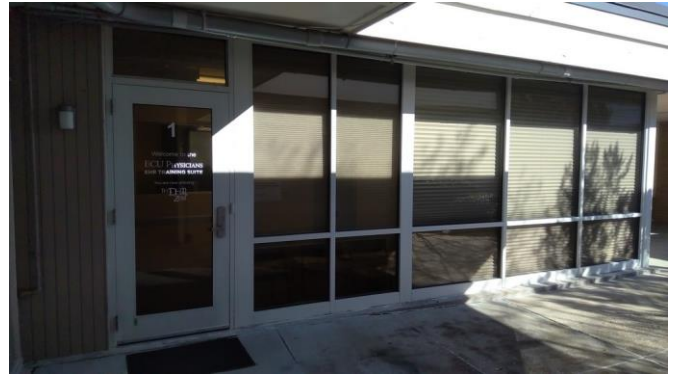
099030a 1/26/2023 Metal-framed doors and glazing Exterior
