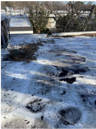
099027a 1/26/2023 EPDM roof Roof
