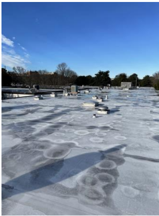
099021a 1/26/2023 EPDM roof Roof
