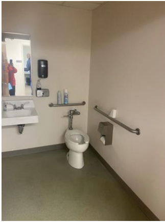
099004a 1/26/2023 Sheet vinyl, painted walls, acoustical tile ceiling, lavatory, accessible water closet Restroom
