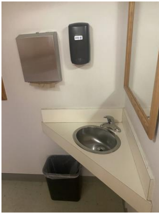
099017a 1/26/2023 Painted wall, vinyl tile floor, stainless steel lavatory Restroom
