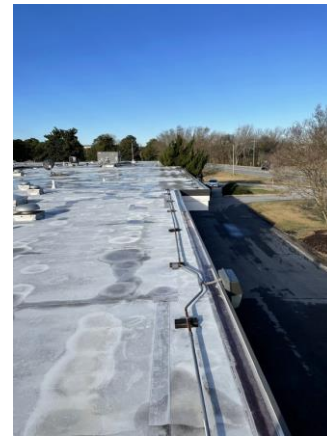
099022a 1/26/2023 EPDM roof Roof
