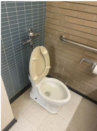
099009a 1/26/2023 Ceramic tile wall, vinyl tile floor, toilet Restroom
