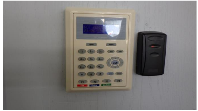
099019e 1/26/2023 HVAC thermostat General office area
