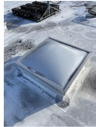
099026a 1/26/2023 Skylight Roof
