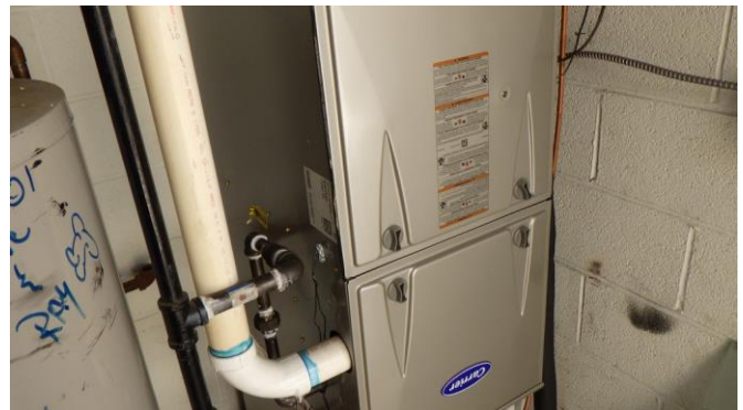
HVAC indoor fan unit Suite mechanical room
