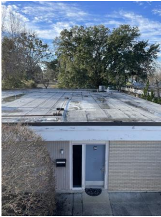
099023a 1/26/2023 Modified bitumen roof, brick exterior Exterior
