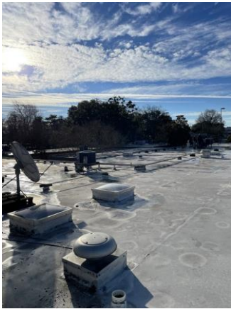
099025a 1/26/2023 EPDM roof with skylight Roof
