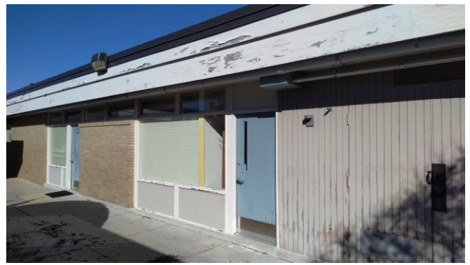
099032a 1/26/2023 Brick exterior, hollow metal door, glazing, weathered paneling Exterior
