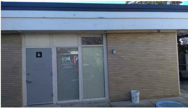
099031a 1/26/2023 Brick exterior, hollow metal door, glazing Exterior
