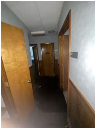
117008a 1/26/2023 Painted hard surface walls and standard doors Corridor
