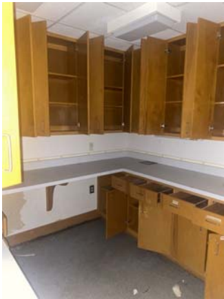
117010a 1/26/2023 Wood casework Reception area
