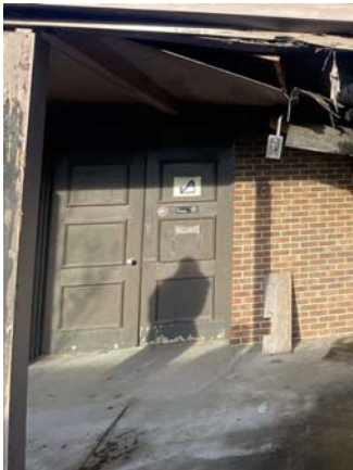
117011a 1/26/2023 Wood panel exterior doors Main entrance
