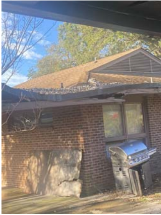
117001a 1/26/2023 Asphalt shingle roofing Main roof
