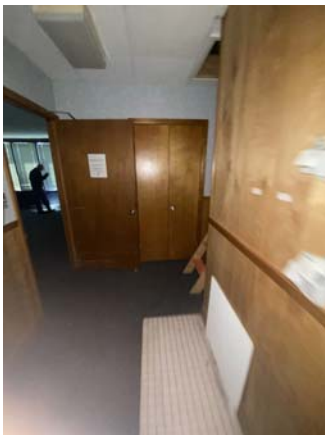
117006a 1/26/2023 Painted hard surface ceiling Common area
