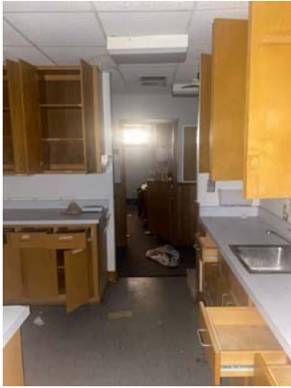
117004a 1/26/2023 Welded seam vinyl Common area
